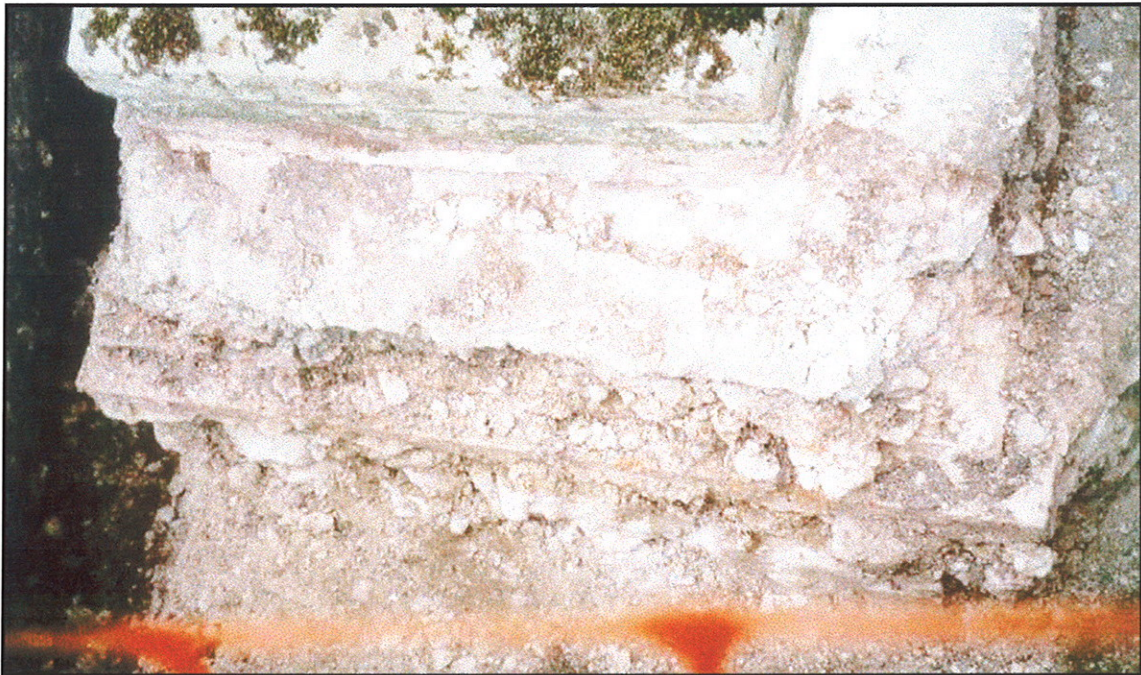
Photo 13: North east buttress of the north transept wall.
