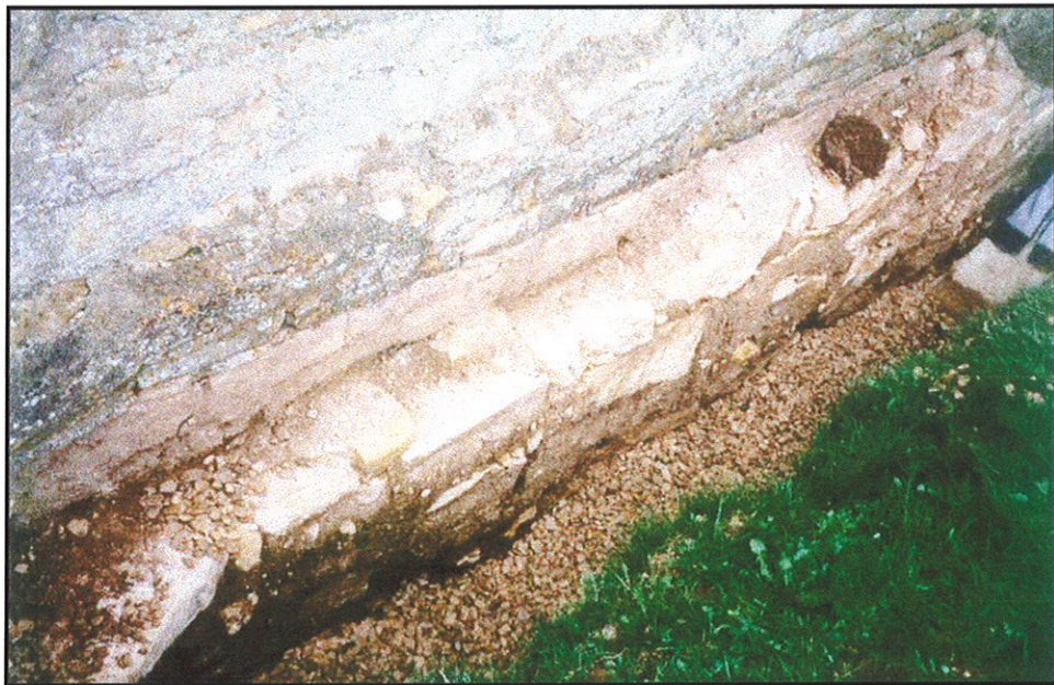
Photo 3: West side of south porch.
