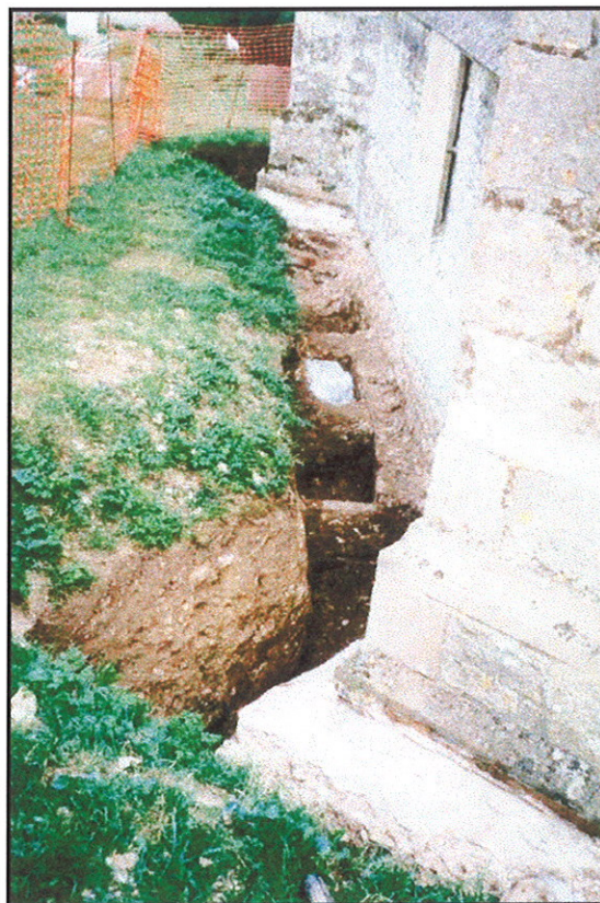
Photo 14 & 15: Foundations of north transept wall, revealing a brick burial vault.
