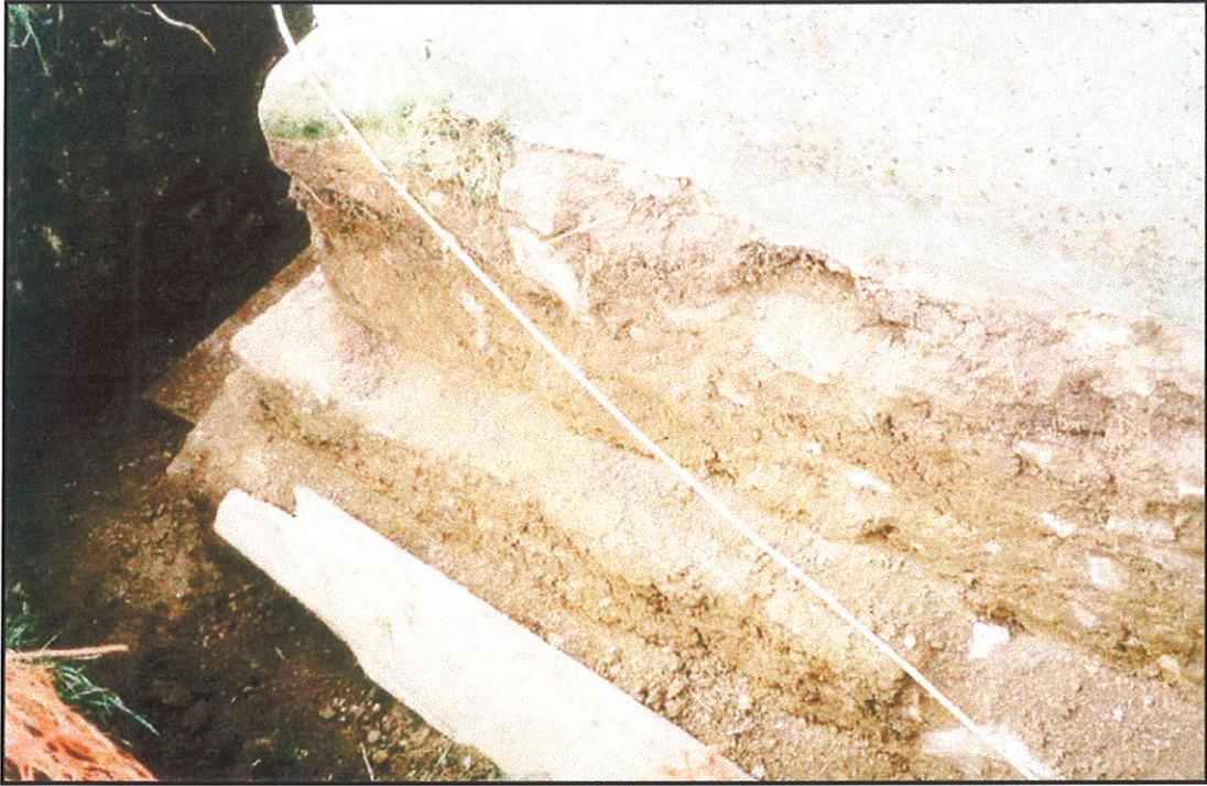
Photo 12: South end of east wall of chancel.
