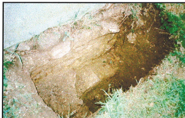
Photo 11: Foundations exposed to the rear of the chancel.
