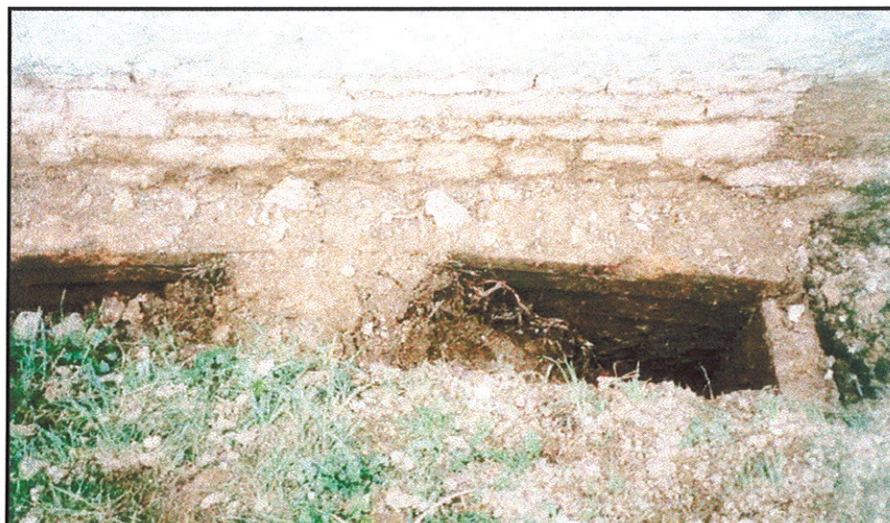
Photo 16: Detail of brick vault by north transept wall.
