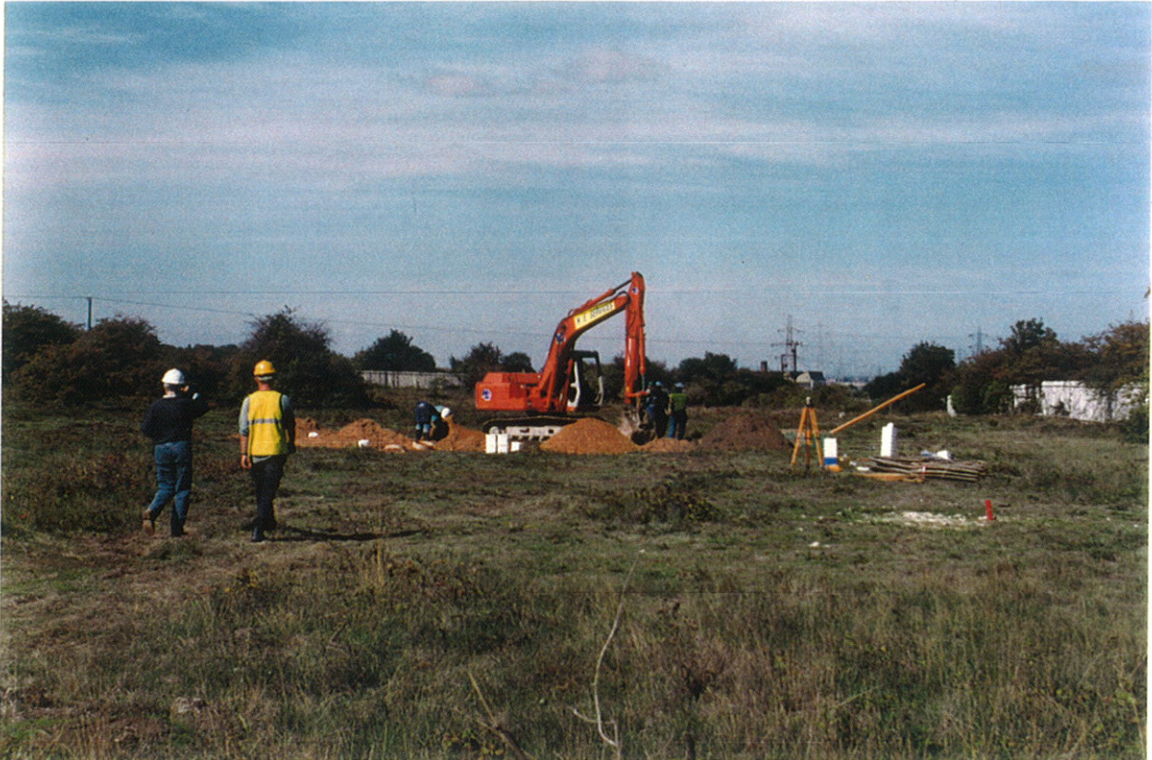
Plate 3. Excavation of Test Pit ARC 2003 TP.
