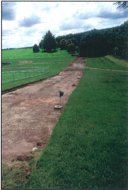
Plate 19 - Turf removal completed on north to south aligned western path of South Parterre garden. Looking south.
