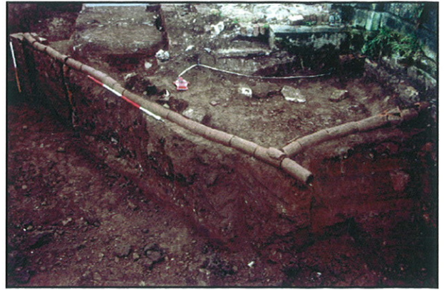
Plate 44 - Trench 20, drainage exposed during excavation of new pumphouse. Looking north.
