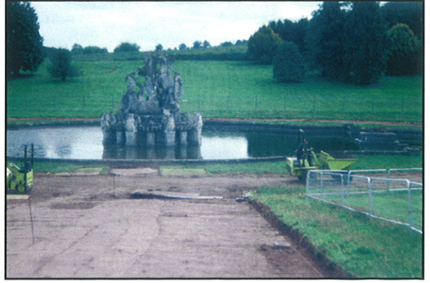
Plate 26 - Central path and fountain path de-turfed. Looking south.
