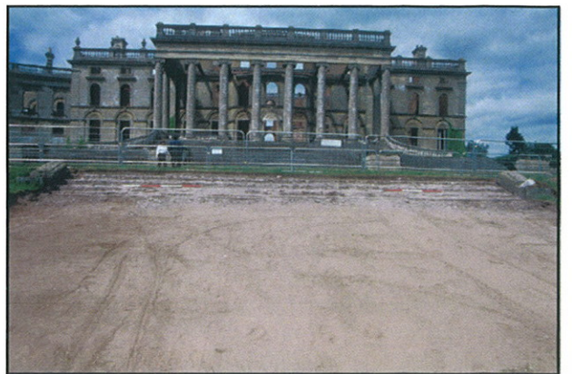
Plate 22 - Trench 5, surviving step foundations of S4 with former path width re-exposed. Looking north.
