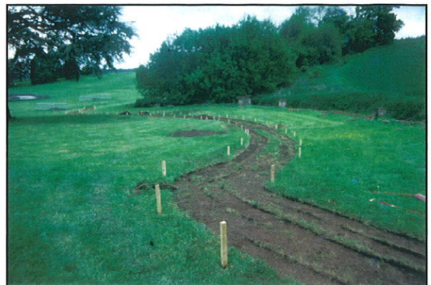
Plate 4 - Turf stripping commenced on new disabled access path at north west corner of South Parterre garden. Looking south east.
