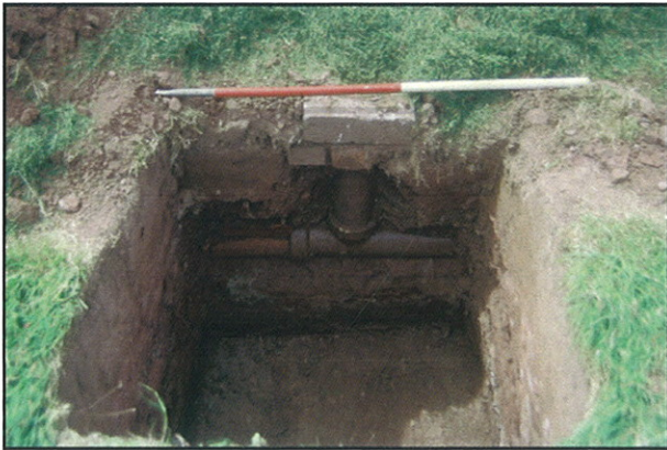
Plate 27 - Trench 11, trial pit excavated by garden contractor to examine drainage. Looking south west.
