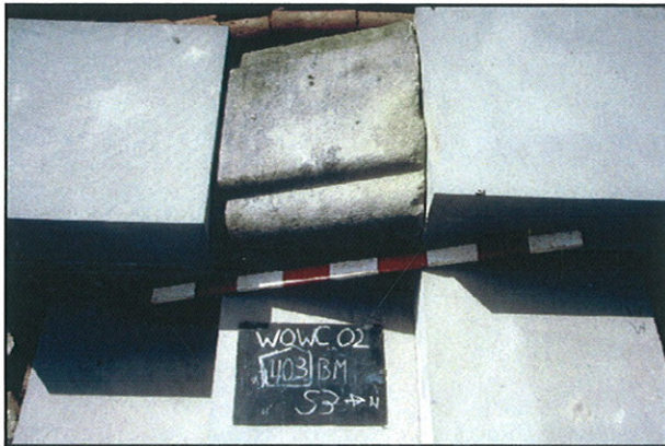
Plate 39 - Trench 3, reinstated stonework on steps S3. Looking west.
