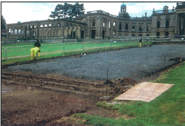
Plate 29 - Trench 6, surviving step foundations S5 with central path being prepared for re-surfacing. Looking north west.
