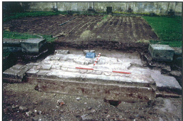
Plate 48 - Trench 15, excavation of step foundations S1 after brick ramp removed. Looking north.
