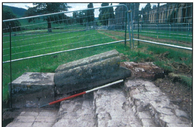
Plate 24 - Trench 5, detail of surviving stringer S4. Looking west.
