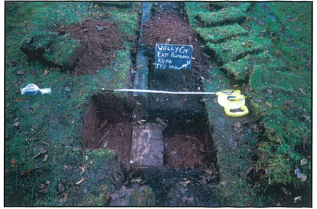
Plate 68 - Trial Pit 1 (East Parterre), examination of construction and survival of bed kerbing in east parterre. Looking north west.
