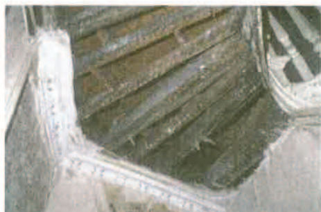
13 Moulding and underside of treaders
