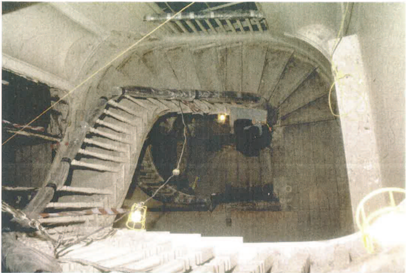
12 Stairs in-situ, looking down from Second floor
