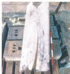
15 Curved string element, splitting after dismantling
