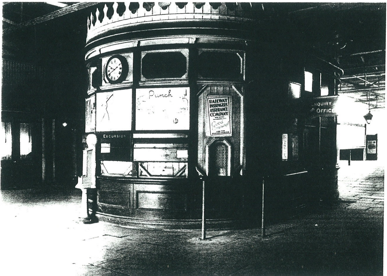
Plate 13 The free-standing Booking Office from the south-east, 1940? It is said that this was originally used at the Great Exhibition of 1851 and it is worth noting that the panelling and the ornate crests exactly copy elements used in both the Crystal Palace and the Oxford Station. This structure is absent the 1876 OS plan and the 1903 tracing of the station which show the Booking Office as being a room in the eastern wing. This structure is visible however, in the early un-dated photograph of the station interior (plate 3). (NRM)
