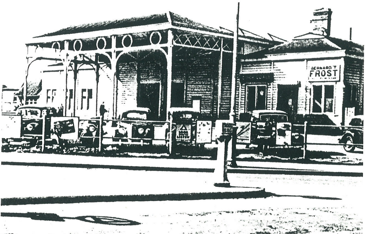
Plate 19 A similar view, also taken in 1951, showing more clearly the replacement lattice girders and rolled steel column supporting them. ( Dr. R. Preston Hendry & R. Powell Hendry )
