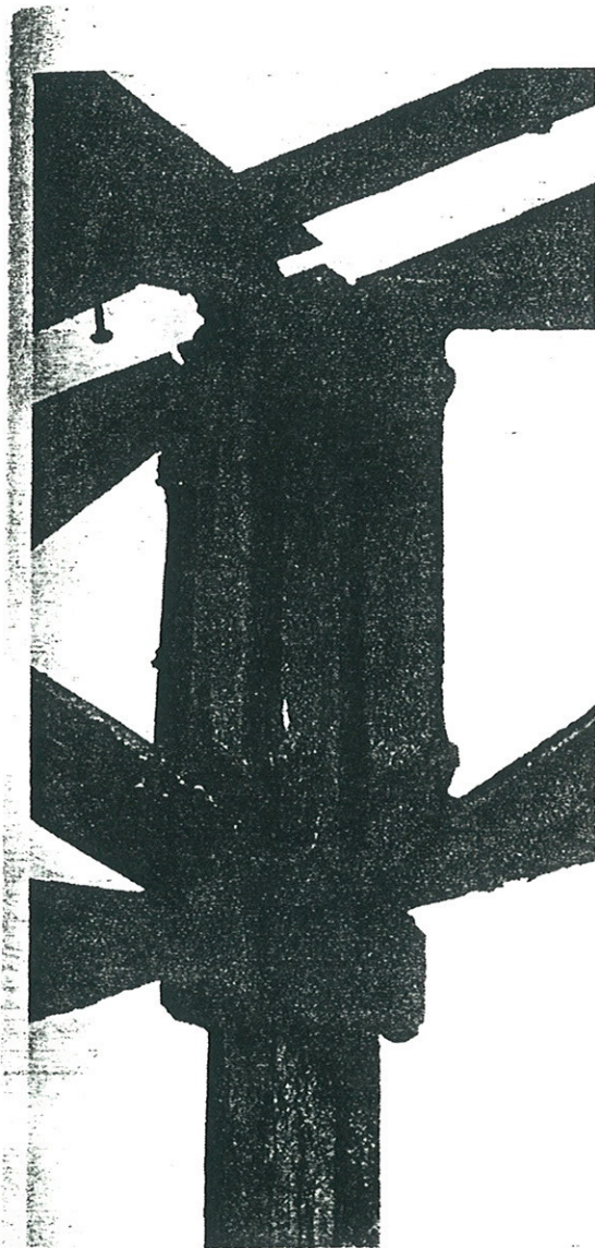
Fig 3. Beam to column fixing at Oxford Station
