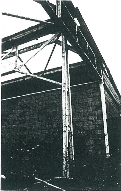
Plate 38 Rail-built C5 type column supporting inserted T2 type truss.
