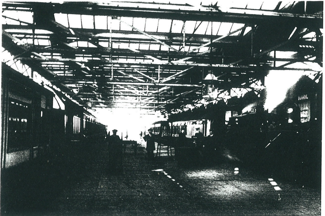
Plate 5 The interior of the trainshed looking north, 1914. The transverse ridge-and-furrow roofing is clearly shown extending the full length of the trainshed. Note the raised platform level ( Oxford County Libraries )
