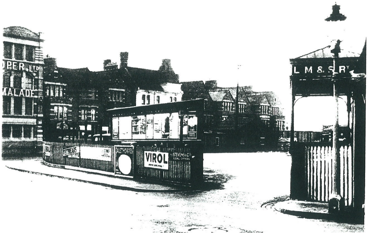
Plate 8 The forecourt and porte-cochère of the LMS station. This, and the following three photographs are dated to early 1936 by the flag on Victoria Buildings opposite being flown at half mast, marking the death of George V in January of that year. (BR/OPC)
