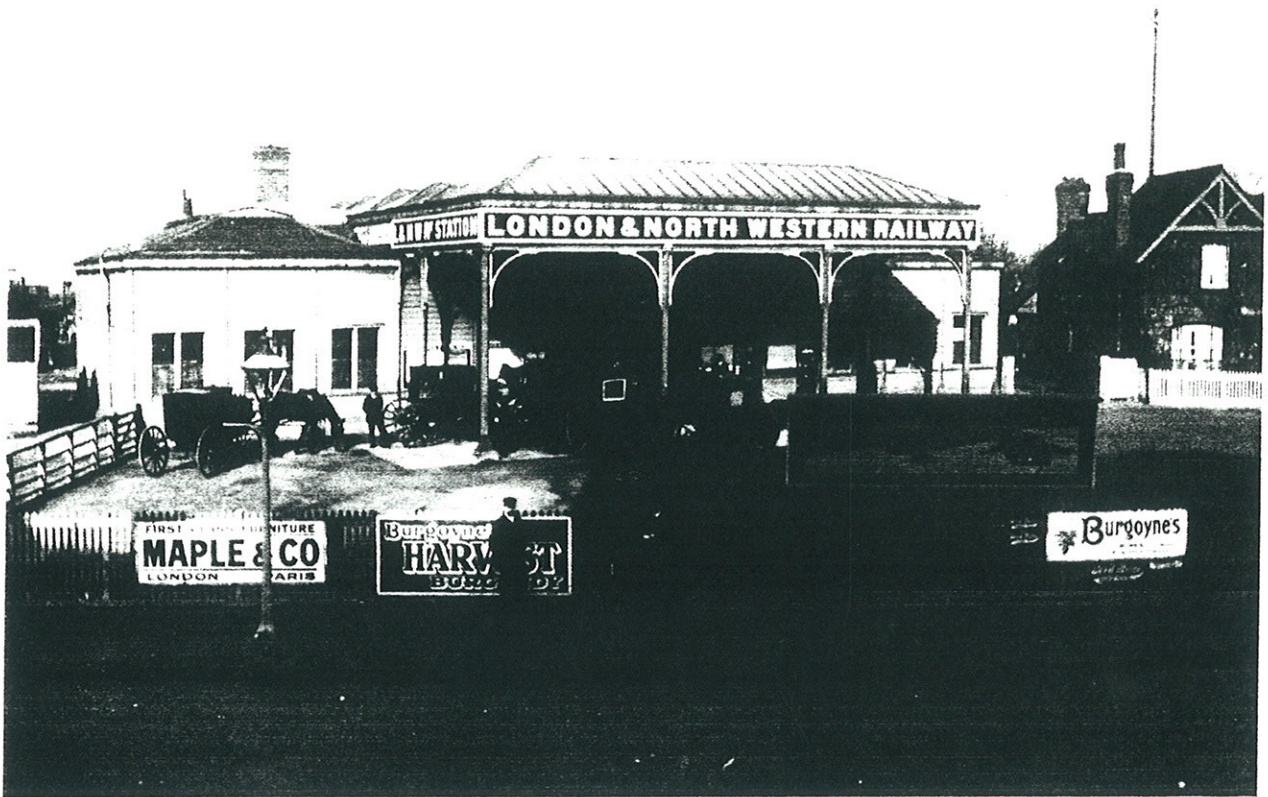
Plate 4 The exterior of the LMS station in 1914 showing the porte-cochère. Note the later style of transverse ridge-and-furrow roof over the concourse/trainshed and the timber cladding of the side extending to ground level. ( Oxford County Libraries )
