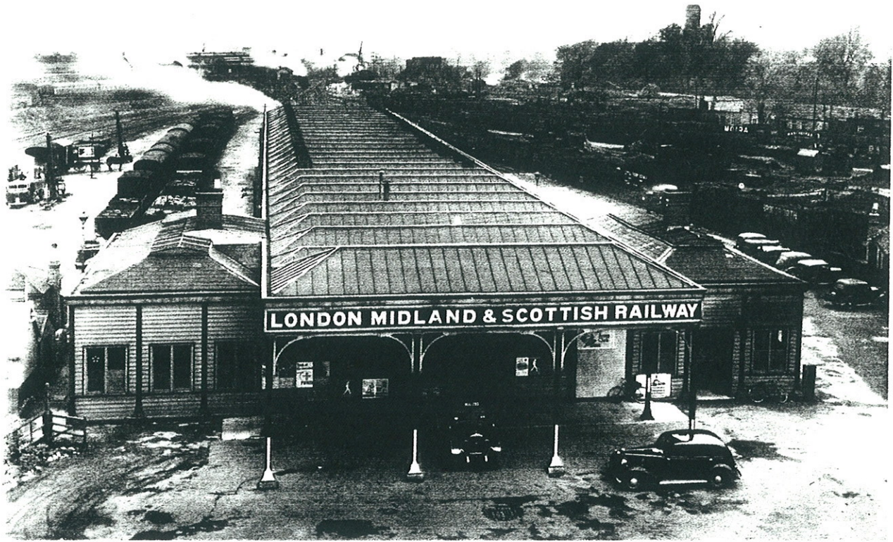
Plate 12 The LMS station, 1st May 1940, clearly showing clearly the roofs of both the trainshed etc as well as of the flanking wings. This, and the following three photographs, appear to have all been taken on the same day. (NRM)
