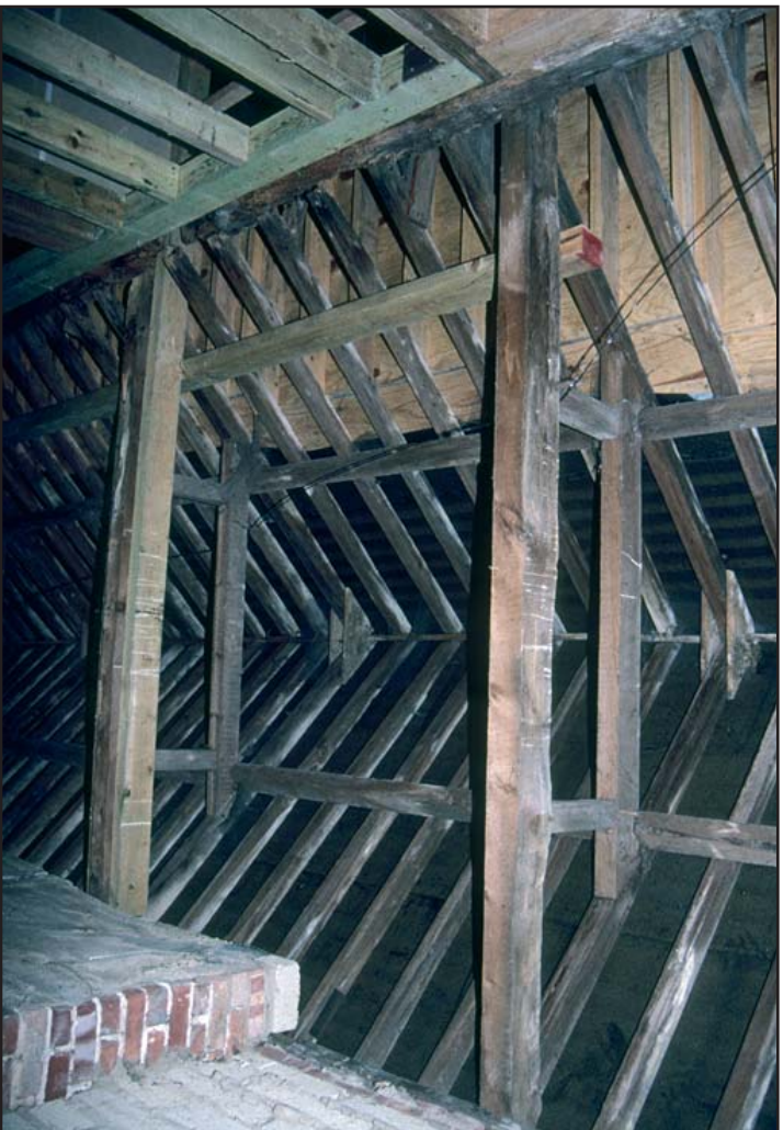
Plate 24: Queen post trusses above extension (F4)
