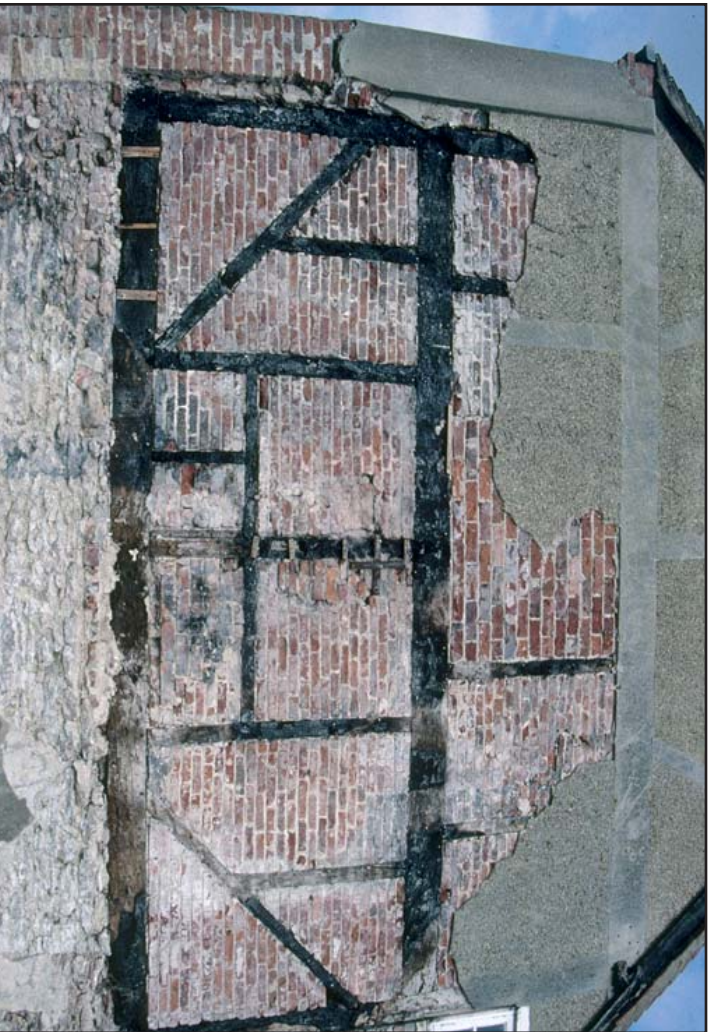
Plate 7: Primary framing in east elevation
