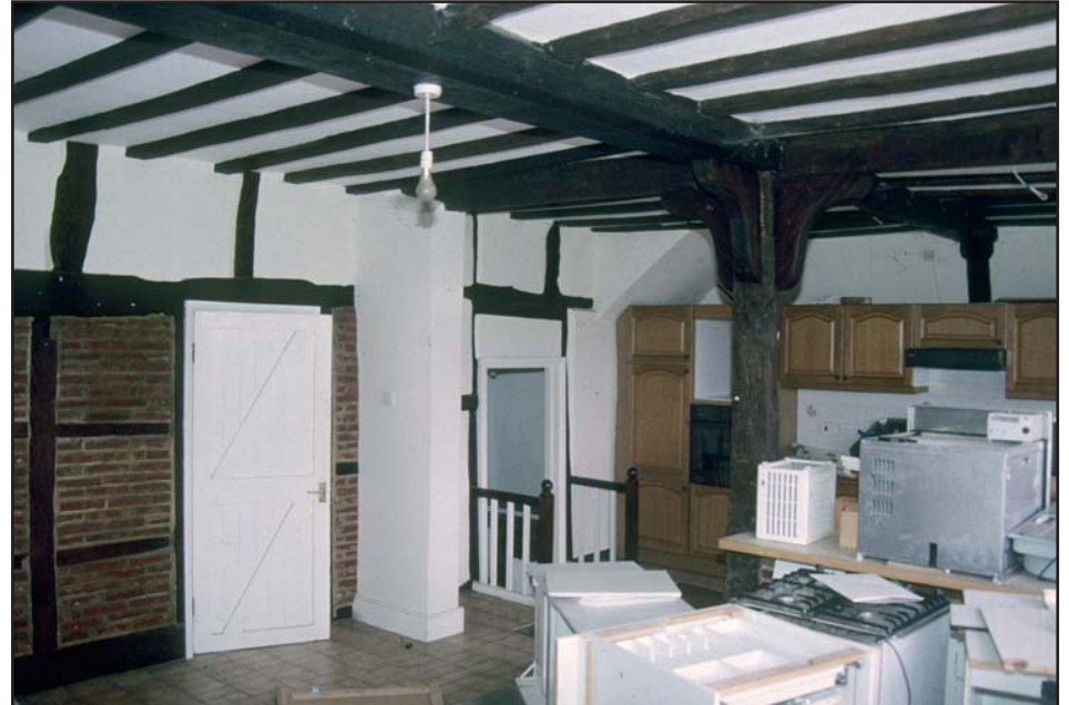
Plate 13: Kitchen (G7) in primary house
