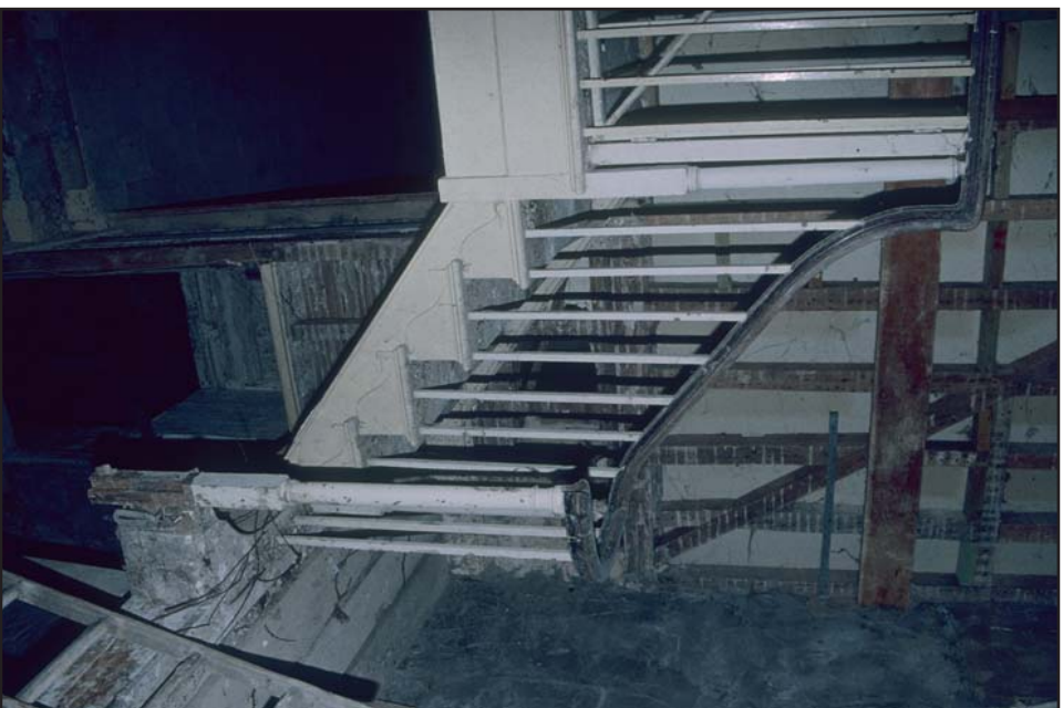
Plate 23: Staircase in Georgian extension (F4)
