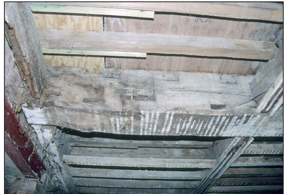
Plate 15: Very large reused joist in G1
