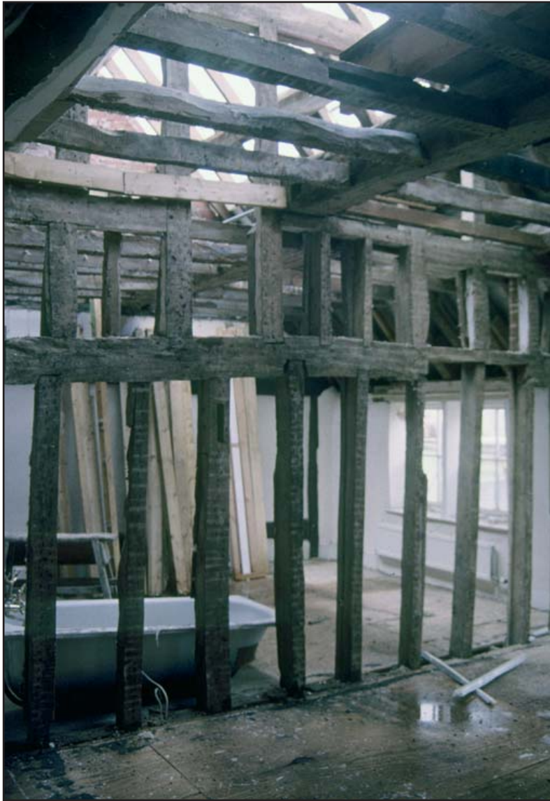
Plate 17: Cross Frame II at first floor looking east
