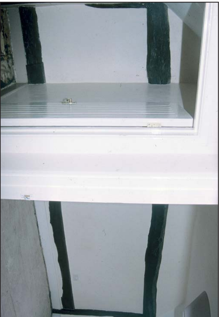
Plate 20: Tie and rail in East wall (Cross Frame I)
