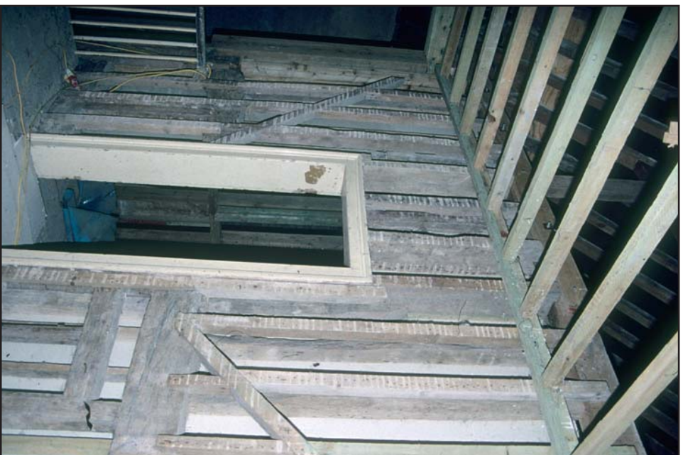
Plate 21: Secondary door between F3 and F4. Truncates primary tie-beam
