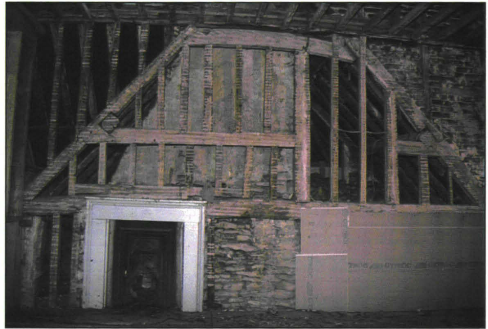
Plate 18: Primary truss and chimney in east wall of F5
