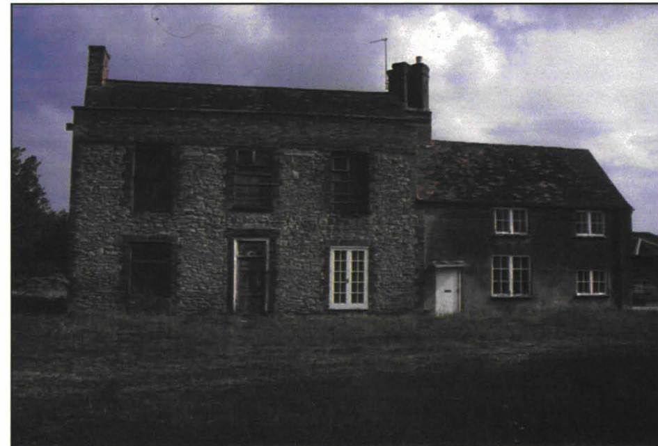
Plate 4: Front (south) elevation, original house to right.
