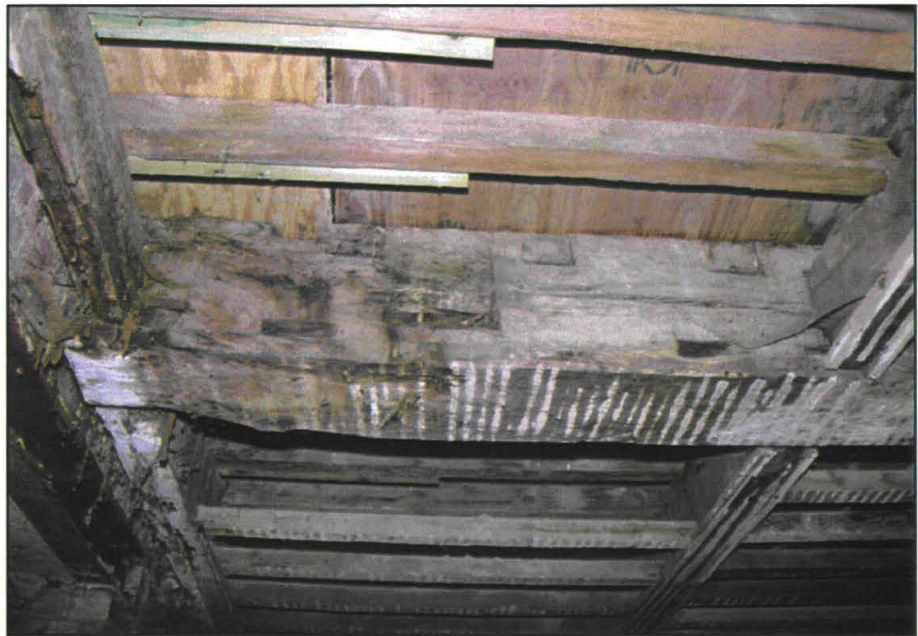
Plate 15: Very large reused joist in G1
