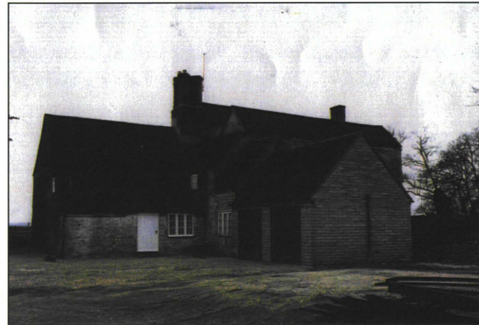
Plate 2: View from NE before demolition of garage
