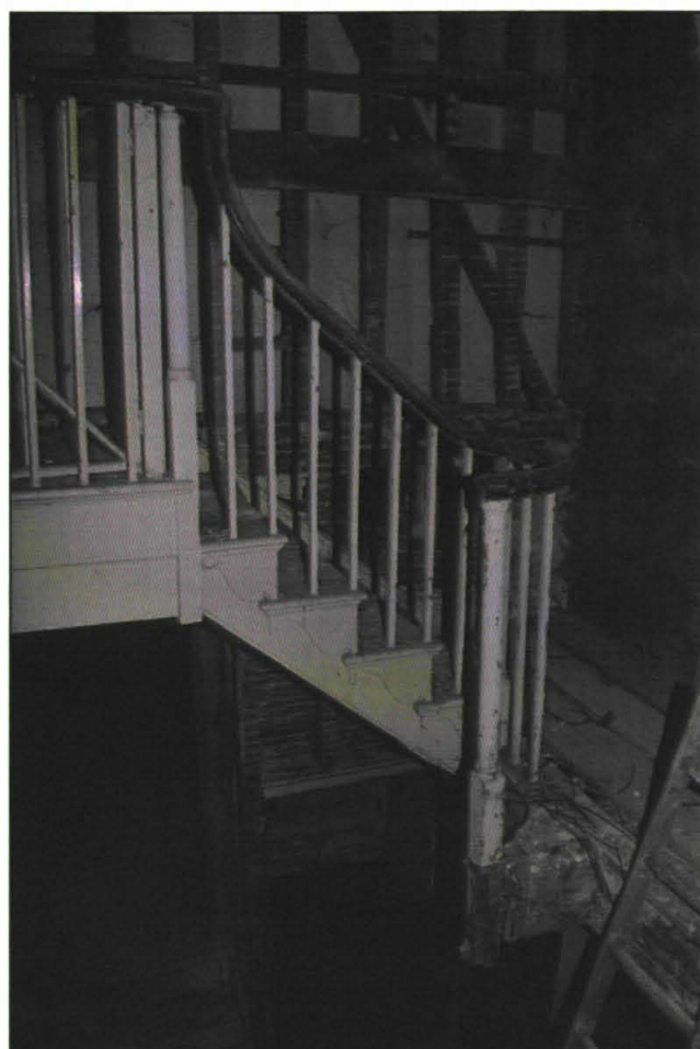
Plate 23: Staircase in Georgian extension (F4)
