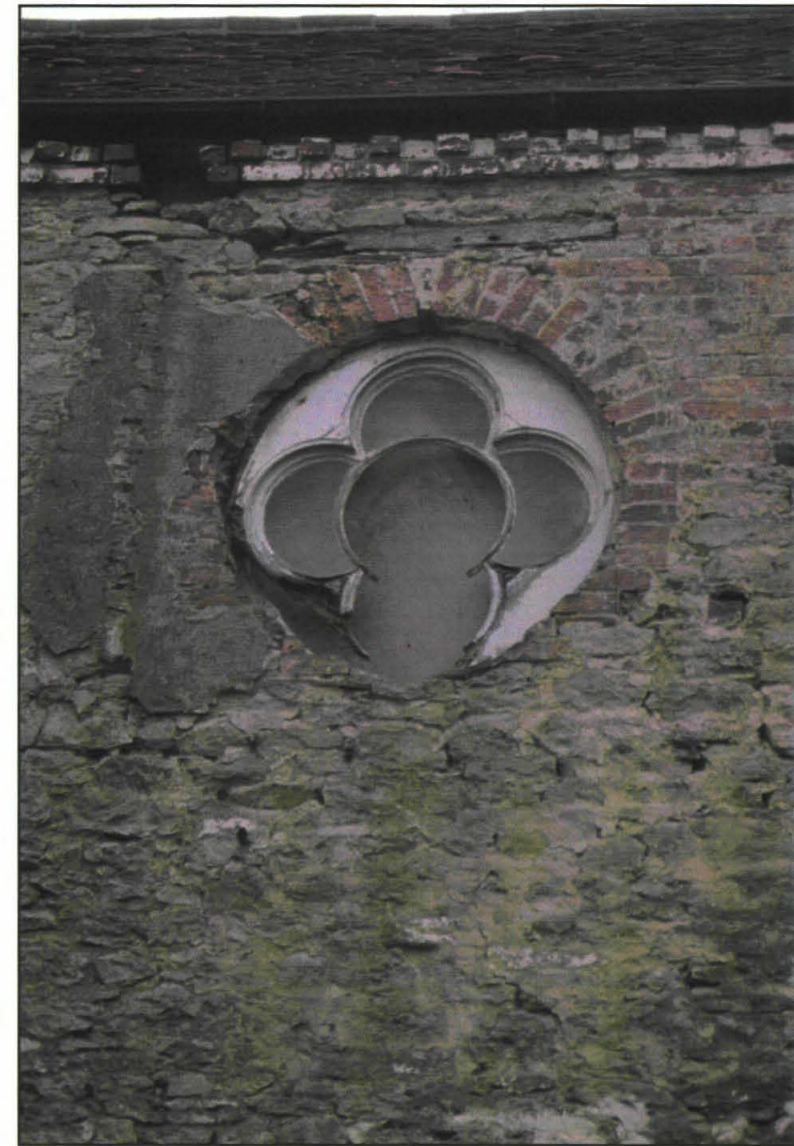
Plate 10: Bulls eye window in north elevation
