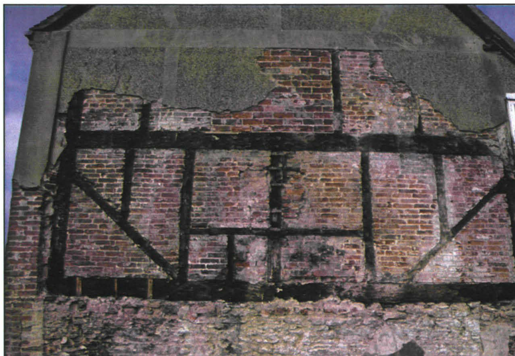
Plate 7: Primary framing in east elevation
