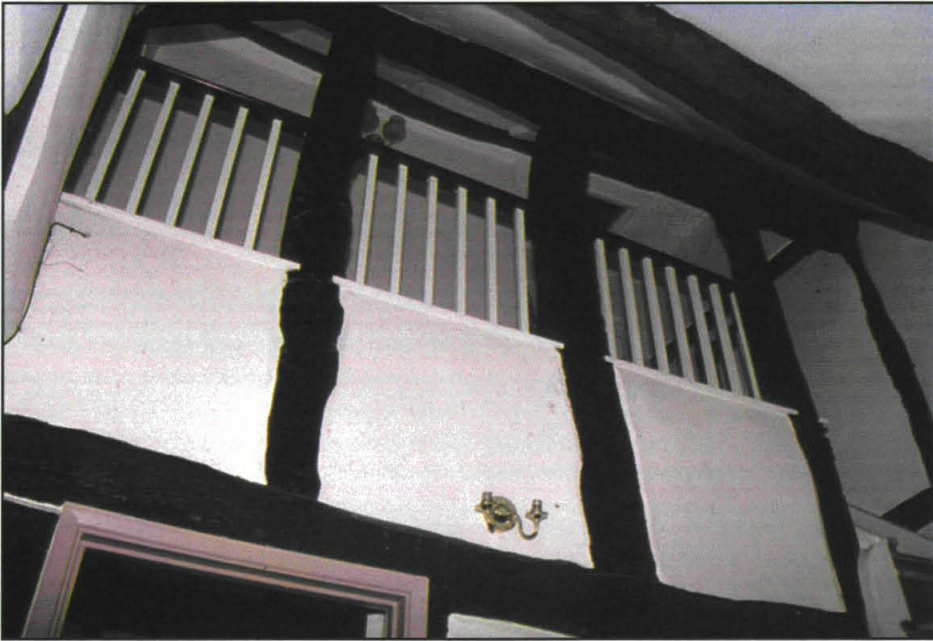
Plate 14: Primary studs in north wall of house (G8)
