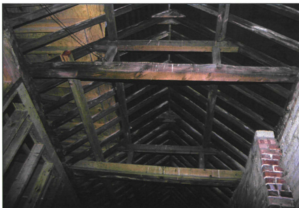
Plate 24: Queen post trusses above extension (F4)
