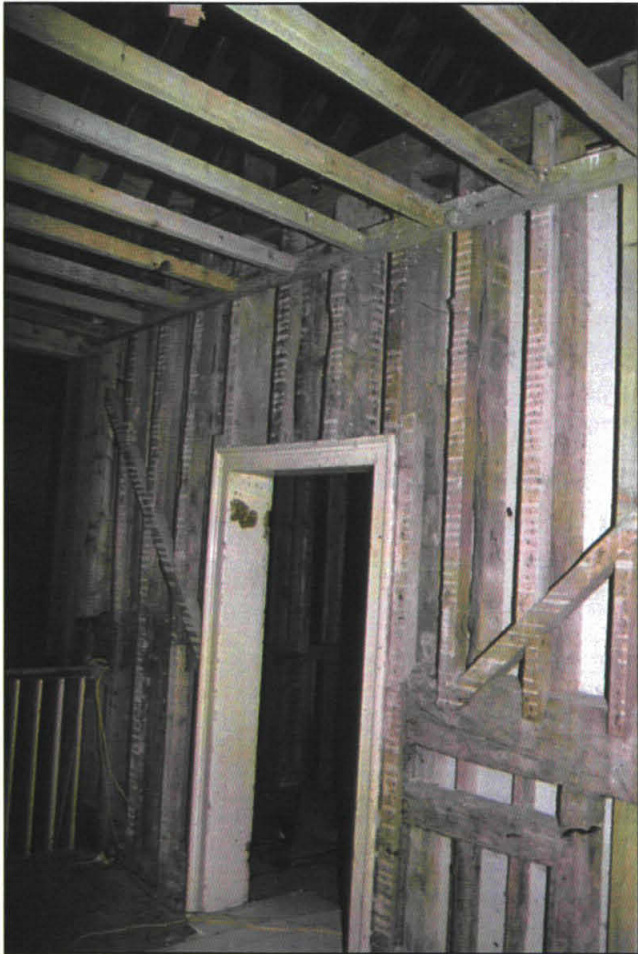
Plate 21: Secondary door between F3 and F4. Truncates primary tie-beam
