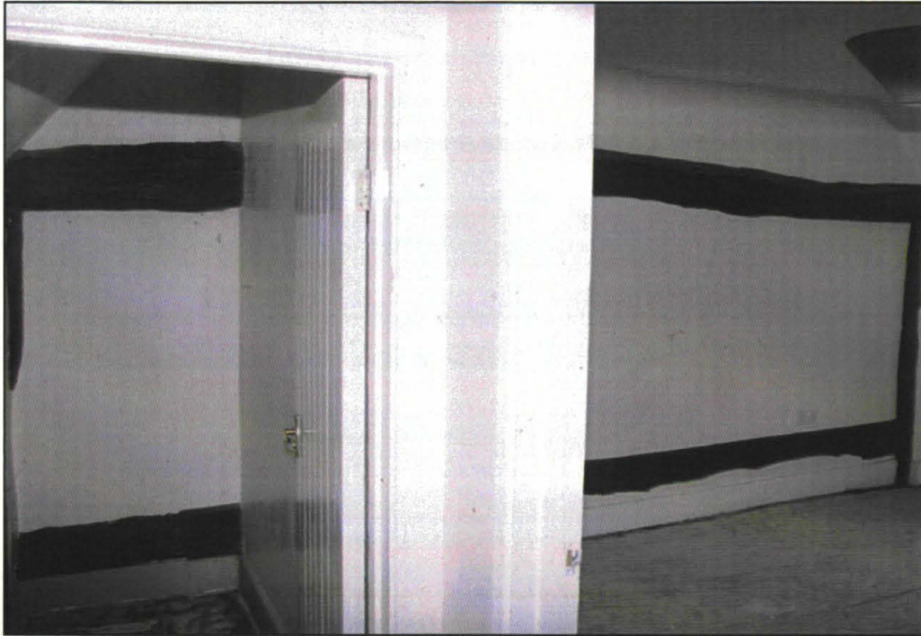
Plate 20: Tie and rail in East wall (Cross Frame I)
