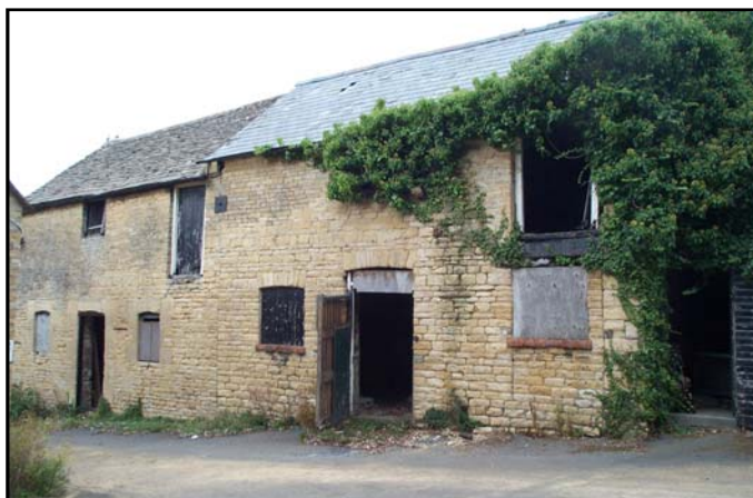
Plate 5: Stabling at the rear of the inn
