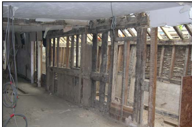
Plate 16: The North Range gallery, east end (interior)
