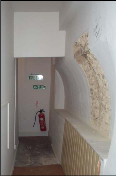
Plate 7: Bowed wall in the South Range
