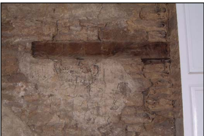
Plate 12: The West Range, south room Wall painting under panelling 2003
