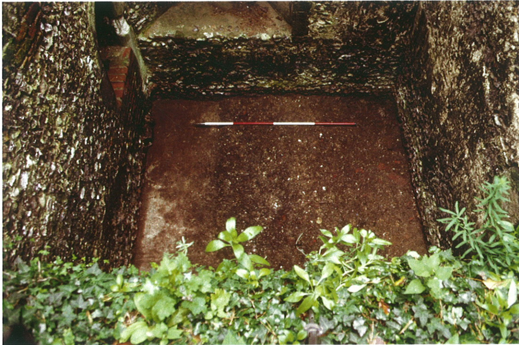
Plate 4: Concrete 13 and rough surface 10 within tower
