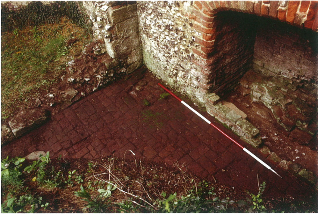
Plate 1: Fireplace and brick floor 7
