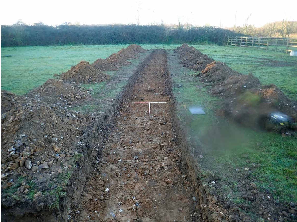
Plate 4: Trench 80 (west part) looking south-west
