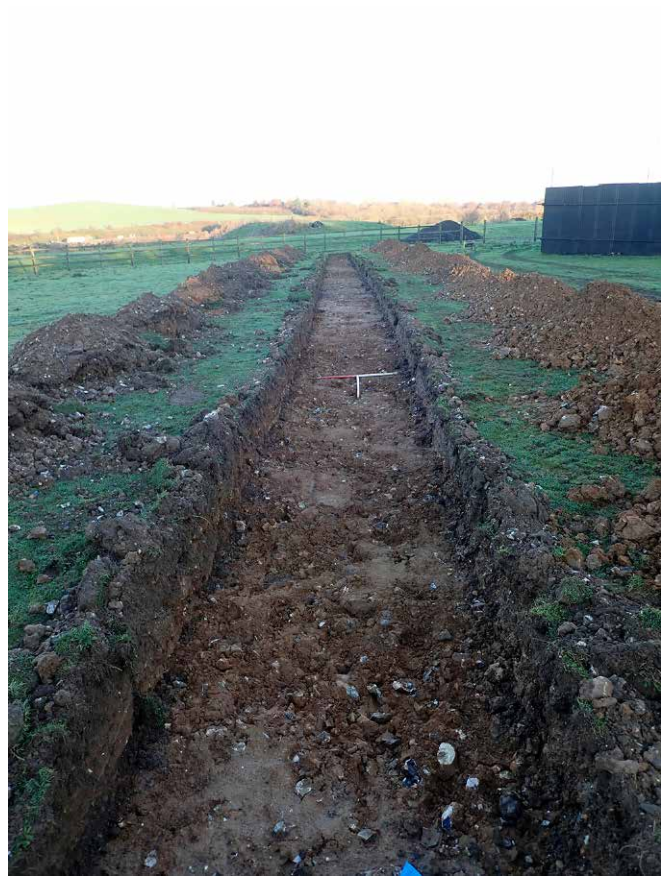
Plate 1: Trench 79 stripped, looking SSE
