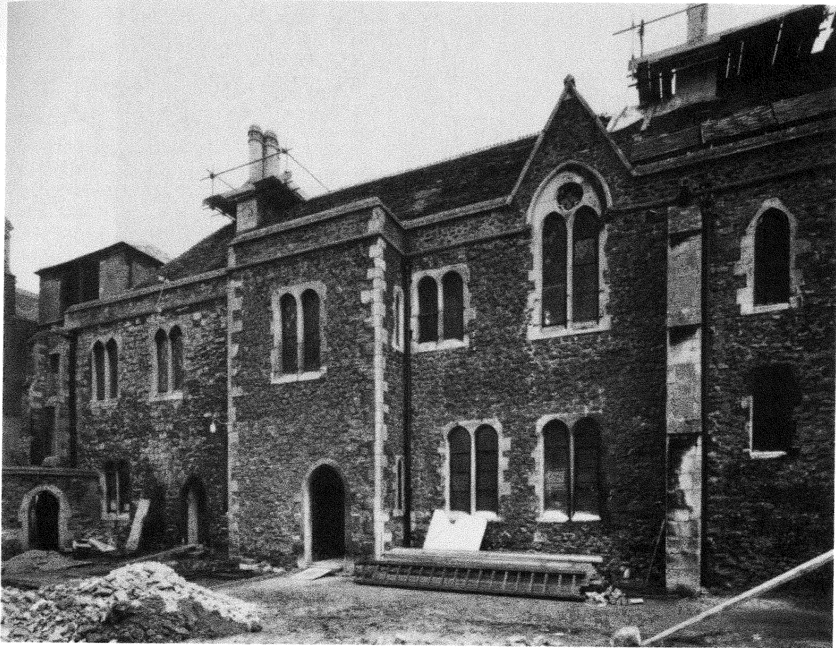
Plate 1. North Range, south elevation. (Crown copyright)
