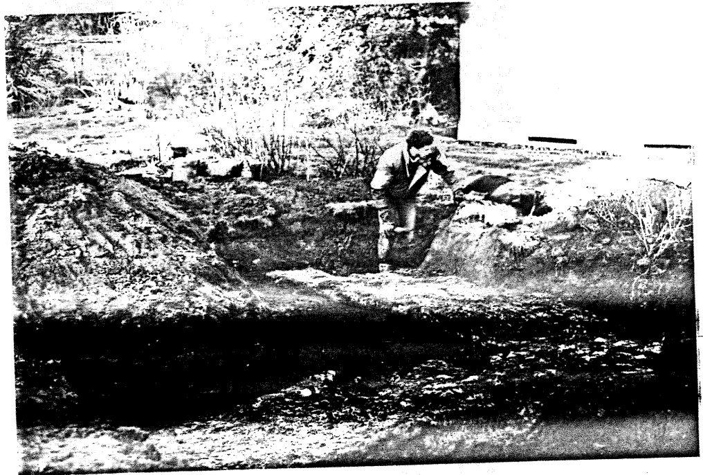
Plate V South-east corner of building.1 (south)
