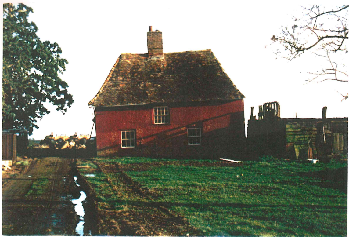
West Facing External Wall of Ryder's farm And 17 th Century Barn (by T.Malim, 1993)
