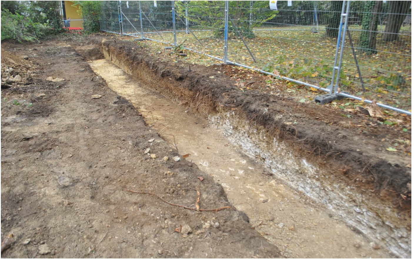
Plate 5: Shot of service trench with possible hedge line linear feature
