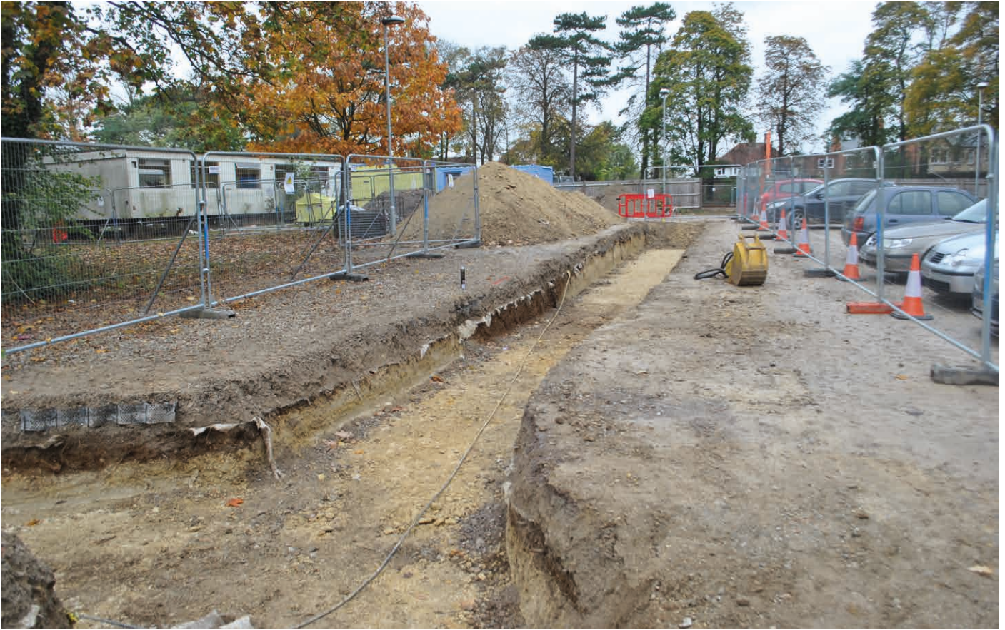
Plate 3: Shot of service trench with large feature
