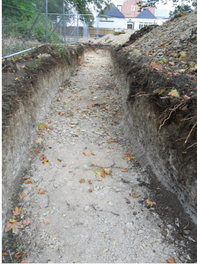
Plate 7: Base of service trench connecting the substation
