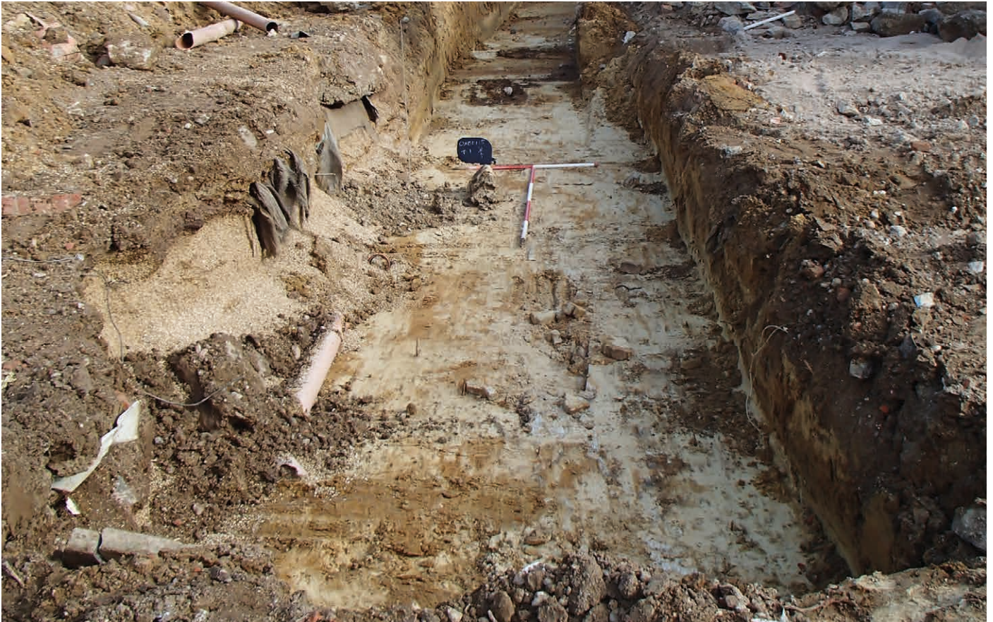
Plate 1: Overall shot of Trench 1
