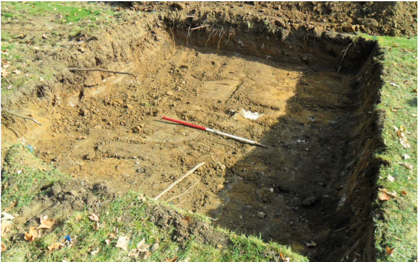
Plate 6: Foundation excavation of the substation
