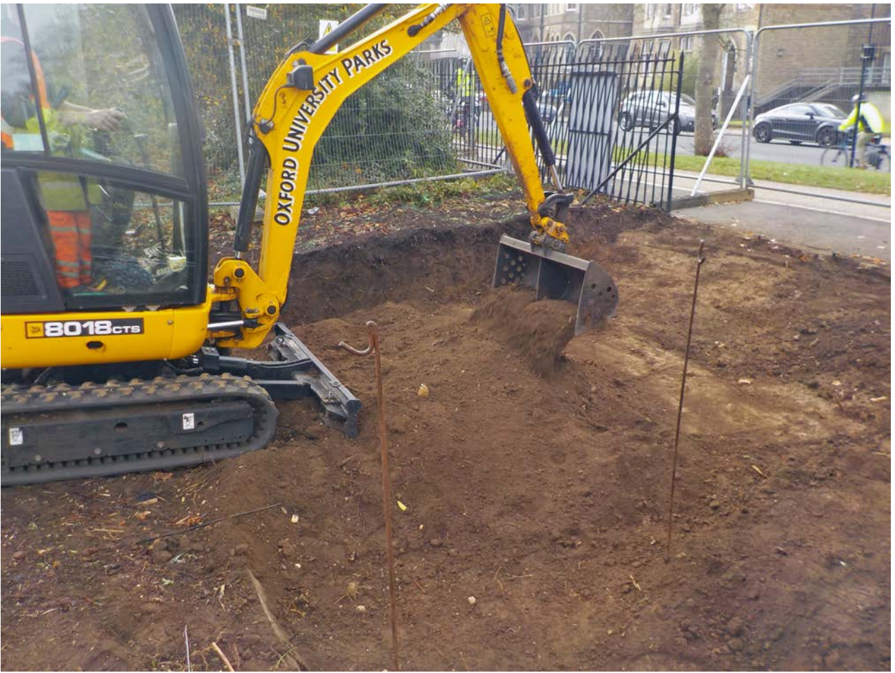
Plate 1: Ground reduction in progress, looking south-west
