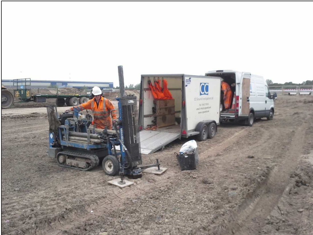
Plate 11: Borehole sampling of the Middle Wentlooge Formation
