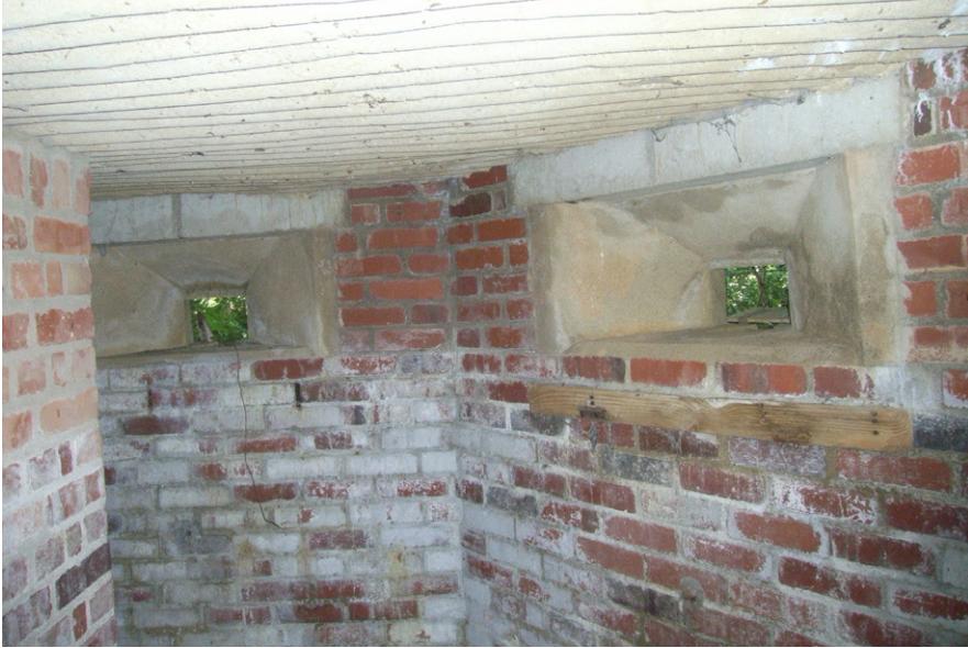
Plate 5: Type 24 pillbox, internal view showing anti-ricochet wall to left and embrasures to right (with hatch visible) (OA142)
