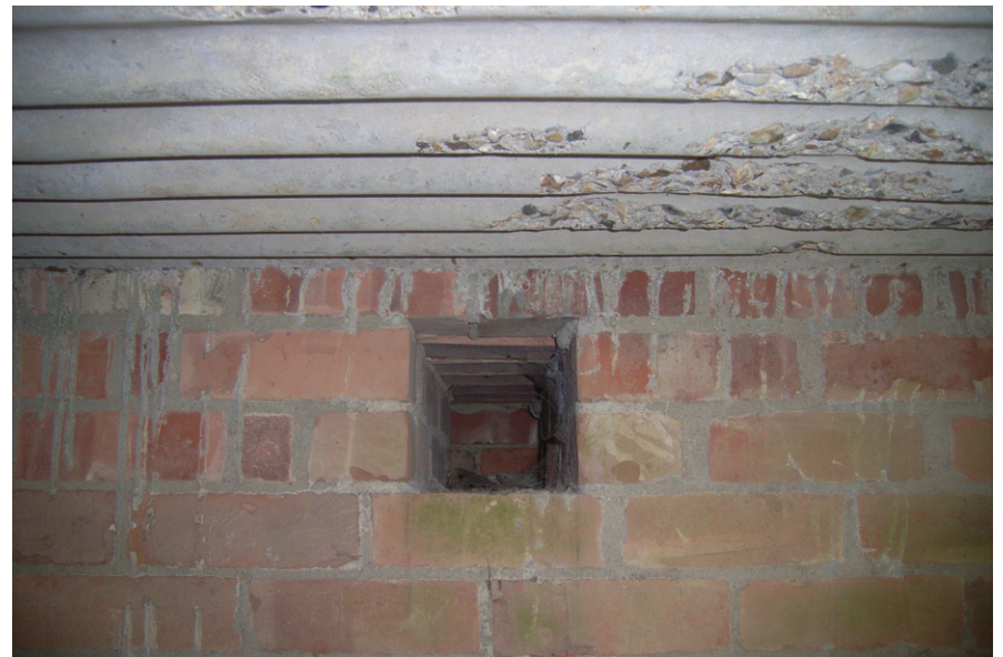
Plate 12: Vickers gun emplacement, air vent in rear wall (OA144)
