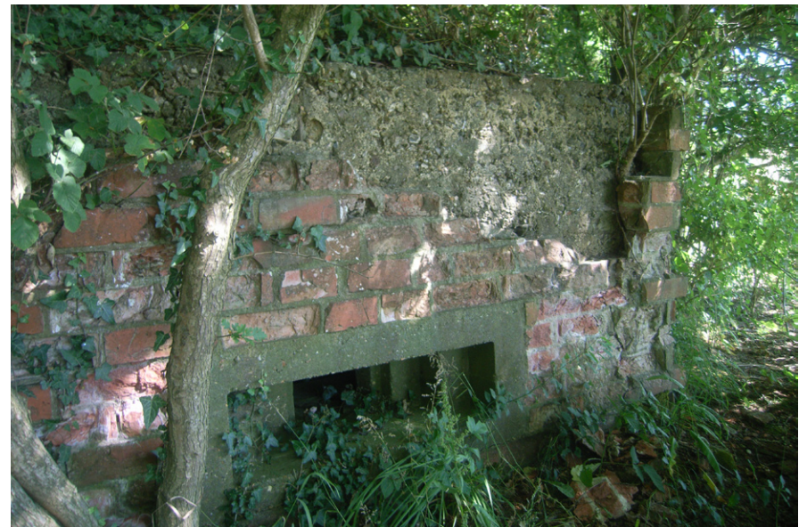
Plate 16: Type 24 pillbox, showing exposed concrete core (OA136)
