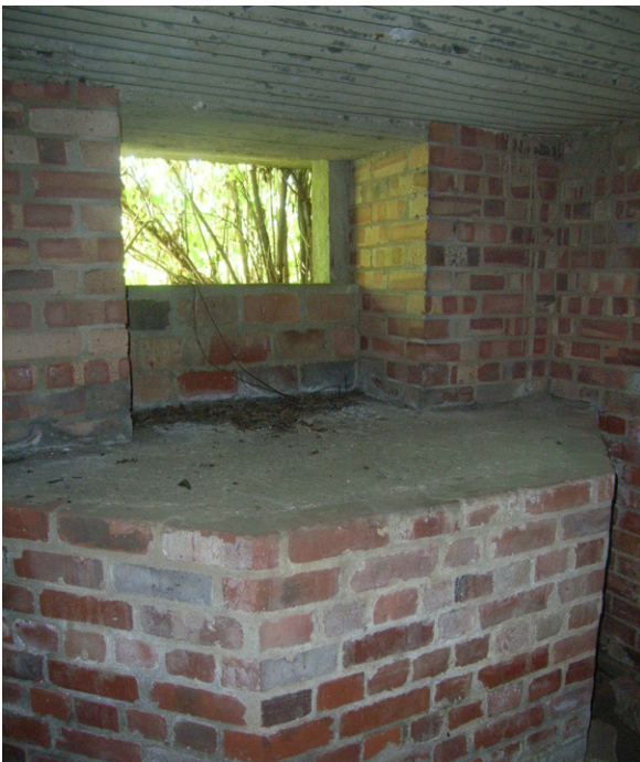
Plate 9: Vickers gun emplacement, stepped embrasure (OA138) (taken in 2010 survey)
