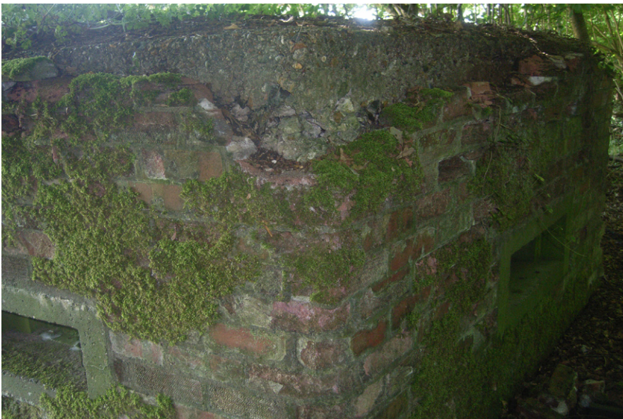
Plate 15: Type 24 pillbox, showing exposed concrete core (OA152)
