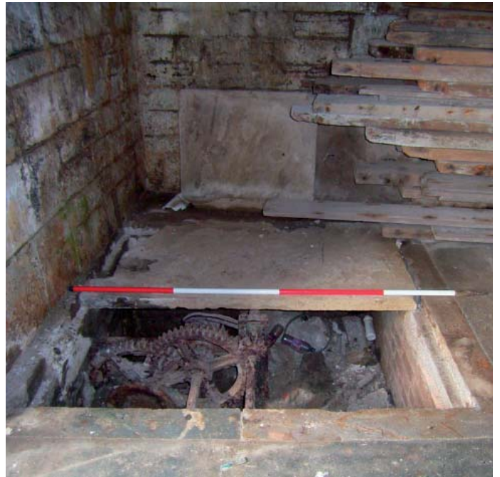
Plate 8: Drawbridge gearing mechanism
