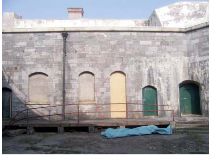
Plate 18: Window in room 12 opened into doorway into inner courtyard
