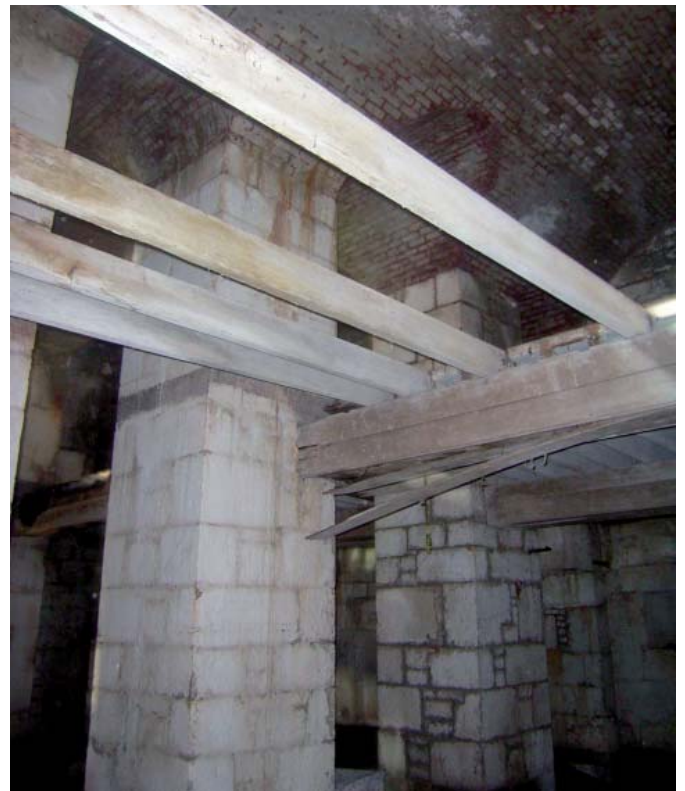
Plate 60: Collapsed floor of upper tier showing layout and construction of caponier
