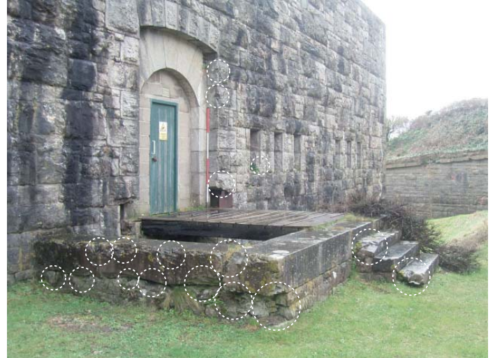
Plate 42: Damage to the south-west drawbridge from the trails of the 32pdr
