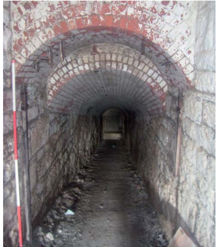
Plate 58: Tunnel into the North-west Double caponier with remains of iron gate
