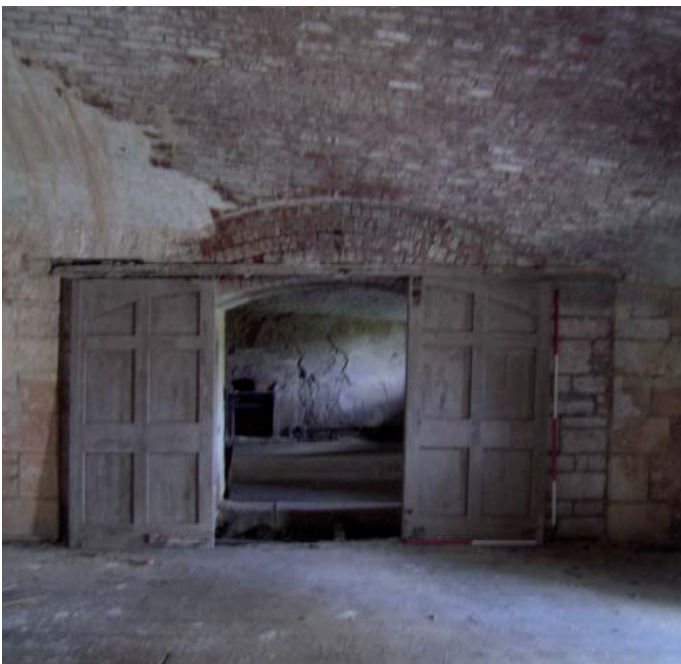
Plate 15: Sliding doors between room 8 and room 9A
