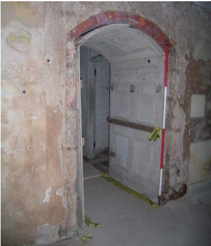
Plate 19: Panel work surviving in arch of central passageway
