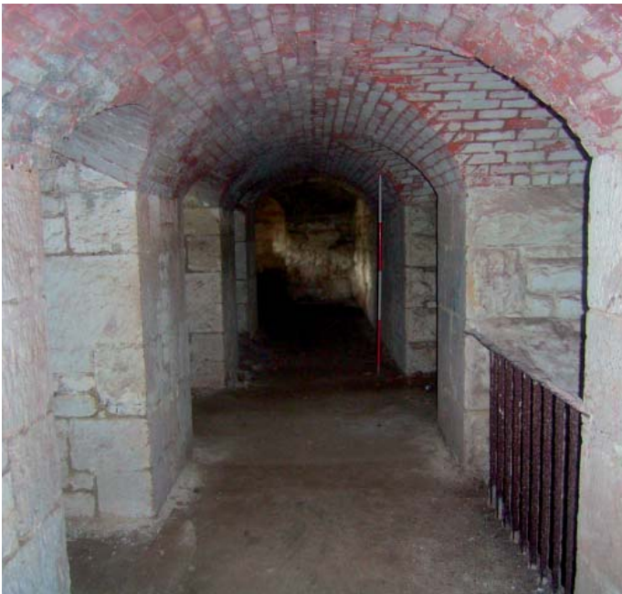
Plate 59: Passage of upper tier with entrance to caponier on the left and entrance from tunnel on right. Railing on right are over stairs into the lower tier
