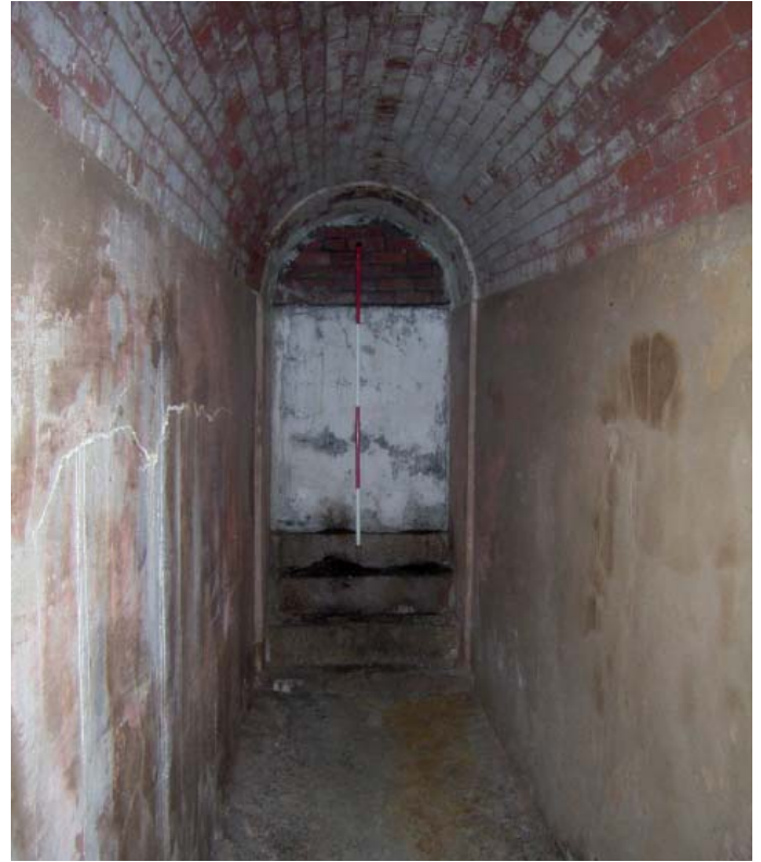
Plate 22: View along passageway (room 19) to blocked doorway onto keep roof
