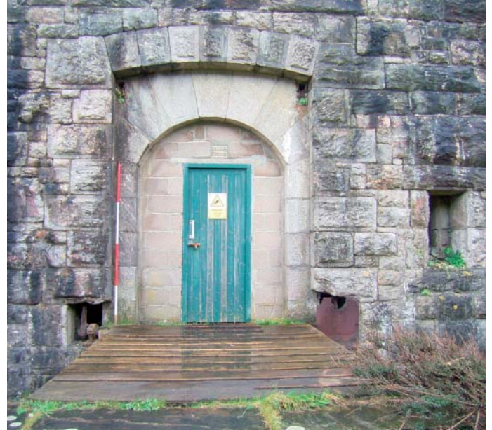
Plate 30: The drawbridge and sally port from the south west caponier
