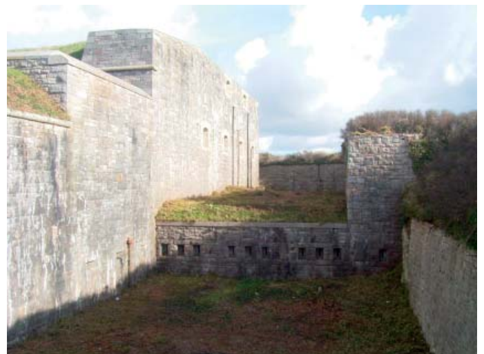
Plate 24: View of galleries facing along ditch with flanking loopholes
