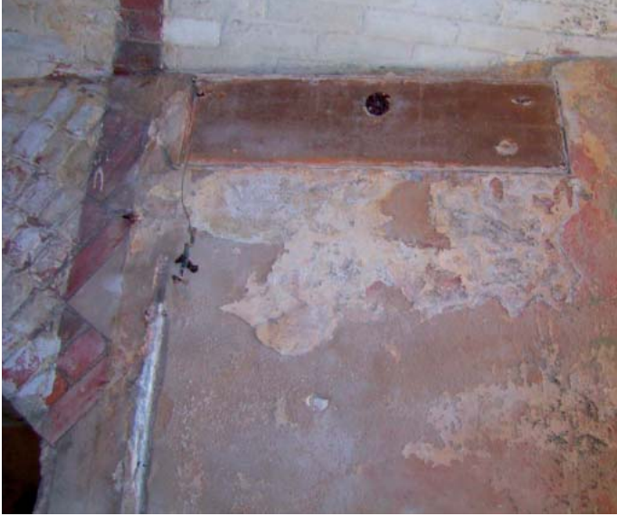
Plate 13: Board on wall for bell pull system
