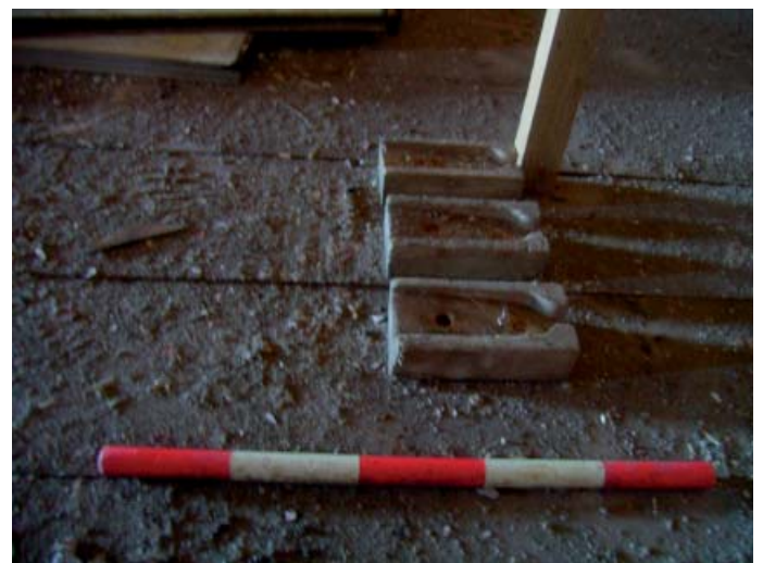
Plate 12: Wood blocks on floor for rifles in rack
