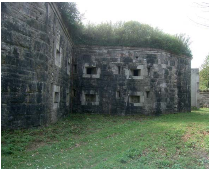
Plate 63: The flanking faces of the North-west Double caponier with modern backstop of the moat range behind
