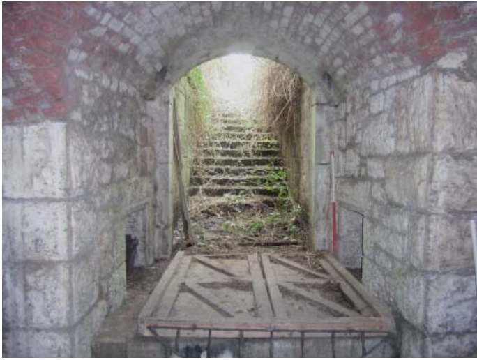
Plate 33: View across drawbridge from passage to NW Double caponier up steps to Chemin de Rondes
