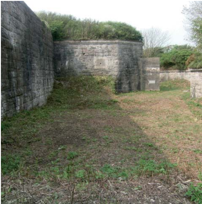
Plate 61: View along ditch towards north-east caponier of double caponier showing later range butt and protective ricochet wall
