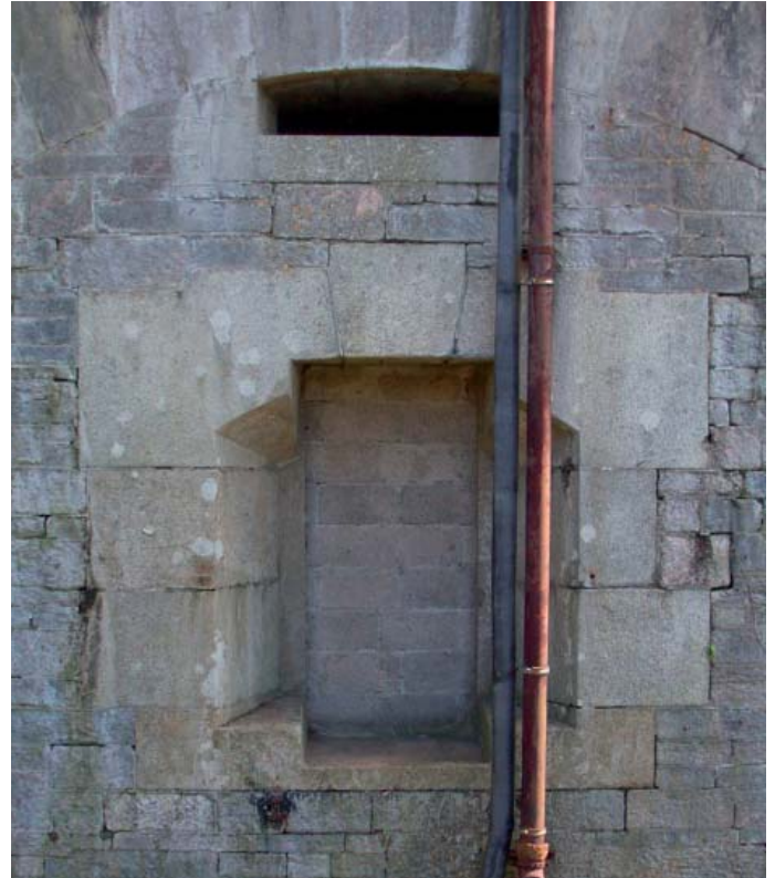
Plate 14: Doorway into room 8 from footbridge across ditch with the sockets in wall below
