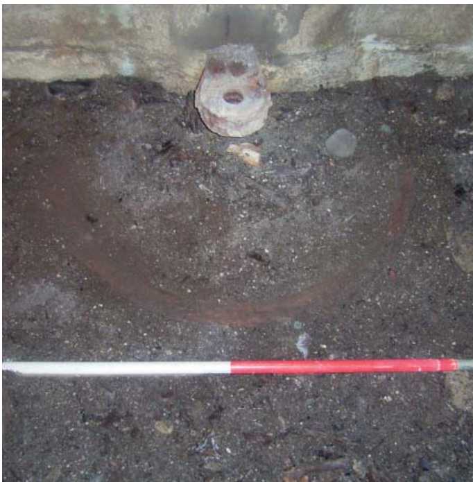
Plate 39: Pivot lug and smaller racer track in north-east caponier
