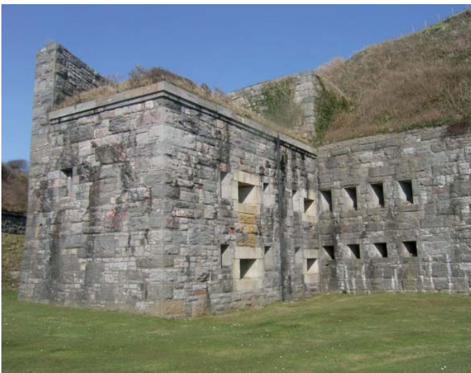
Plate 47: View of the south west caponier showing the granite embrasures and flanking loopholes
