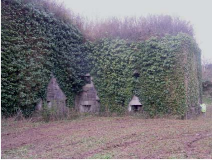
Plate 65: View of the North-east caponier showing the embrasures with drop ditch in front
