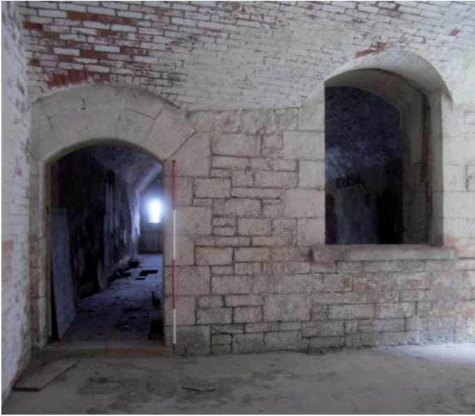
Plate 17: Door and window facing into passage B from room 10
