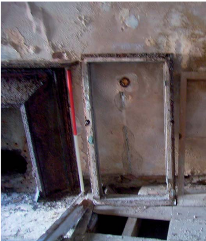
Plate 27: Fitting for bell pull system along side fireplace
