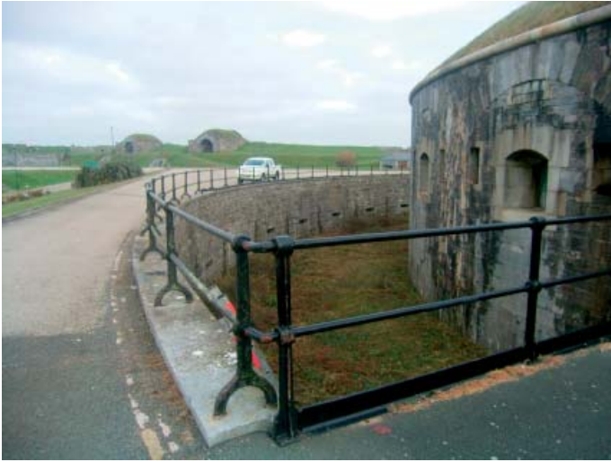
Plate 1: View from bridge into keep showing counter-scarp loopholes and trace of drop ditch
