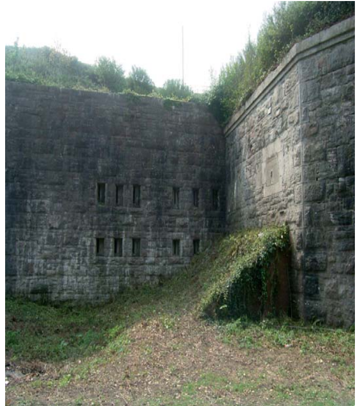
Plate 62: Detail of butt against east face of caponier showing blocked embrasures and loopholes
