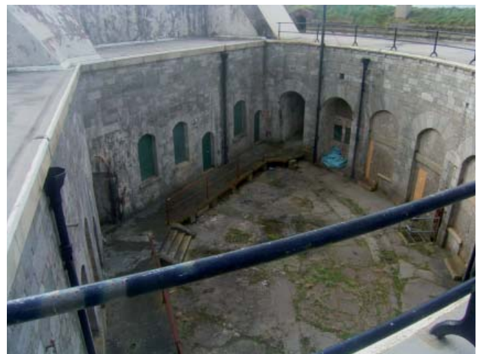
Plate 56: Inner court of the keep looking towards the entrance passage
