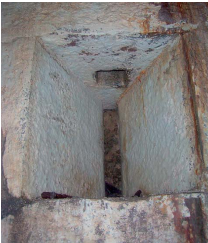
Plate 43: Air vent in the top of loophole in lower tier of double caponier
