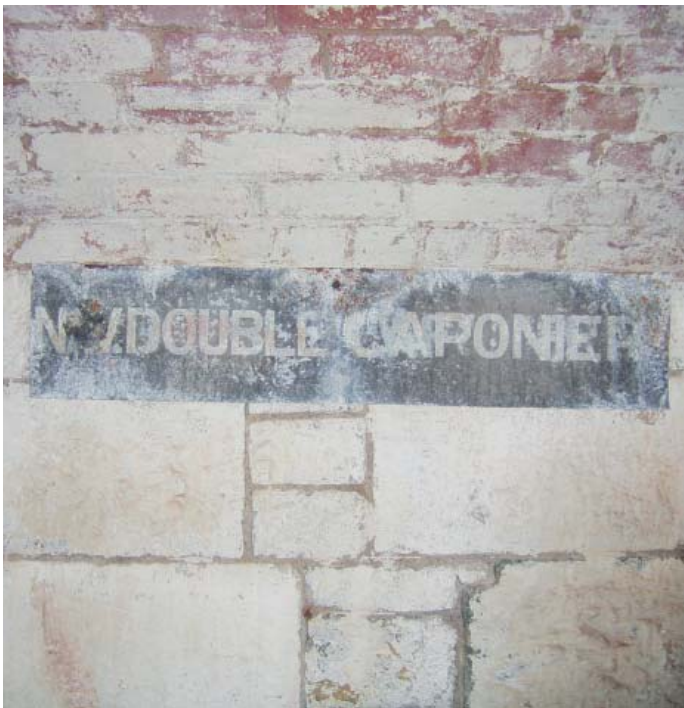
Plate 35: Galvanized sign in upper tier of double caponier
