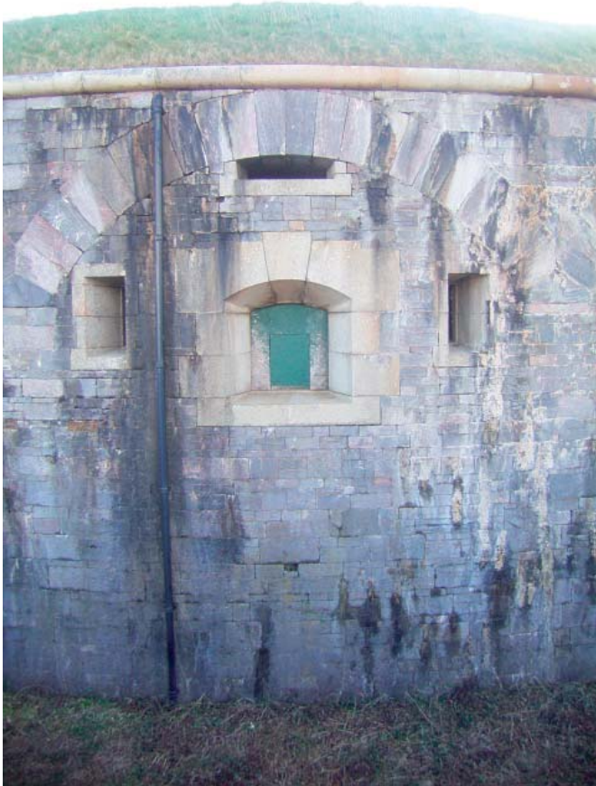
Plate 53: Detail of external view of the keep embrasure and flanking loophole
