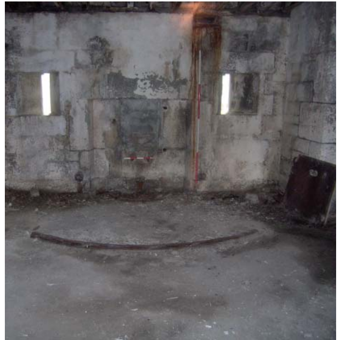
Plate 38: Racer tracks and pivot for mounting the 32pdr SBBL in north-west caponier.
