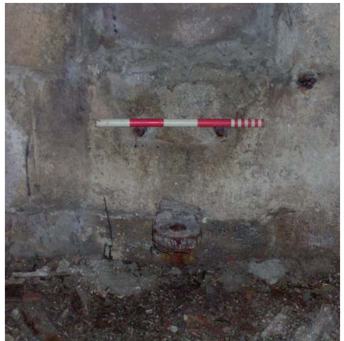
Plate 40: Pivot lug and repair to mounting in north-west caponier from the trails
