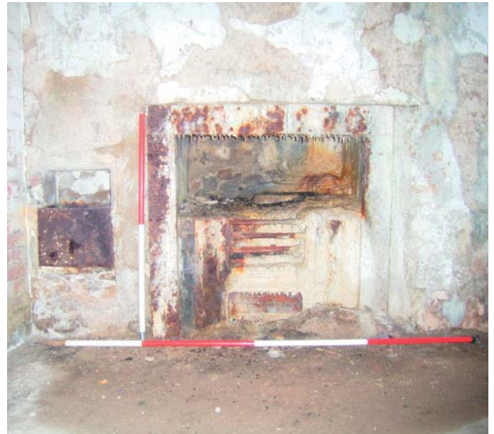
Plate 20: Small cast fireplace and range with cast iron sink to left in room
