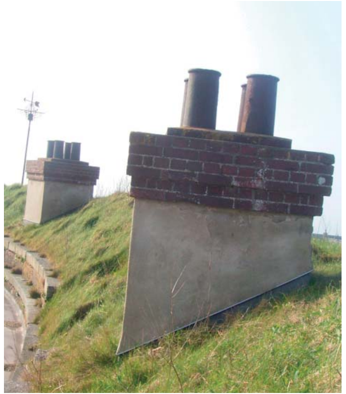
Plate 2: Chimney in earth rampart of keep roof
