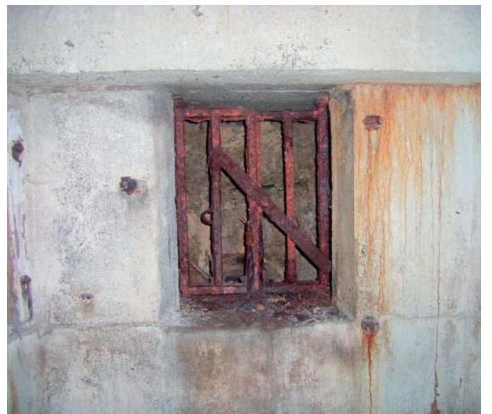
Plate 44: Metal grill of caponier embrasure in place behind later blocking
