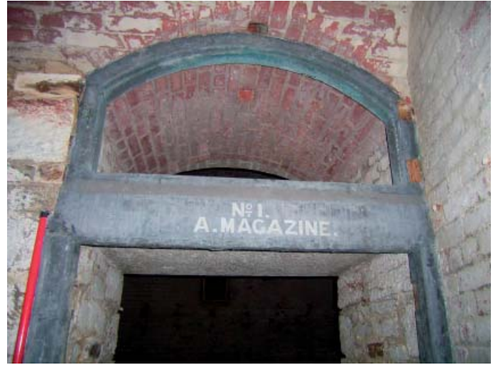
Plate 26: Entranceway into the No1 magazine showing tin covered doorframe and light recess above
