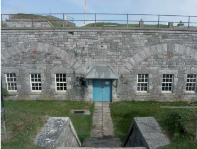
Plate 57: Rooms flanking the entrance of tunnel to the North-west Double caponier
