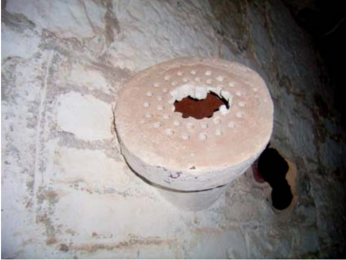
Plate 29: A ceramic vent in end of pipe from store into passage
