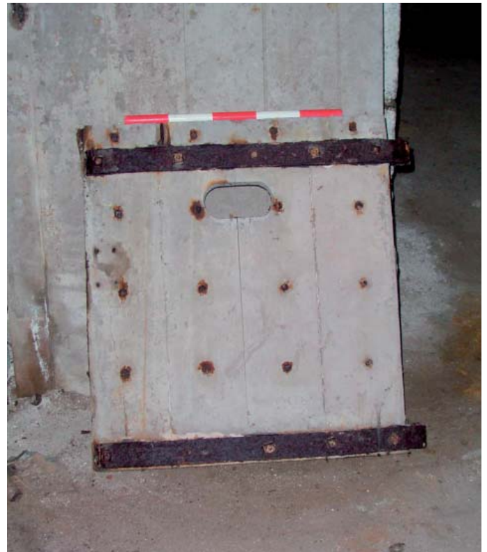
Plate 32: Iron shutter of caponier embrasure, showing wood back, slit and brackets
