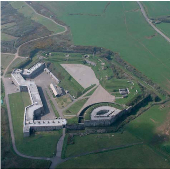
Plate 49: Aerial view of Tregantle Fort showing the entrance and the keep
