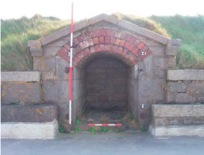
Plate 3: Gun store in earth rampart of keep roof
