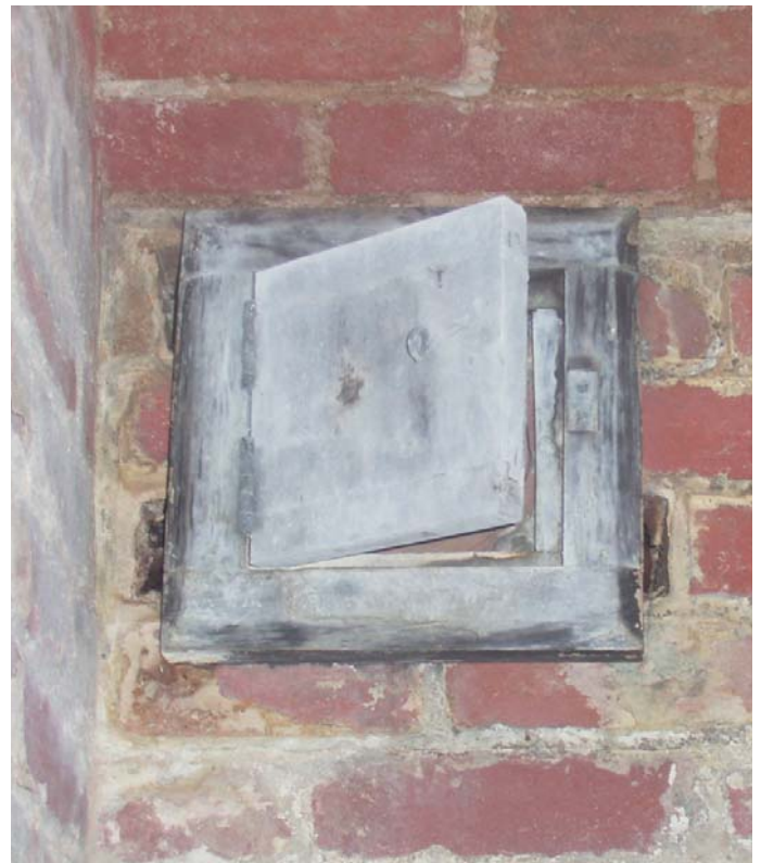
Plate 28: Wood cover over vent from store into passage
