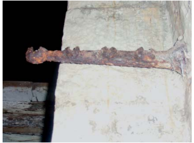
Plate 34: Cast iron bracket of shelf in caponiers
