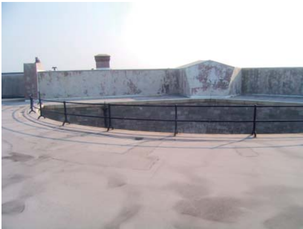
Plate 7: Iron railing around the top of the inner courtyard
