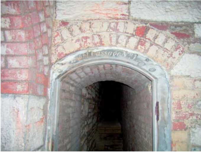
Plate 25: Entranceway into lighting passage of magazine
