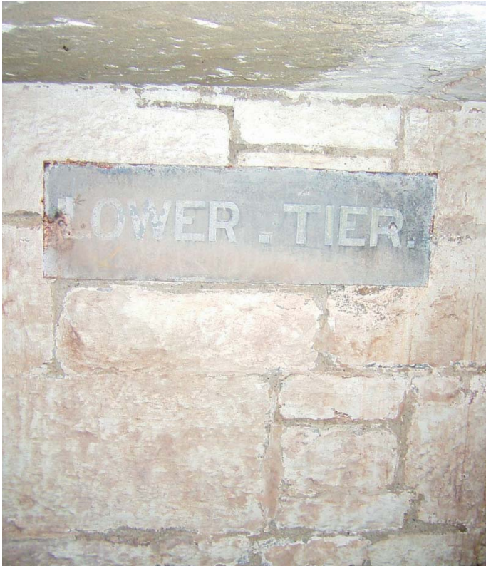
Plate 37: Galvanized sign in Lower tier
