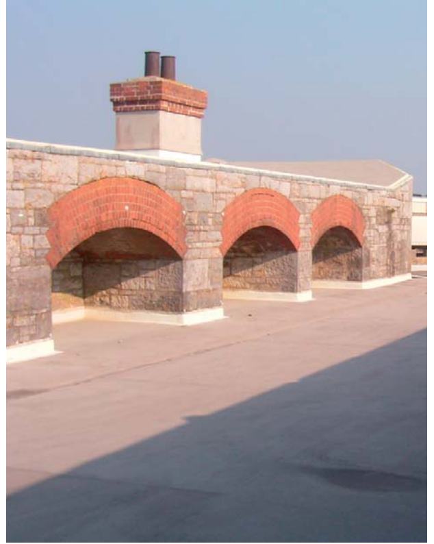
Plate 6: Brick arch ready stores behind embrasures on keep roof
