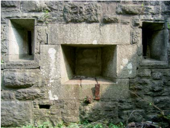
Plate 41: External view of repair to mounting in north-west caponier from the trails
