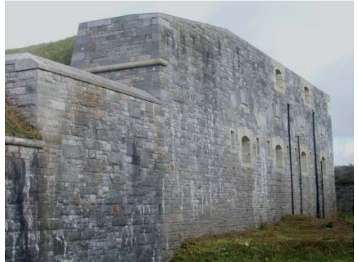
Plate 54: The south-east face of the keep from the bridge into the fort
