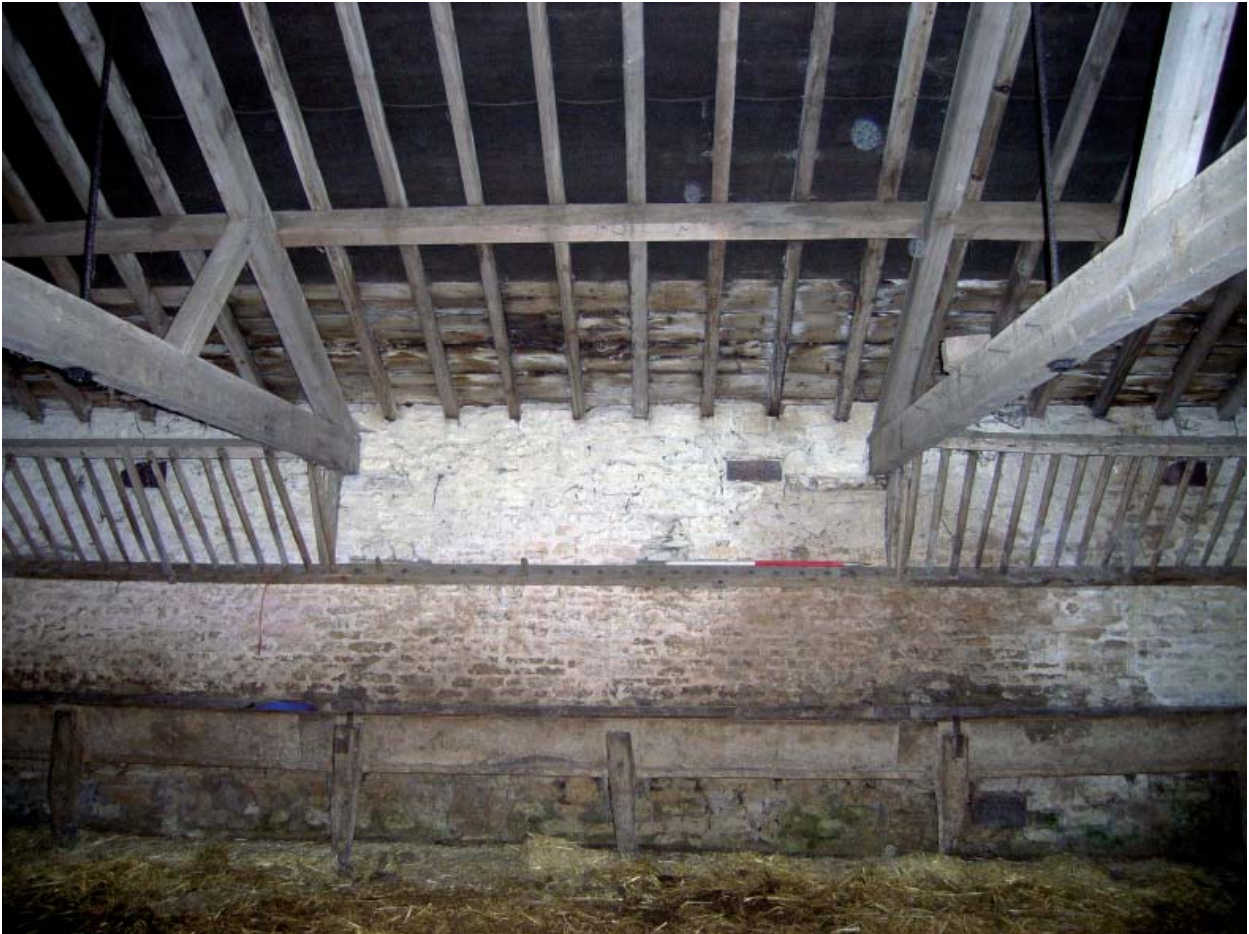
Plate 45: Barn 5; manger and hayrack along south wall in the Easternmost Stable/Loosebox
