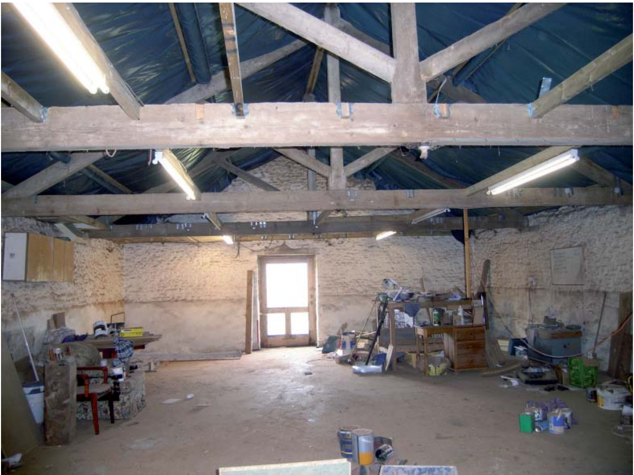
Plate 27: Barn 2; Modern Carpenter's Shop, first floor looking west
