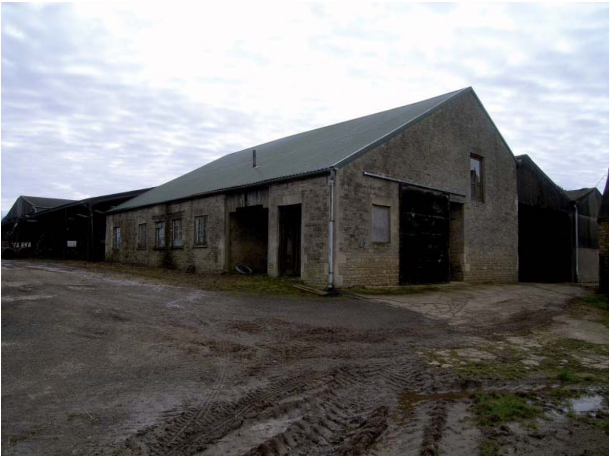
Plate 10: Barn 2; north and west elevations
