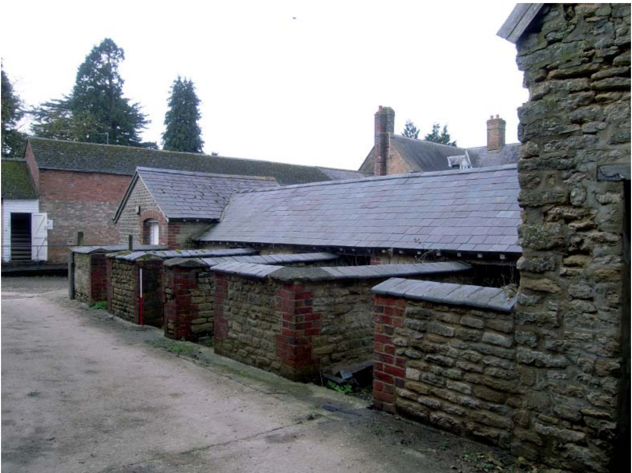
Plate 36: Barn 3; Pigsties and associated building looking south west
