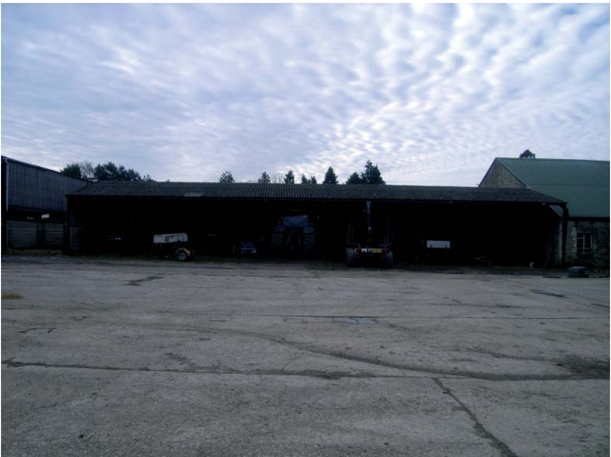
Plate 8: Barn 1; north elevation
