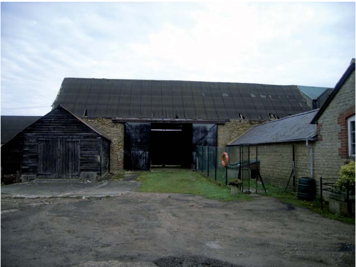
Plate 30: Barn 3; south elevation
