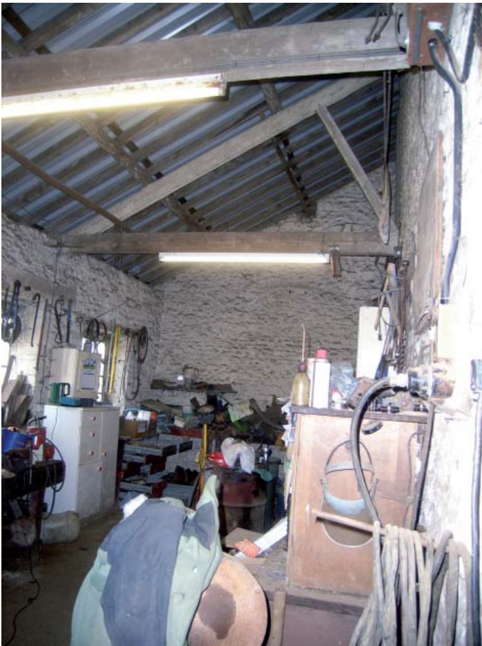
Plate 18: Barn 2; Roof truss in the General Workshop
