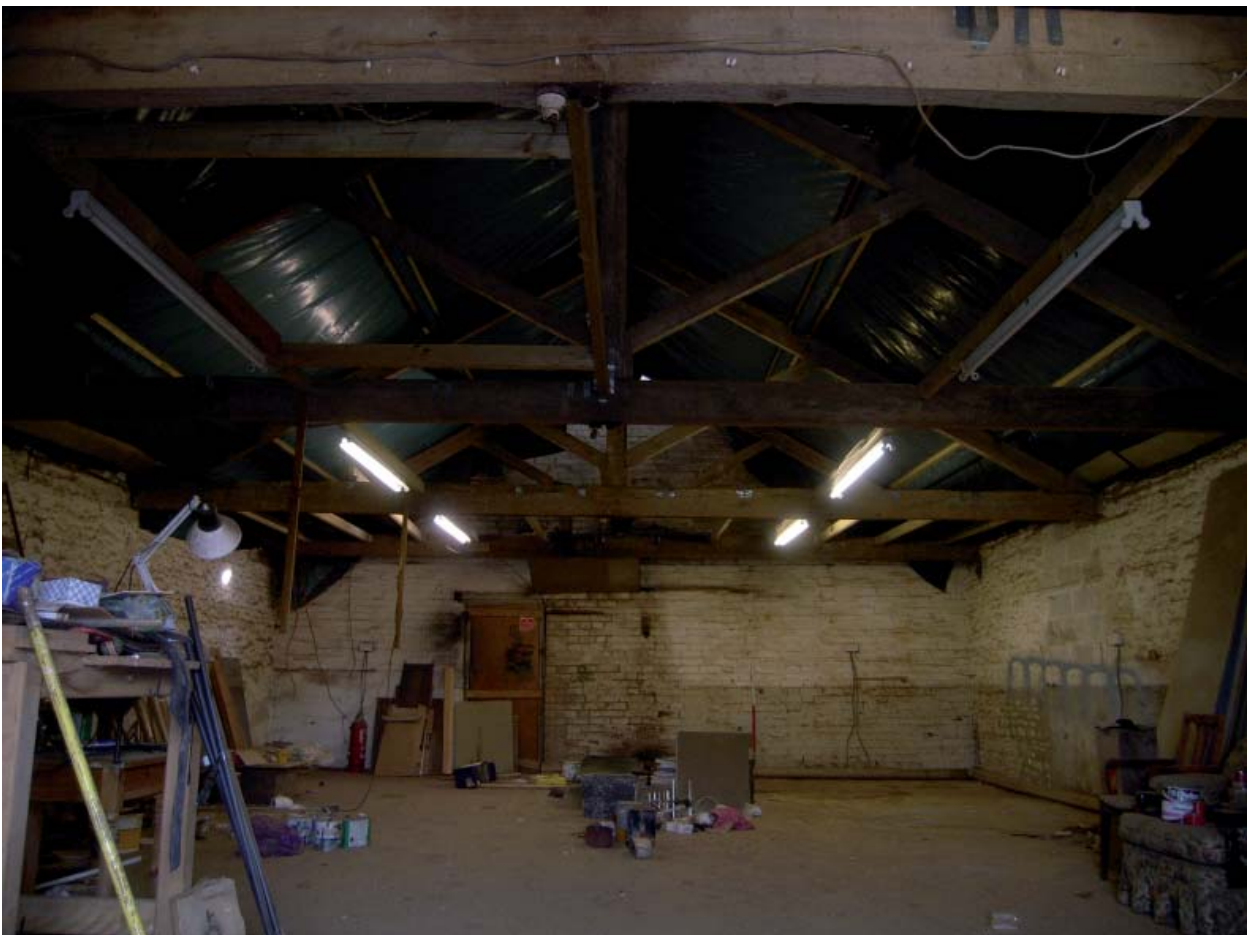
Plate 26: Barn 2; Modern Carpenter's Shop, first floor looking east
