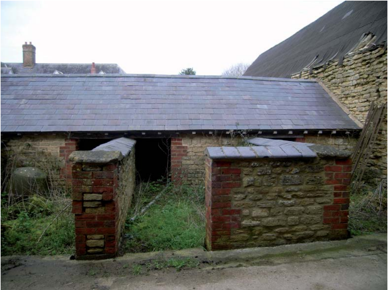
Plate 35: Barn 3; Pigsties to the south of the threshing barn looking west
