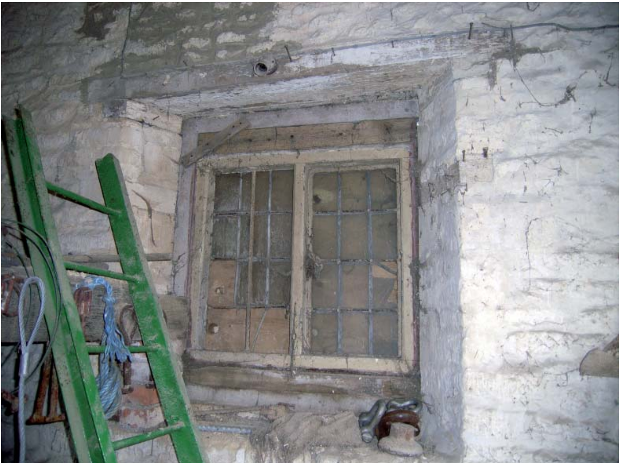
Plate 20: Barn 2; Warming Room window
