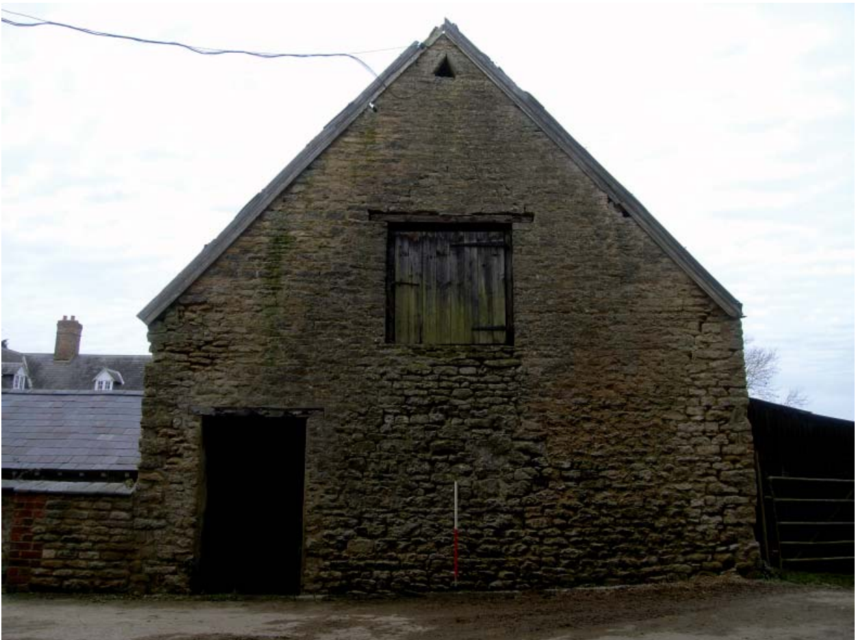
Plate 32: Barn 3; east elevation
