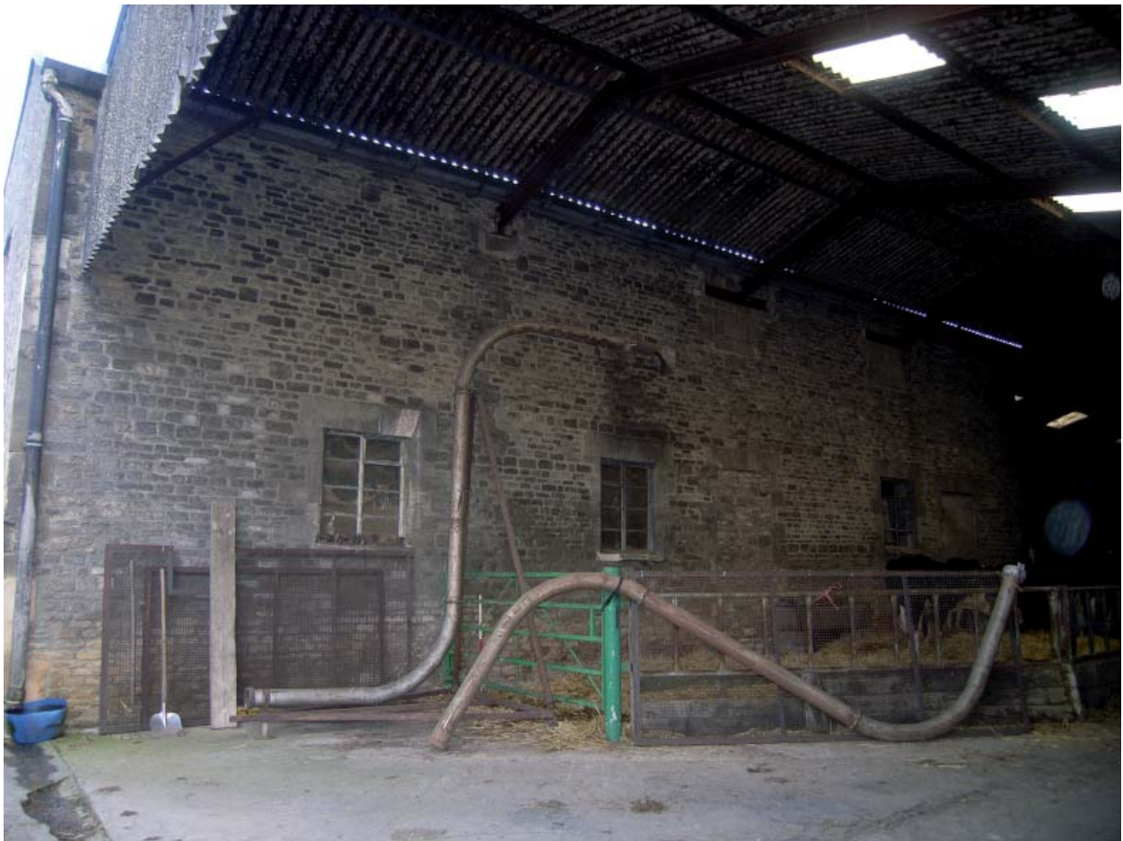
Plate 11: Barn 2; south elevation
