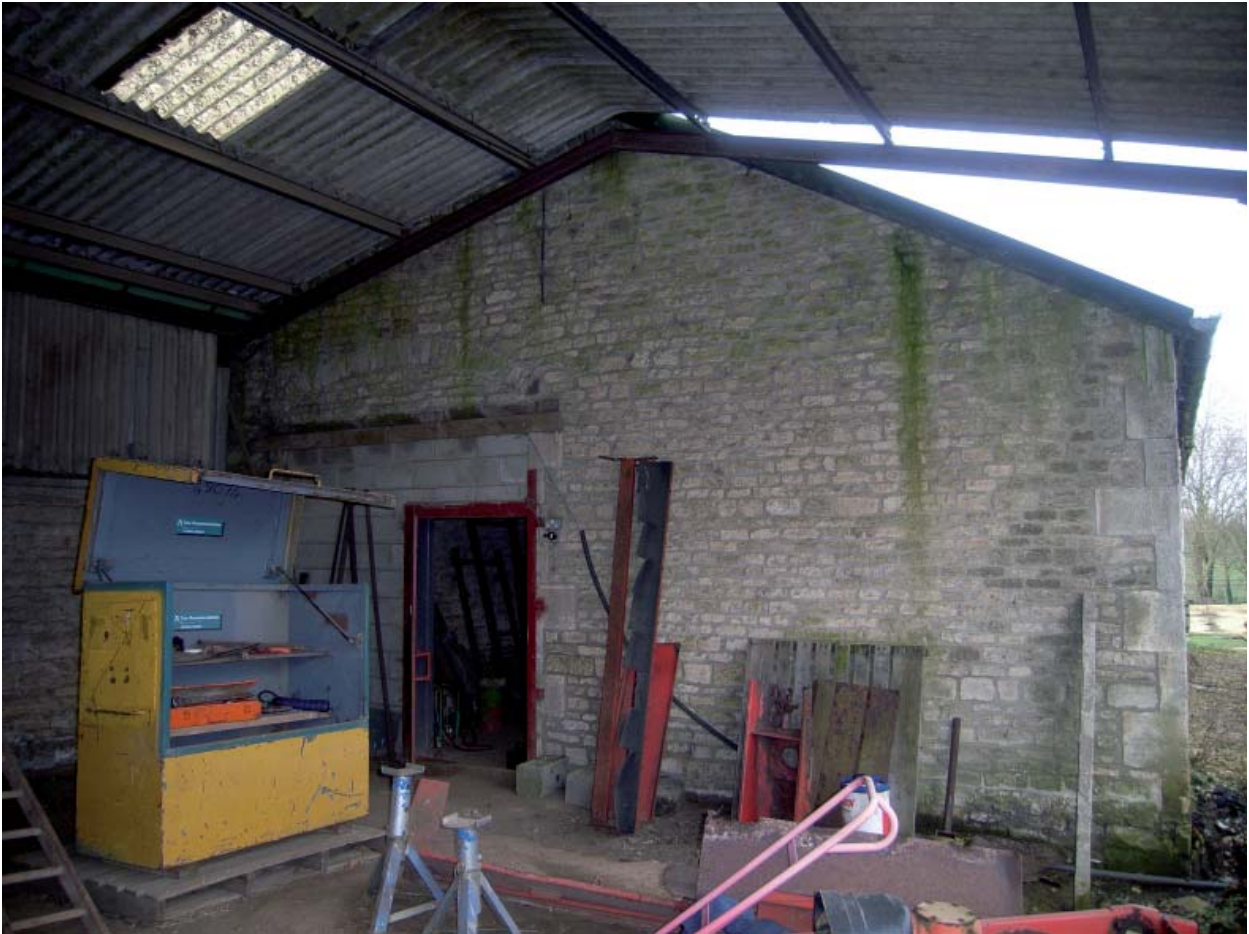
Plate 13: Barn 2; east elevation
