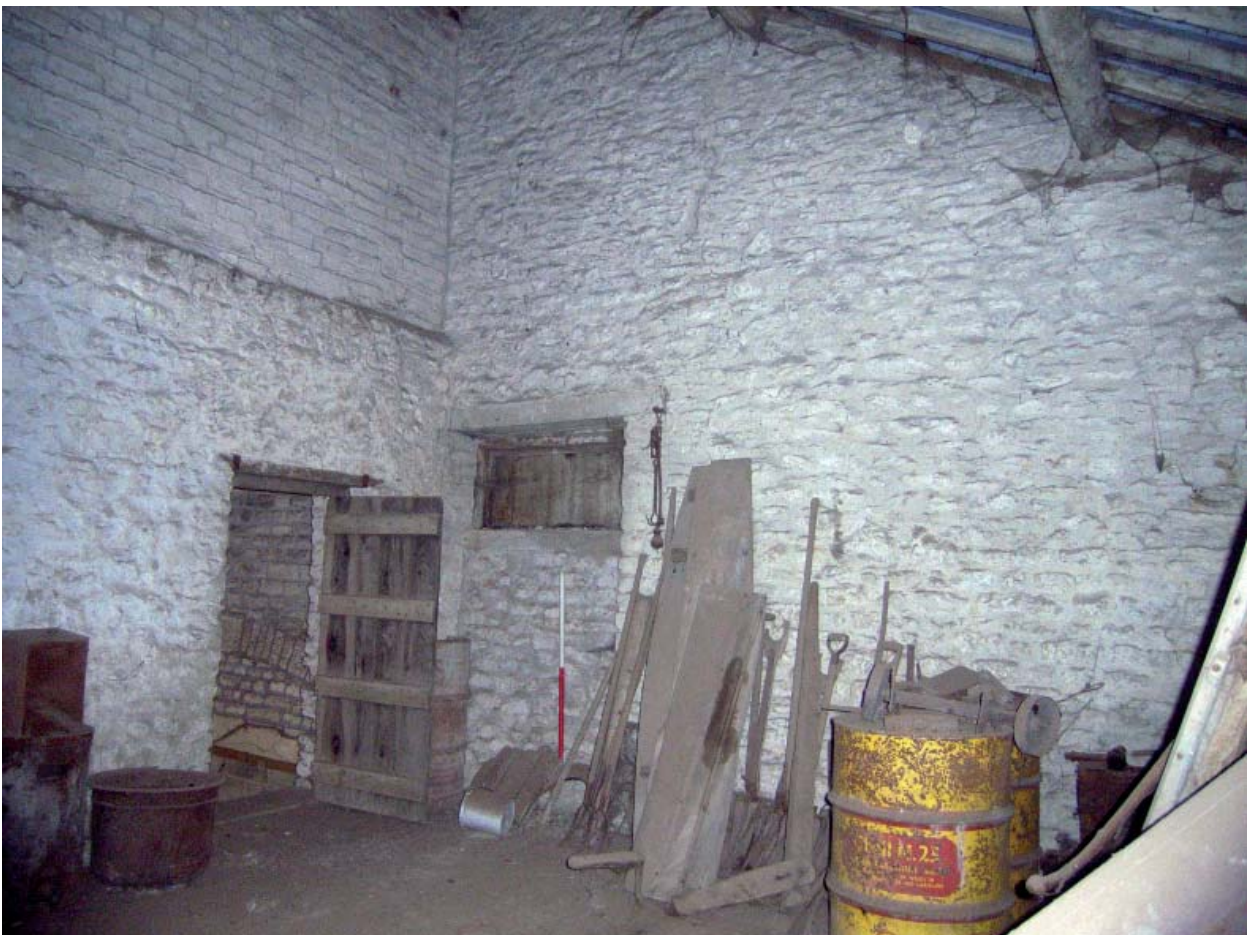
Plate 16: Barn 2; dividing wall between Shepherd's Granary and void over passageway
