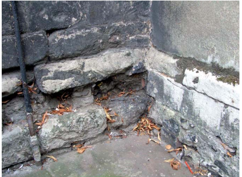
Plate 12: All Saints Vestry, Kingston: North Elevation - detail of join with Holy Trinity Chapel
