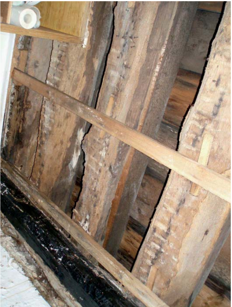
Plate 13: All Saints Vestry, Kingston: Roof timbers inside the vestry
