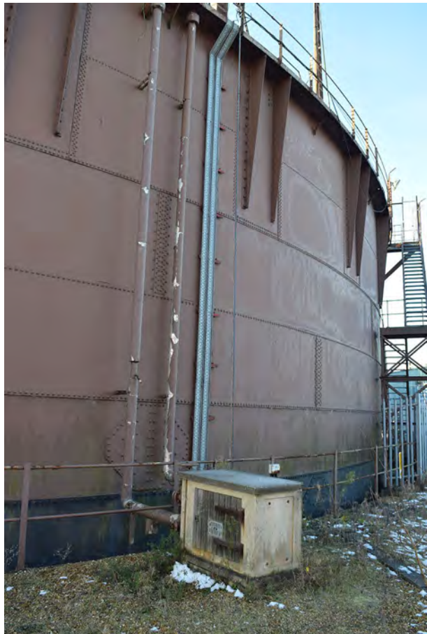
Plate 58: Plant to north side of Holder 71
