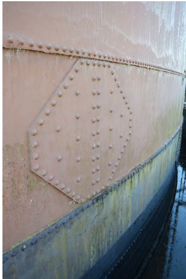
Plate 59: Junction plate to side of Holder 71
