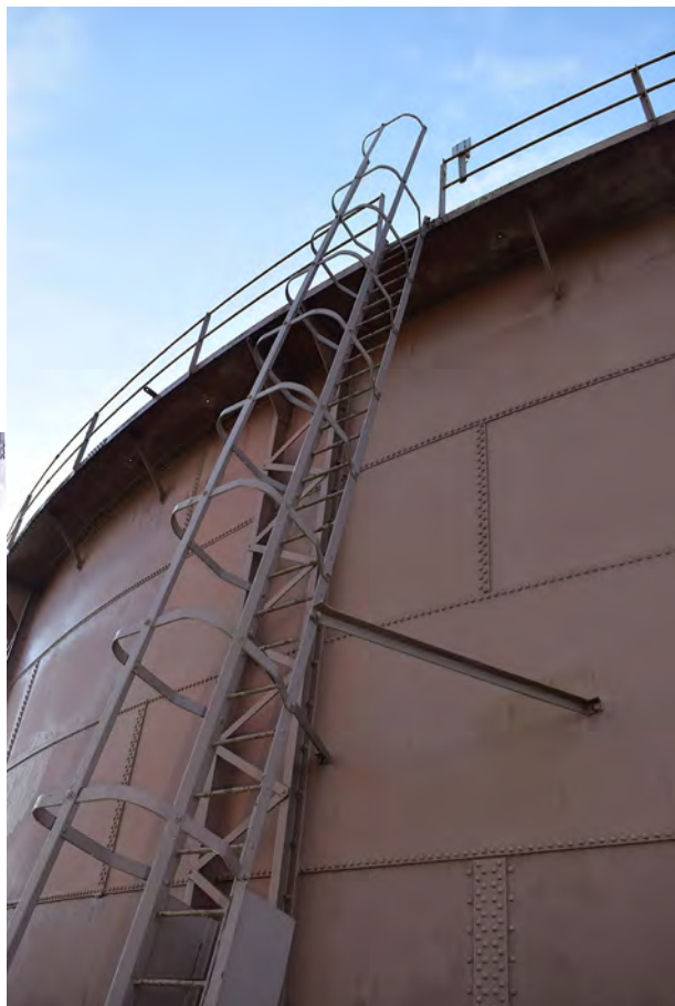
Plate 29: Ladder to side of Holder 70
