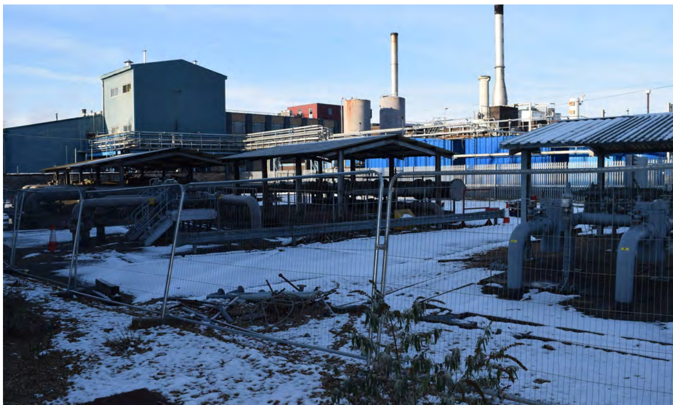
Plate 61: Plant to north-east of gasworks
