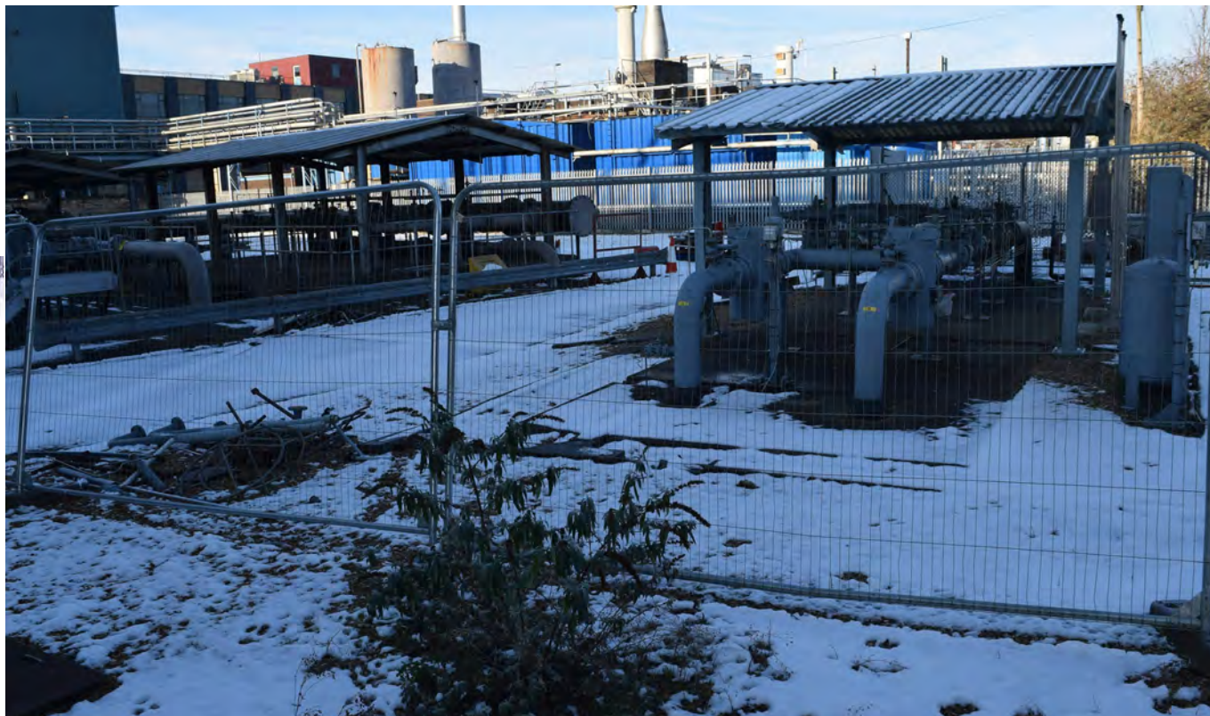
Plate 60: Plant to north-east of gasworks
