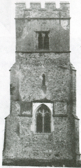
Plate 4 West face of tower (photograph courtesy of Woods Architects)
