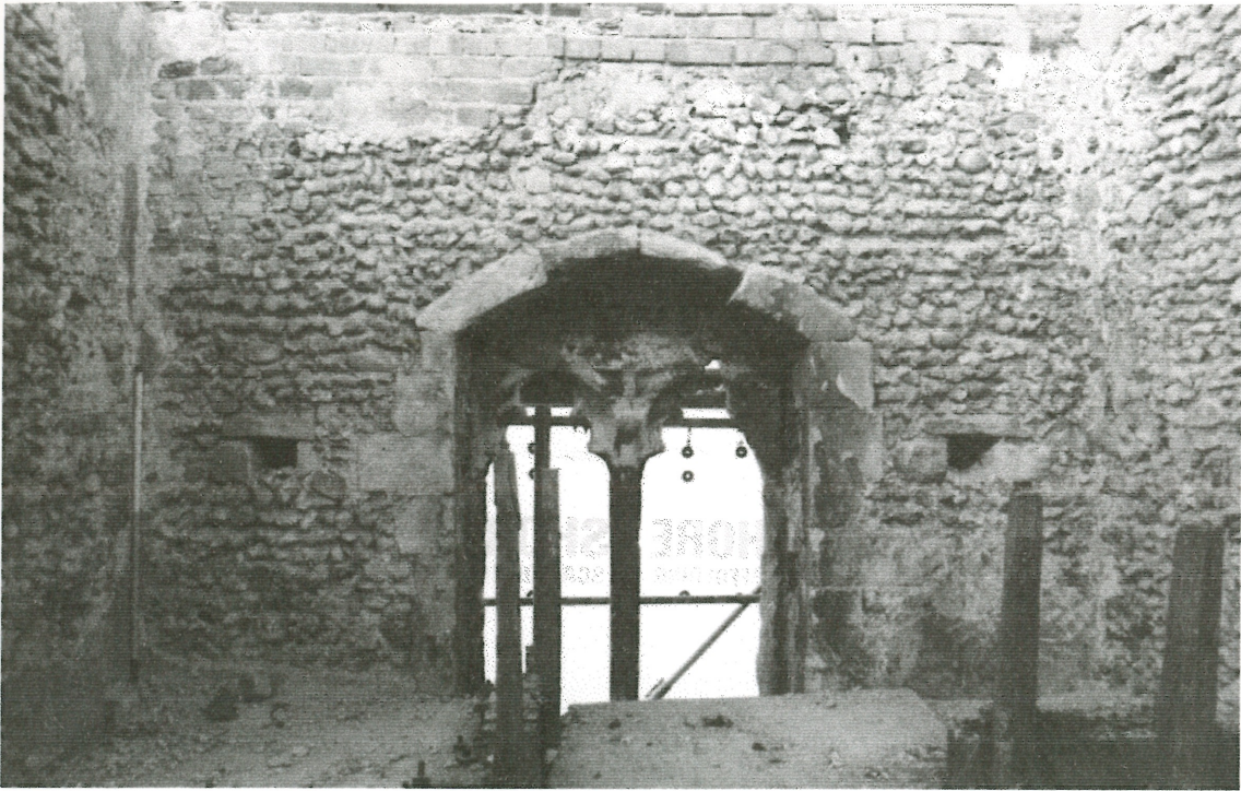
Plate 6 North wall interior at belfry level
