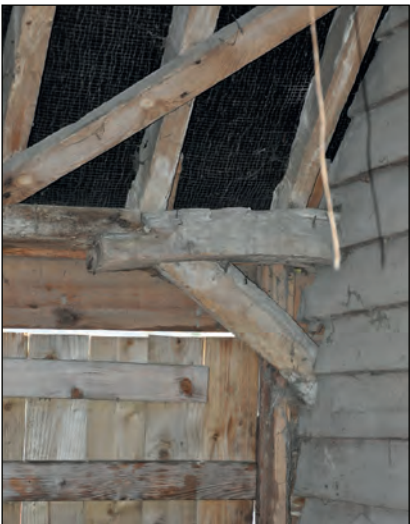
Plate 29: Brace internal to the barn
