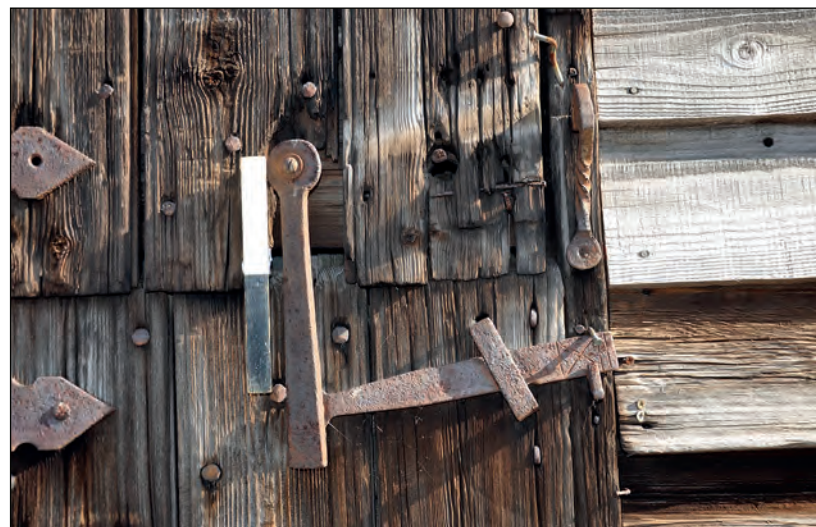
Plate 11: Detail of latch to single door to the the western elevation of the barn
