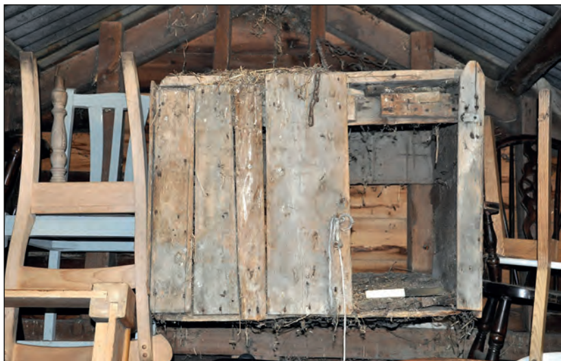
Plate 15: Pigeon or dove box to upper floor
