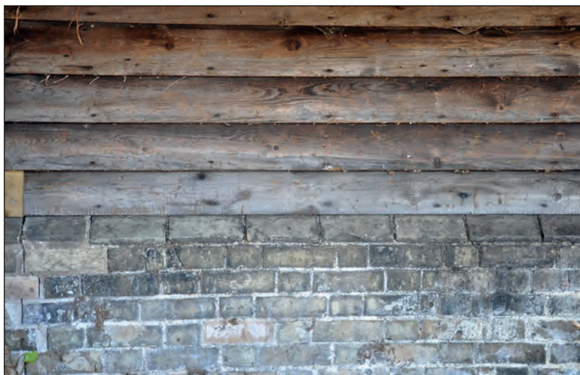
Plate 7: Detail of brick plinth and weather-boards viewed from the east
