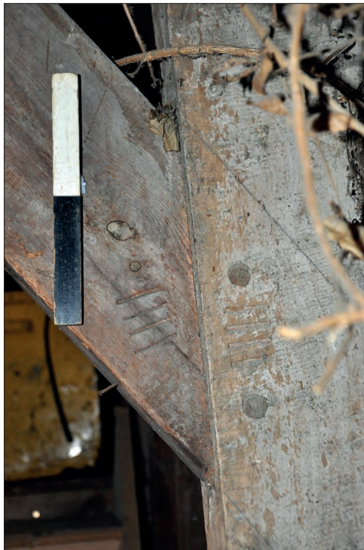
Plate 17: Details of carpenters marks to roof truss viewed from the south
