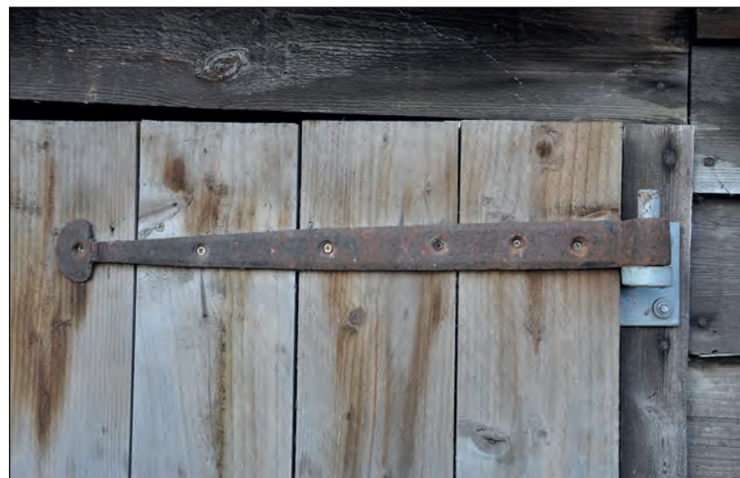
Plate 26: Detail of strap hinge
