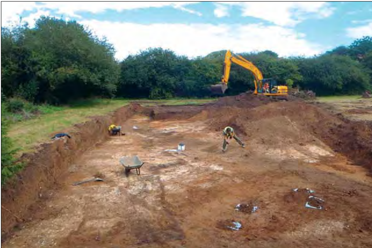
Plate 12: Stripping of the area, looking north-north-west; note cremations in foreground
