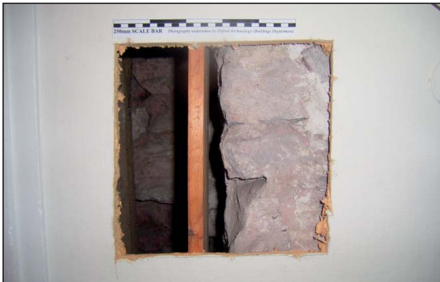
Plate 4: Area 3 opening up - southern reveal of doorway
