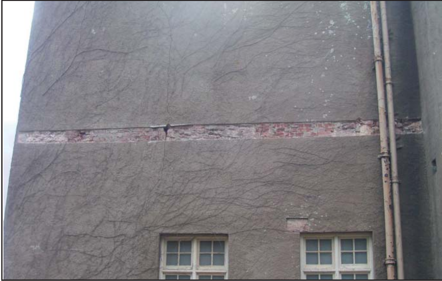
Plate 1: Area 1 opening up on east elevation of south east wing
