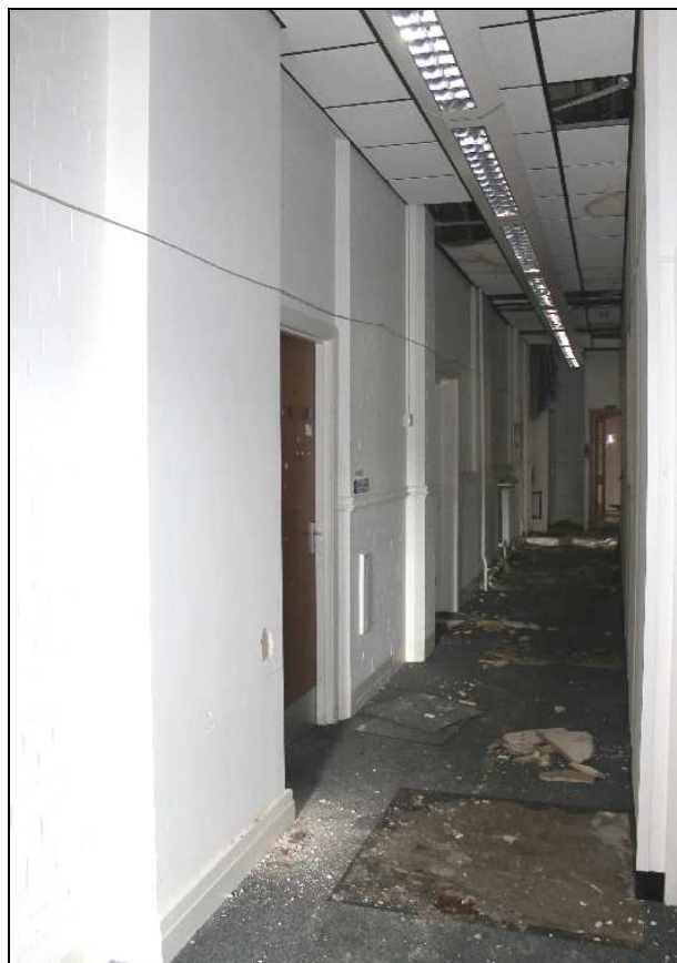
Plate 44: Corridor in South-Western Wing, looking north. Its narrower width is accounted for by a later partition to the right of frame
