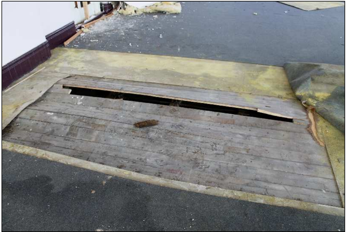
Plate 56: Original polished floorboard beneath the carpet in room 304
