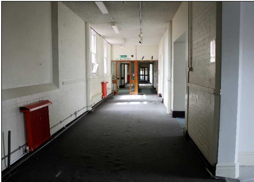
Plate 39: Northern range corridor, facing west
