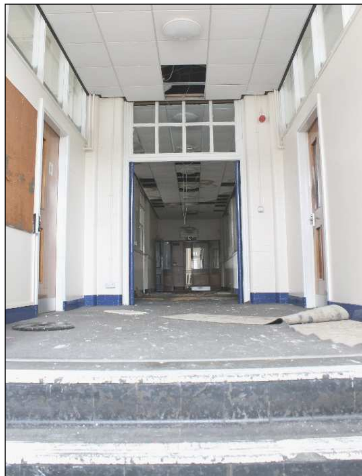
Plate 30: South-western corridor, facing north
