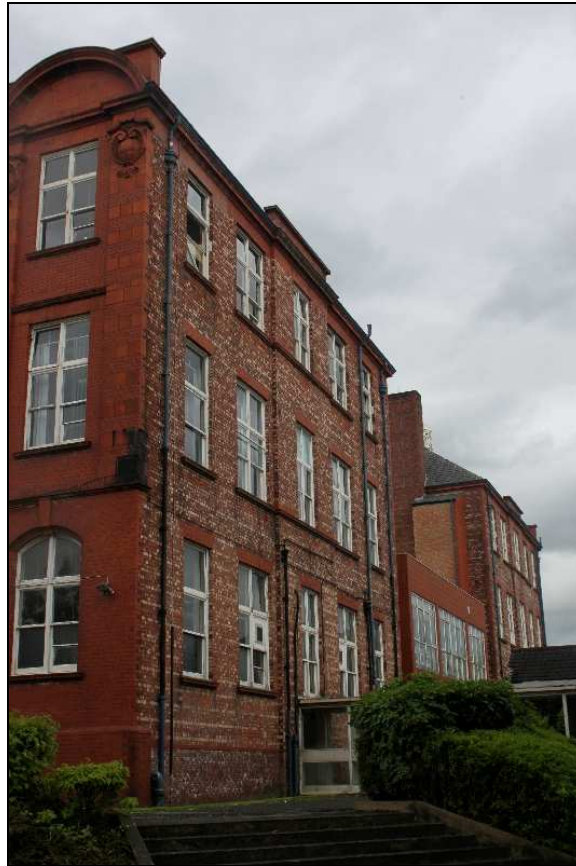
Plate 22: Southern elevation facing north-east. Note the glass sided linking corridor at the base
