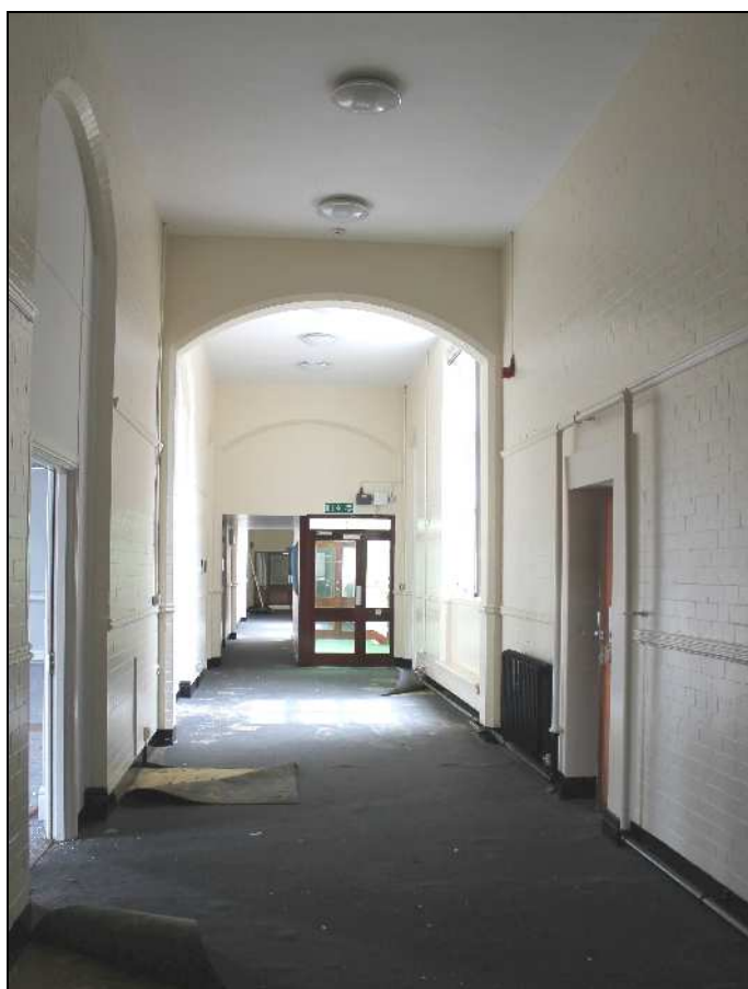
Plate 47: Second-floor corridor in the main northern range, facing east
