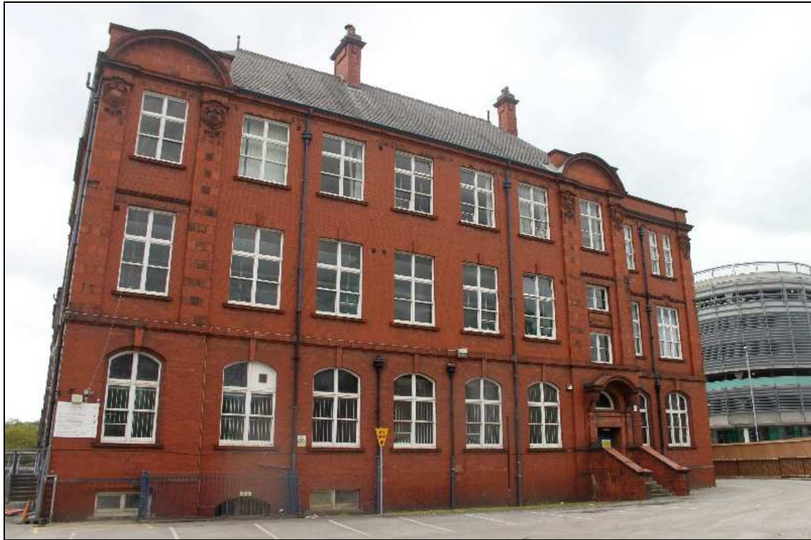
Plate 16: Eastern elevation of the South-Eastern Wing
