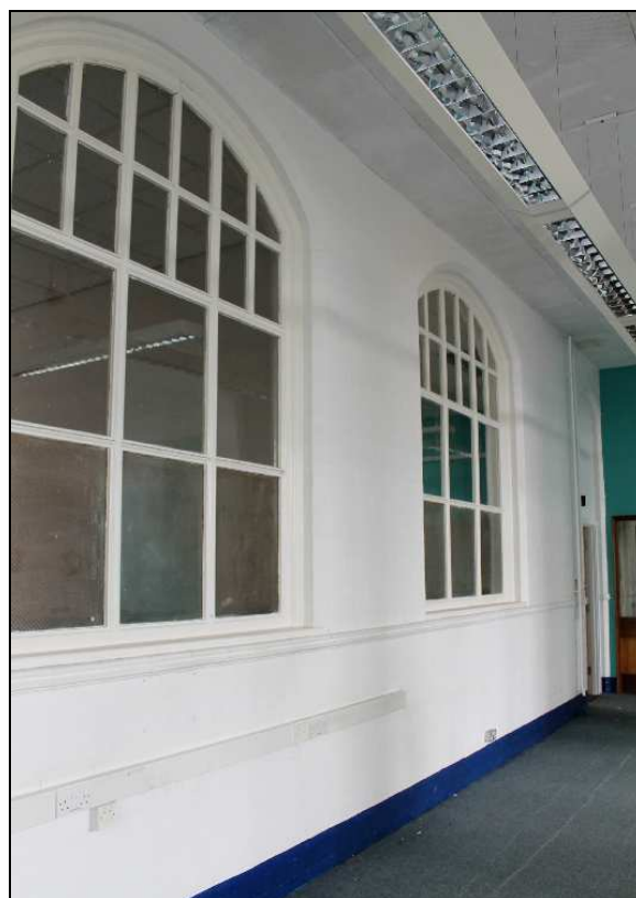
Plate 40: Internal windows in corridor in south-eastern wing, facing north
