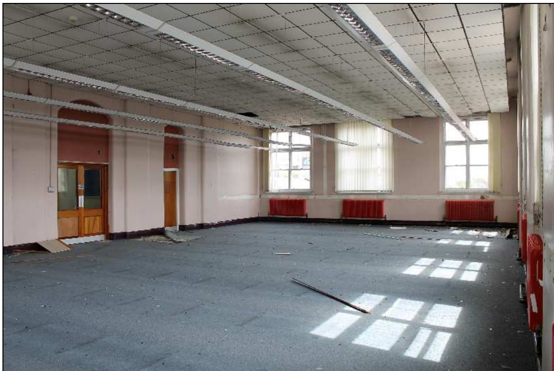
Plate 52: Room 317 at southern end of the South-Eastern Wing, looking east
