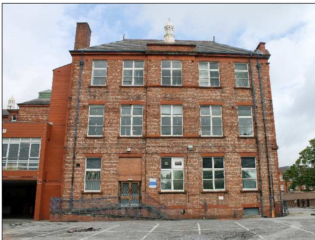
Plate 18: Southern elevation of the South-Eastern Wing
