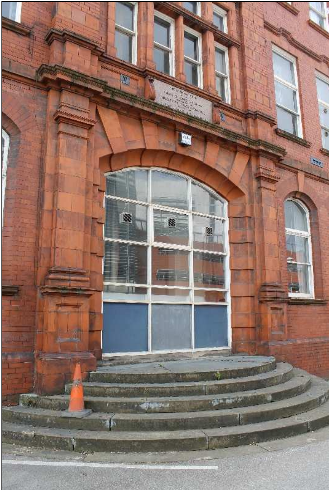
Plate 5: Semi-circular steps to original entrance
