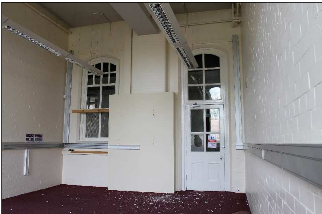
Plate 32: Typical design of internal windows and doorways lighting the corridors
