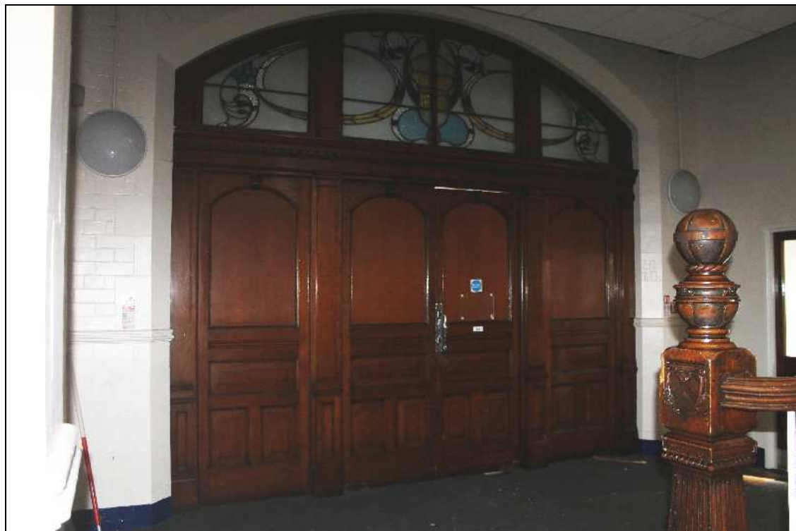
Plate 26: Timber partition defining entrance to original lobby with stairs to right of frame
