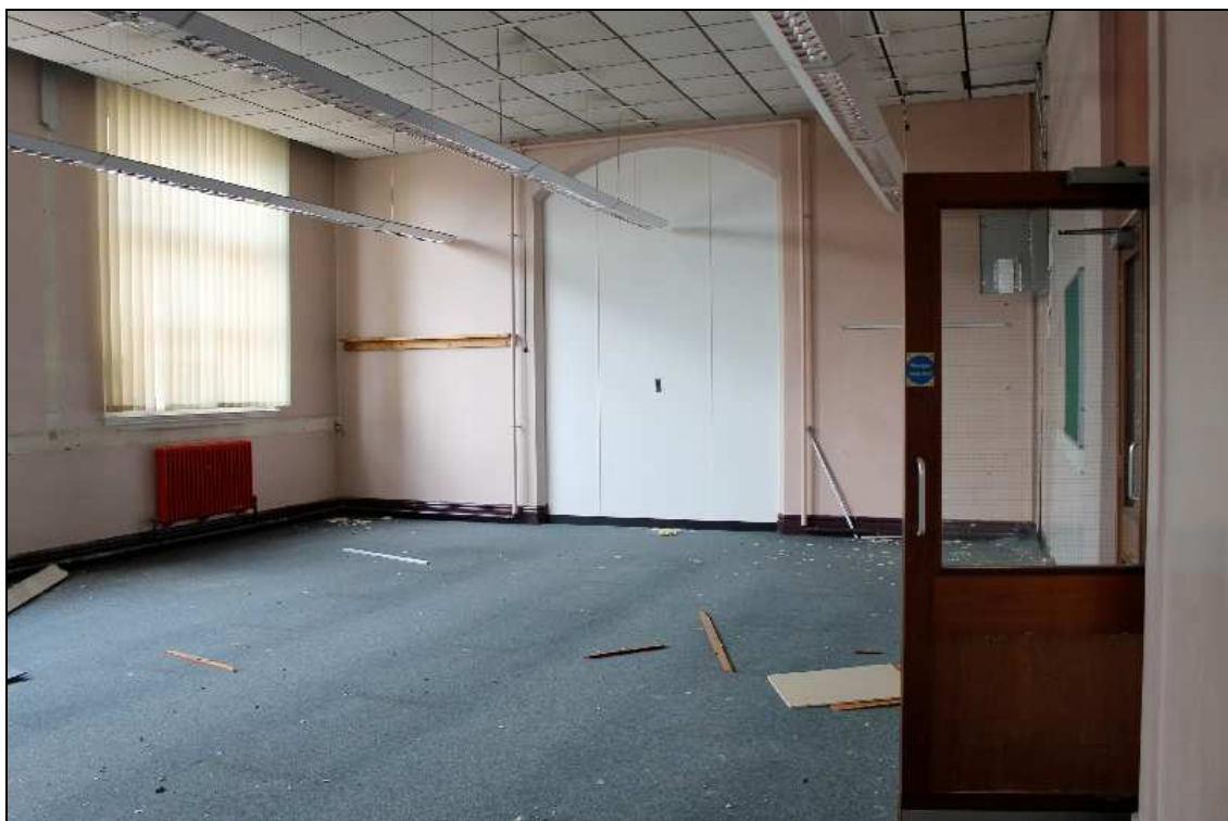
Plate 53: Large blocked opening in room 318, looking north
