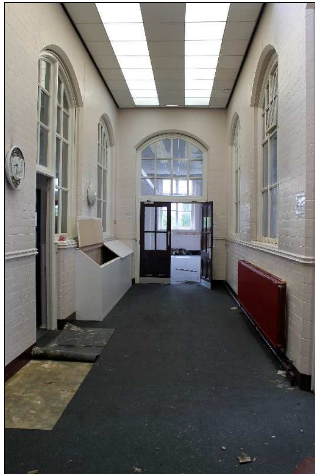
Plate 54: Corridor in South-Western Wing, looking south
