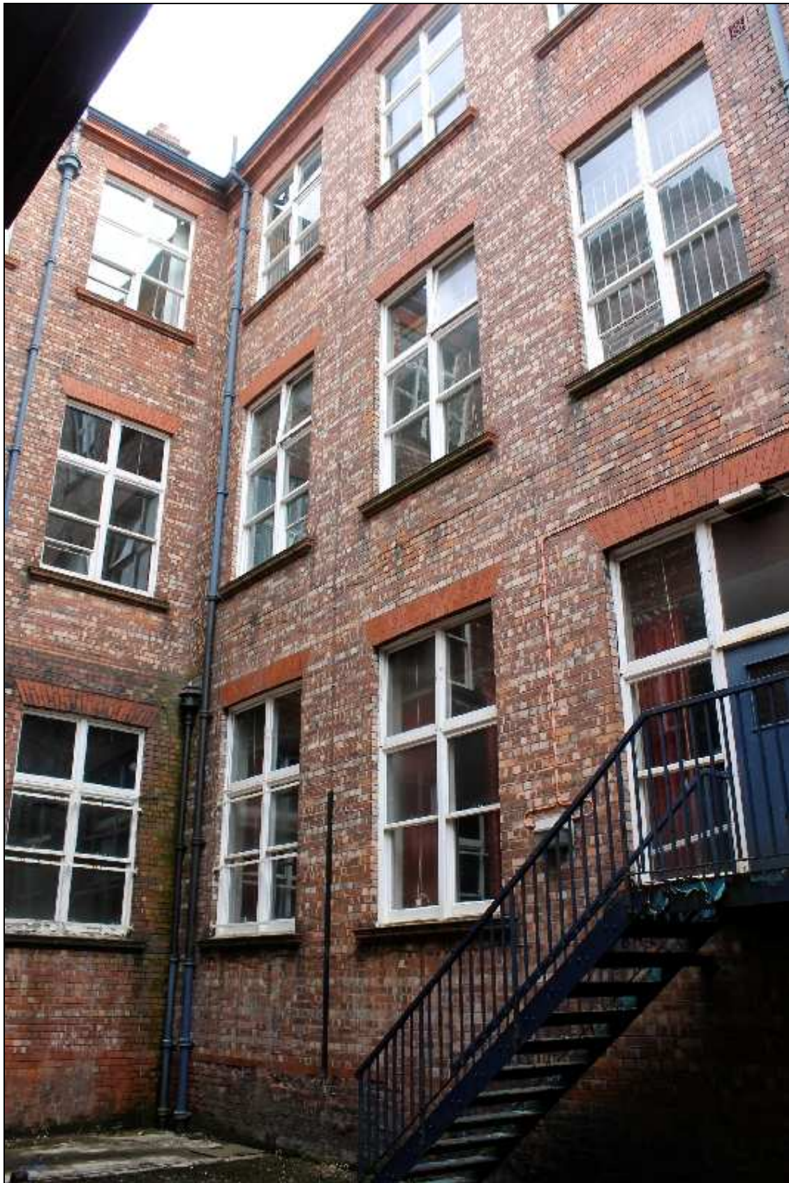
Plate 20: Western elevation of the South Eastern Wing, ground-floor facing north-east, with doorway to right of frame
