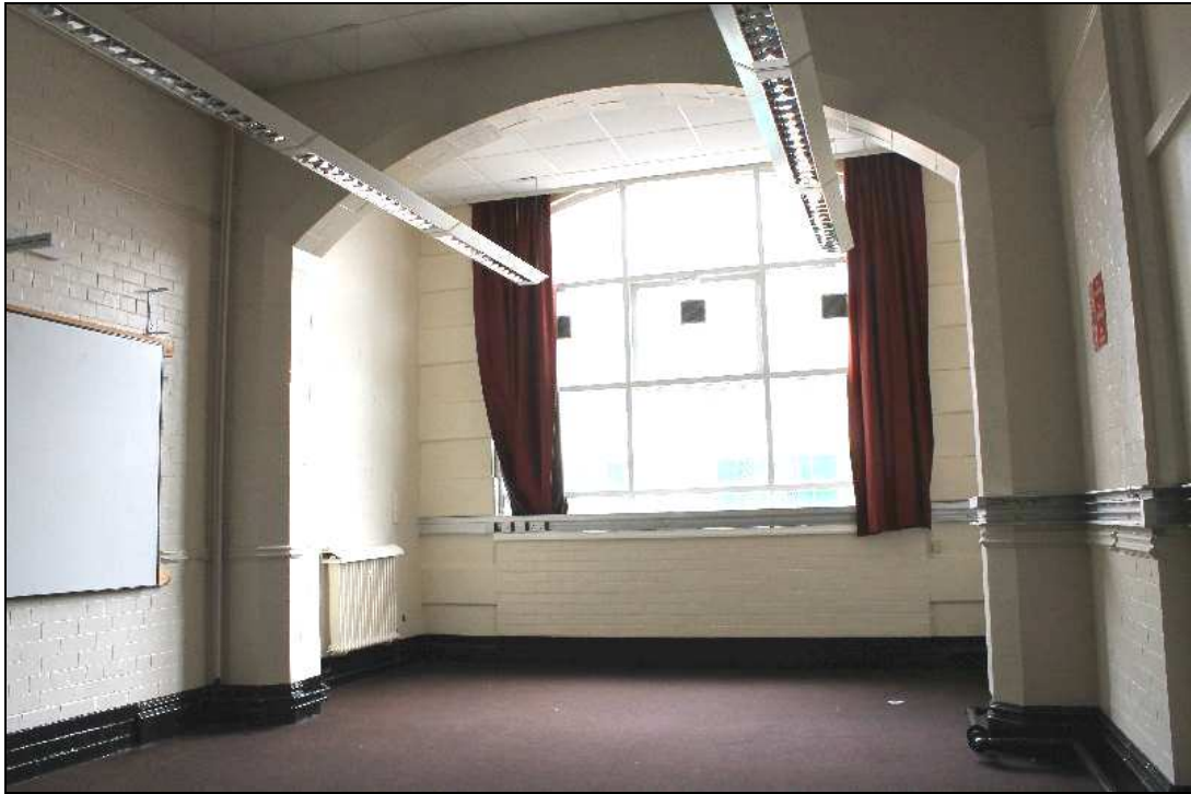
Plate 27: Original entrance lobby, facing north
