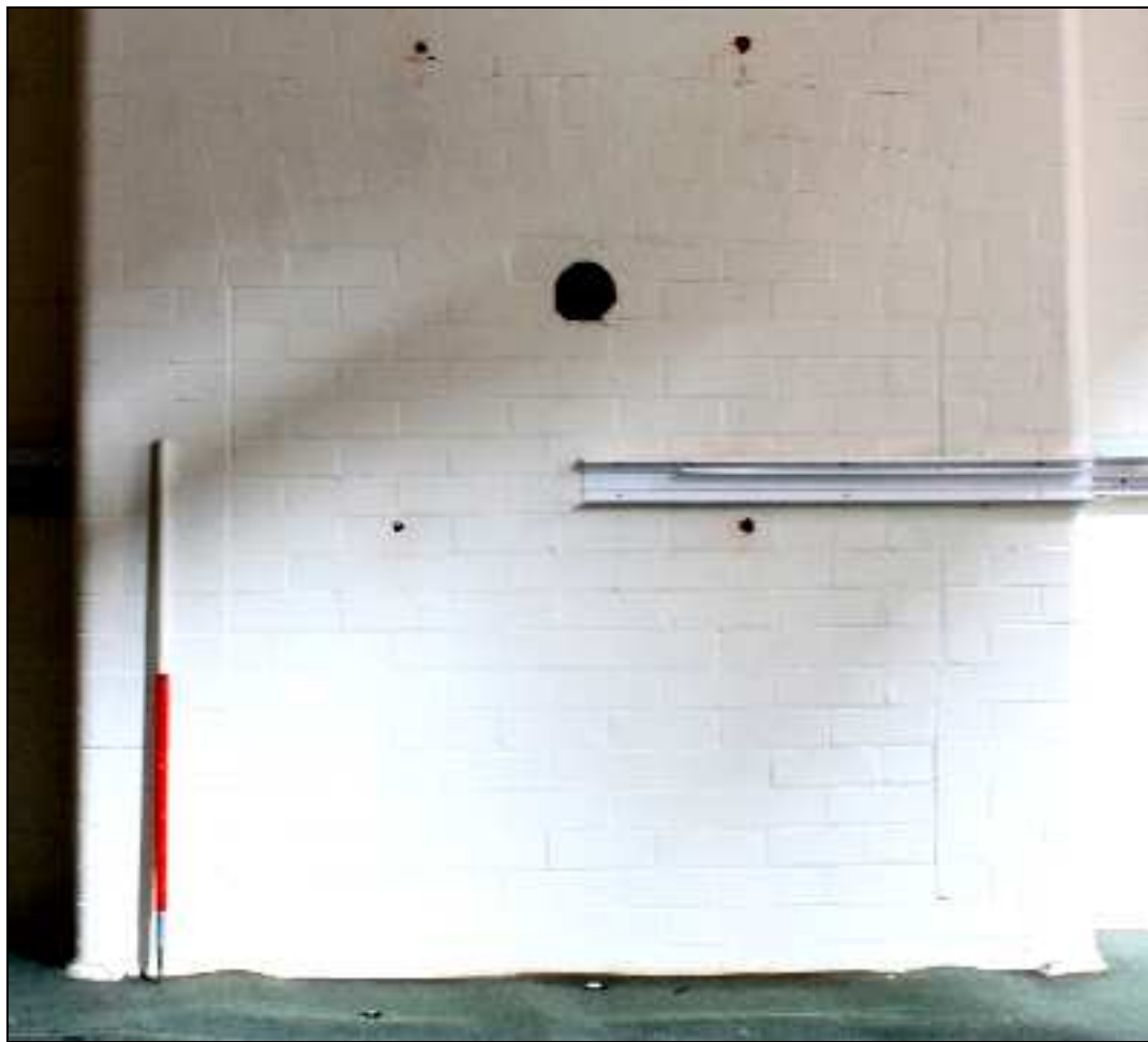
Plate 36: Blocked fireplace in lecture room 101, typical of those in the rest of the building. 1m scale
