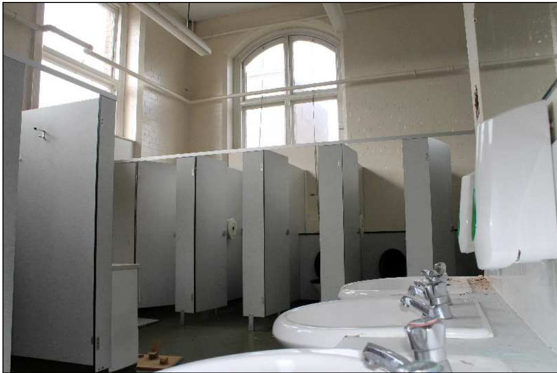
Plate 31: Toilet block in south-western corner of the South-Western Wing
