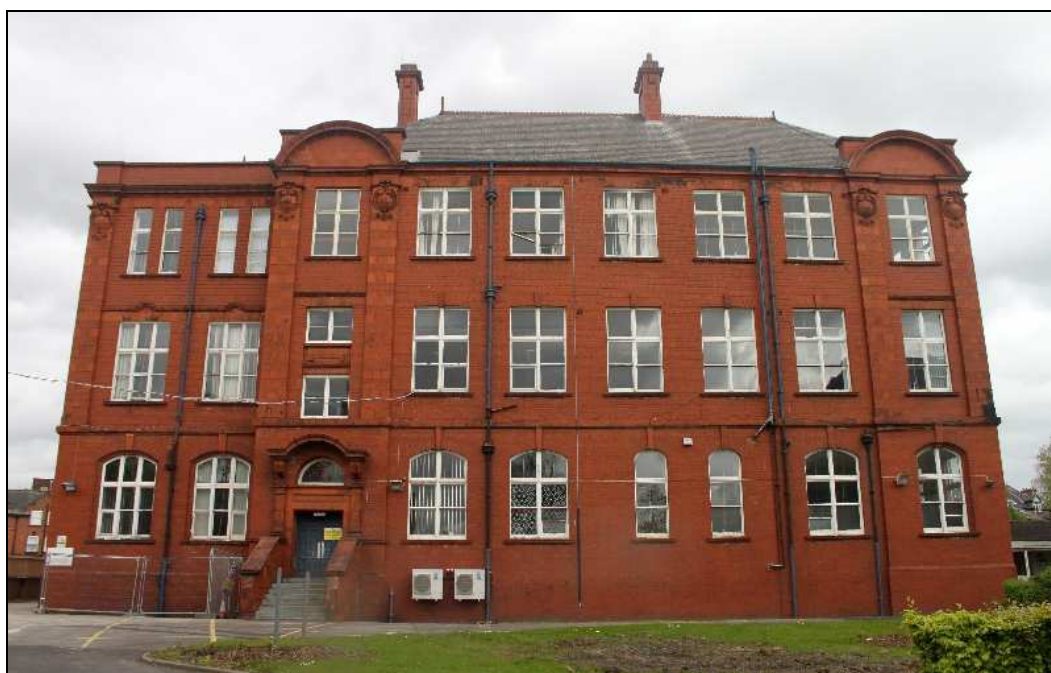
Plate 21: Western elevation of the South-Eastern Wing, ground-floor facing north-east
