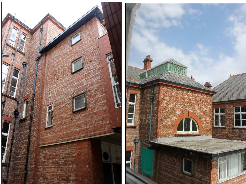
Plates 14 and 15: Stair tower with extension to right and privy tower to left. Southern elevation of Stair Tower in right hand frame, facing north-east
