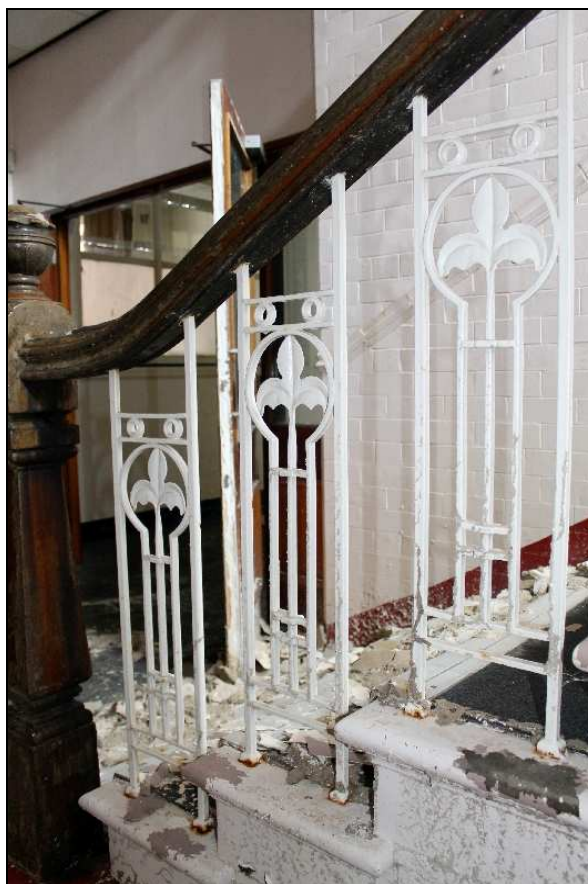
Plate 35: Wrought-iron staircase rails
