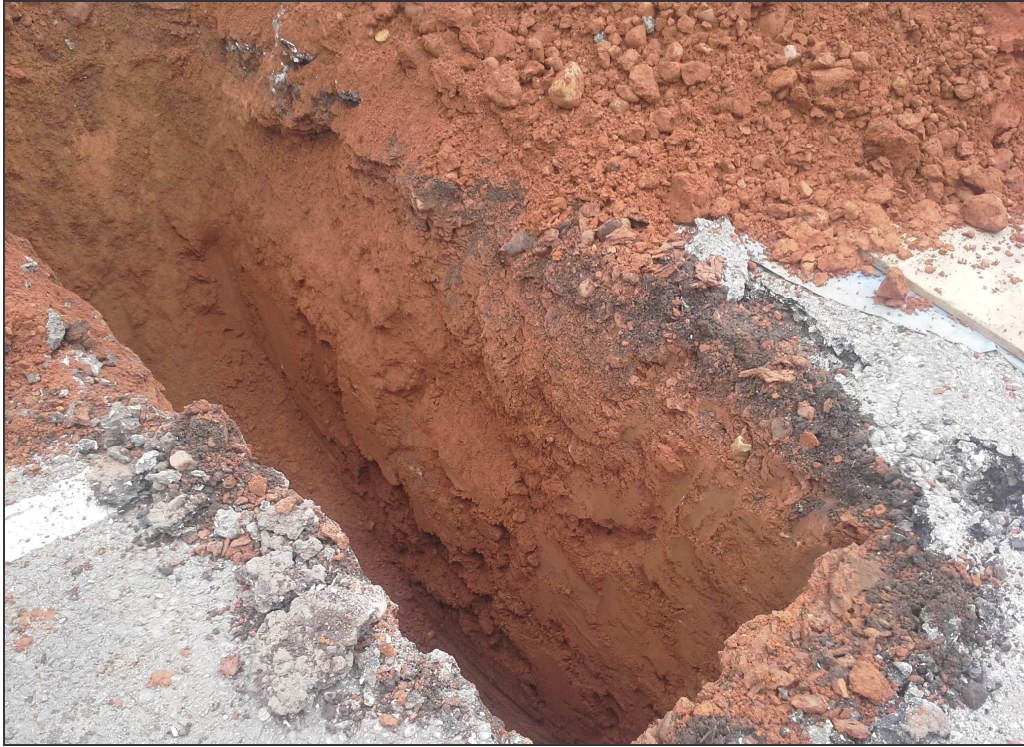
Plate 11: The natural geology exposed immediately beneath the modern surface in Trial Pit 204
