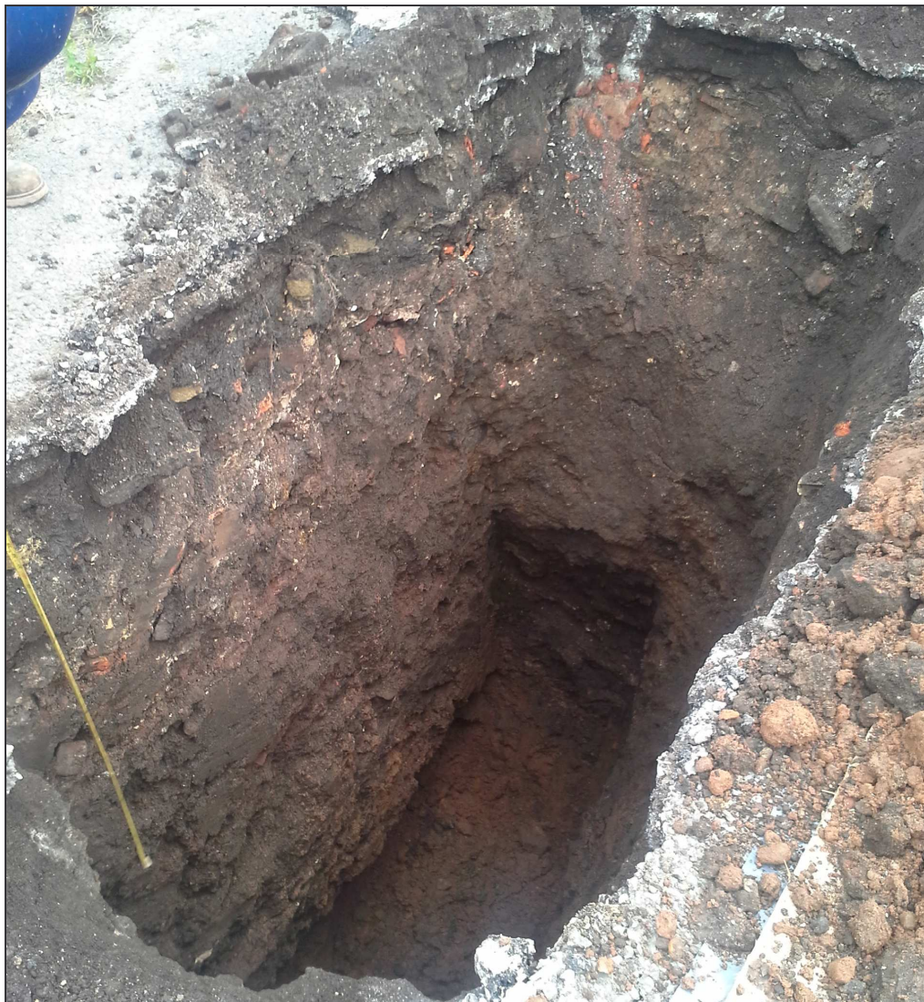
Plate 11: The natural geology exposed immediately beneath the modern surface in Trial Pit 203
