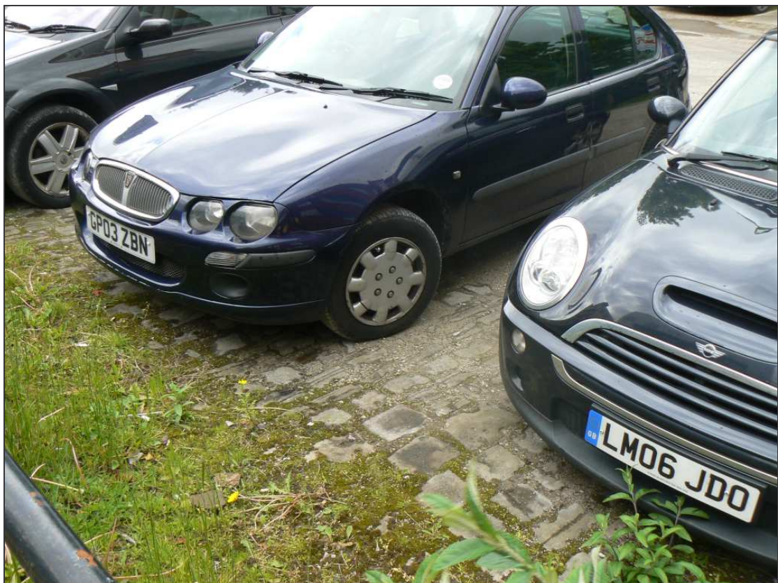
Plate 11: Historic surfacing of Back Old Mount Street surviving in the modern car park
