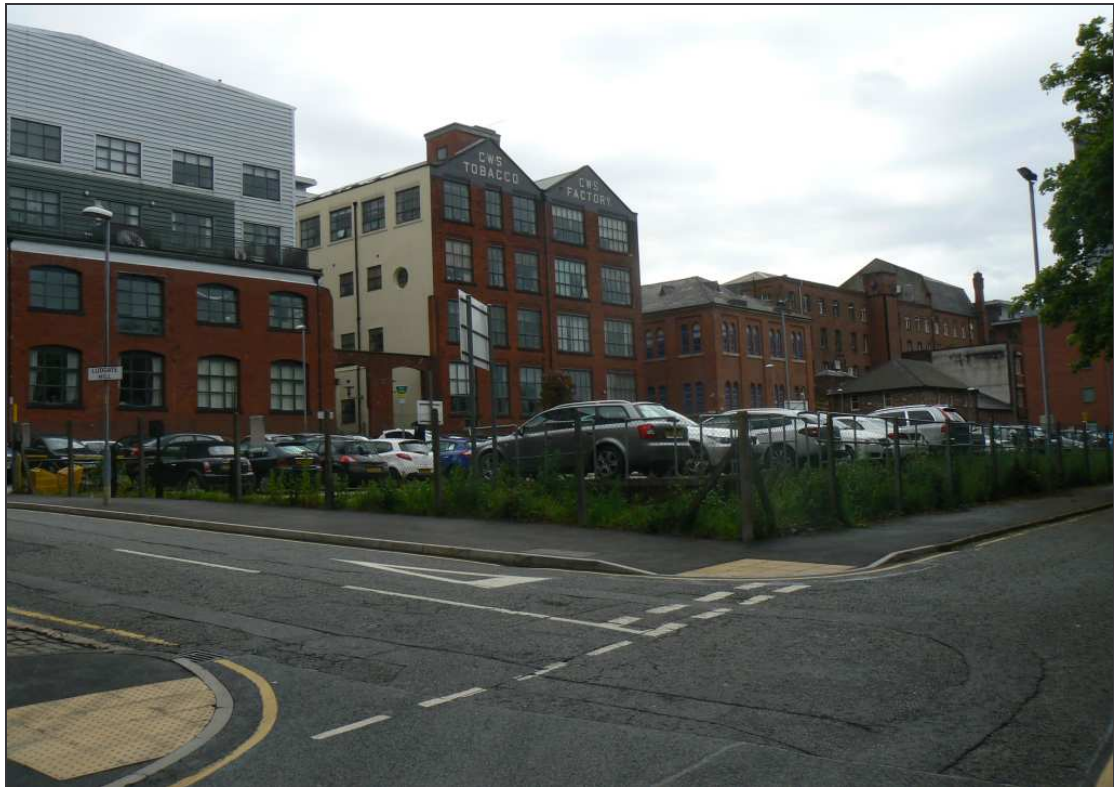
Plate 10: General view of the Site Area from the north-west
