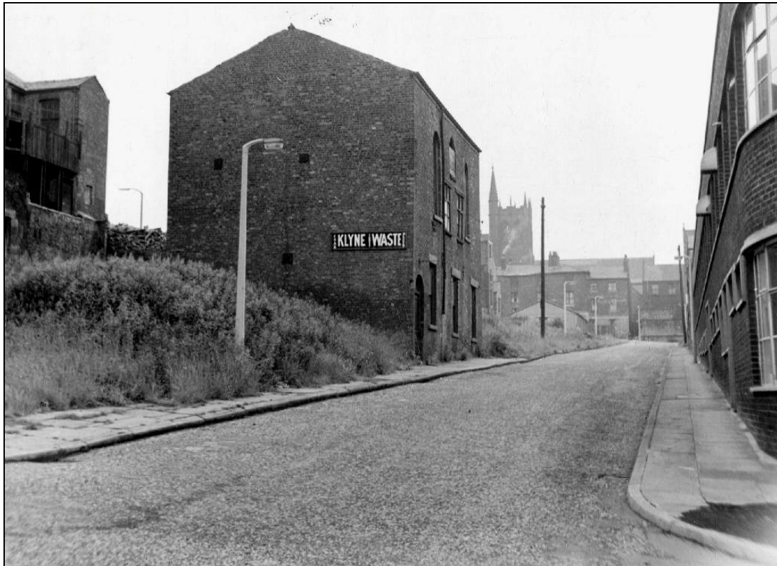
Plate 7: View along Fernie Street in the mid-1960s, showing the former synagogue (Site 07) and the rear part of the buildings fronting onto Cheetham Hill Road (Site 08)
