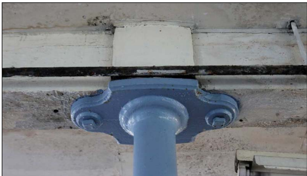
Plate 23: Detail of Type 2A column head without the lineshaft bolting face
