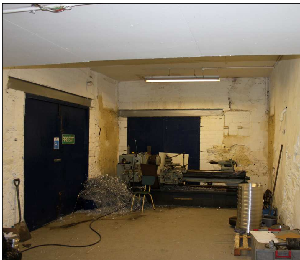
Plate 34: Interior of the engine house at ground-floor level
