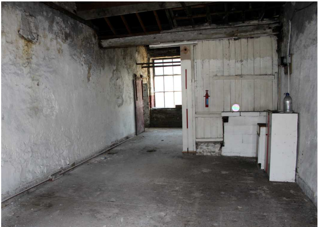
Plate 40: The second floor of the engine house, looking towards the western wall, showing central bearing box set into the south wall
