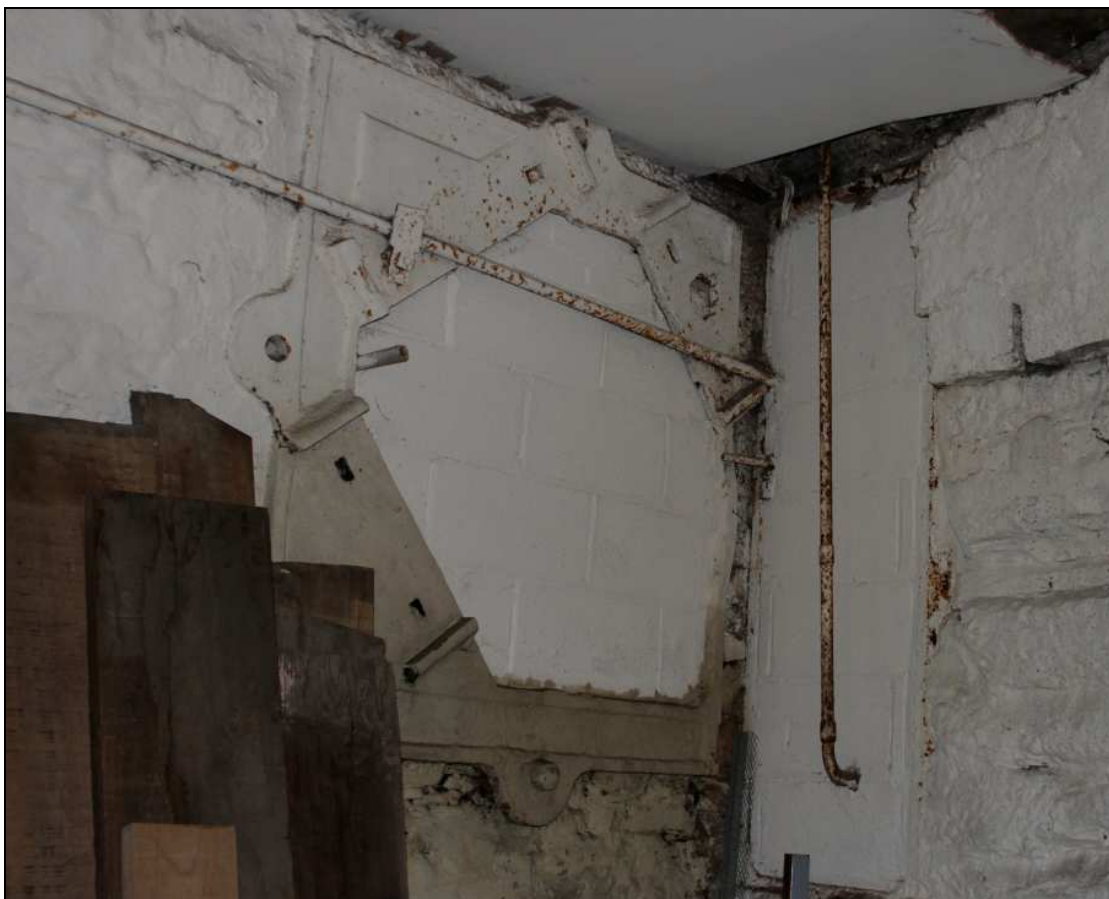
Plate 46: Substantial bearing box set into the north wall of the boiler house/warehouse
