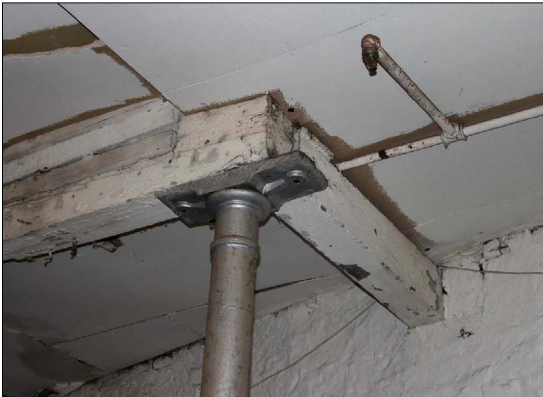
Plate 44: Column (Type 5) inserted to support remodelled joists
