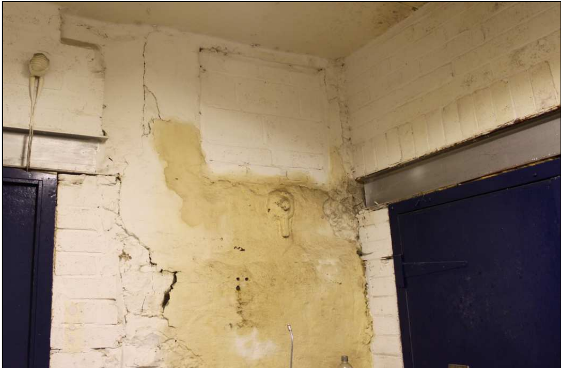
Plate 35: Bearing box situated in the north-eastern corner of the engine house, carrying the main drive shaft into the spinning block
