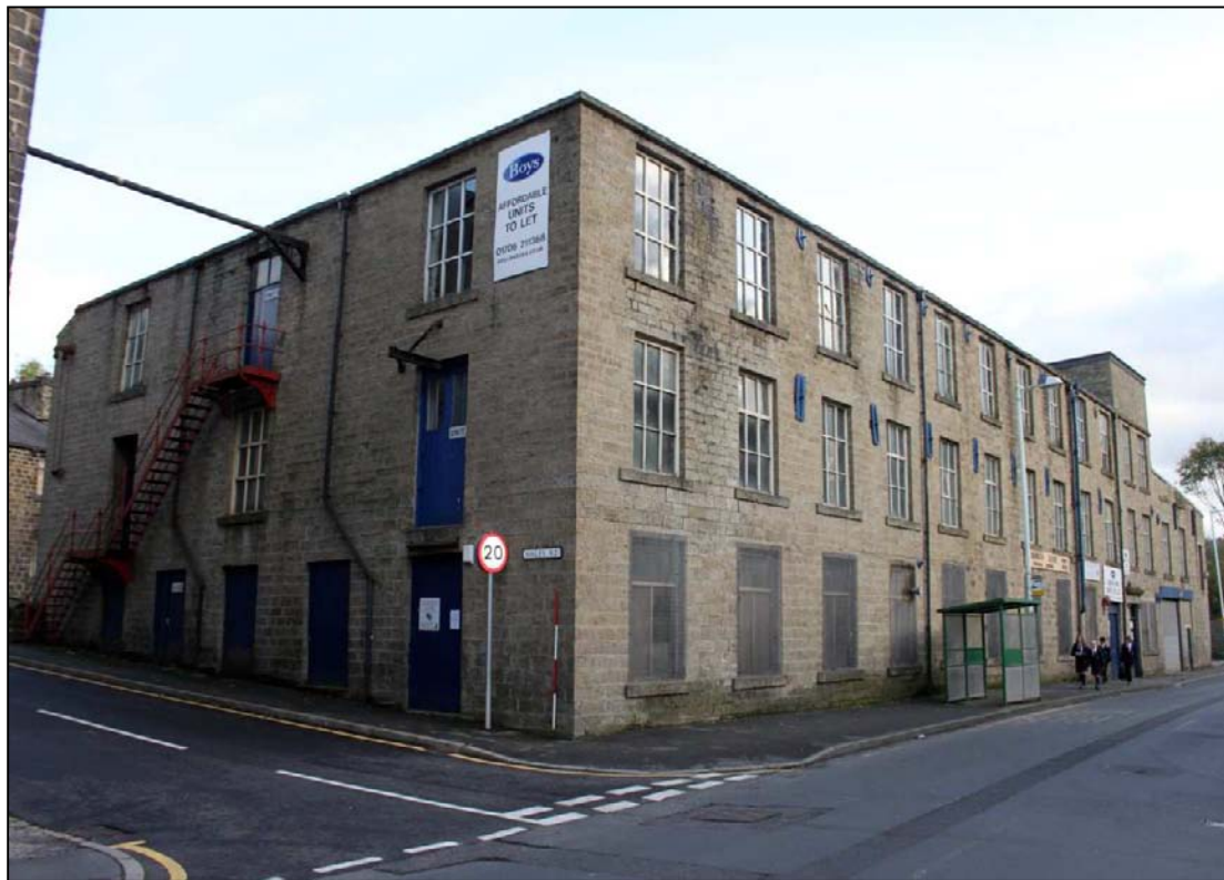
Plate 7: The western and northern elevations of Albion Mill, looking south-east
