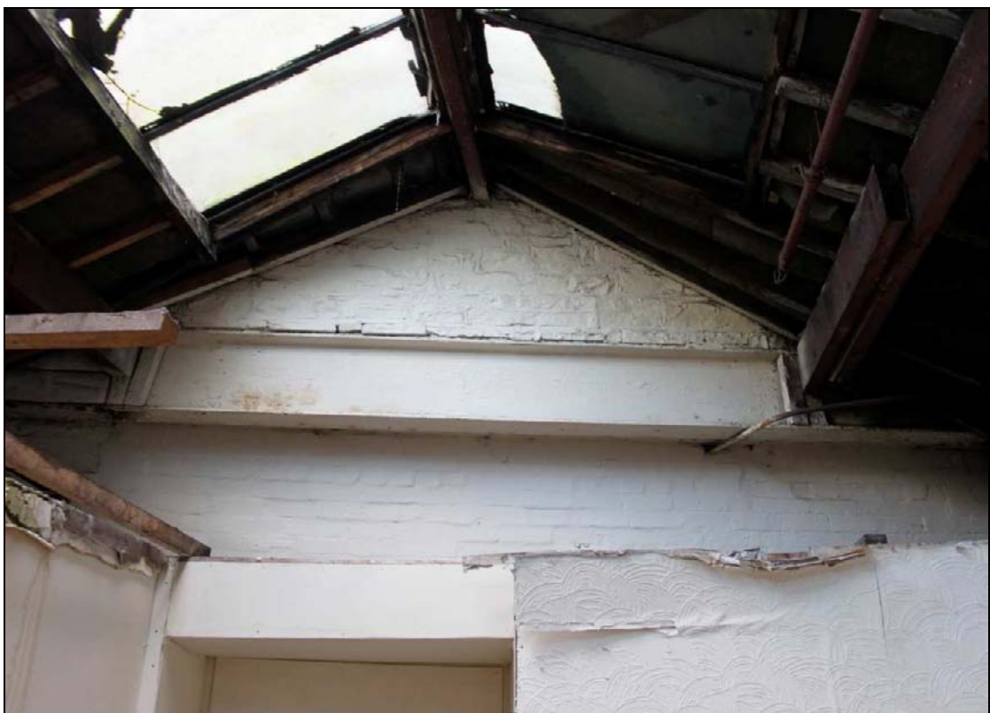
Plate 54: Detail of the steel lintel against the southern wall of the link block
