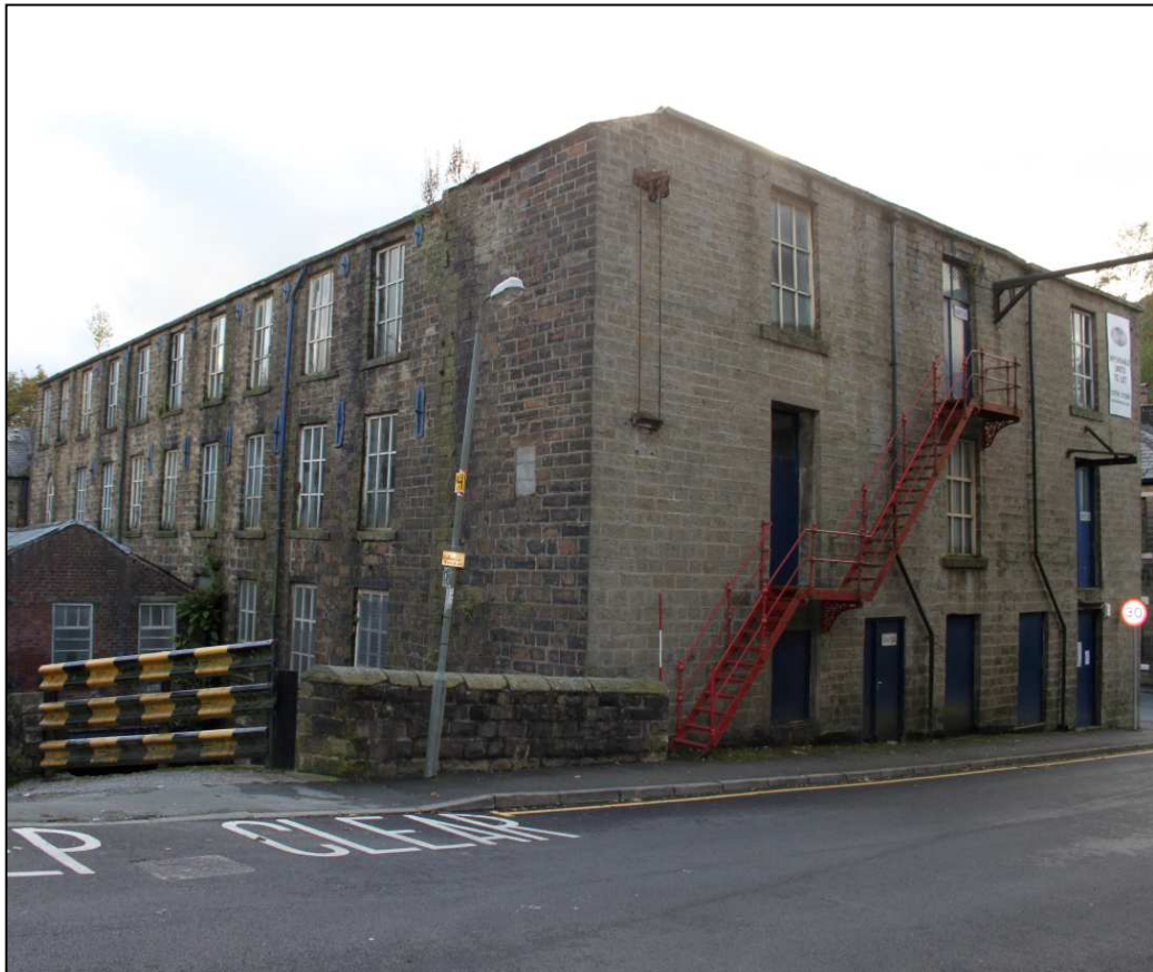
Plate 10: The northern and eastern elevations of Albion Mill, showing the iron fire-escape stair to Wales Road, looking south-west
