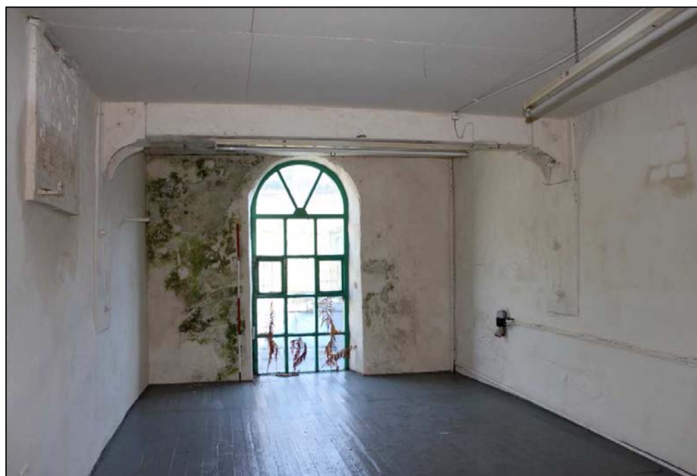
Plate 37: The first floor of the engine house
