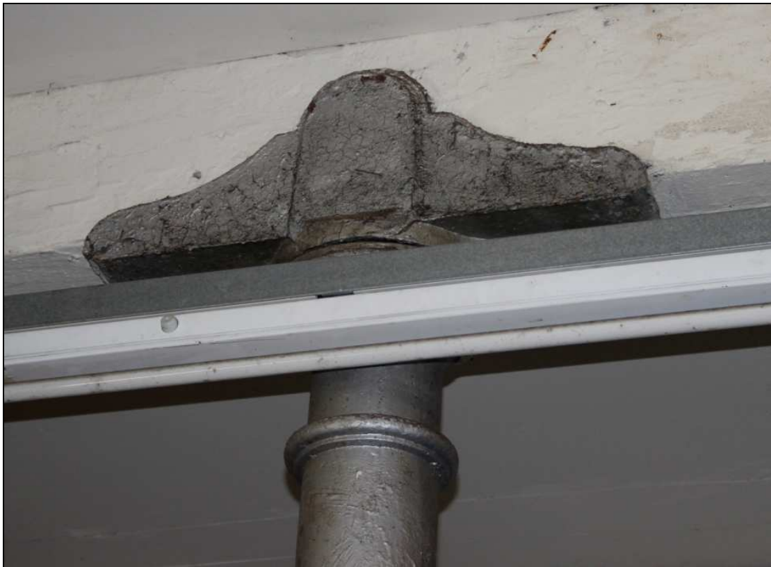
Plate 45: Column (Type 6) incorporating a crush box in its casting
