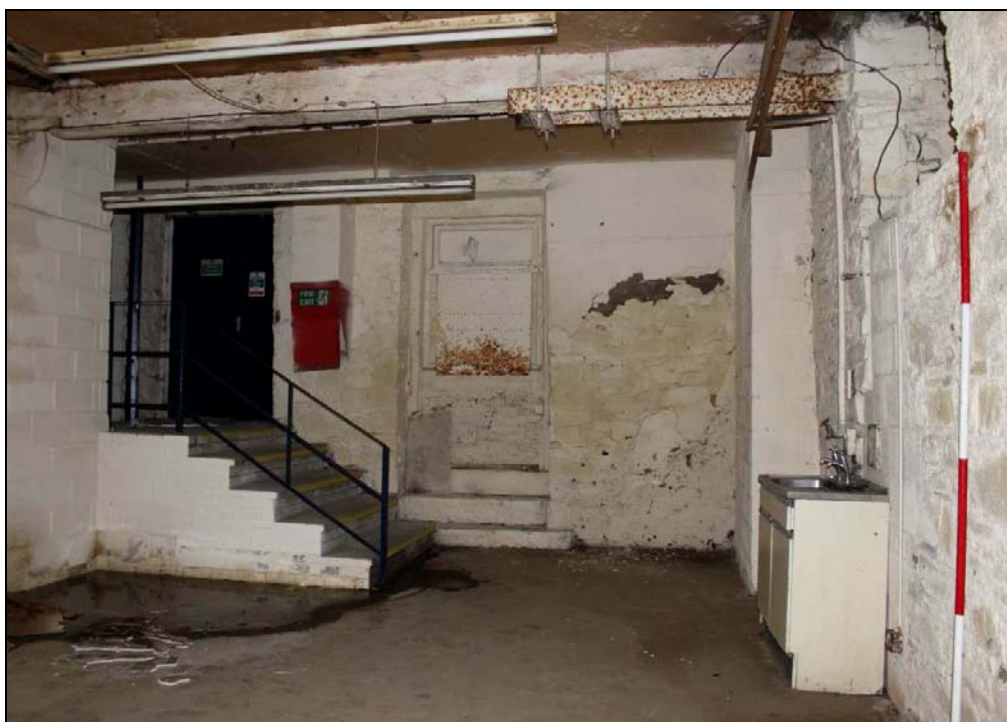
Plate 19: Original and replacement access steps from the ground floor to Wales Road
