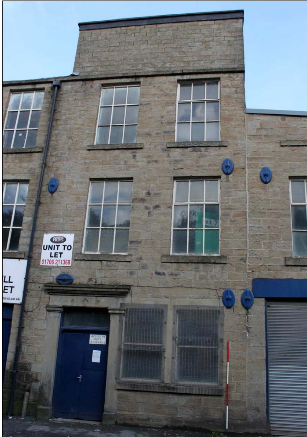
Plate 32: The west-facing elevation of the engine house
