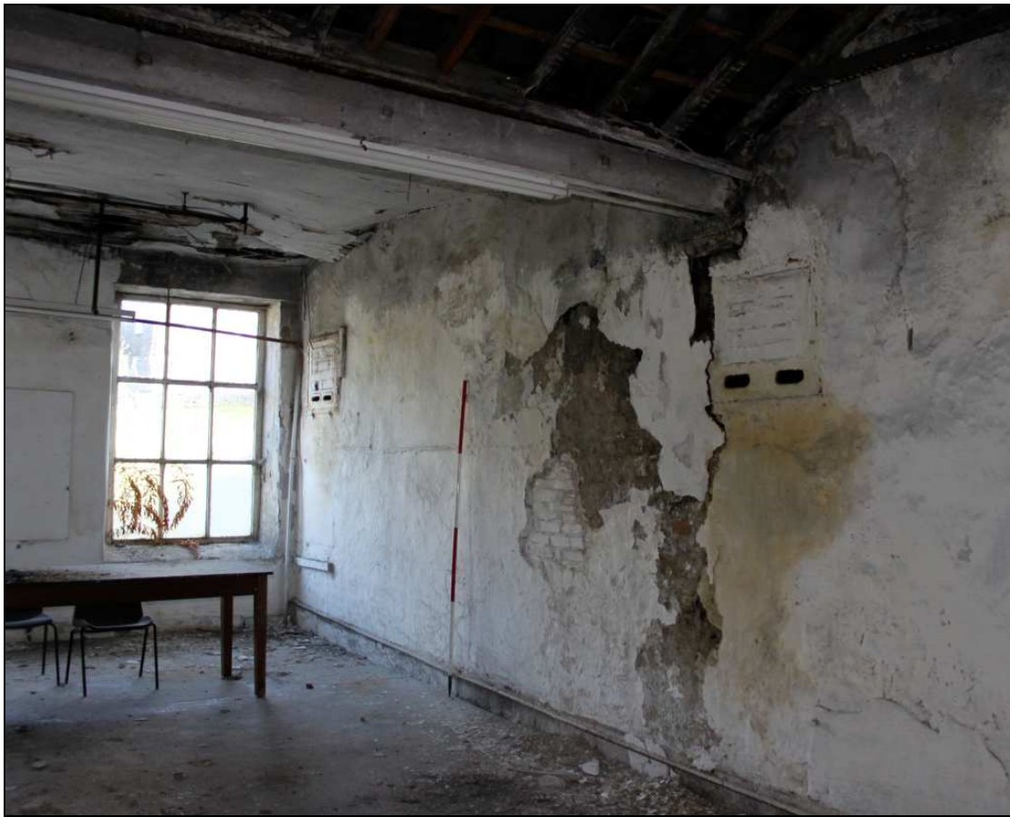
Plate 39: The second floor of the engine house, showing bearing boxes set into the south wall
