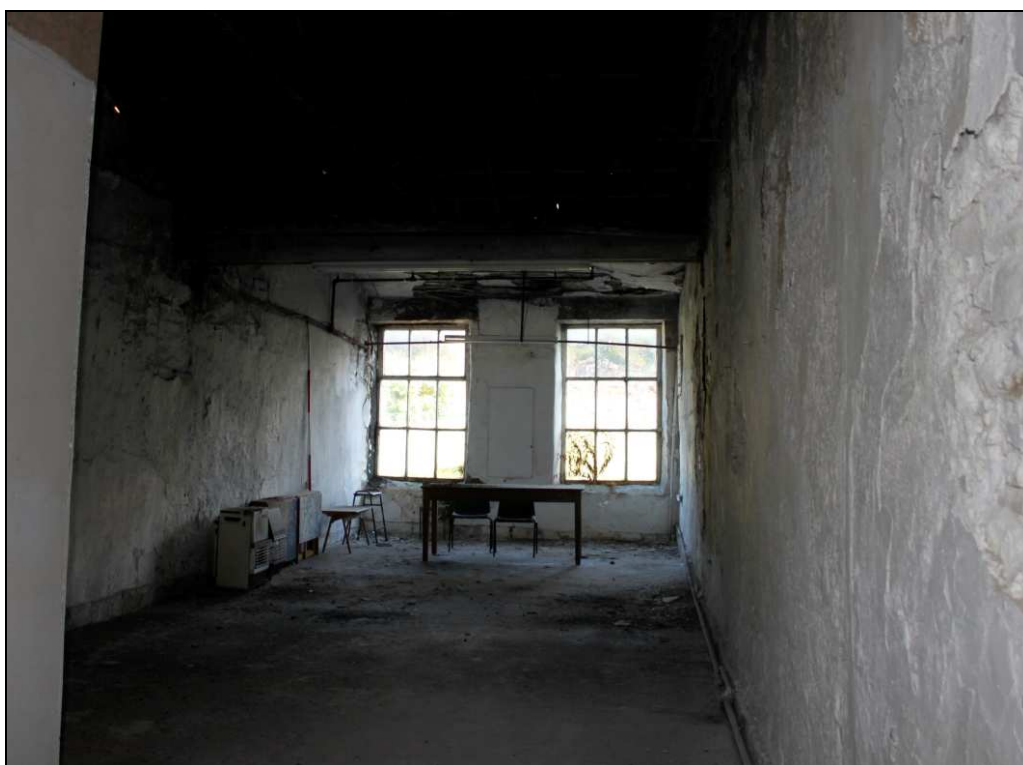
Plate 38: The second floor of the engine house, looking towards the eastern wall
