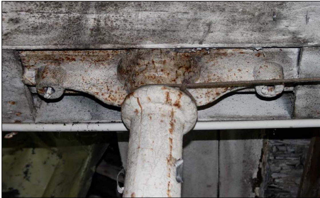
Plate 29: Detail of the Type 1B column capital
