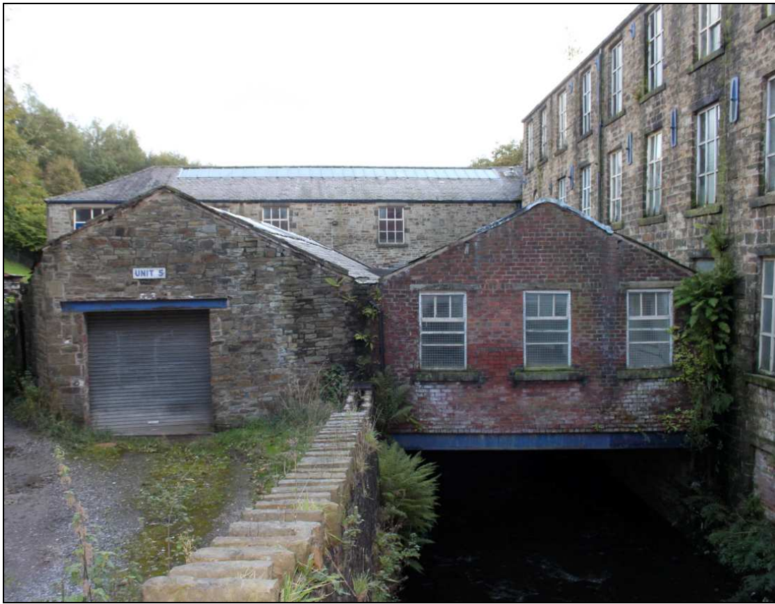
Plate 51: The north elevation of the link block, spanning the Whitewell Brook
