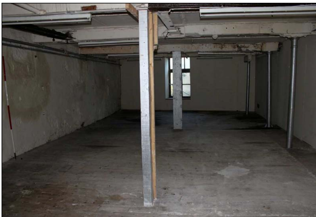
Plate 47: View across the first floor of the boiler house/warehouse
