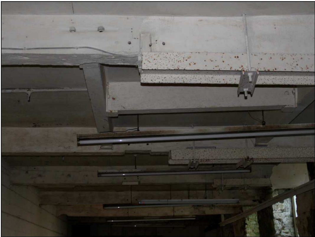
Plate 17: Bolt holts in the beam marking position of a lineshaft
