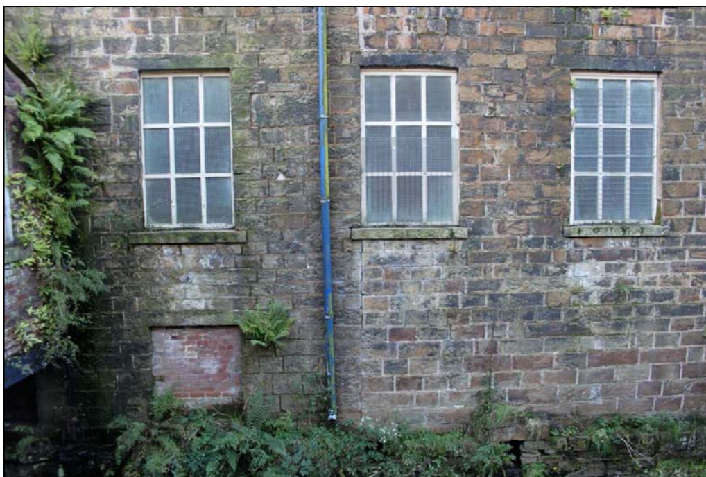
Plate 31: Blocked basement window in the eastern wall of the spinning block, also showing the construction break between Bays 4 and 5
