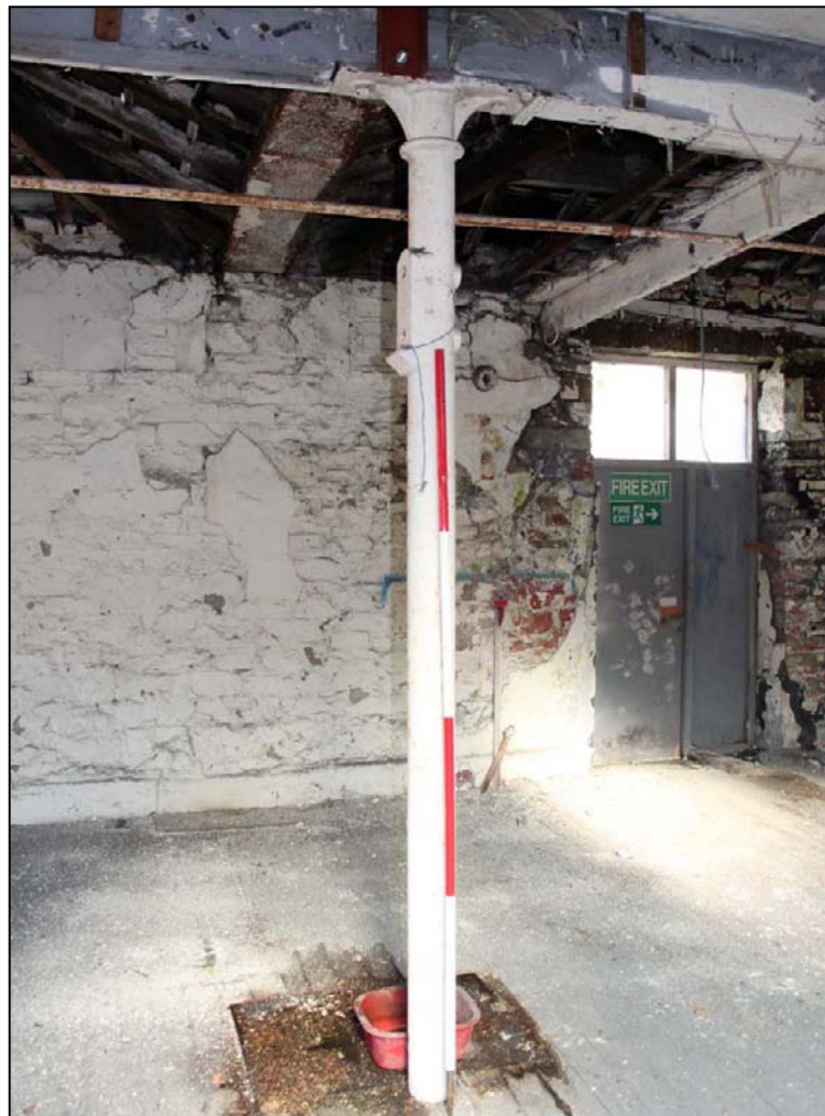
Plate 30: Type 4 column on the second floor of the spinning block
