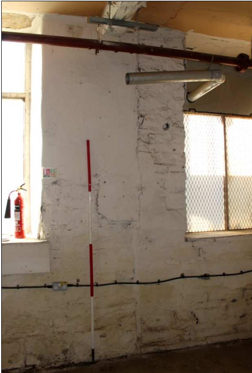
Plate 20: Butt joint in the east wall, denoting a construction break
