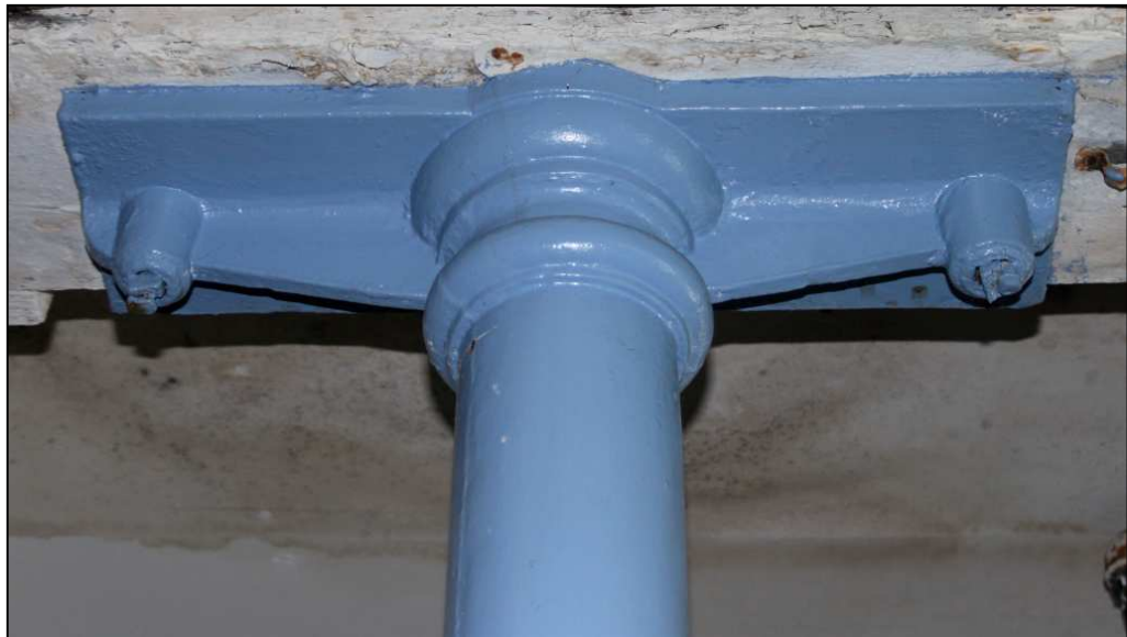
Plate 22: Detail of Type 1A column head without the lineshaft bolting face
