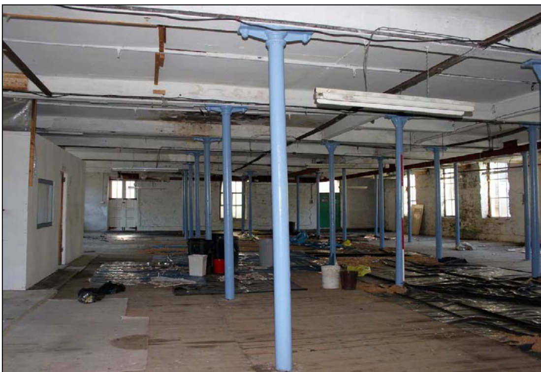
Plate 27: View north across the first floor, showing the two doors in the north elevation
