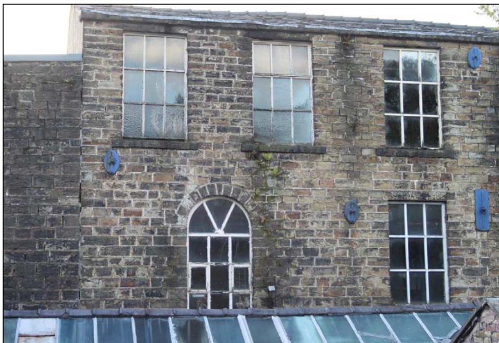
Plate 33: East-facing elevation of the engine house
