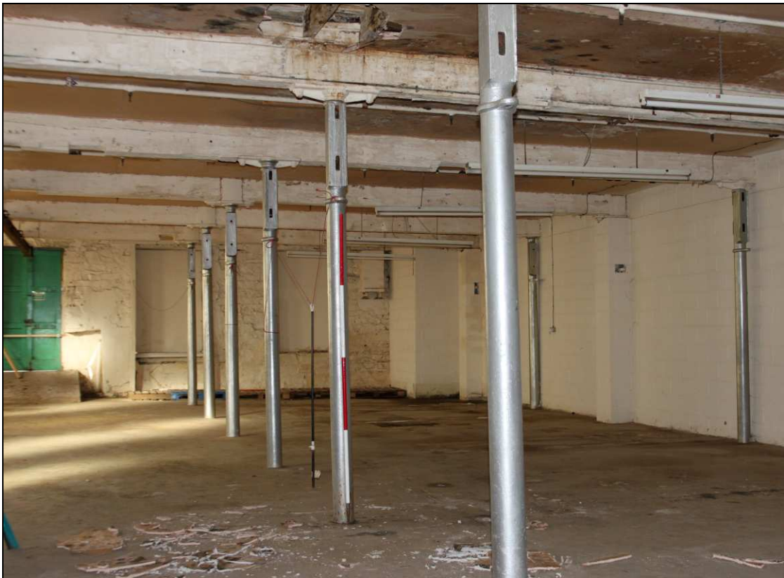
Plate 12: General view across the ground floor of the western part of the spinning block, showing two rows of columns and modern cinder-block partition
