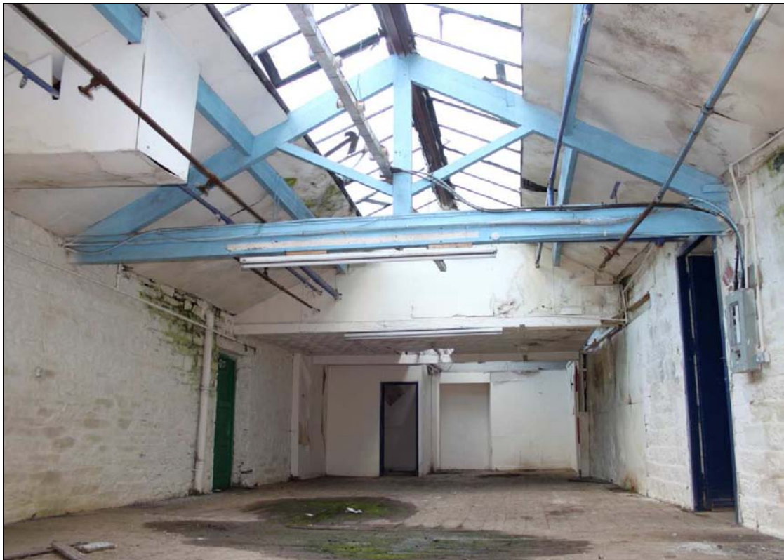
Plate 53: The interior of the southern part of the link block
