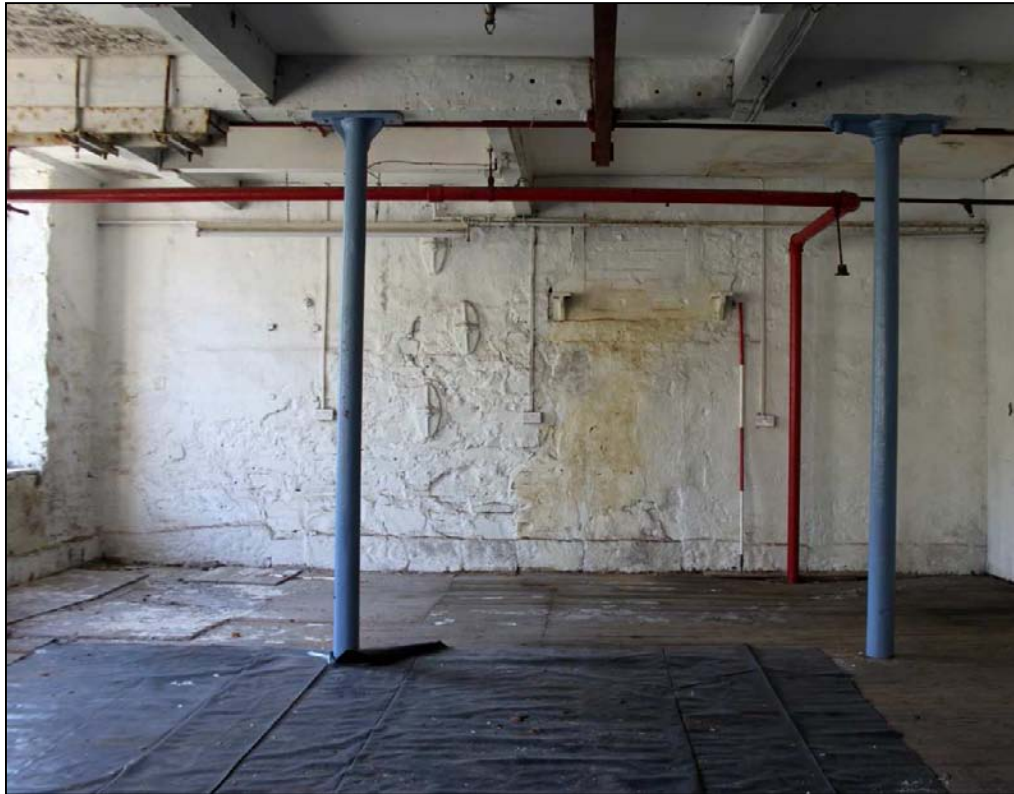
Plate 25: Large bearing box set into the south wall of the spinning block
