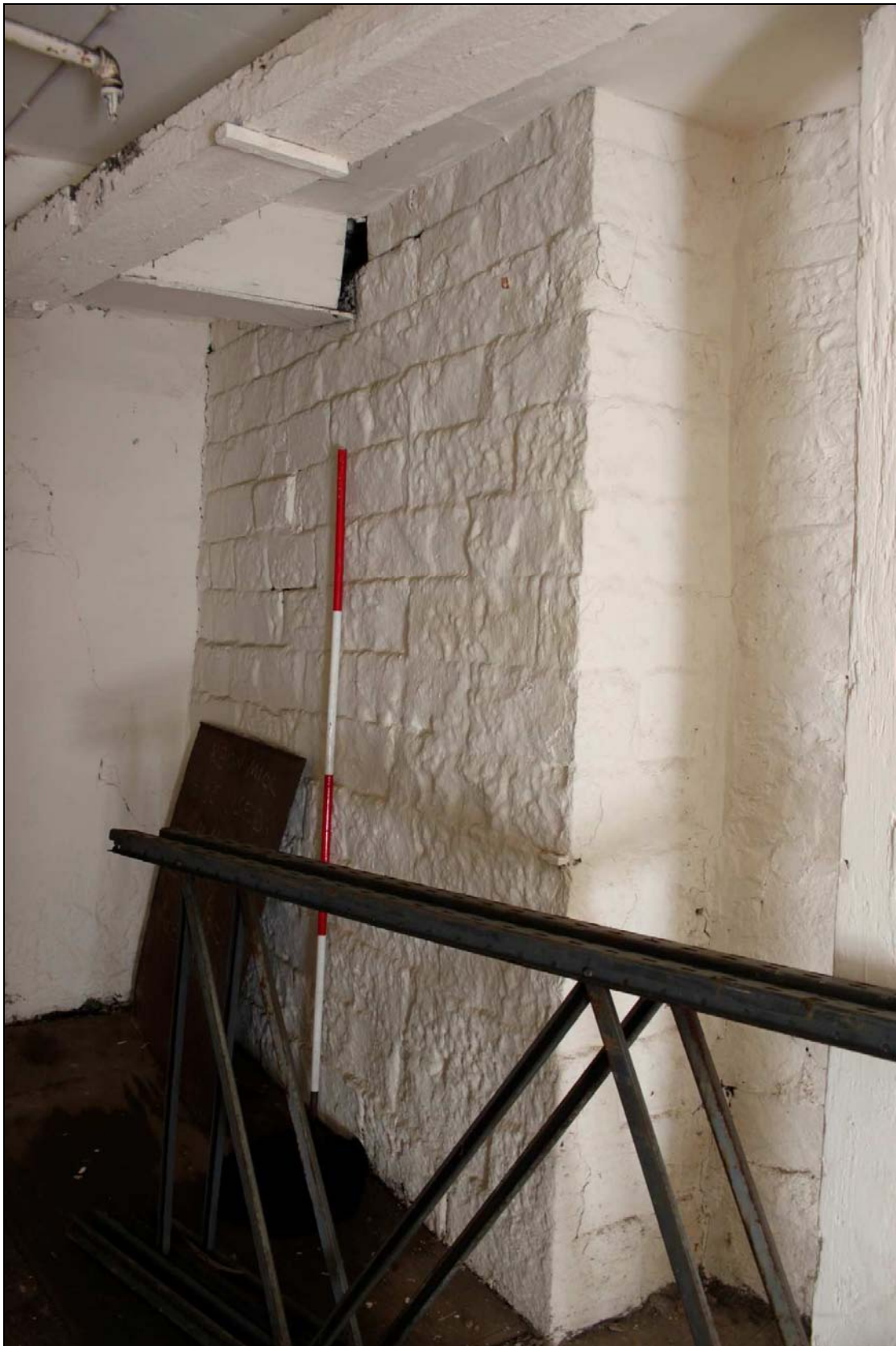
Plate 49: The chimney passing through the first floor of the boiler house/warehouse
