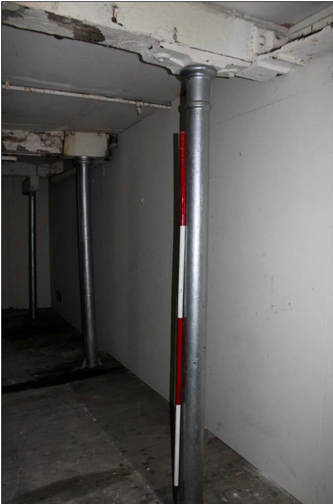
Plate 48: Detail of the columns on the first floor of the boiler house/warehouse
