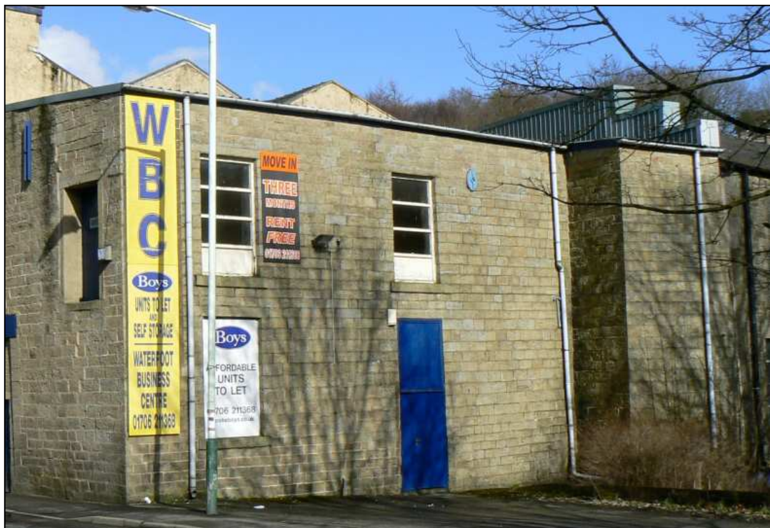
Plate 42: The south elevation of the boiler house/warehouse
