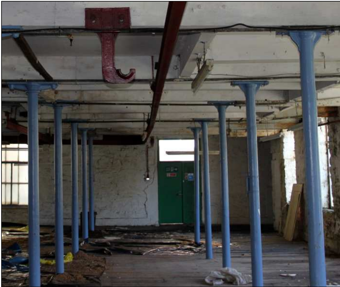
Plate 26: Surviving lineshaft hanger on the first floor of the spinning block
