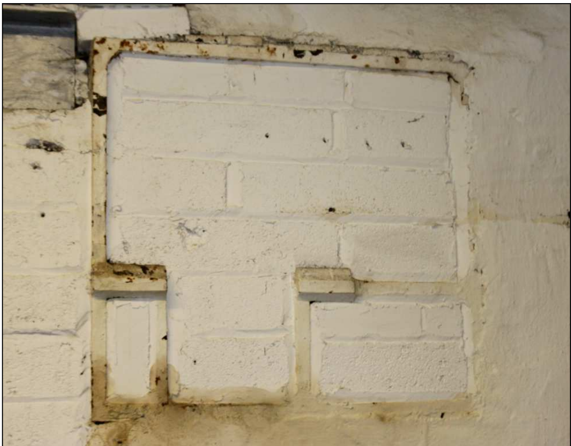
Plate 36: Bearing box in the eastern wall of the engine house
