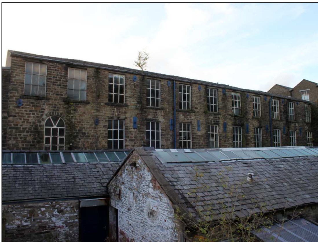
Plate 8: The eastern elevation of Albion Mill, showing the first and second floors rising above single-storey buildings to rear, with contiguous engine house at the southern end
