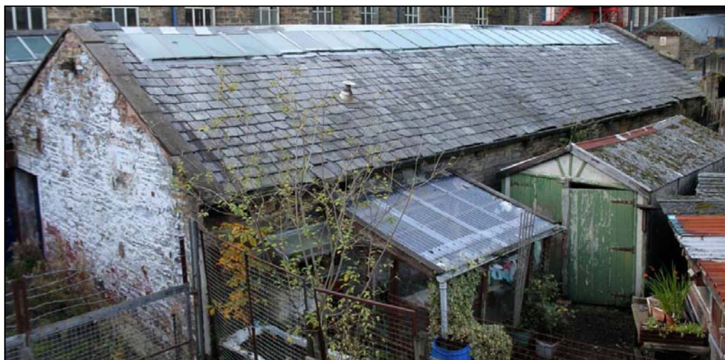
Plate 55: View across Unit 5, looking north-west
