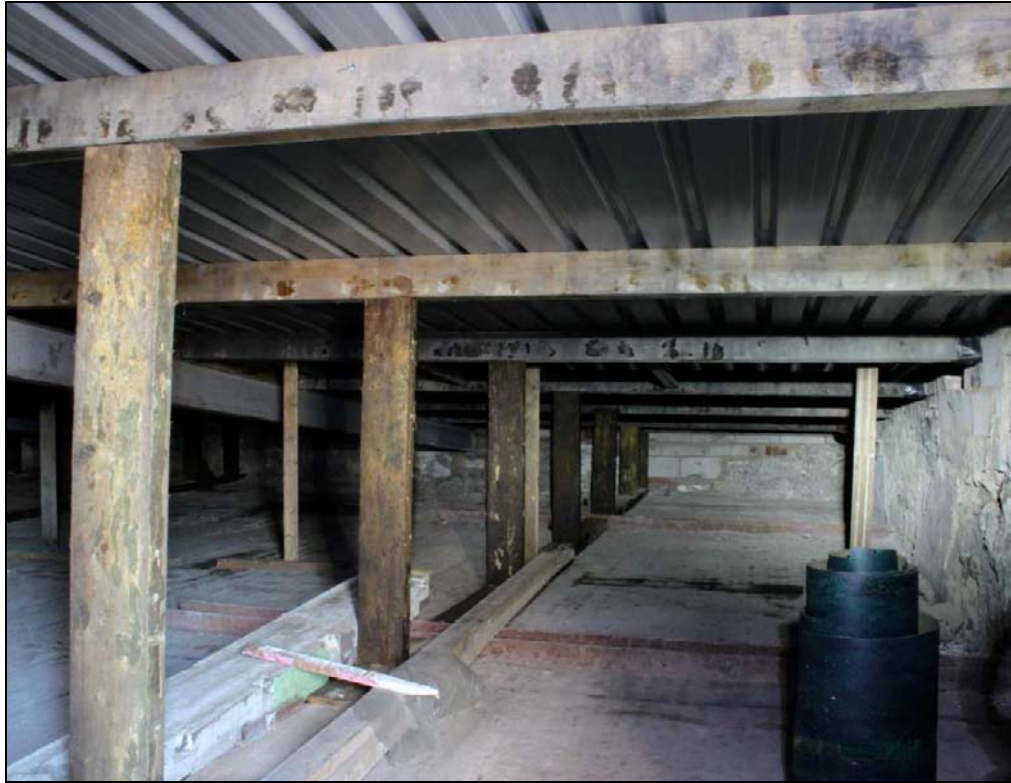
Plate 50: The modern roof space in the boiler house/warehouse
