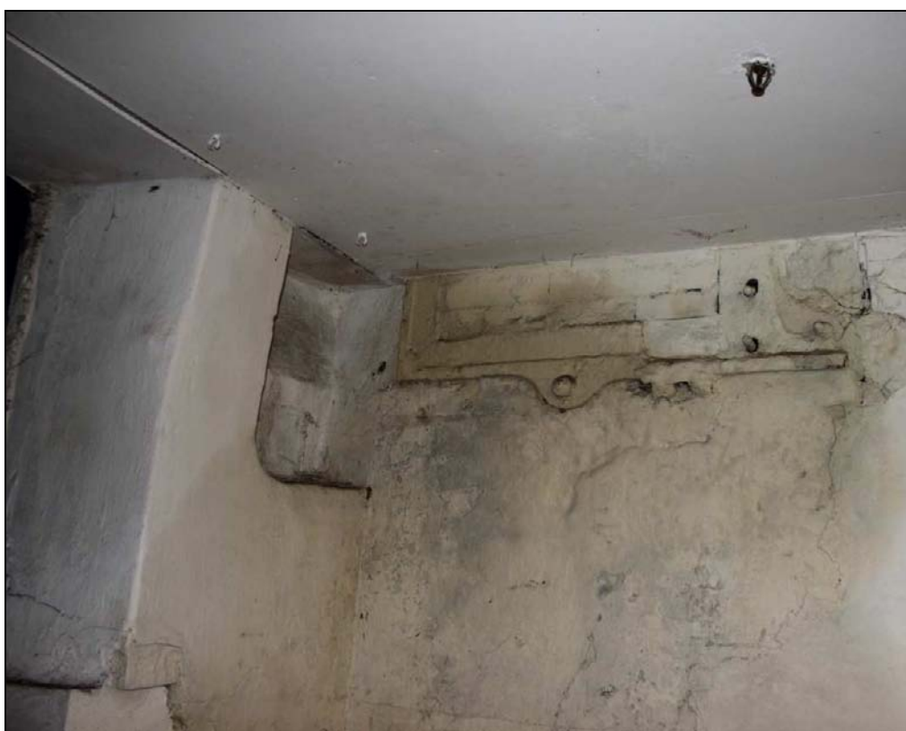
Plate 16: Bearing box set into the eastern end of the wall dividing the spinning block from the engine house, together with a cut-out in the eastern wall for bevel gearing.
