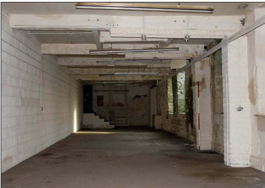
Plate 13: General view across the ground floor of the eastern part of the spinning block, showing the concrete floor and the late cinder-block partition
