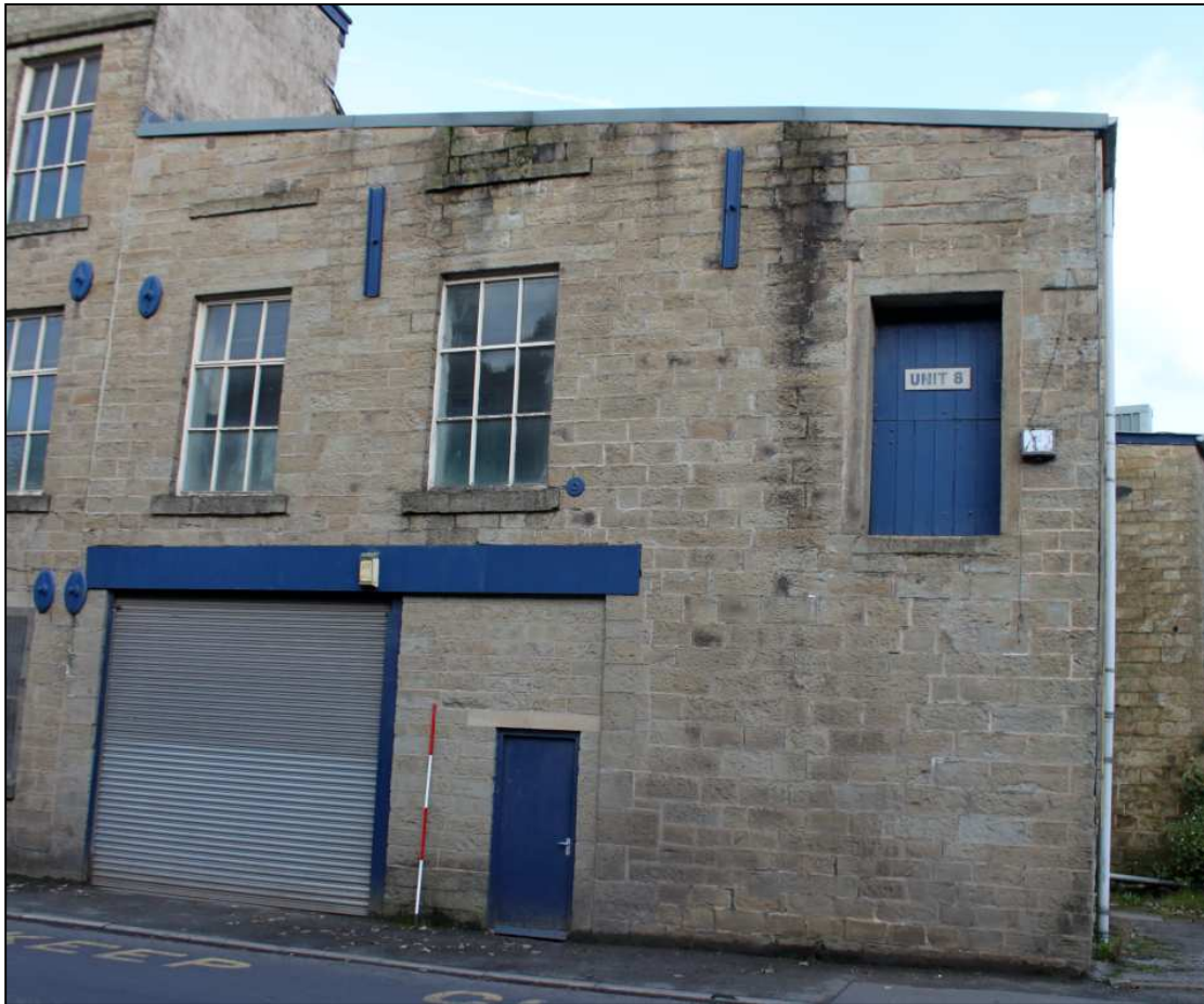
Plate 41: The front elevation of the boiler house/warehouse
