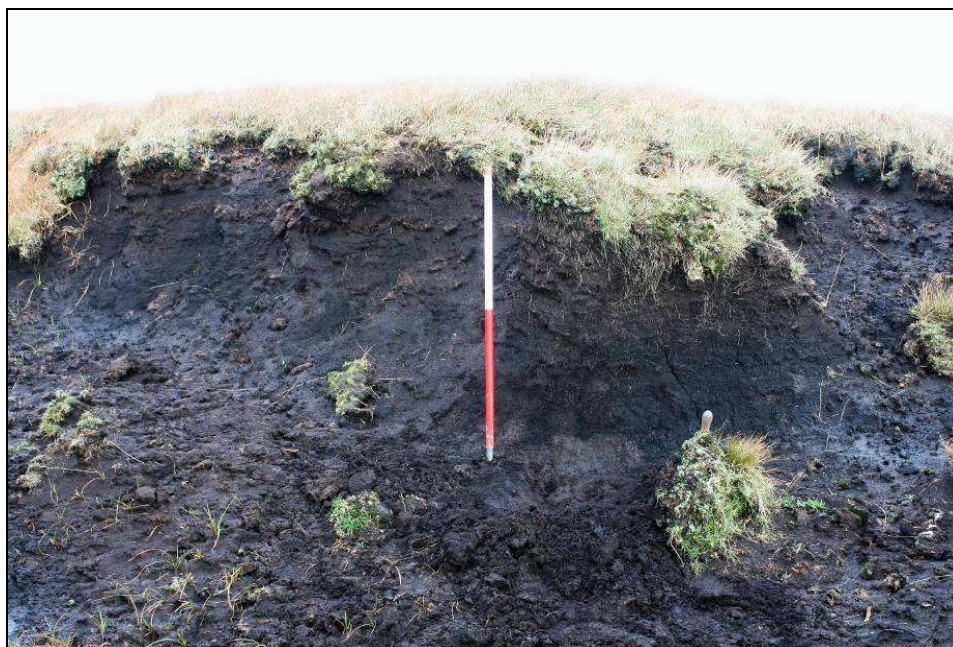
Plate 26: A section of exposed peat >1m thick, showing cascaded peat hags, located near West Weather Syke on Simon Fell (Site E4)
