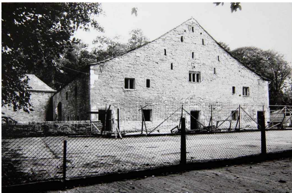
Plate 7: Photograph of the northern elevation of the barn taken in 1984. The three windows visible on the plan of 1981 have already been blocked
