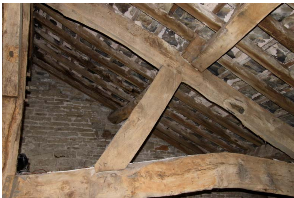
Plate 52: Example of assembly marks on the truss assemblies
