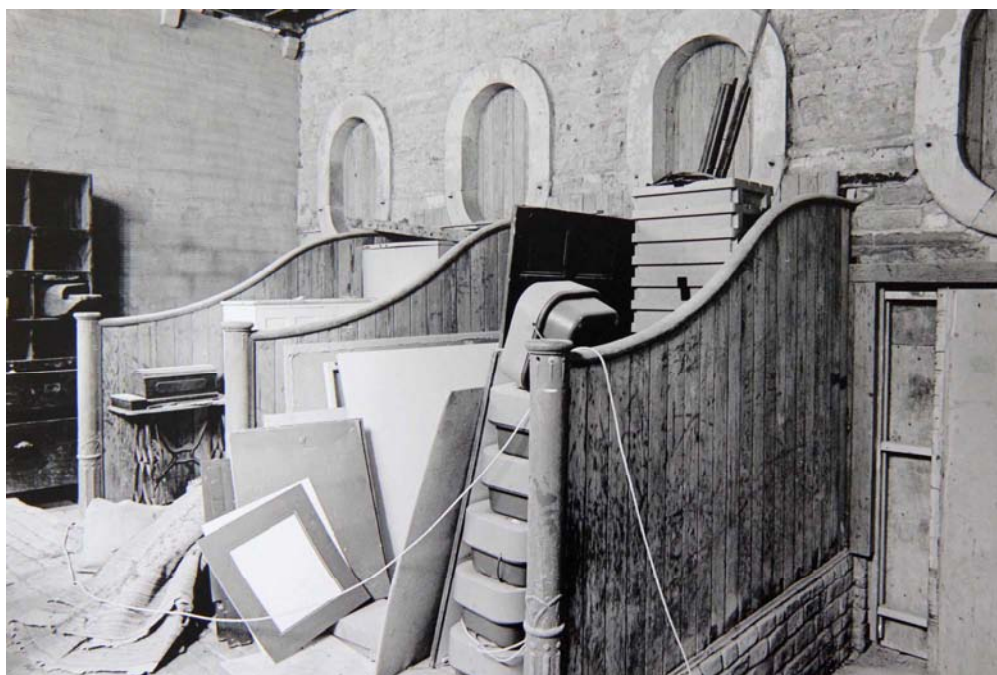
Plate 16: the central stable circa 1987 at the southern end of the barn facing north west. The eastern connecting door is visible to the right
