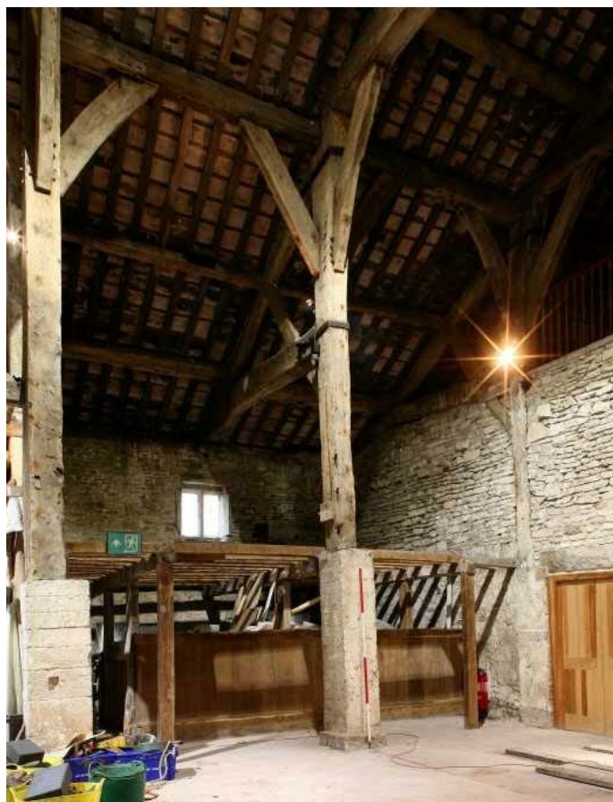
Plate 47: Example of an arcade post
