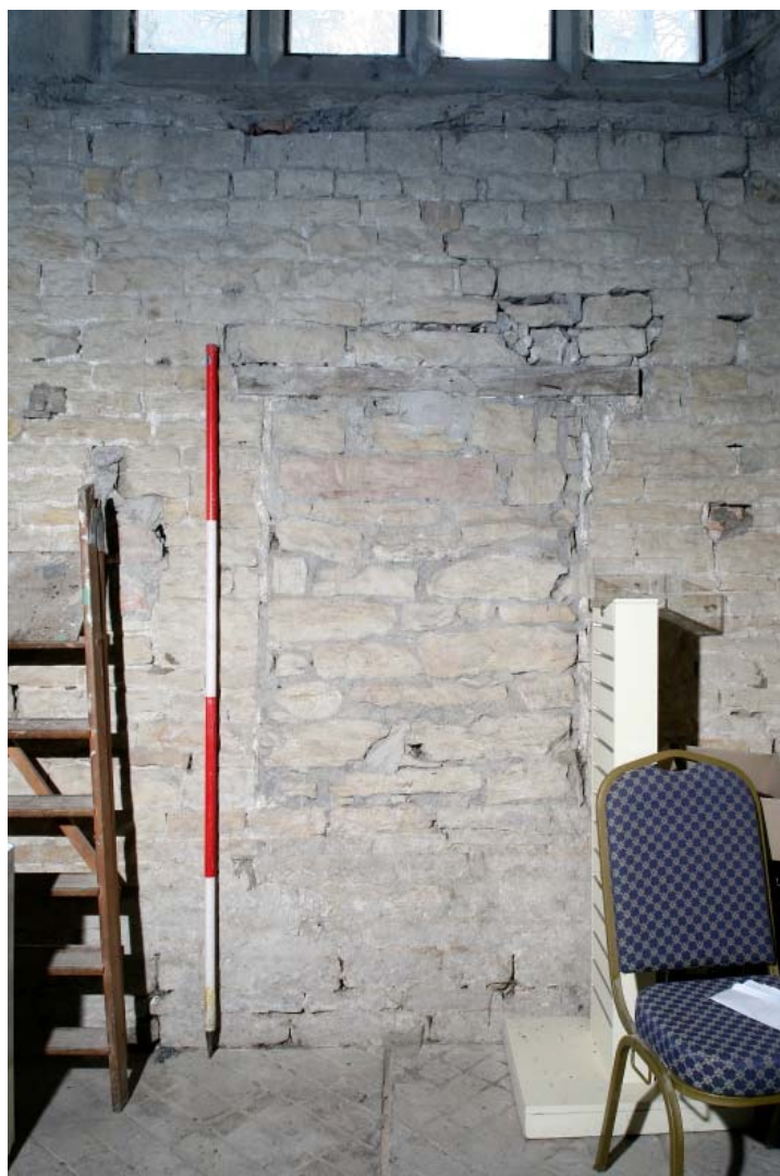
Plate 41: Blocked aperture to the right of the main door on the internal aspect of the south wall of the main barn within Room 1
