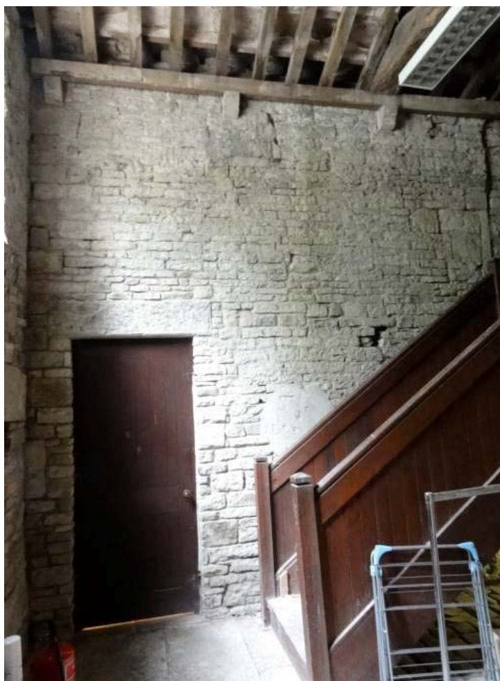
Plate 5: The southern end of the western wall of the Great Barn, looking west. The character of the wall suggests it is probably original, as does the blocked opening just visible above the stairs, near the top of the wall
