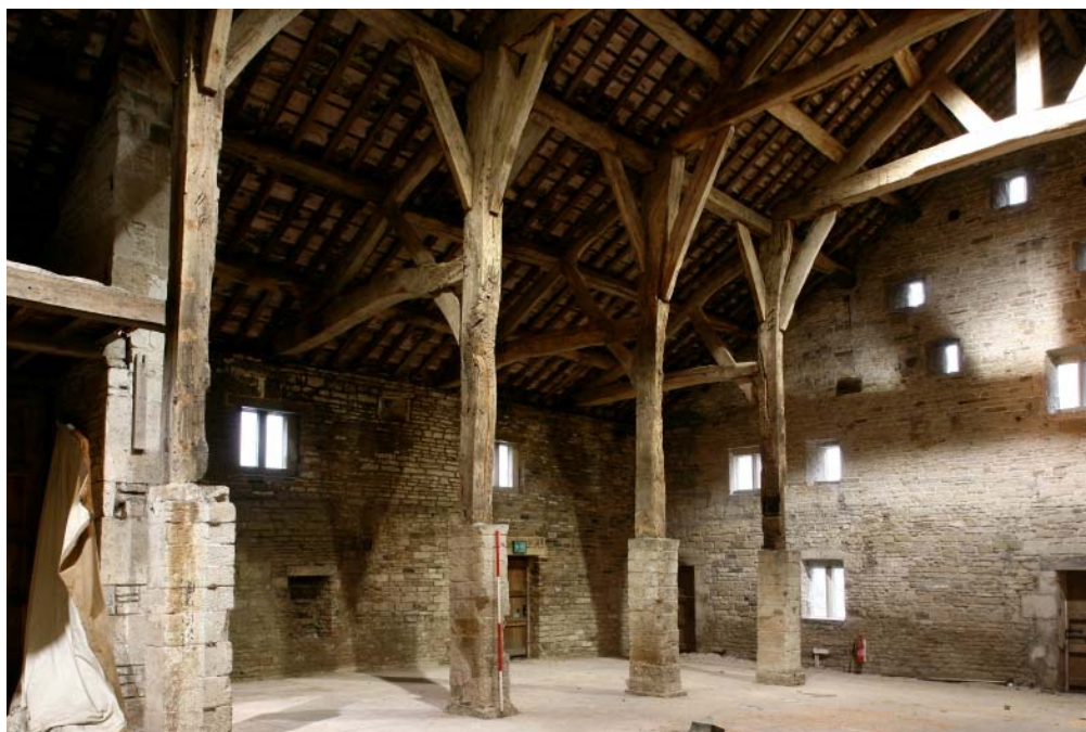
Plate 48: Side aisle on the west side of the barn
