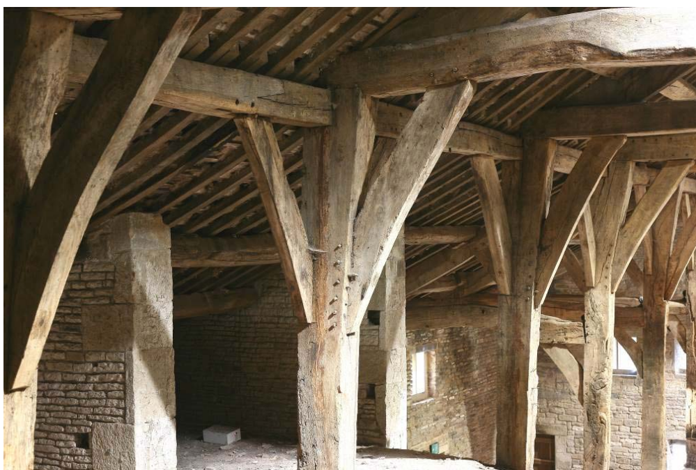
Plate 51: Example of the bracing at the junction of truss, aisle plate and aisle post
