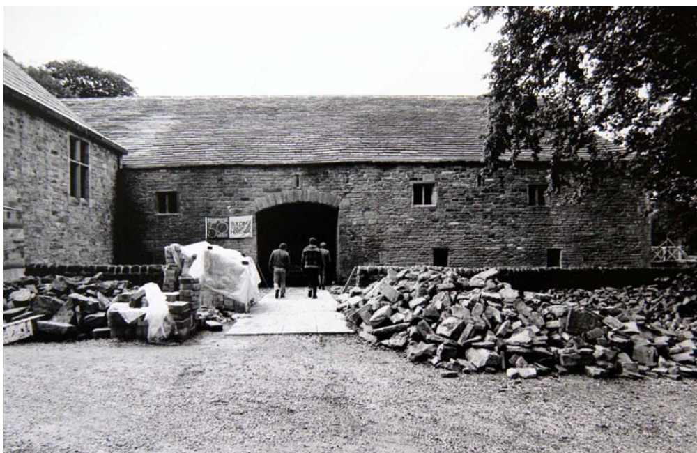
Plate 12: The eastern elevation of the barn taken in 1984. The three ground floor windows visible in the plan of 1981 have been blocked but the two remaining windows have not yet been widened and refurbished
