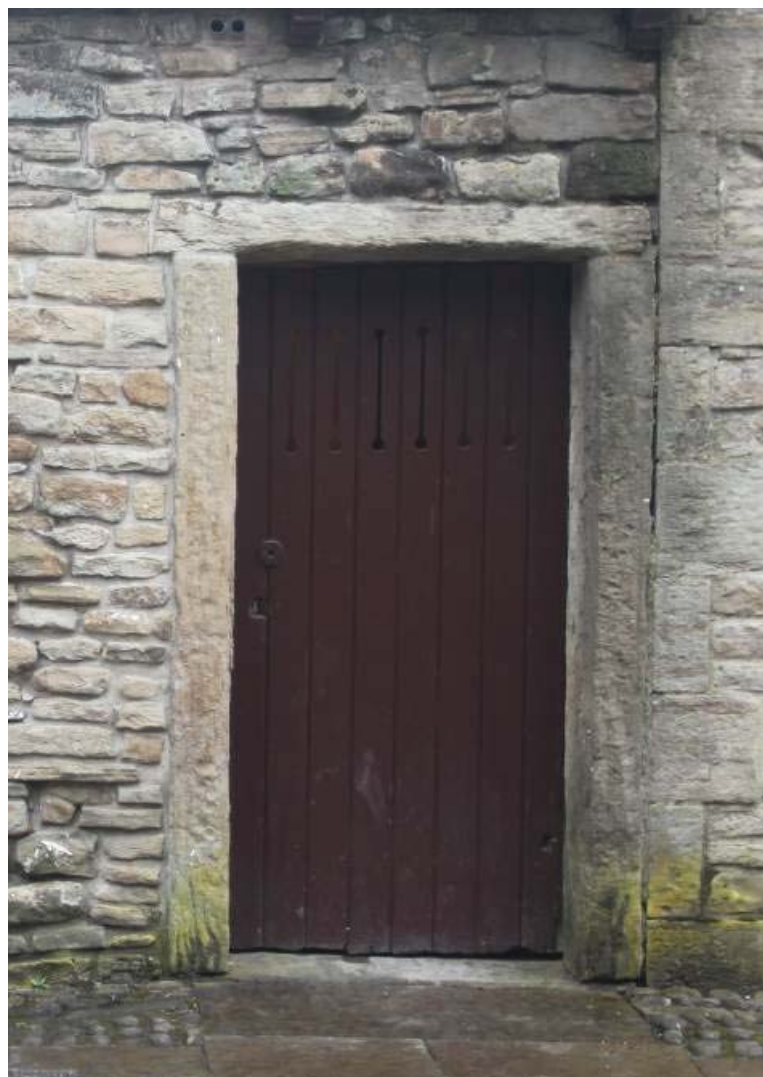
Plate 28: Door on southern elevation of store/toilet block, with ventilation slits set into the upper half
