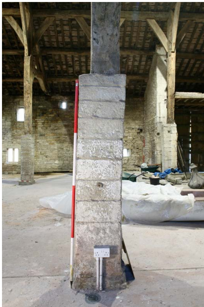
Plate 49: Example of a stone plinth supporting an arcade post showing the wooden peg
