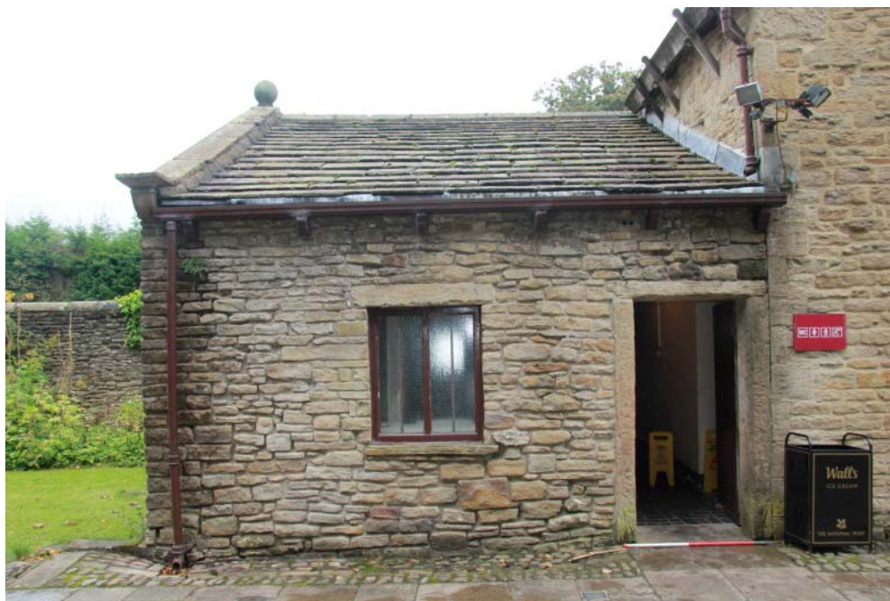
Plate 27: The south elevation of the toilet wing
