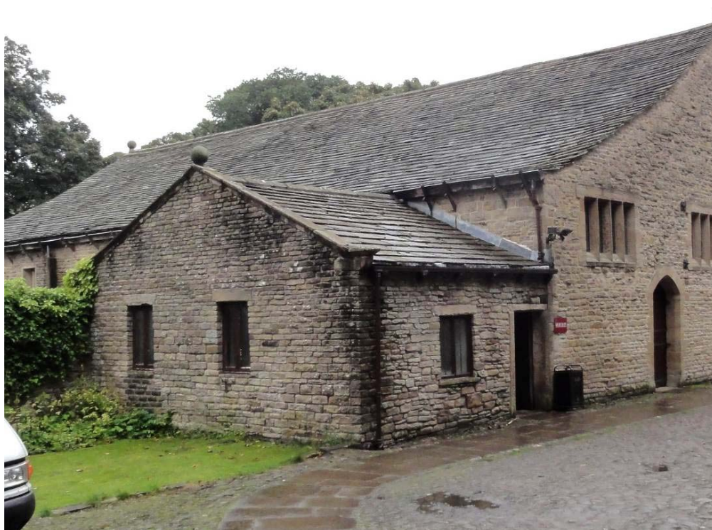
Plate 36: Gable elevation of the toilet extension
