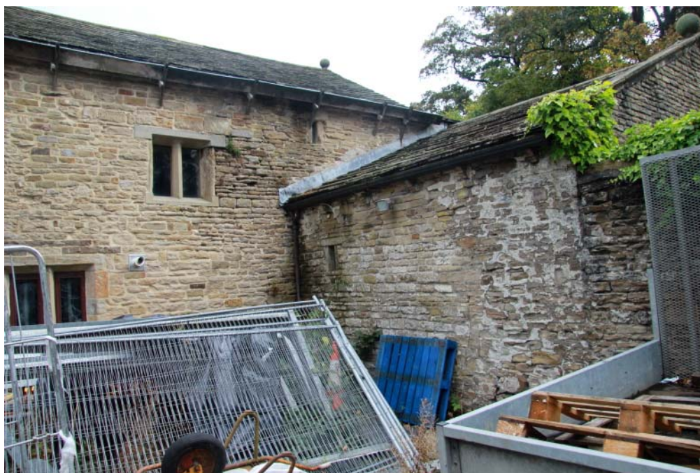
Plate 35: Join between the toilet extension and the west elevation of the barn
