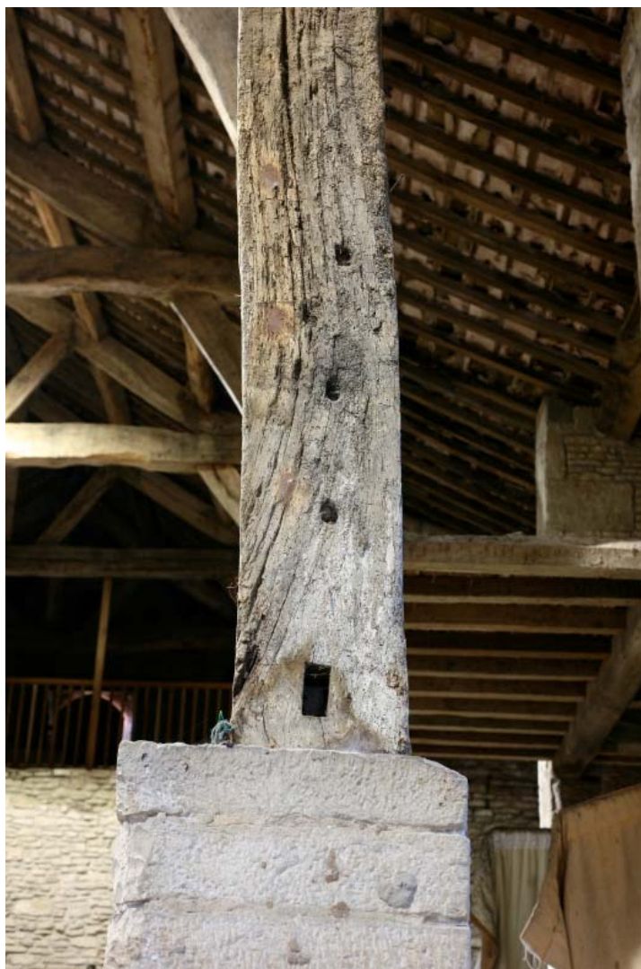
Plate 53: Example of stave/peg holes on an aisle post
