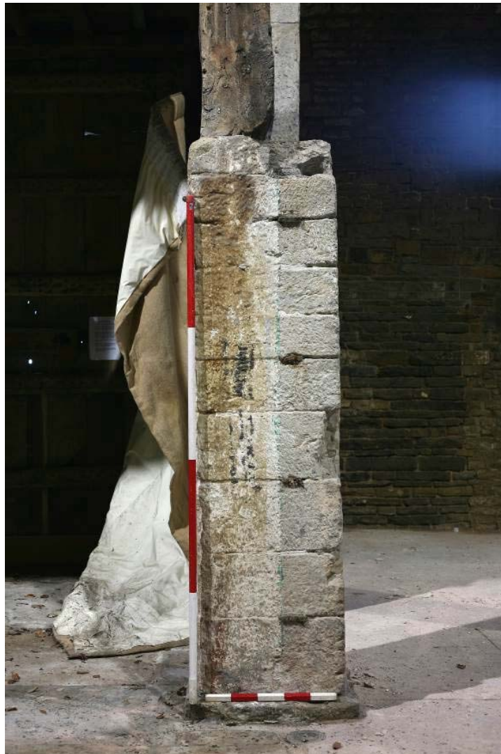
Plate 54: Example of vertical scarring on a stone plinth
