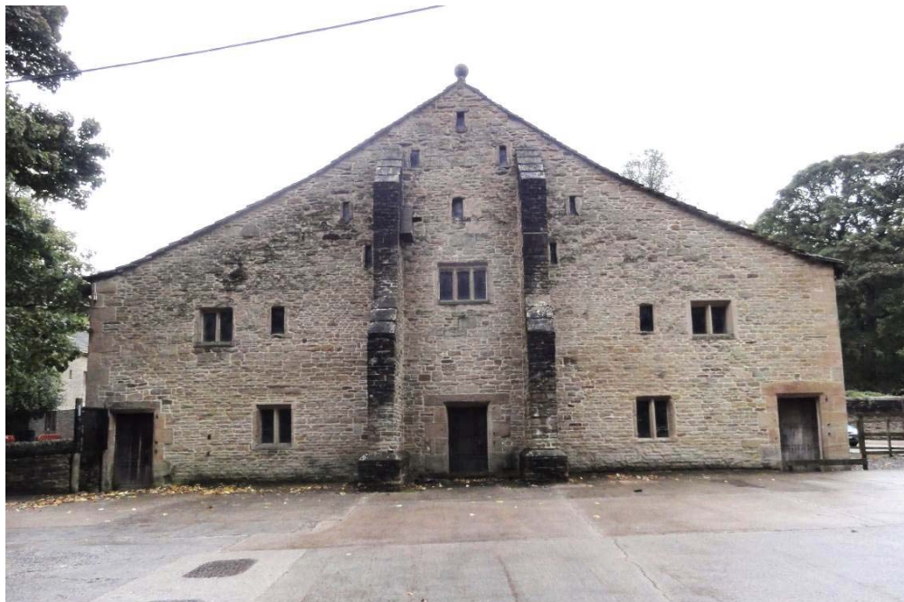
Plate 33: The rear (north) gable elevation of the main barn
