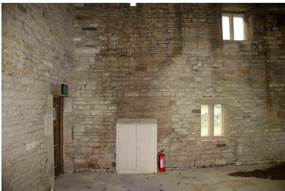
Plate 13: The northern end of eastern wall of the barn, facing east. The northern most blocked window is just visible behind the cupboard
