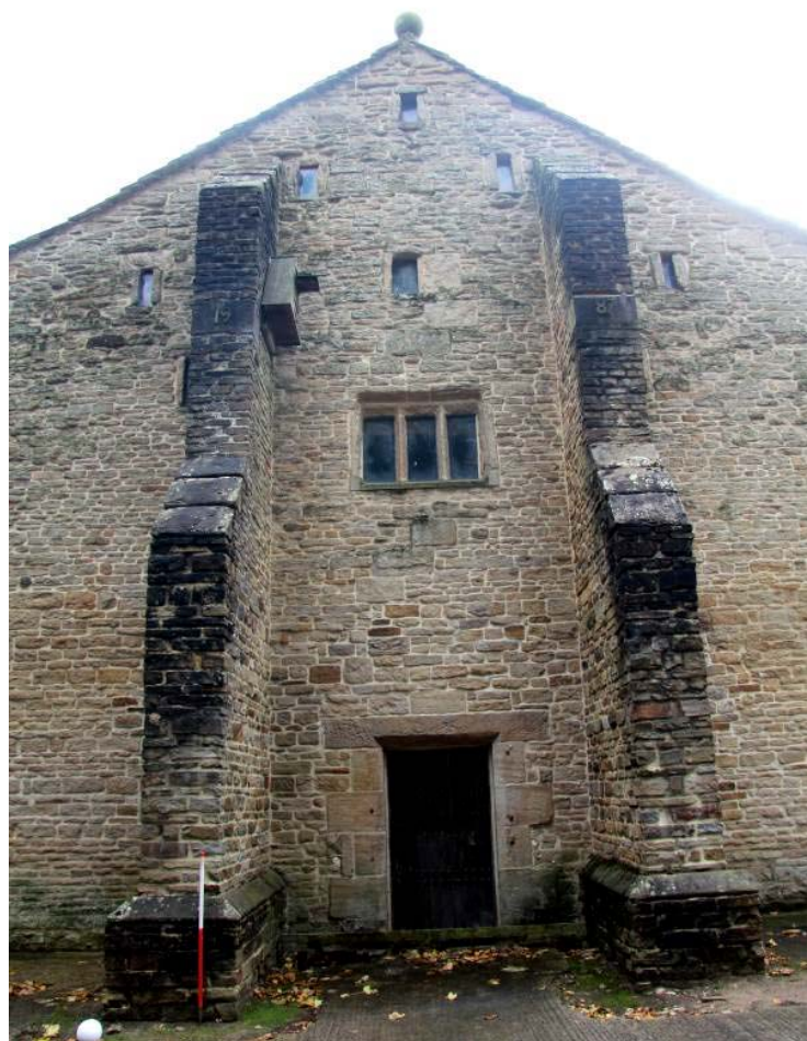
Plate 9: The supporting buttresses at the northern gable end of the Great Barn, with date stone towards the top recording their construction in 1987
