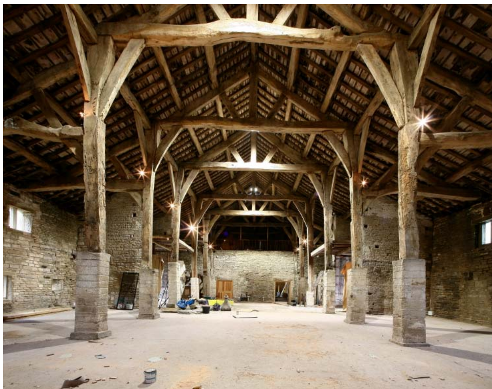
Plate 46: Interior view of the barn showing the aisled construction
