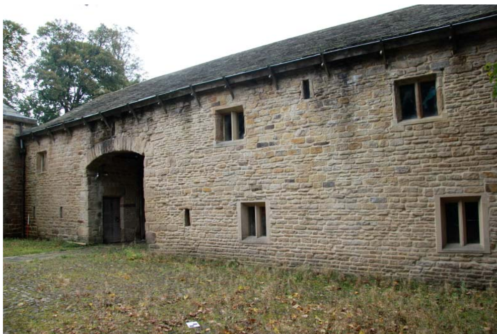
Plate 29: The east elevation of the main barn
