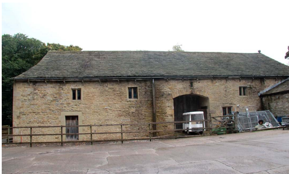
Plate 34: The west facing elevation of the main barn
