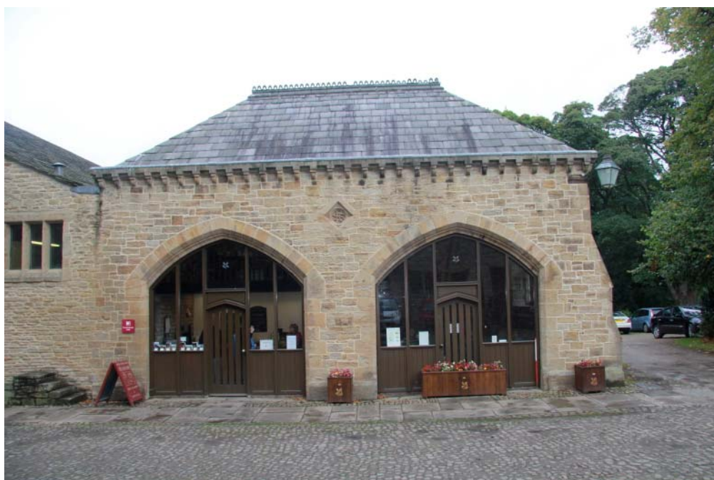
Plate 26: The south elevation of the carriage house
