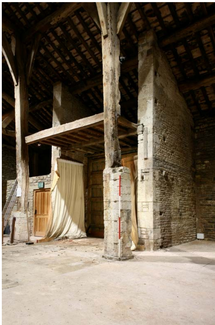
Plate 55: Internal porch on the west side of the barn
