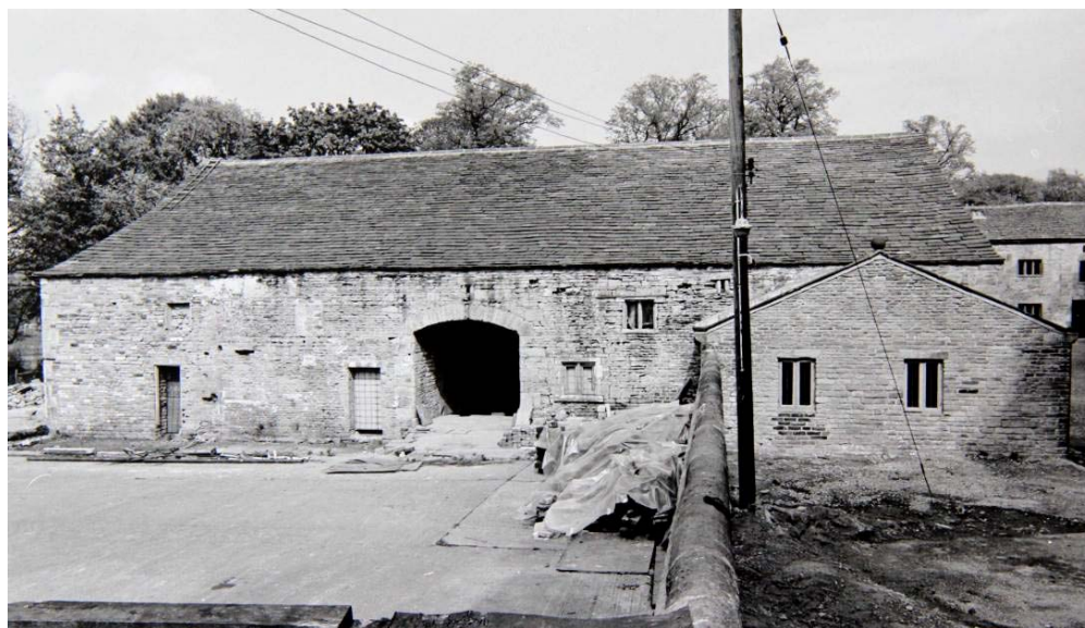
Plate 11: The western elevation of the barn taken in 1987, showing that the north-western extension had been removed by this date. The pedestrian doorway to the left of centre has since been in-filled
