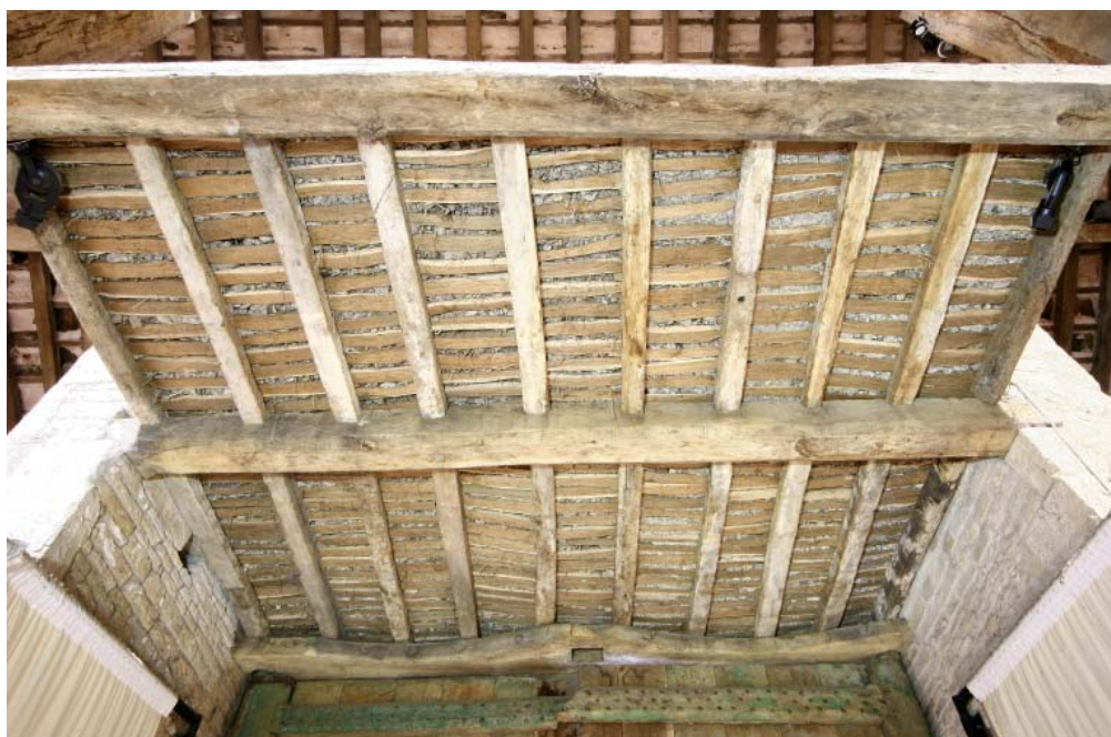
Plate 59: Example of the nature of the construction of the ceiling over the porches
