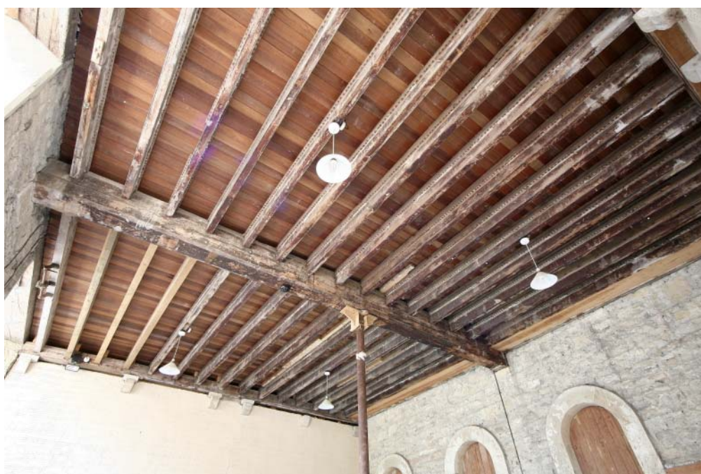
Plate 38: The ceiling in Room 1
