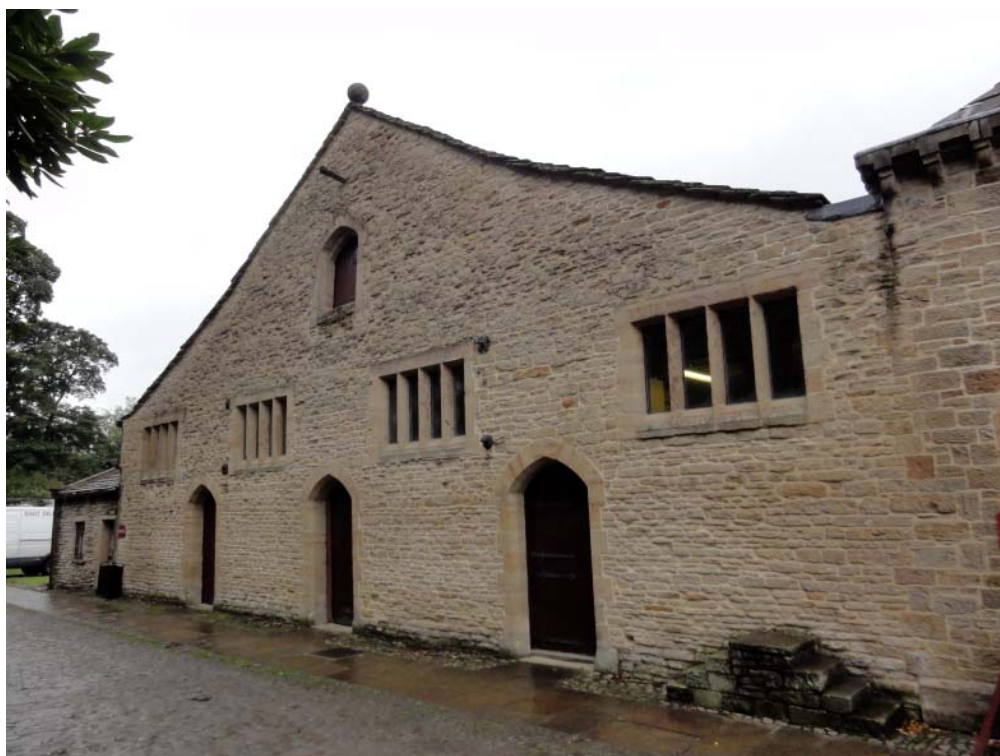
Plate 22: Principal elevation of the barn
