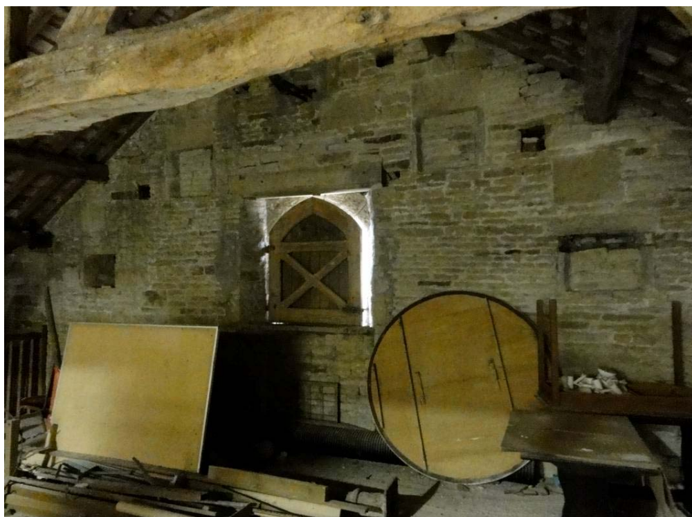
Plate 3: The interior of the upper portion of the southern elevation showing apertures blocked by the later outer skin
