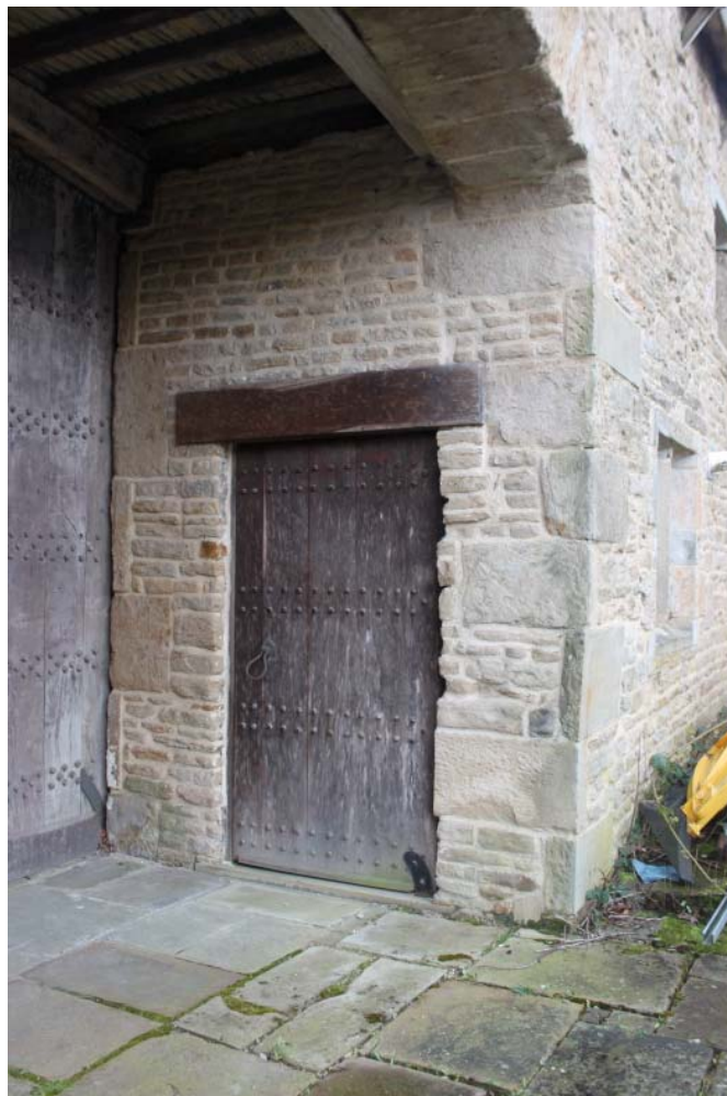
Plate 58: Pedestrian door way in the south wall of the east porch
