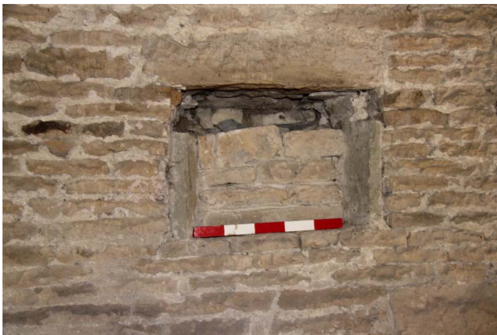
Plate 66: Example of a blocked aperture on the south internal elevation of the barn
