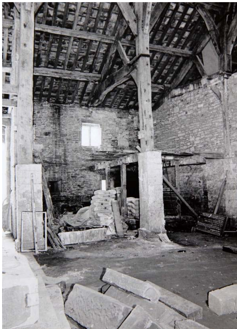
Plate 14: the interior of the barn in 1987, showing the shippon in the south-eastern corner during restoration, and also showing a clay floor surface (prior to its replacement with concrete in 2000)
