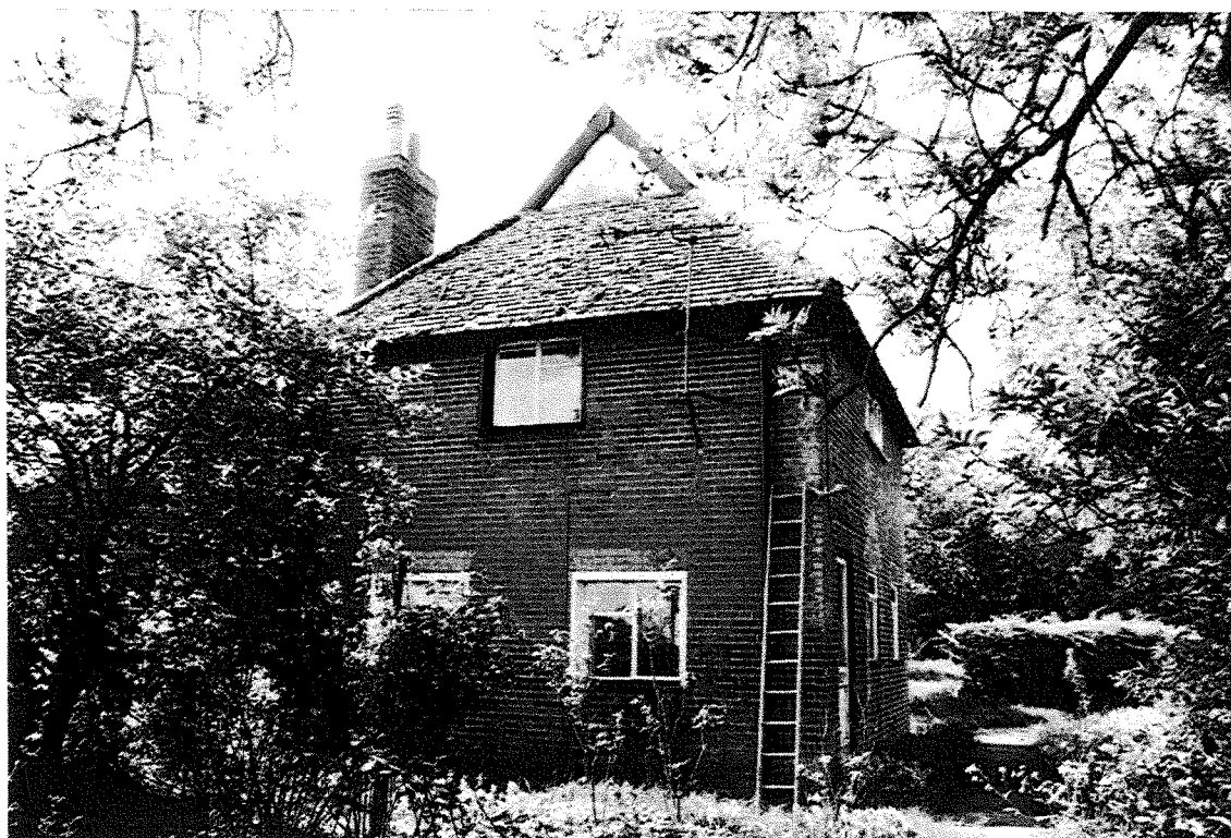
Plate 4 The dovecote from the north-east (showing inserted windows and new door position)
