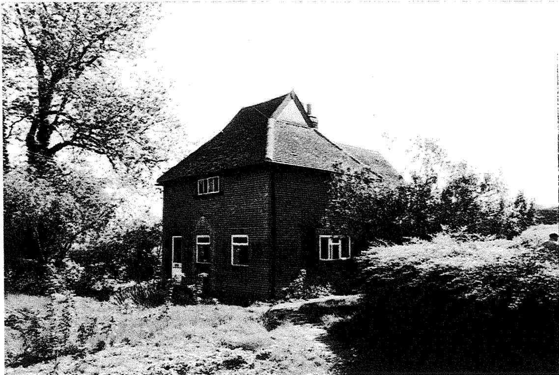
Plate 2 The dovecote from the west (showing scar of porch and new door position), 1995
