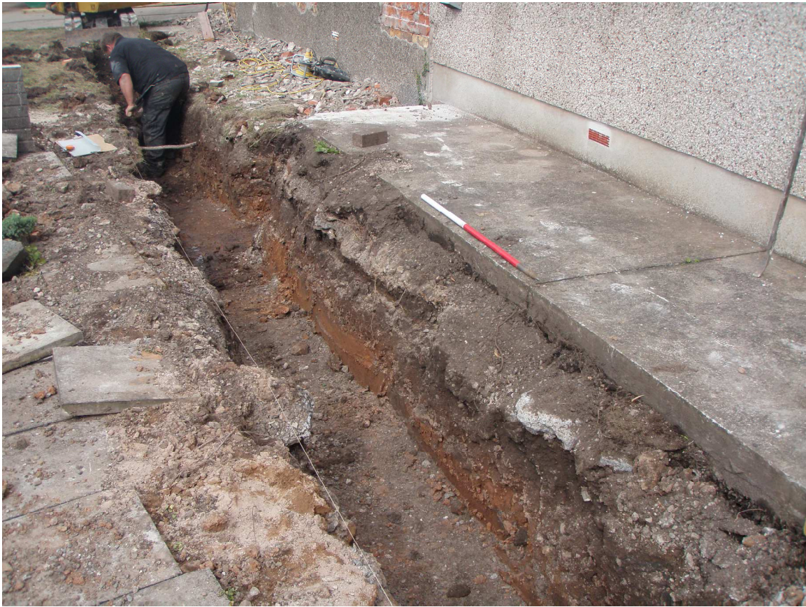
Plate 4: deposits within the new foundations
