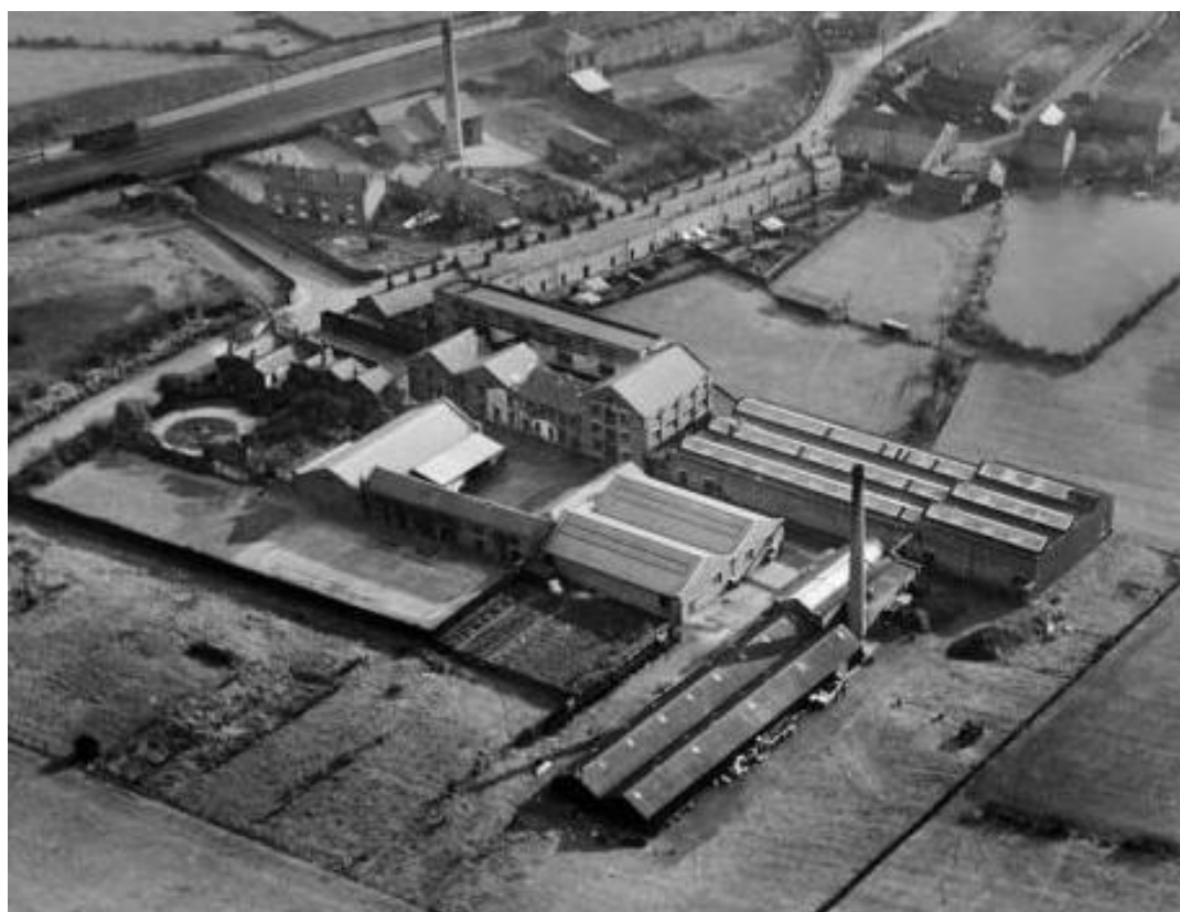
Plate 7: Aerial view across Stothert's chemical works in 1929
