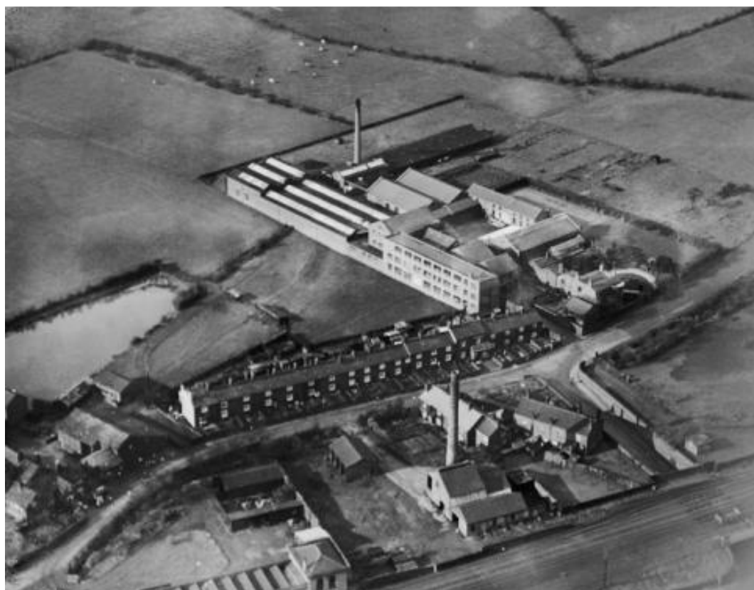
Plate 6: Aerial view across Bag Lane in 1929
