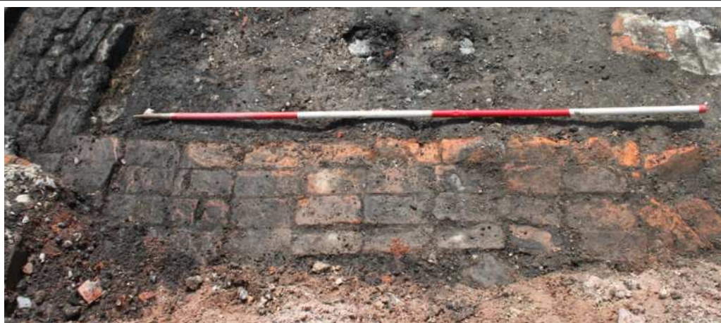
Plate 8: North/south-aligned wall 307, butted by slightly lower wall / floor (308)
