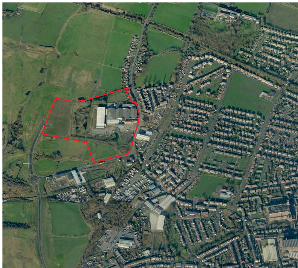
Plate 1: Recent satellite view of the site, prior to the demolition of the modern factory, showing the indicative boundary of the application area
