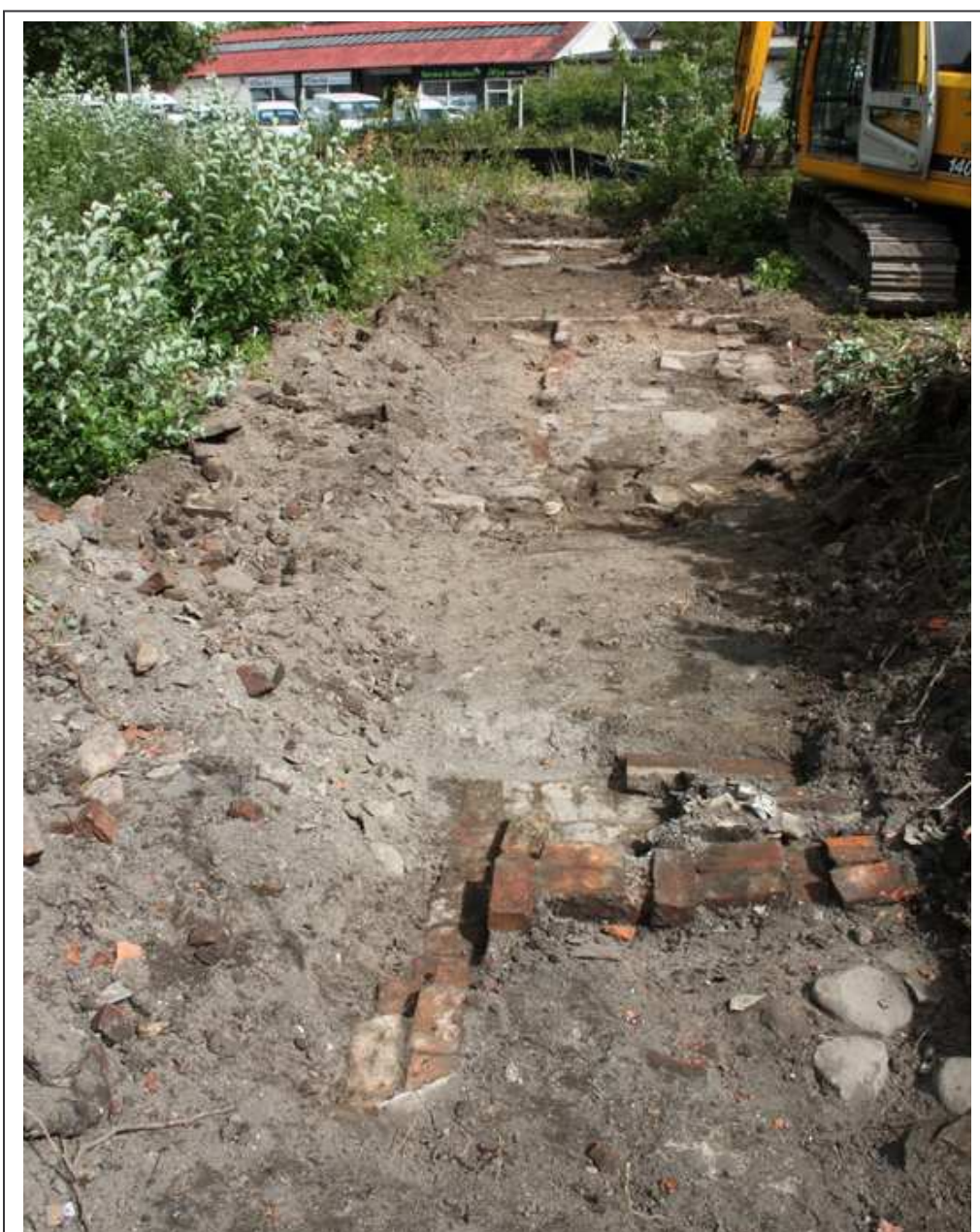
Plate 19: General view of Trench 6, looking east
