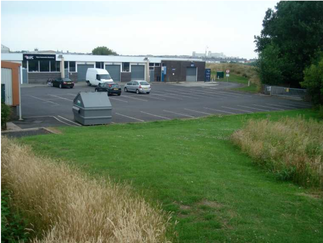
Plate 10: Approximate location of the buildings named Higham or High Holme on nineteenth century maps (Site 10), looking west
