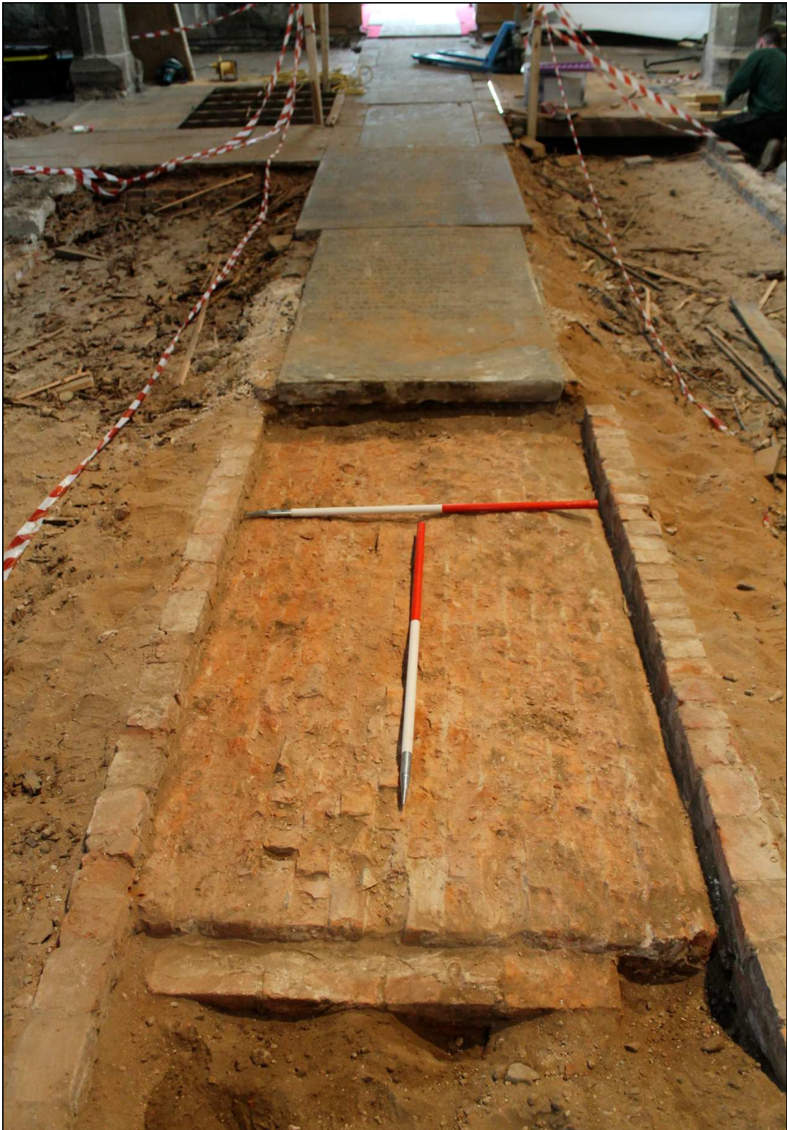
Plate 13: Surface of the barrel vaulting of the Greg Crypt exposed beneath the ledger stones
