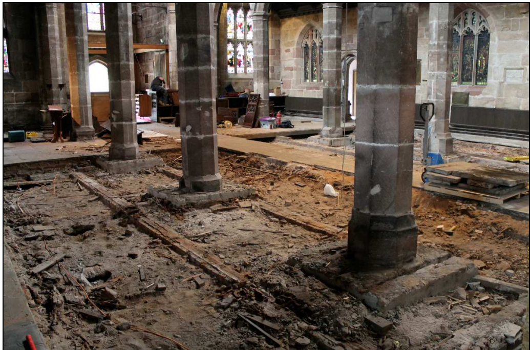
Plate 3: General view across the nave during the reordering works
