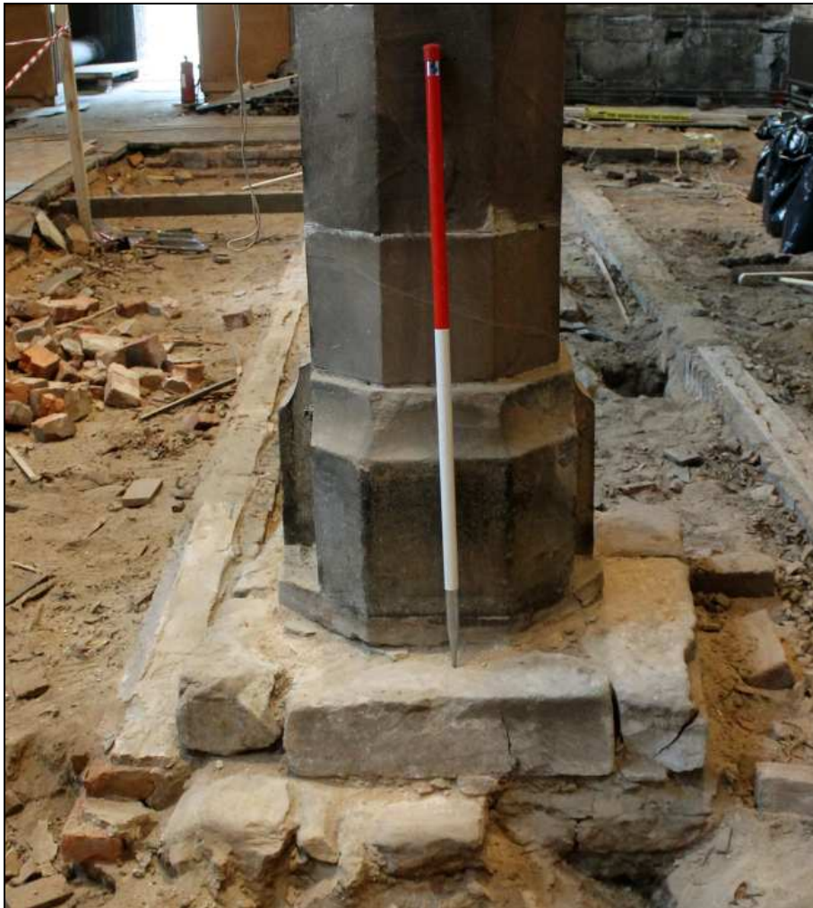
Plate 5: Column base B
