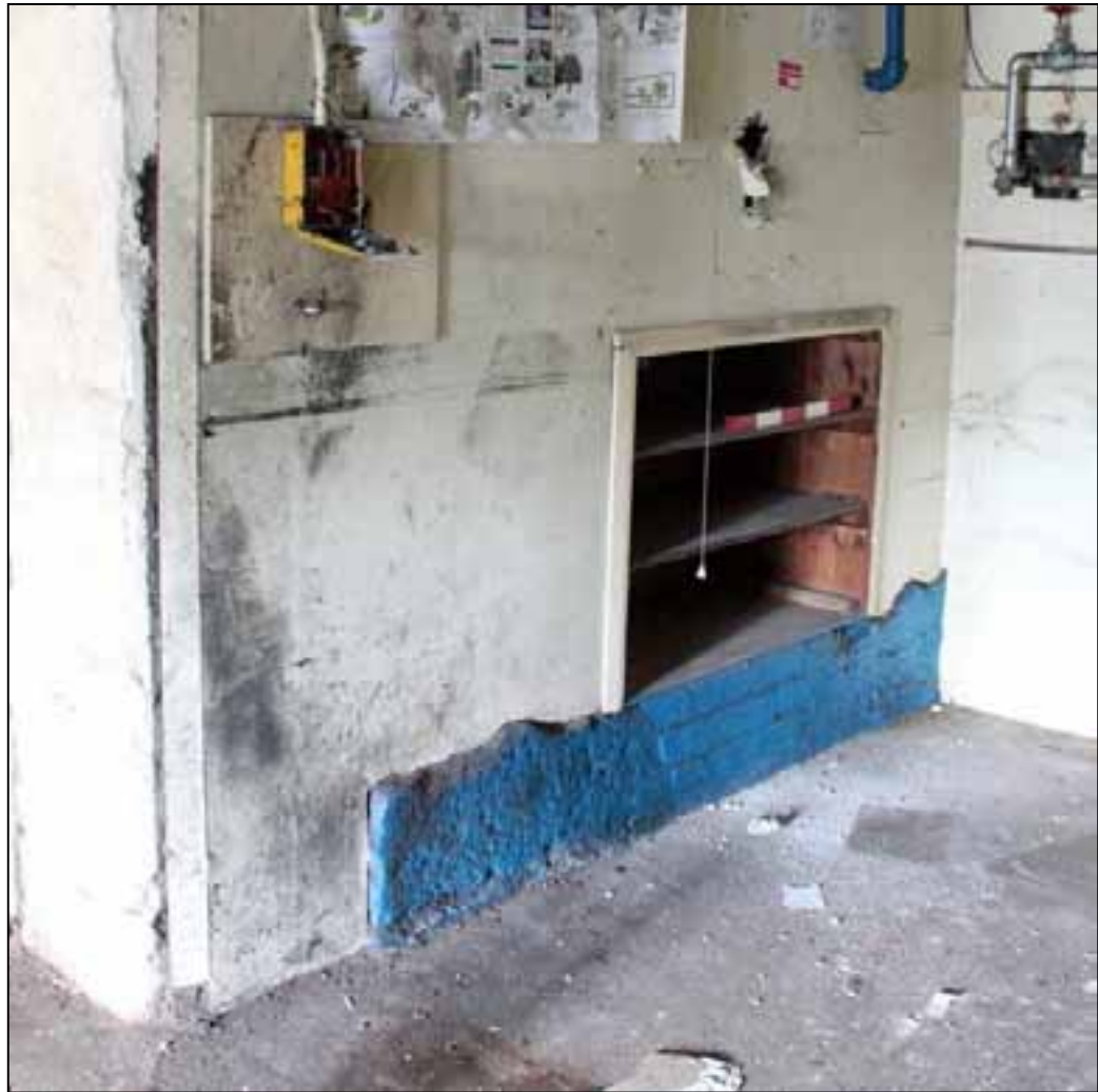
Plate 45: Pad for axle mounting, with curved rebate infilled with brick
