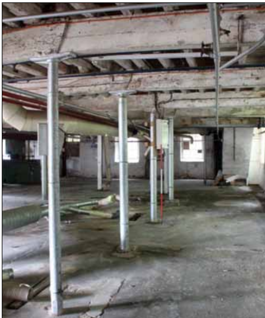
Plate 28: Inserted columns on the ground floor
