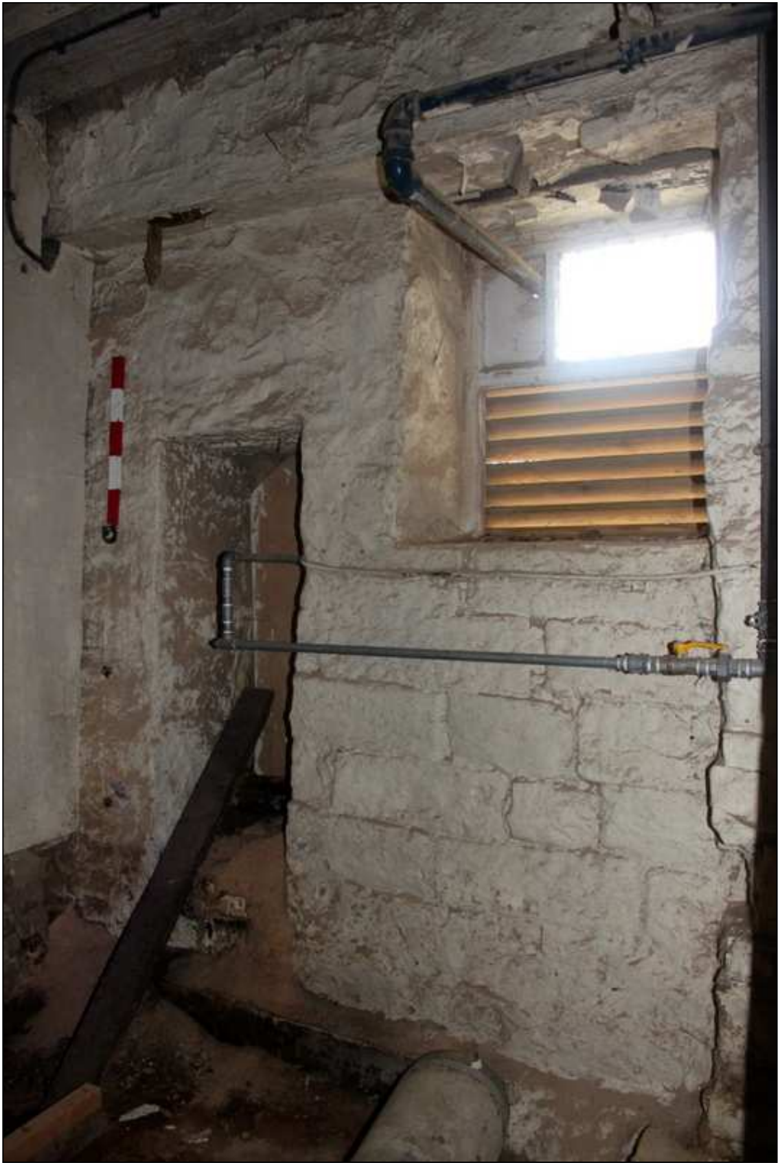
Plate 44: Blocked aperture in the south wall of the engine house, with possible bearing box on the left
