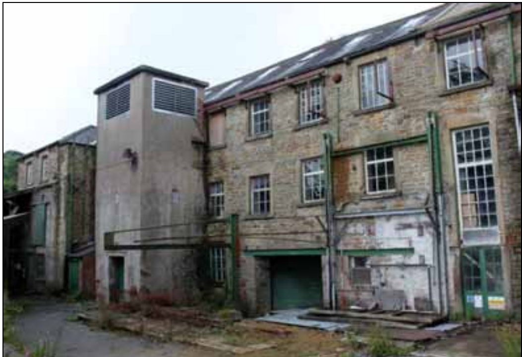
Plate 4: The south-facing elevation of Kirk Mill
