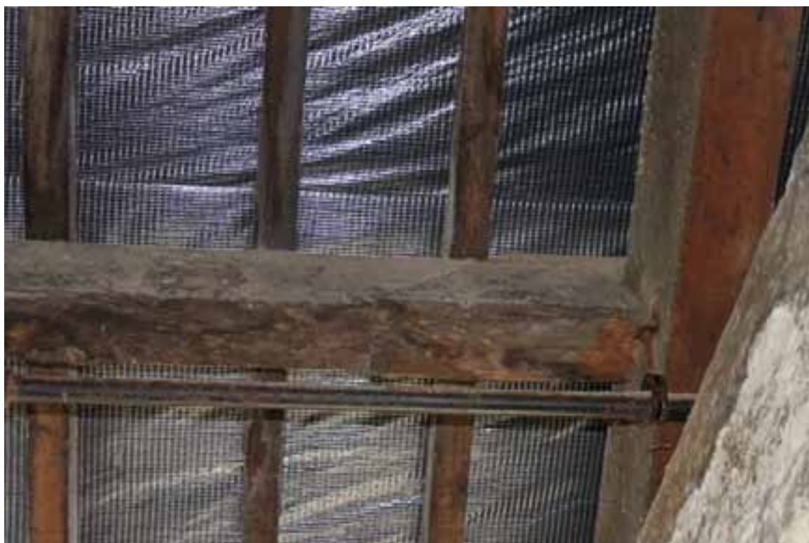
Plate 89: Scarf joint in purlin of west wing
