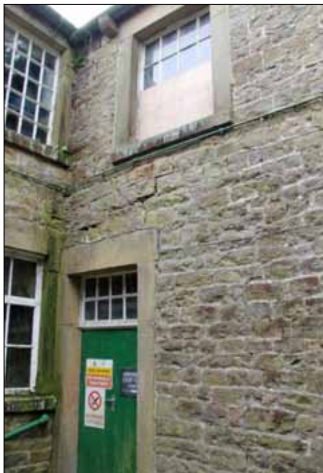
Plate 15: East wall of stair tower
