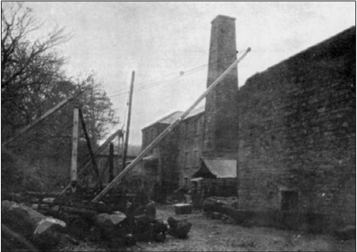
Plate 2: Kirk Mill from the south-east, 1924
