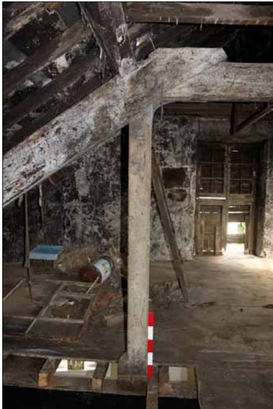
Plate 96: Queen strut truss above east extension
