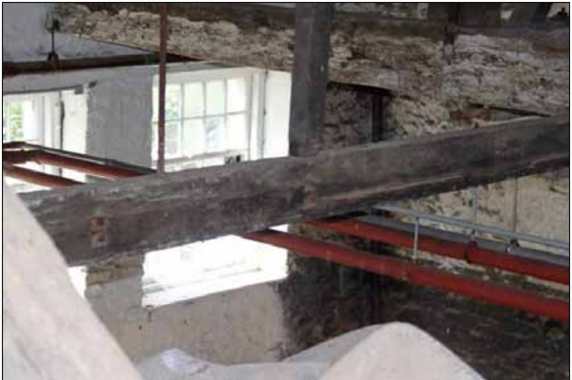
Plate 86: Mortices for ceiling joists above west wing
