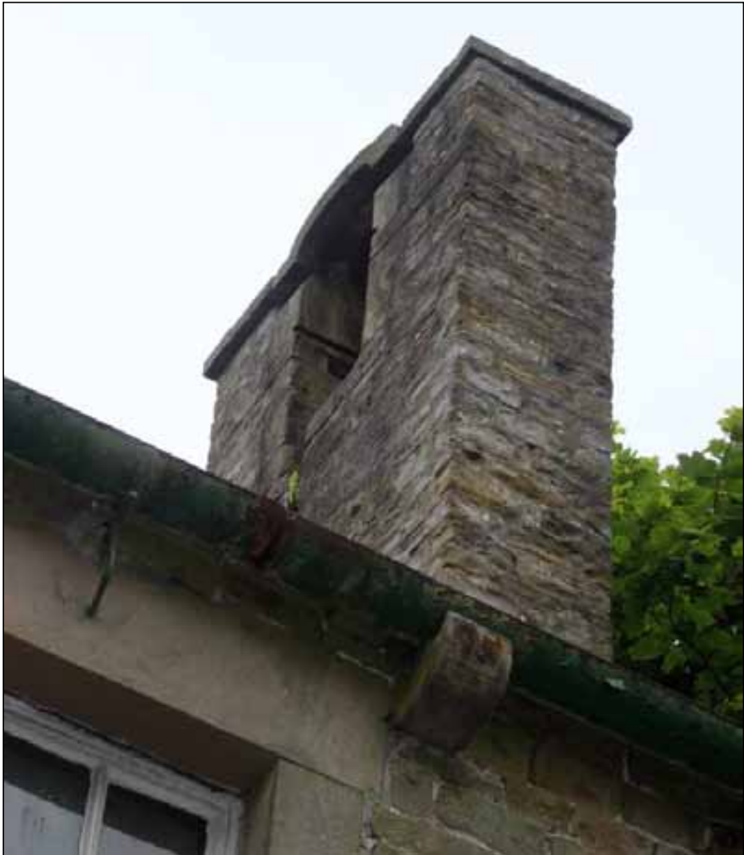
Plate 17: Bell cote above stair tower
