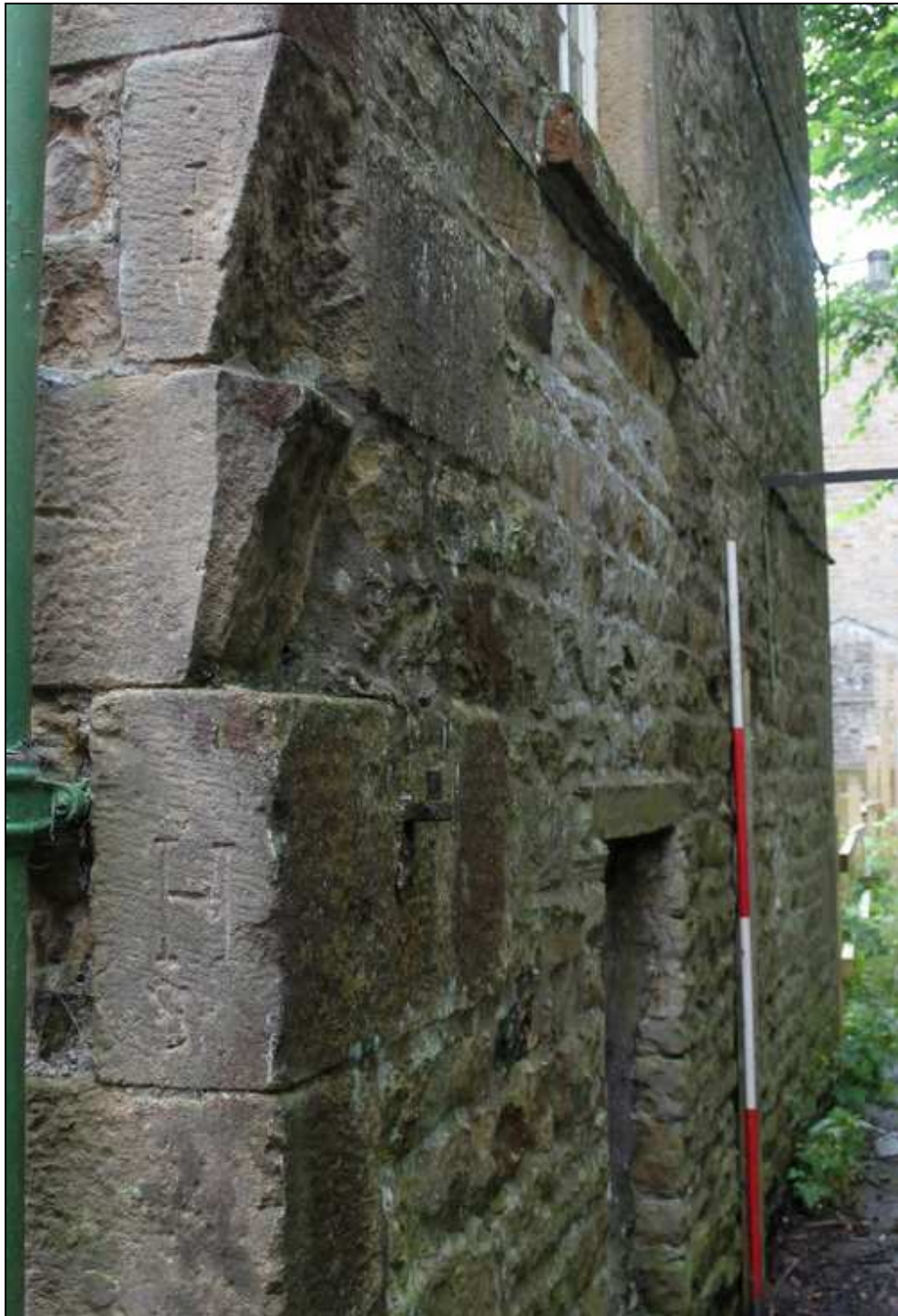
Plate 16: Mason's marks on stair tower quoins
