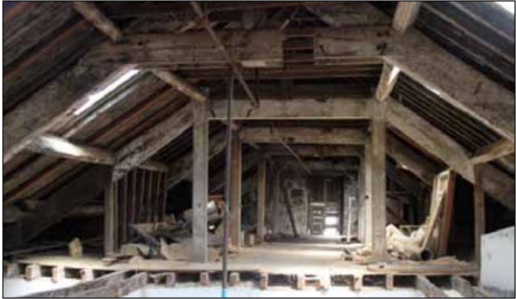
Plate 94: Queen post trusses above engine and wheel houses
