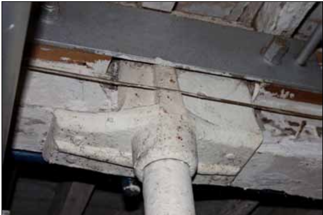
Plate 53: L-section column head plate
