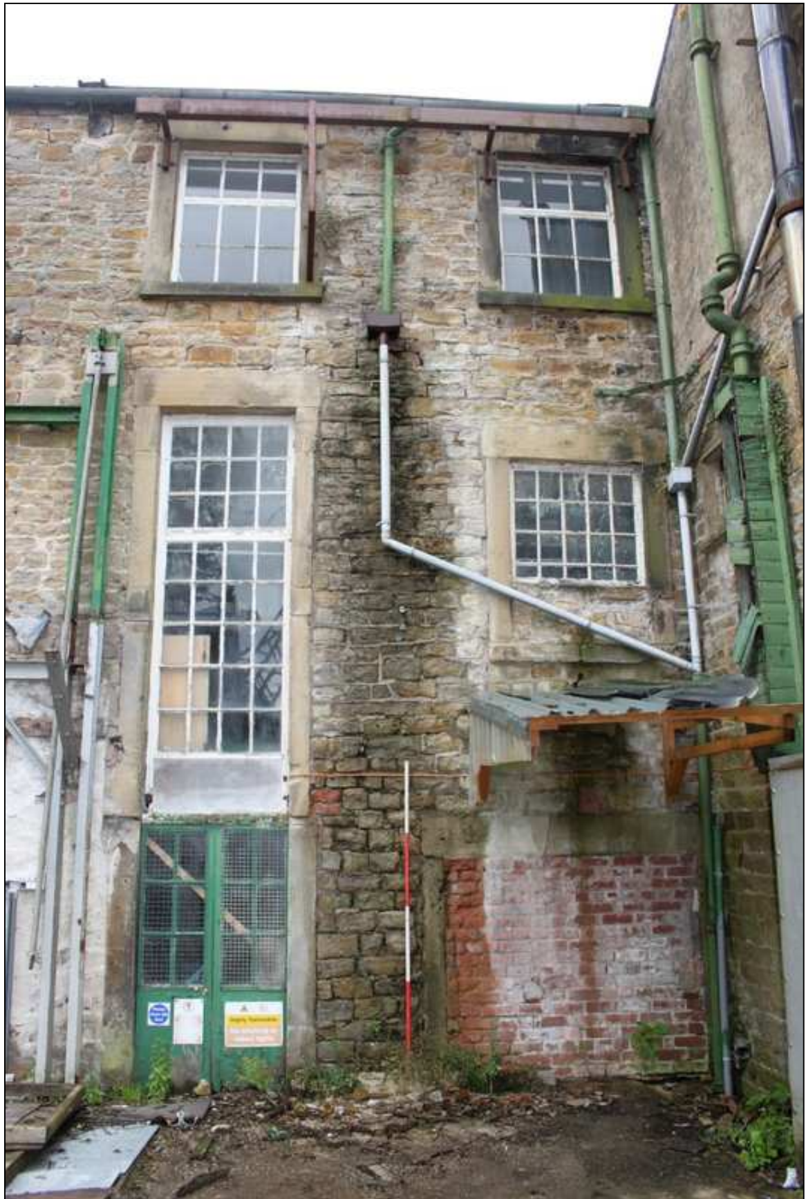
Plate 8: Façade of engine and wheel houses
