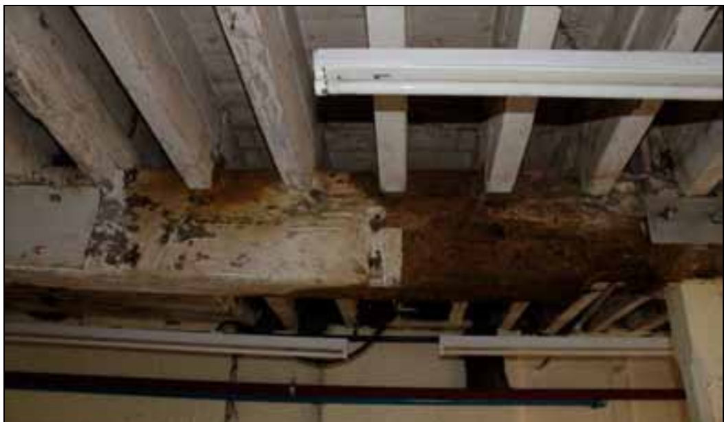
Plate 48: Scar of large drum and chamfered prop
