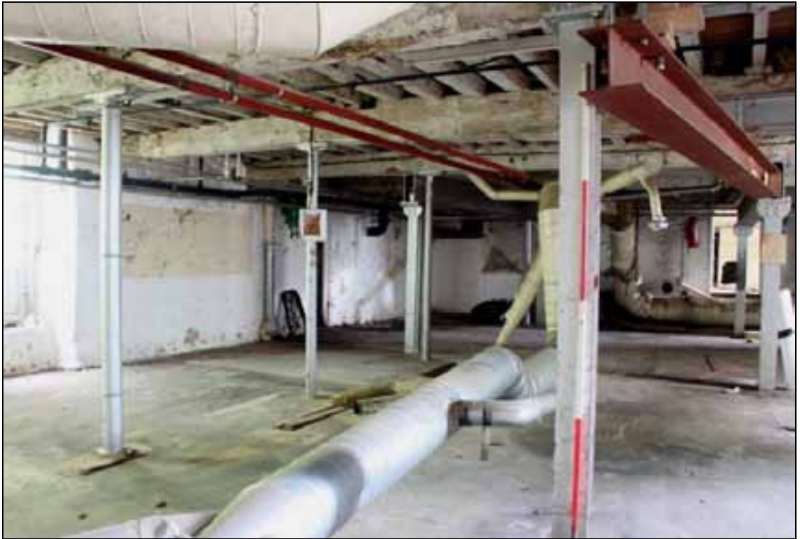
Plate 6: General view of the ground floor
