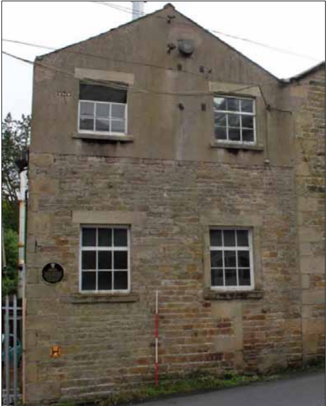
Plate 21: Southern extension to the east wing
