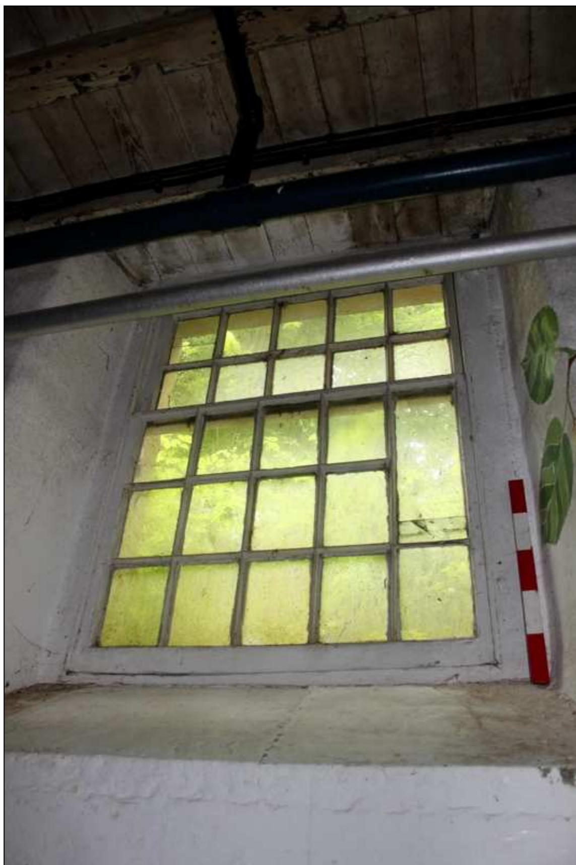
Plate 32: Vertical sash window in north wall
