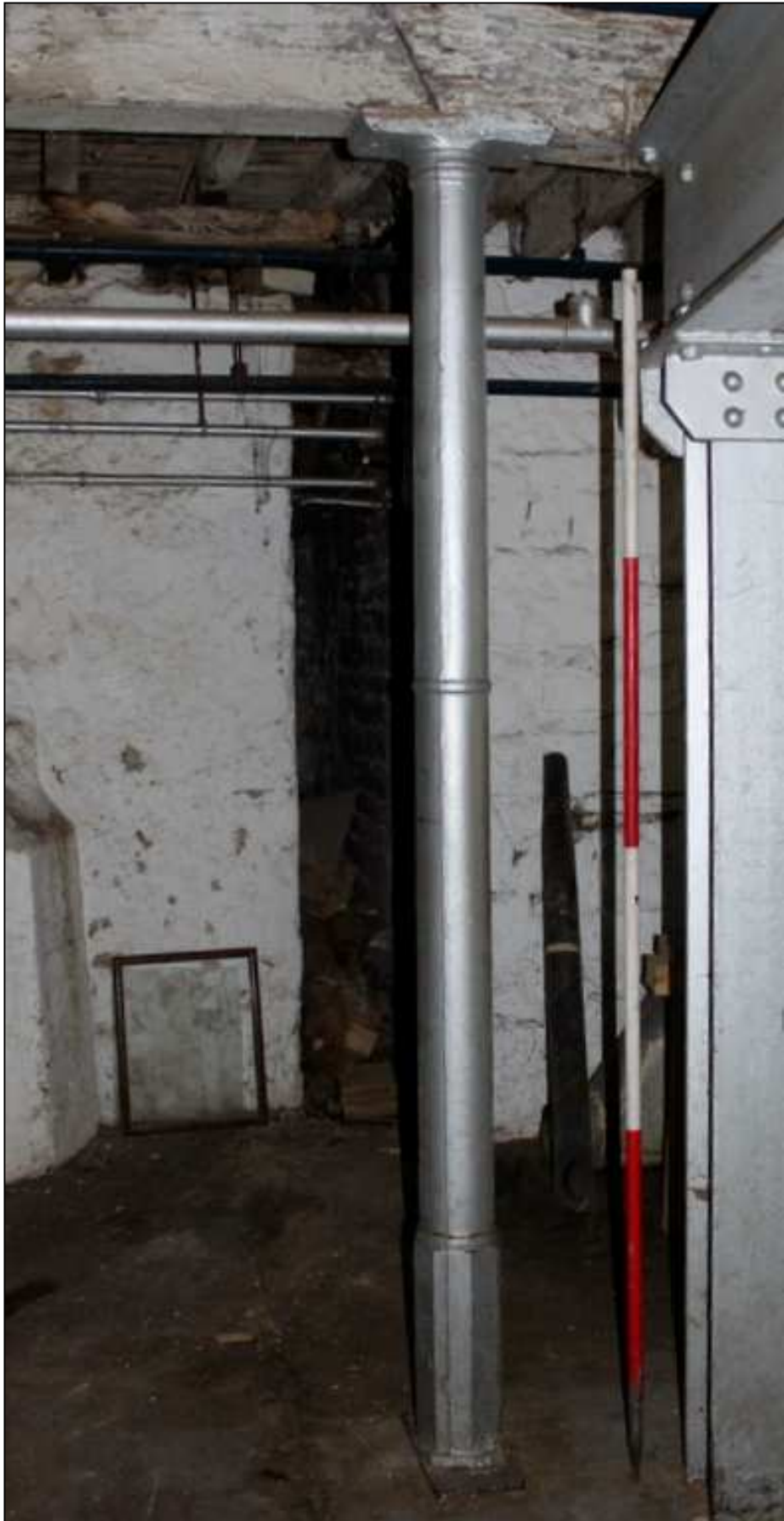
Plate 30: Column with astragal in shaft
