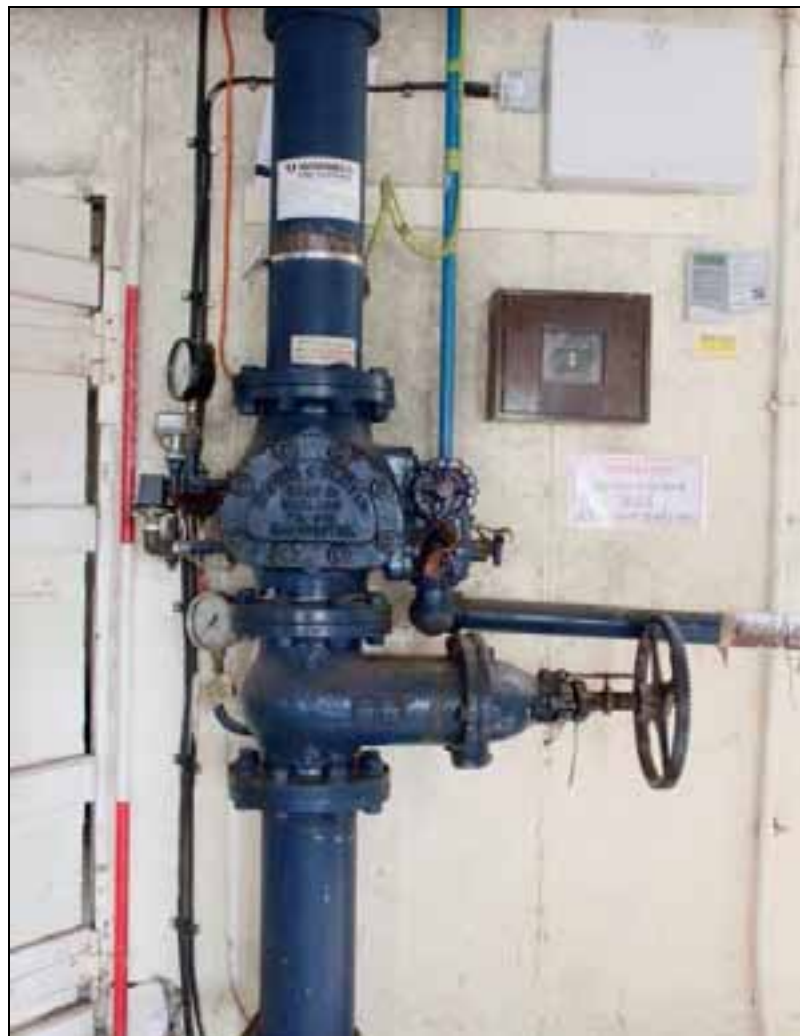
Plate 62: 'Christmas tree' control valve of sprinkler system
