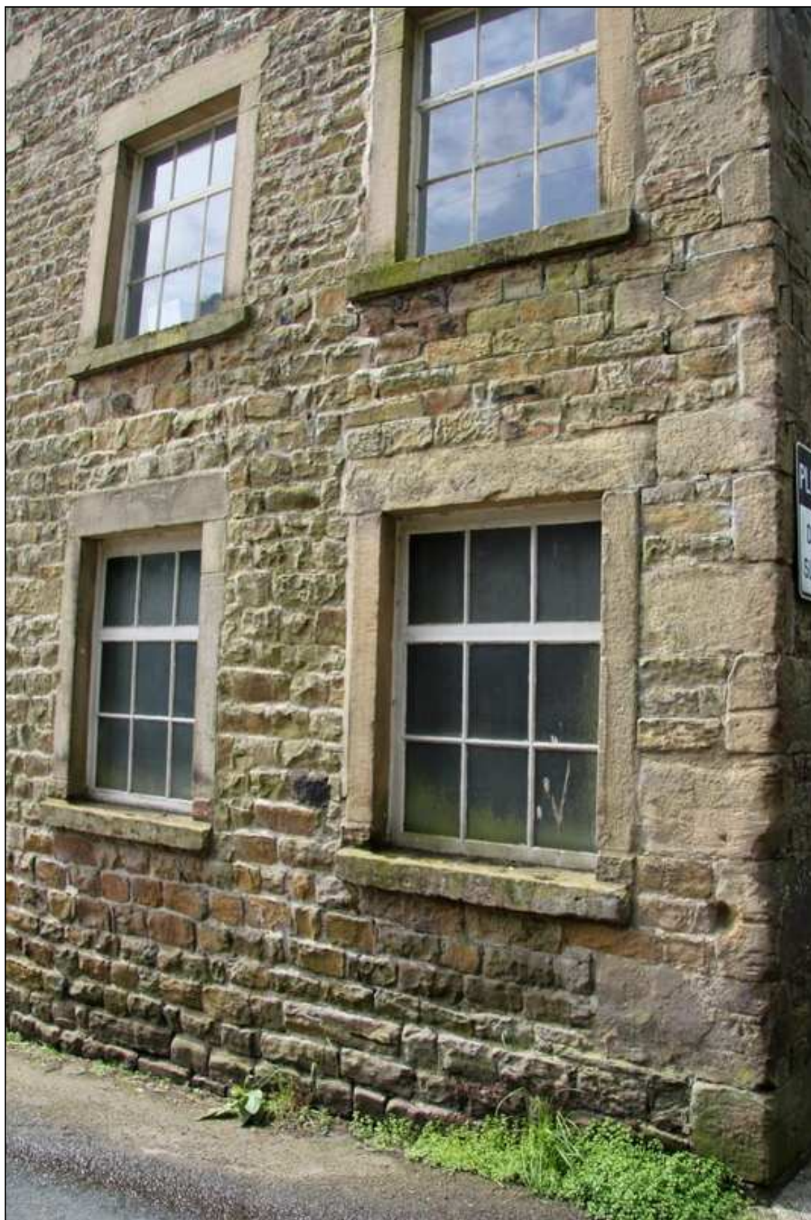
Plate 20: North return of the east wing, showing rebuilt wall and inserted windows
