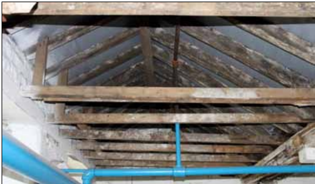
Plate 90: Common rafter roof of extended northern bay of main mill
