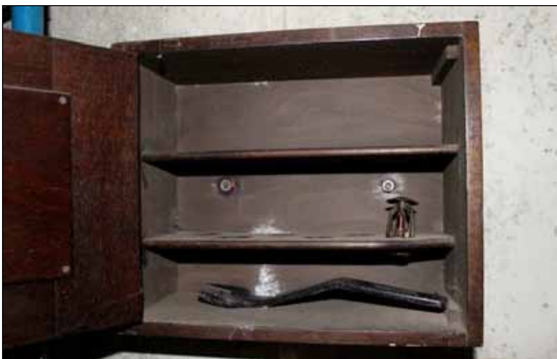
Plate 63: Cabinet housing spare parts for sprinkler system
