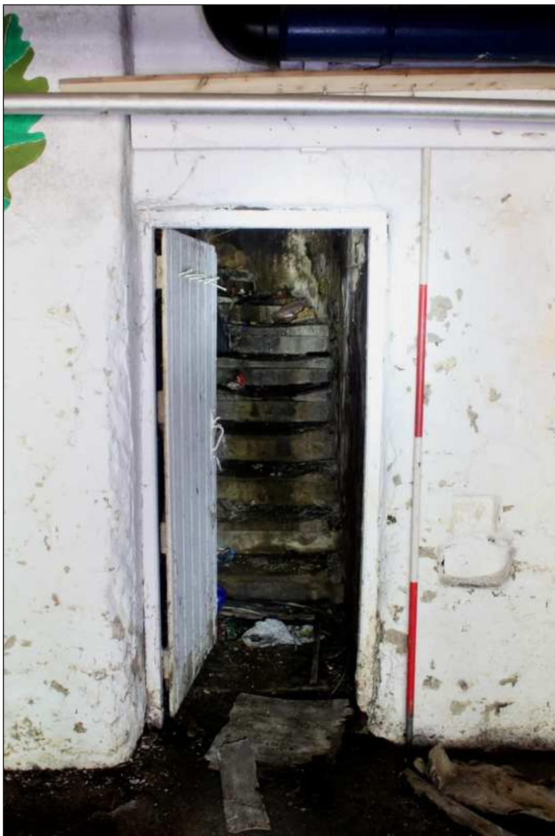
Plate 33: Base of stair tower with spiral staircase
