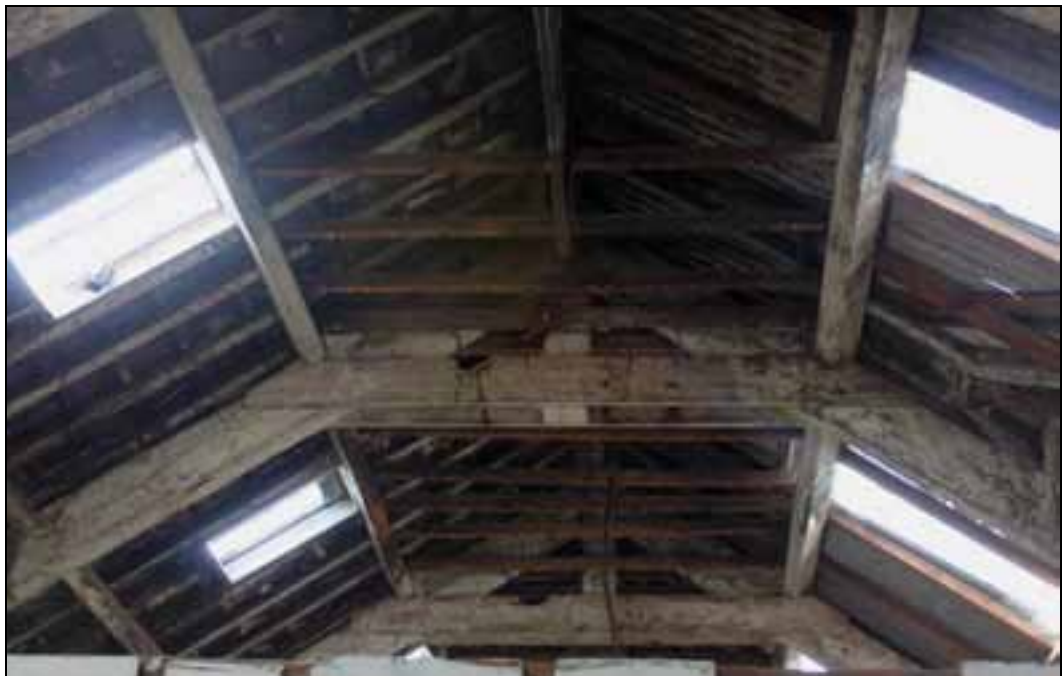
Plate 83: Remodelled king post trusses
