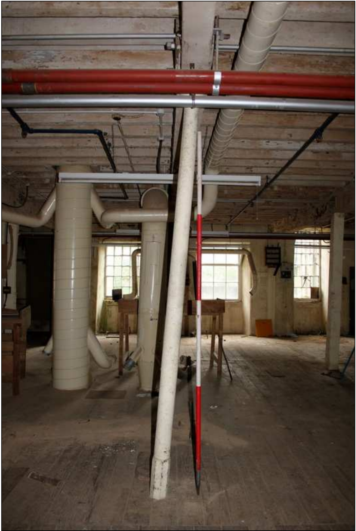
Plate 54: Deflection of first-floor column
