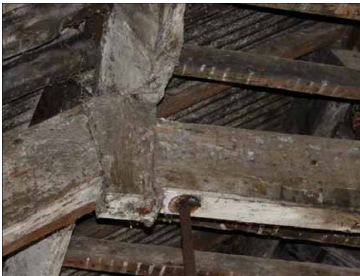
Plate 88: Jowled head of queen post, carrying side purlin, with adjacent replacement rod
