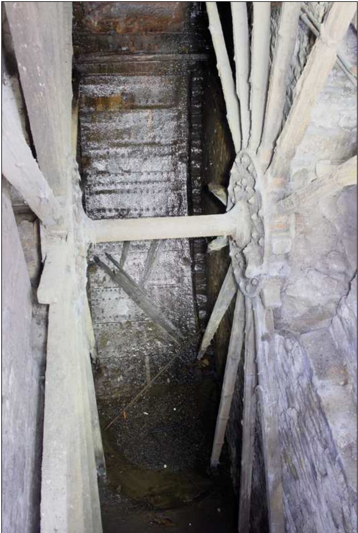
Plate 70: Axle and eastern bearing of waterwheel
