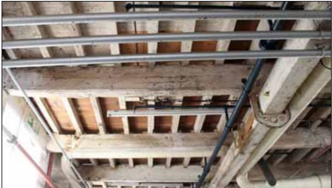
Plate 35: Additional longitudinal ceiling beam in west wing
