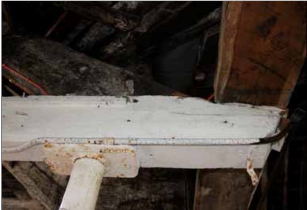
Plate 79: Plain column capital, second floor
