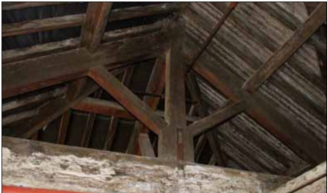
Plate 85: King post truss above west wing
