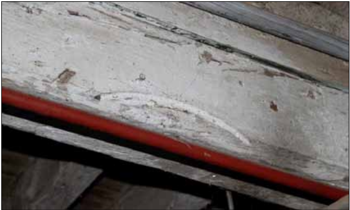
Plate 39: Scar of drum attached to line shaft
