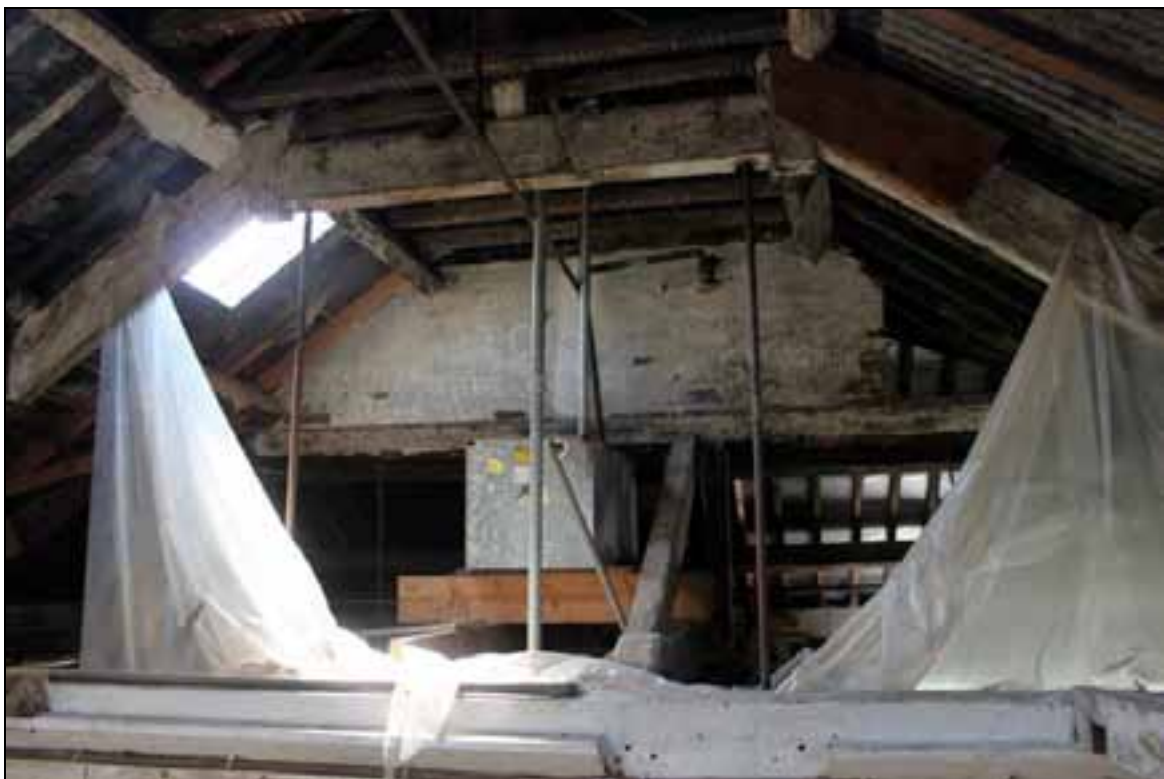
Plate 87: Lath and plaster partition between roofs of main mill and west wing, and queen post truss with replacement iron rods
