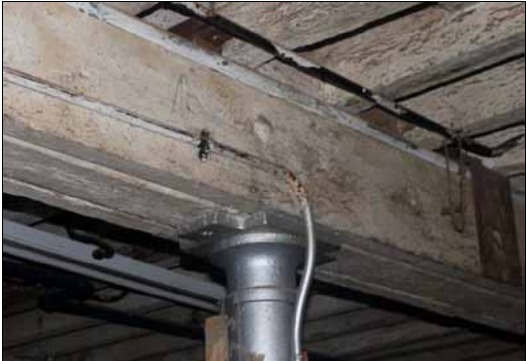
Plate 31: Cruciform-section bolting head of column
