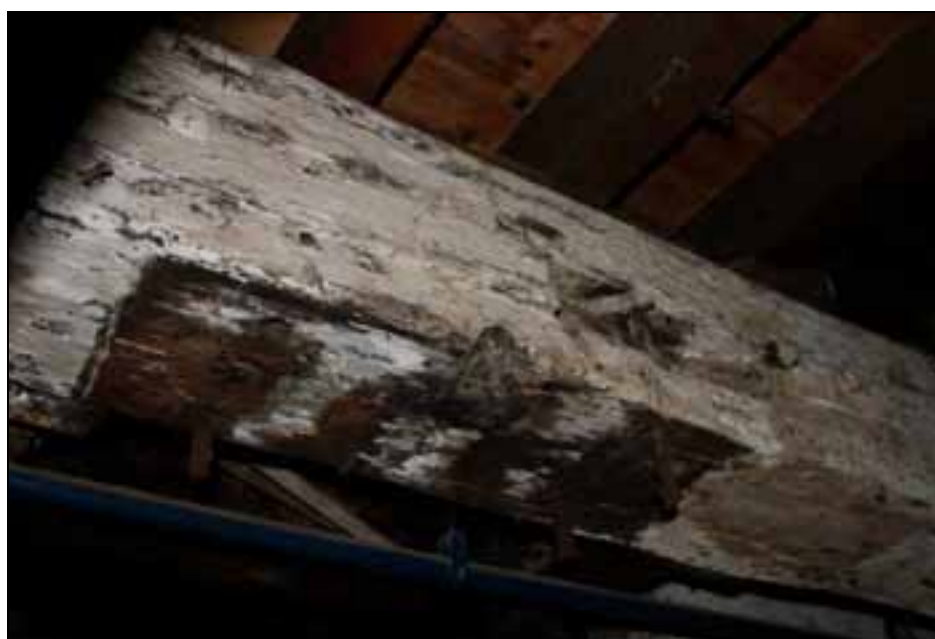
Plate 68: Compression scar and bolts associated with vertical shaft from steam engine
