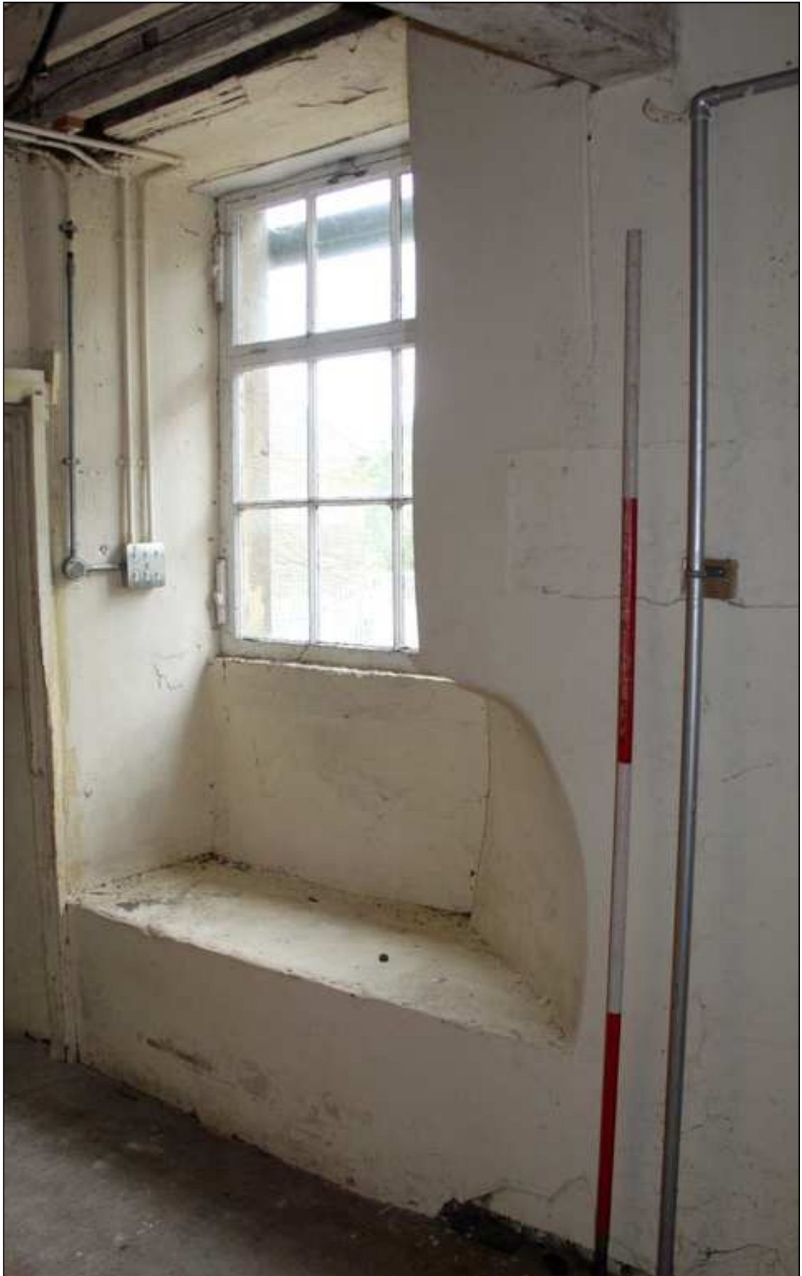
Plate 56: Rebate in south wall, possibly for mule headstock
