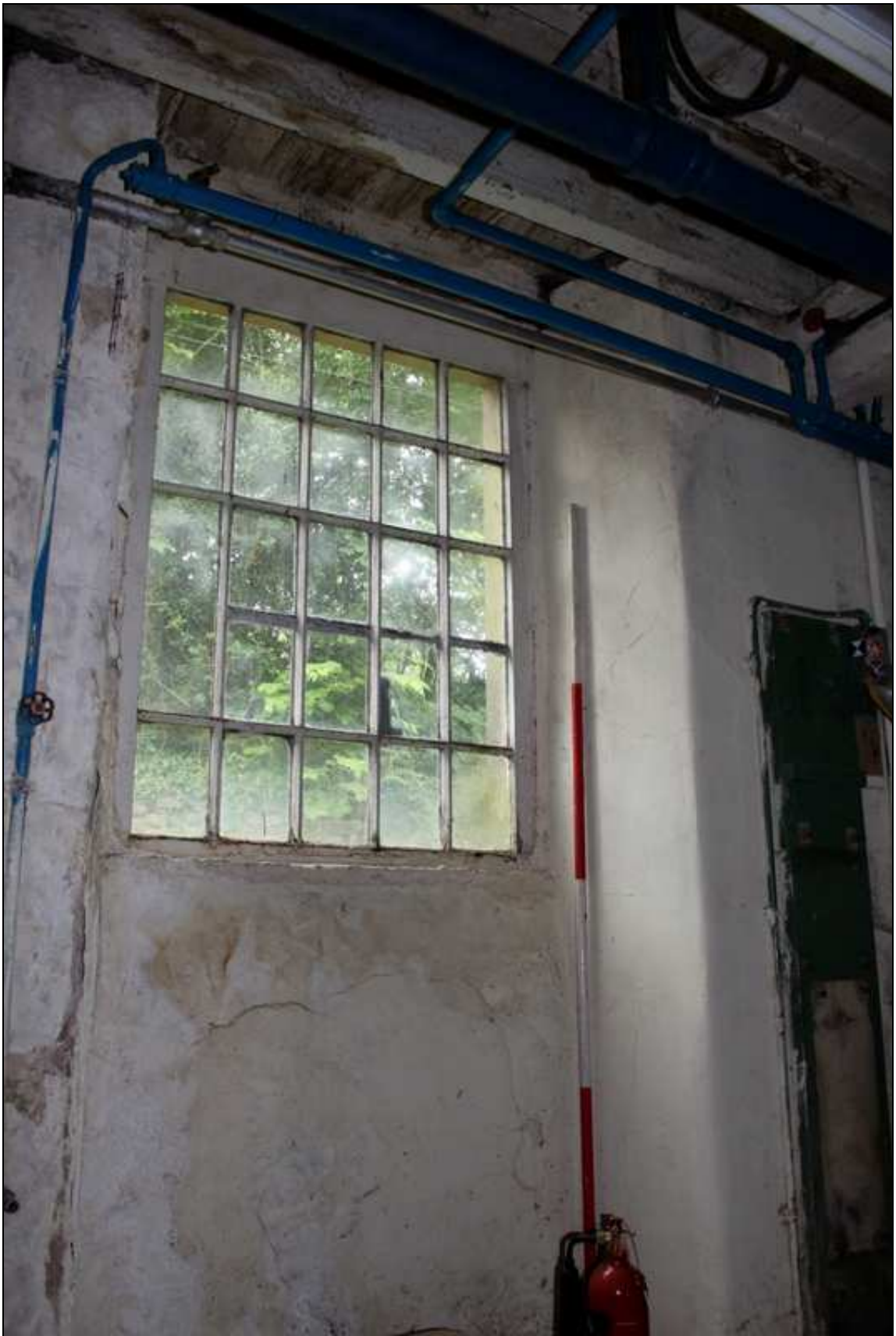
Plate 55: 25-light window in north wall, first floor
