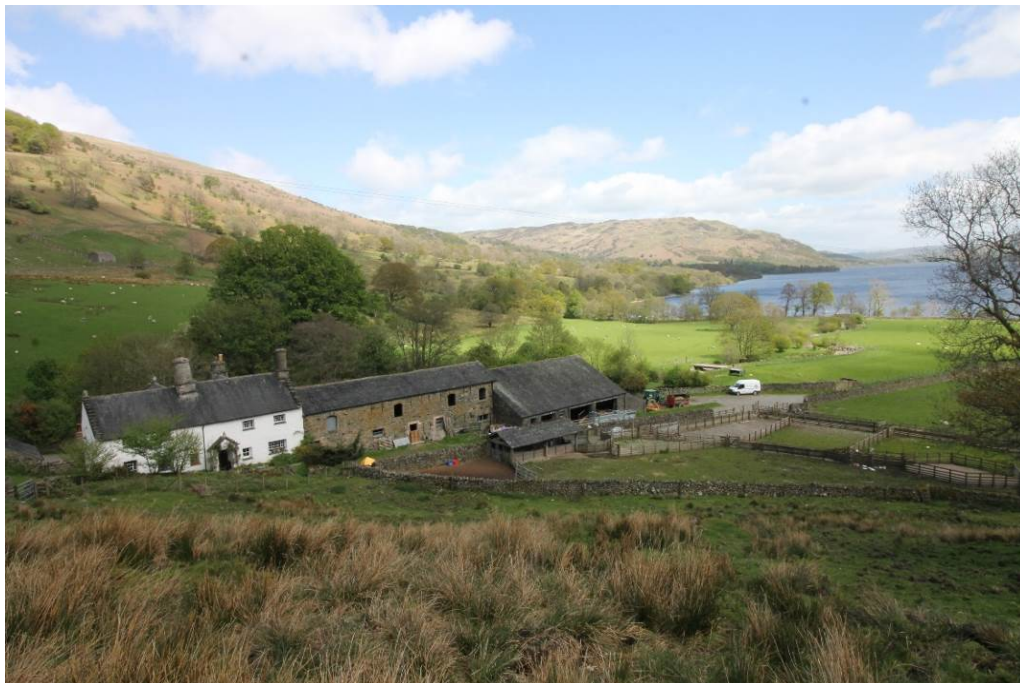
Plate 2: Glencoyne Farmhouse (Site 66)
