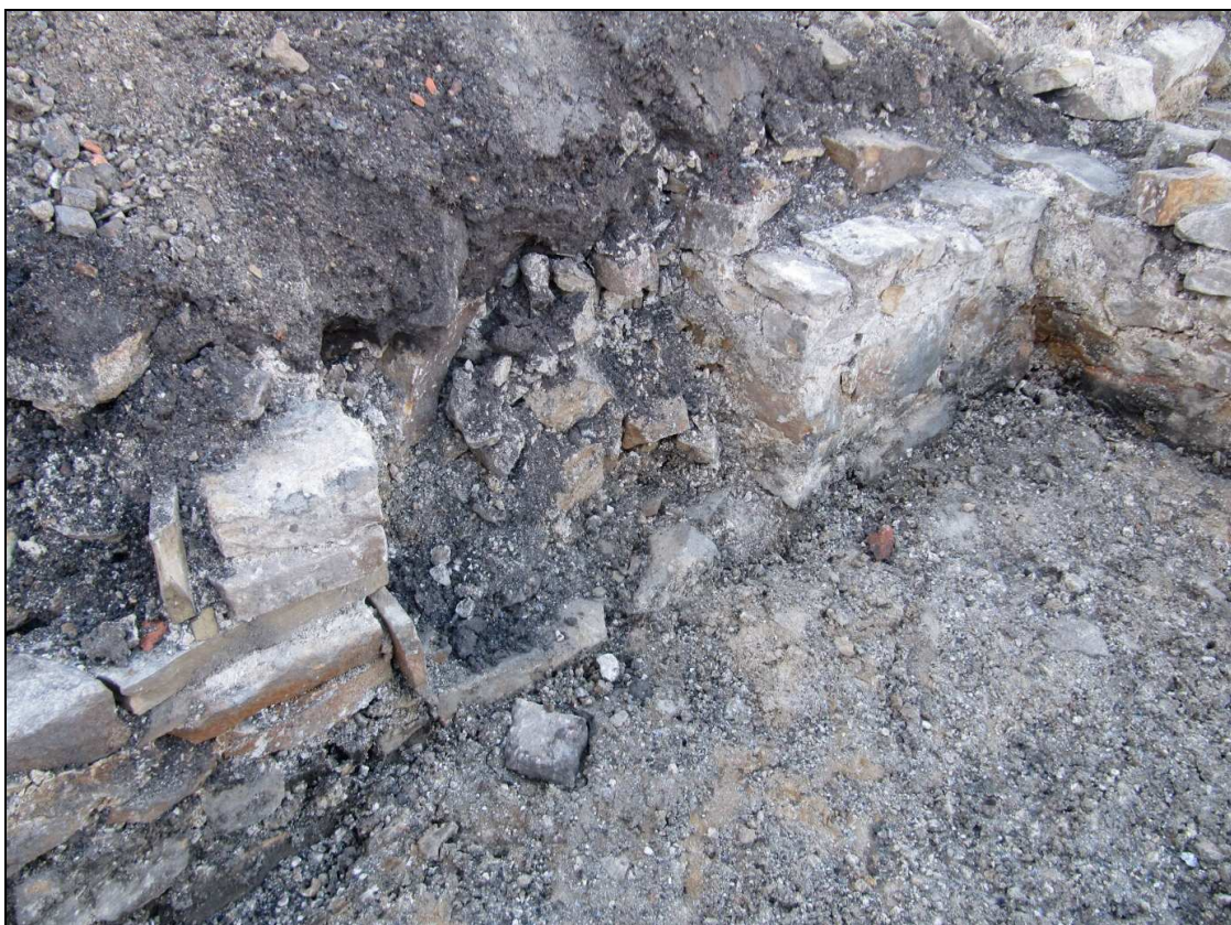
Plate 15: The threshold between the front and back rooms in N° 24 Stanhill Road
