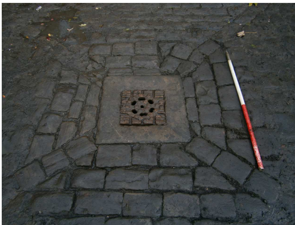
Plate 7: The iron drain cap in the centre of courtyard 1007
