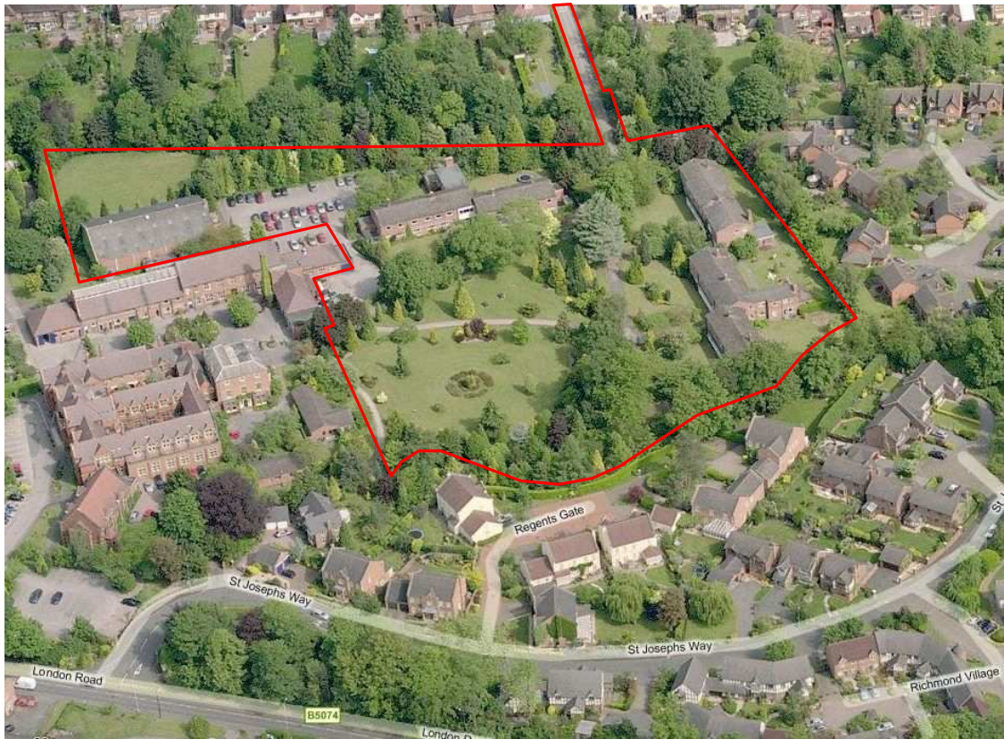
Plate 1: Aerial view of the Scheme Area
