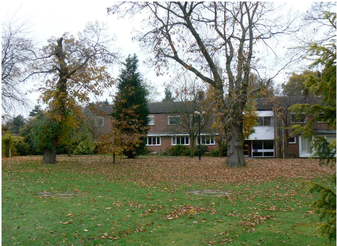
Plate 8: View of the two-storey range across the northern part of the site
