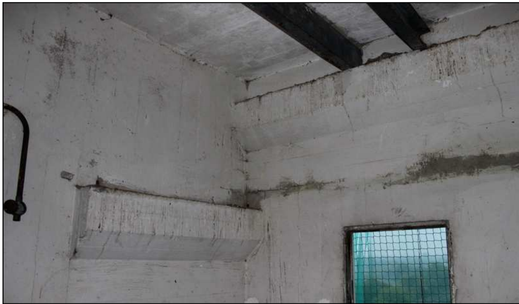
Plate 21: Ceiling beam and supporting rails for hoist in stair tower
