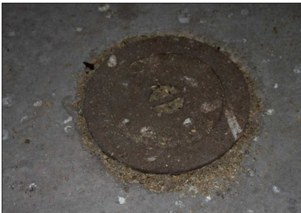
Plate 17: Cover for aperture in ground floor
