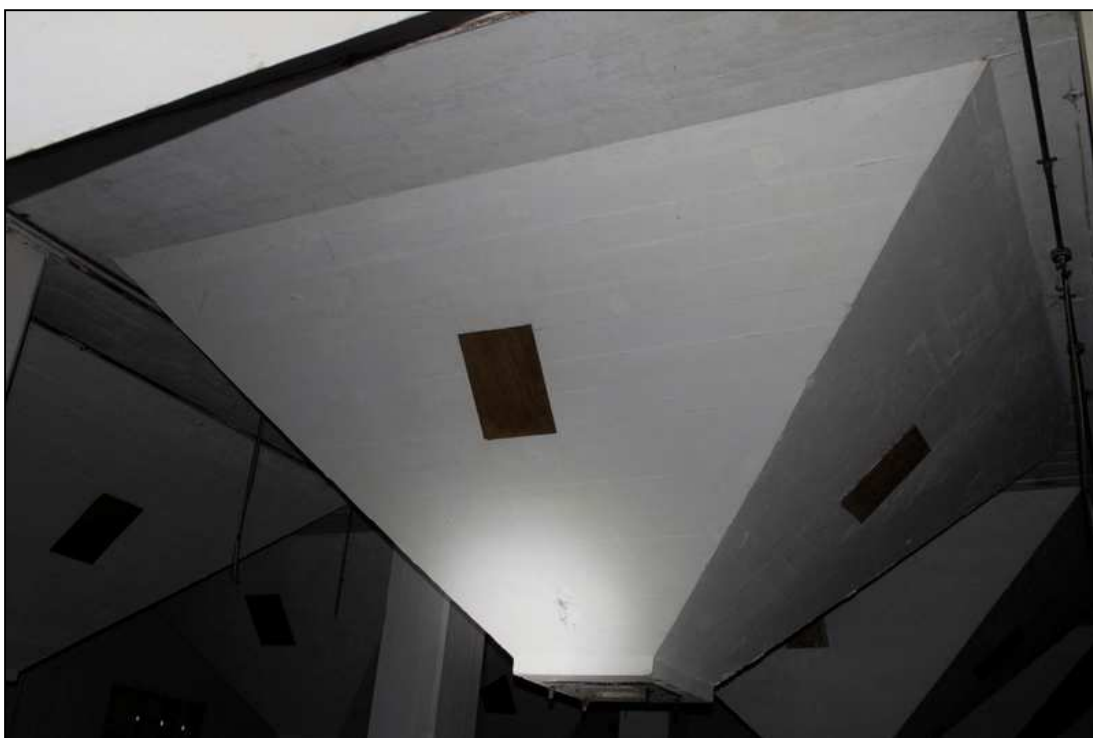
Plate 18: Detail of base of grain silo
