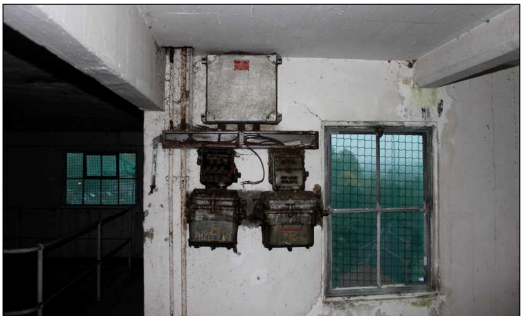
Plate 22: Fuse array in stair tower
