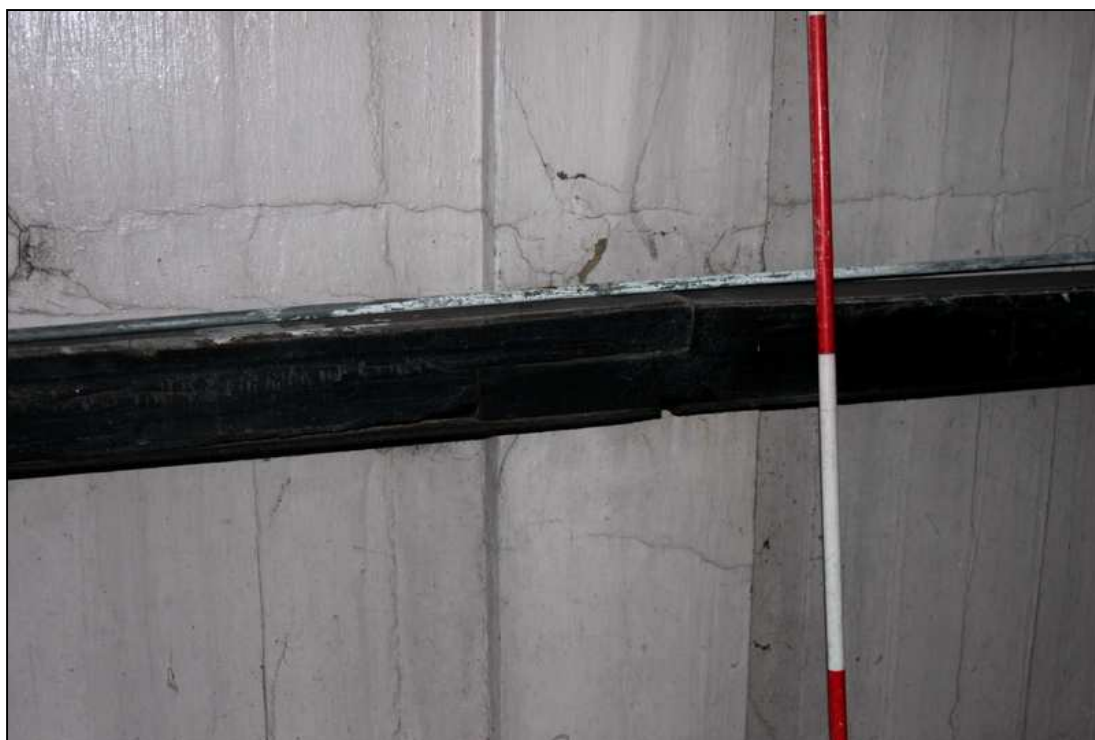
Plate 6: Detail of scarf joint in loading bay fender
