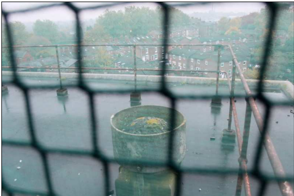
Plate 26: Vent cowl and guard rail on flat roof
