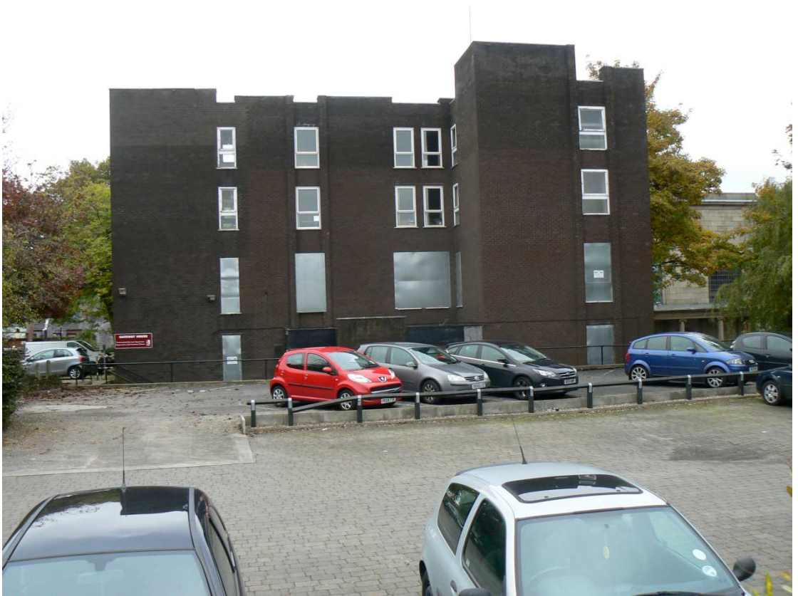
Plate 3: Municipal offices and car parking area forming the western part of the study area, occupying the site of Notre Dame Convent
