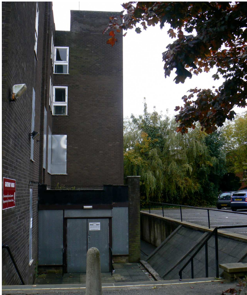
Plate 4: The ground-floor level of the municipal offices
