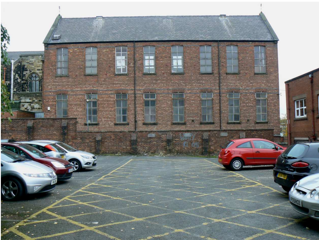
Plate 7: Car-parking area to the east of Worsley Terrace
