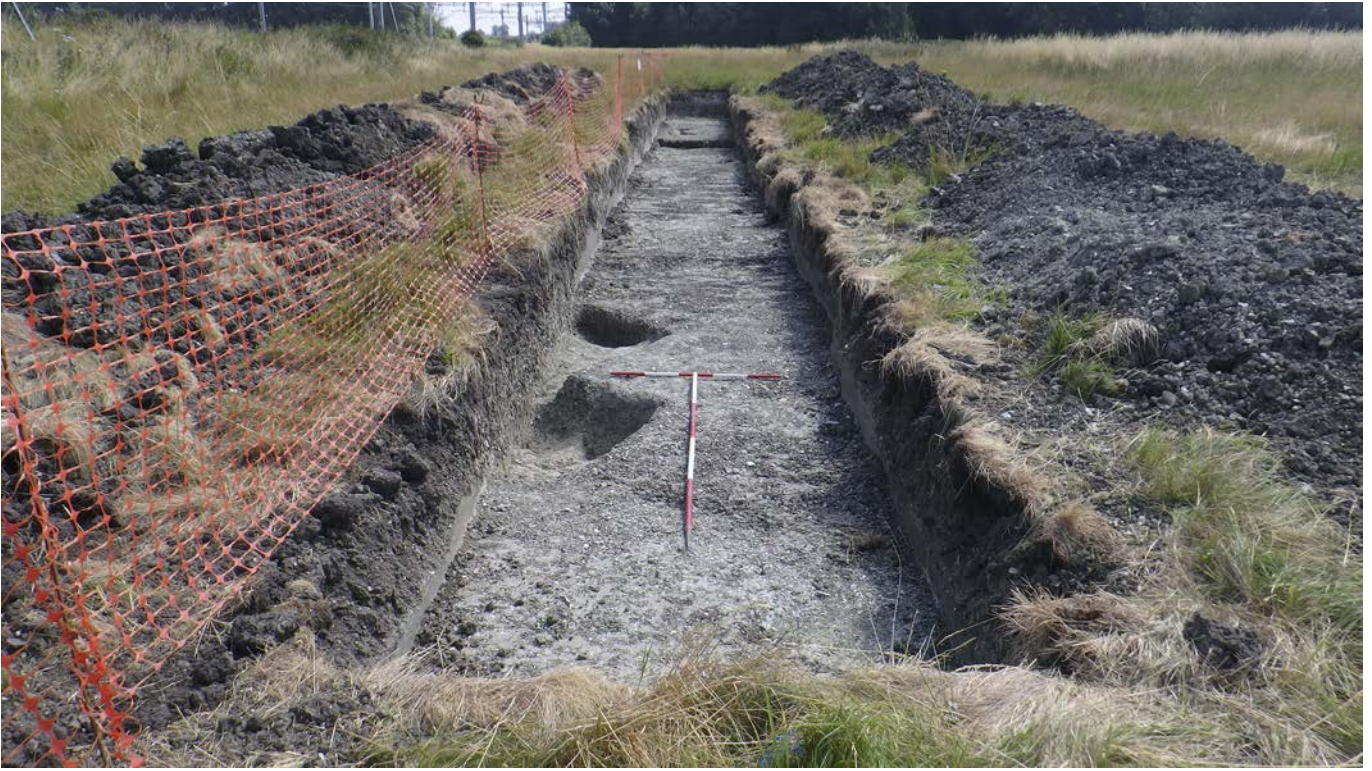
Plate 1: Trench 1 general shot
