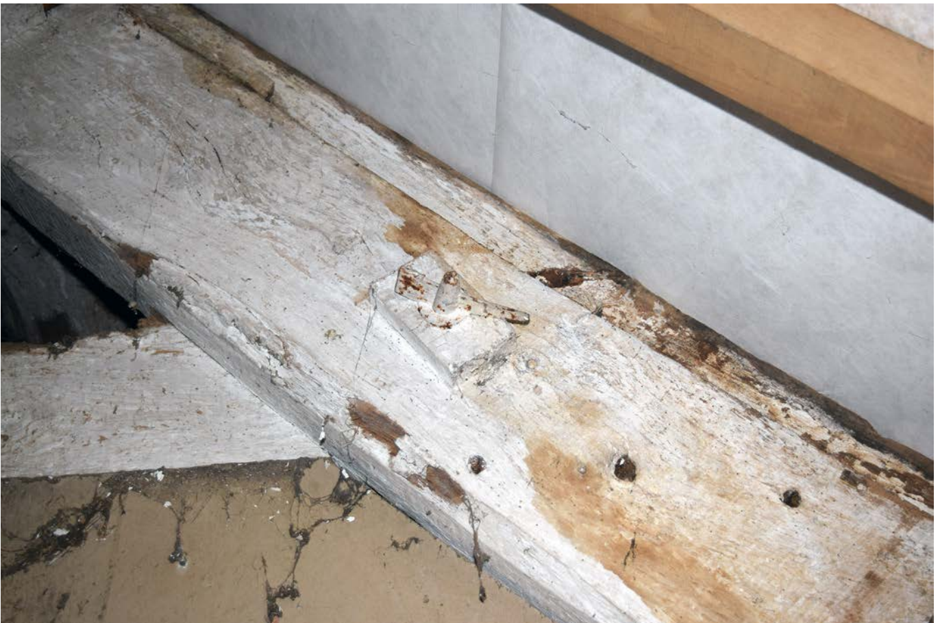
Plate 25: Detail of truss in the attic space of Jobsgreen farmhouse, showing forelock, looking west
