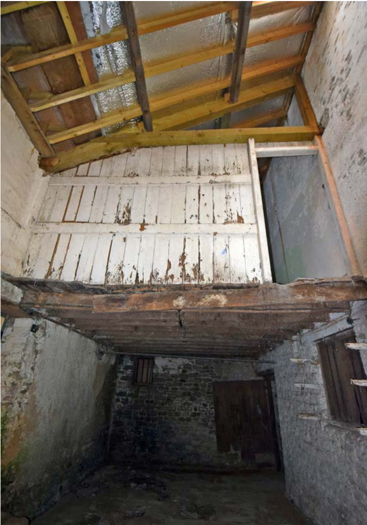
Plate 54: The interior of the central lean-to, looking north
