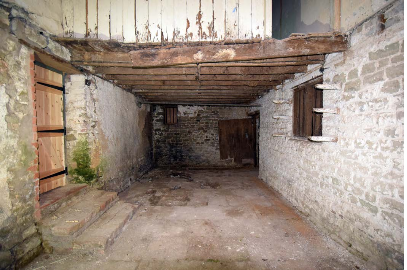
Plate 53: The interior of the central lean-to, looking north
