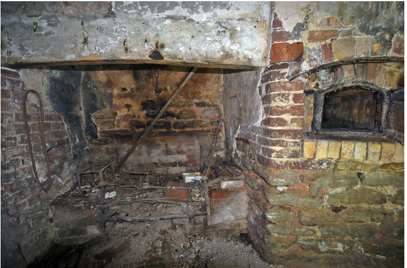
Plate 31: The back kitchen of the kitchen annexe, looking north
