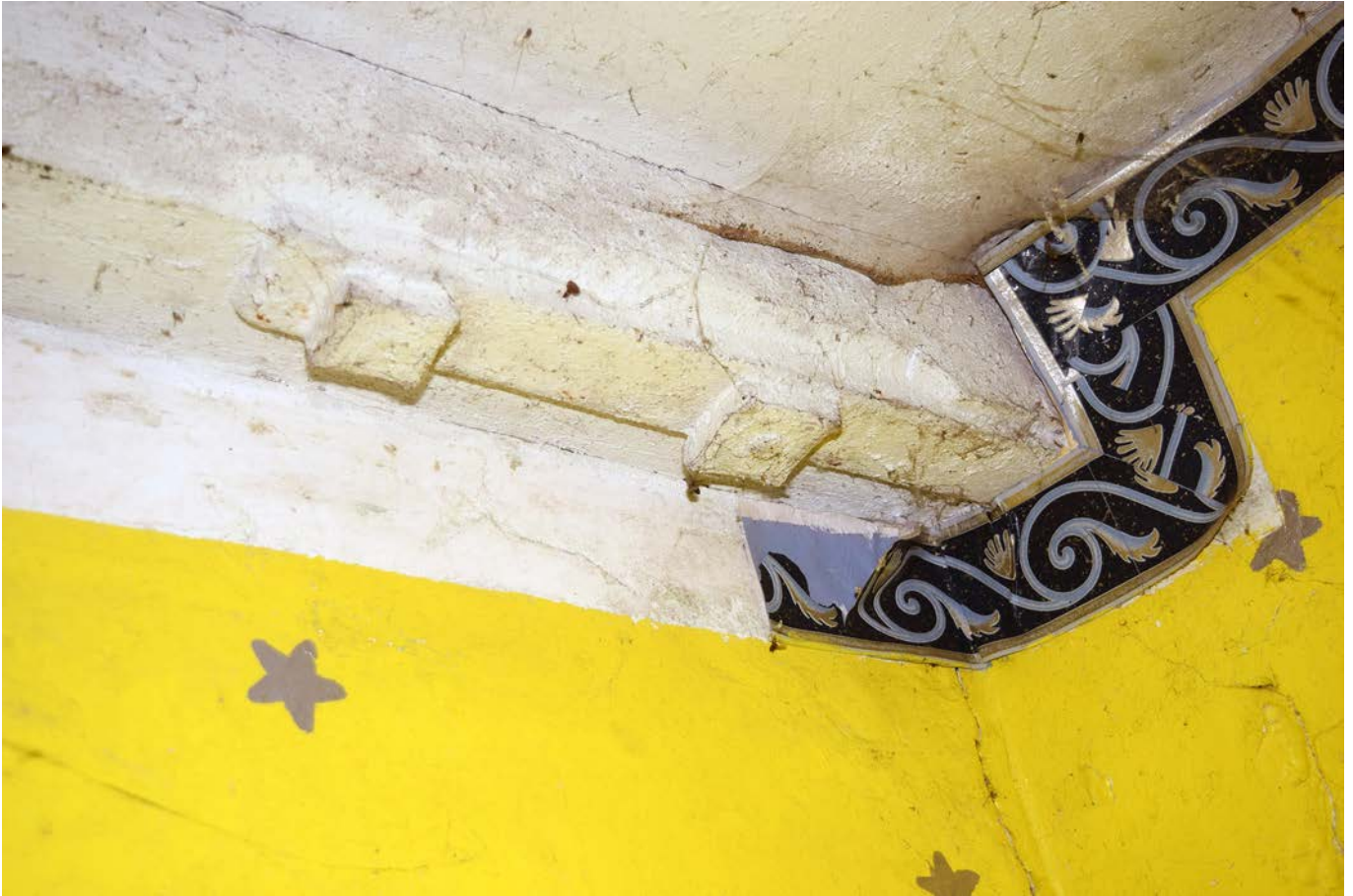
Plate 20: The chamfered beam in the ceiling of the central bedroom in Jobsgreen farmhouse, looking south-east
