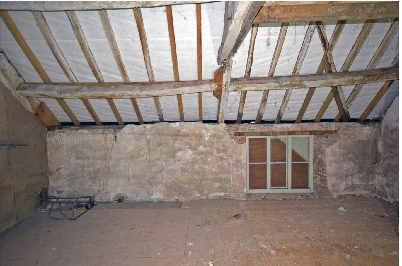
Plate 34: The first floor north room in the kitchen annexe, looking west
