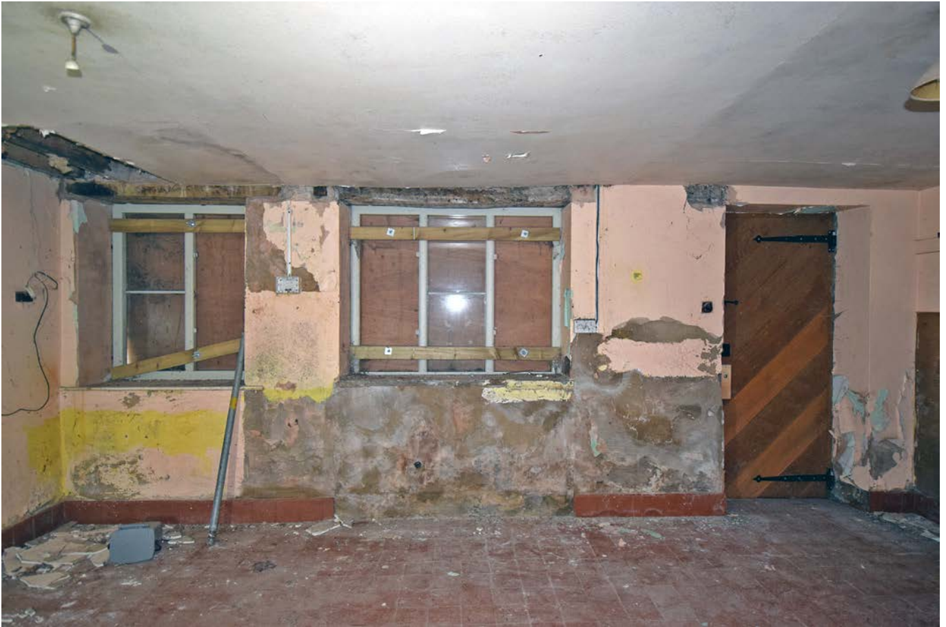
Plate 30: The ground floor of the kitchen annexe, looking west
