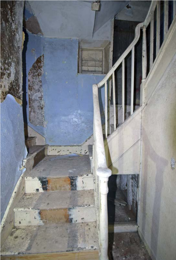
Plate 8: The staircase from the ground floor of Jobsgreen Farmhouse, looking north
