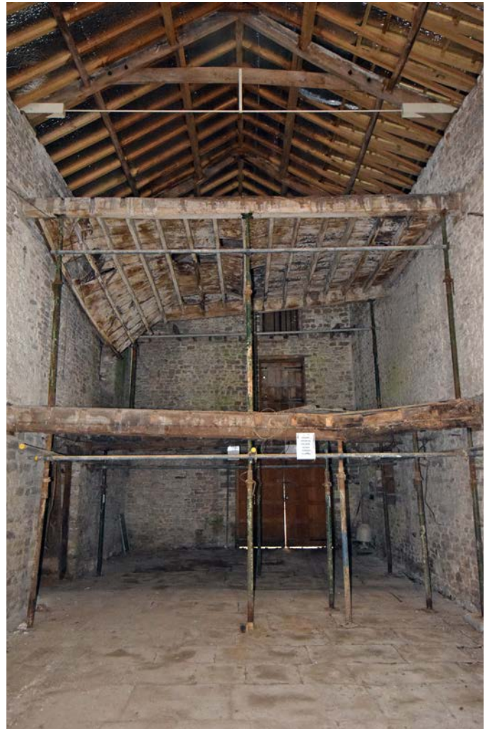
Plate 40: The interior of the central barn, looking north
