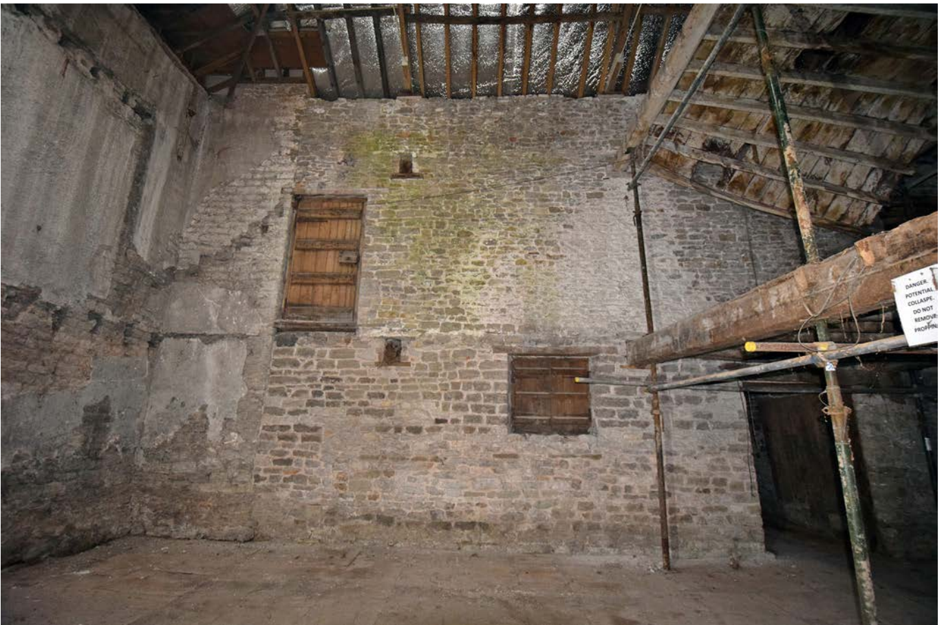
Plate 37: The interior of the central barn, looking west
