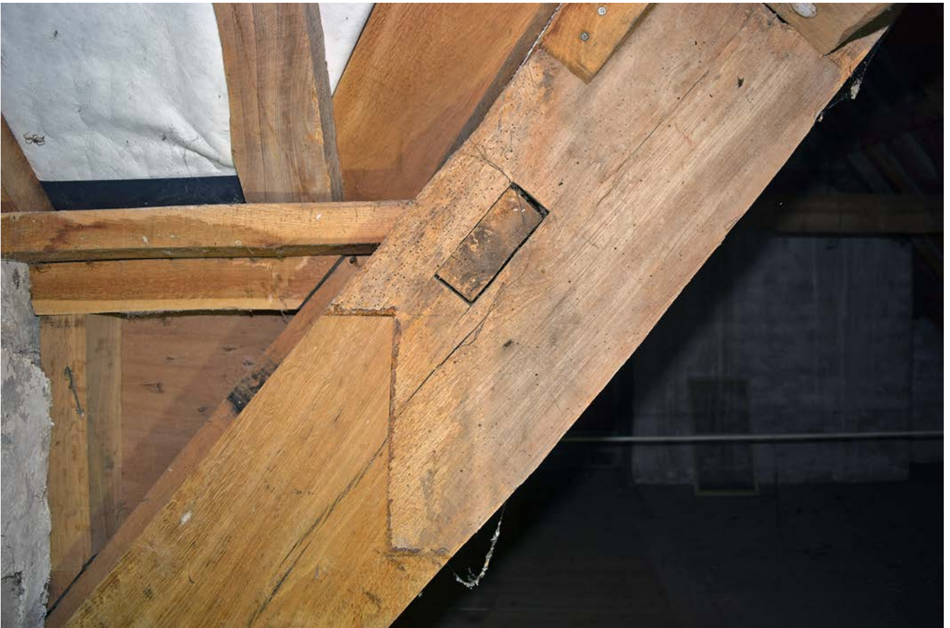
Plate 27: Modern timber repair in north principal rafter in the attic space of Jobsgreen farmhouse, looking east
