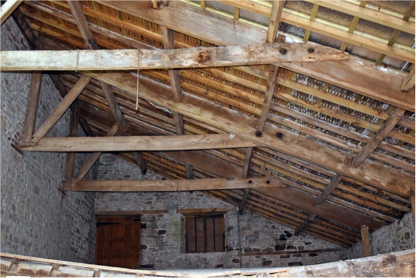
Plate 45: The interior loft space of the east lean-to, looking north
