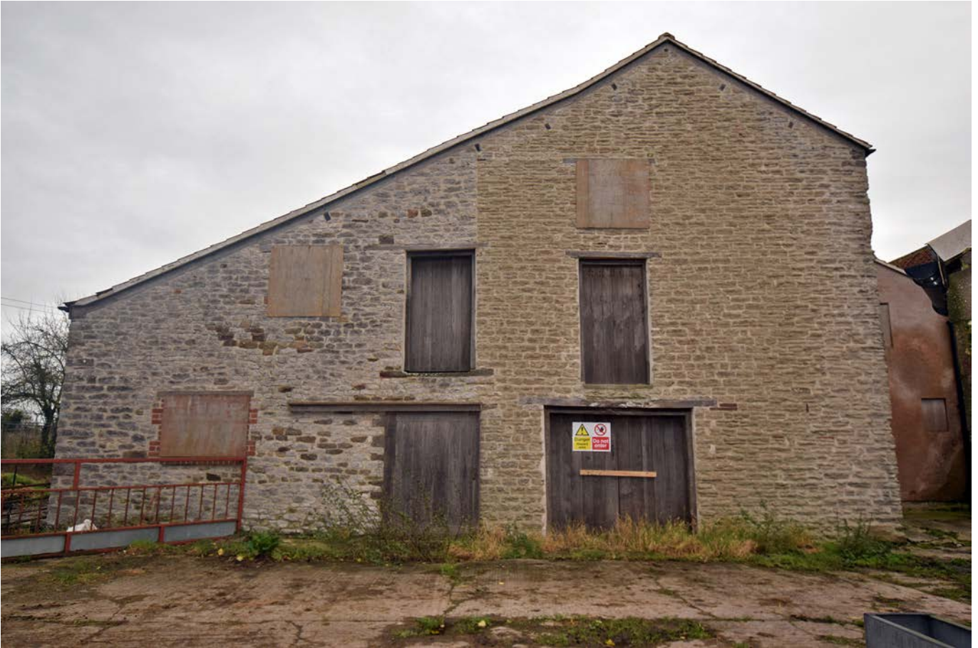
Plate 36: The north elevations of the central barn (right) and the east lean-to (left), looking south
