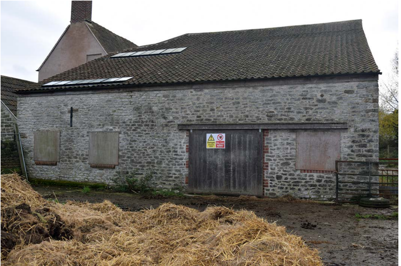
Plate 43: The east elevation of the east lean-to, looking west
