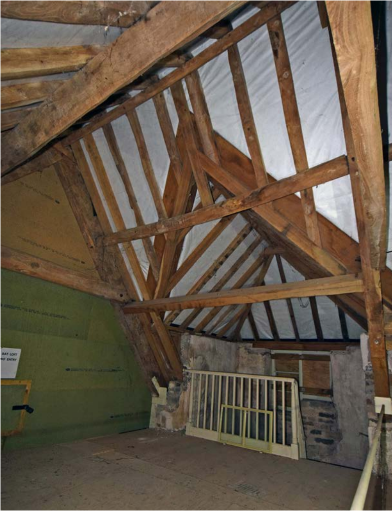
Plate 28: The north stair turret from the attic space of Jobsgreen farmhouse, looking north-west
