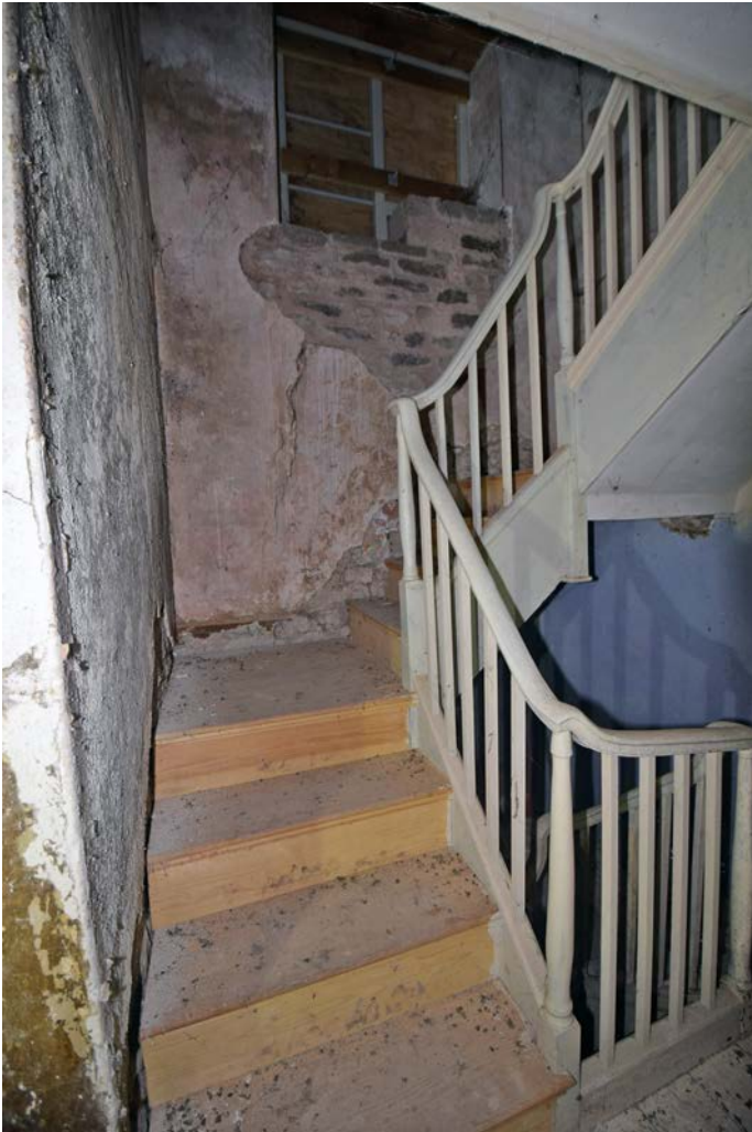
Plate 21: The staircase of the first floor of Jobsgreen farmhouse, looking north-east
