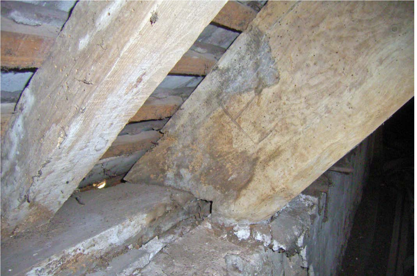
Plate 24: Foot of a south principal rafter in the attic space of Jobsgreen farmhouse, looking west
