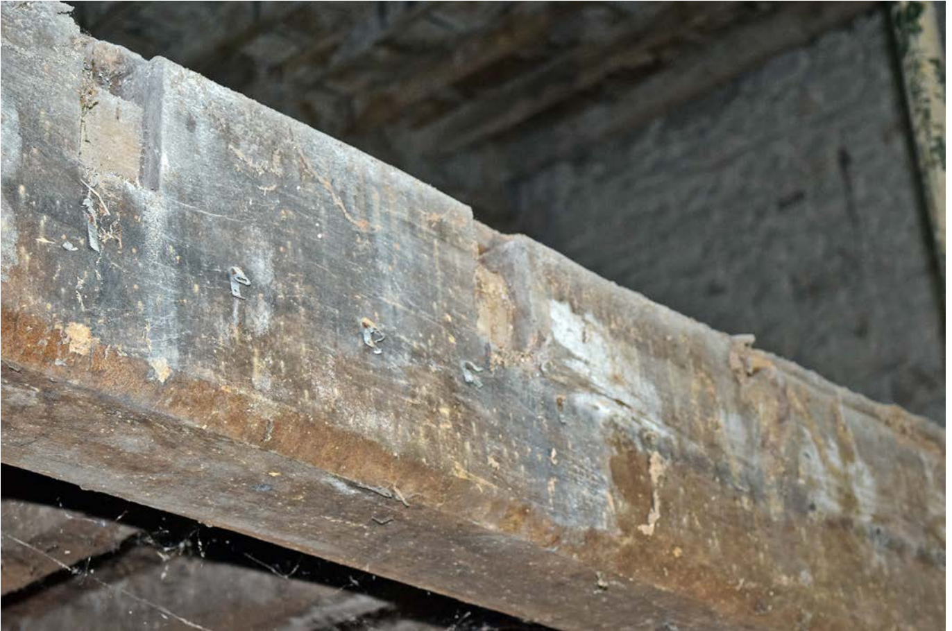
Plate 41: Detail of joinery in the floor structure of the central barn, looking north-east
