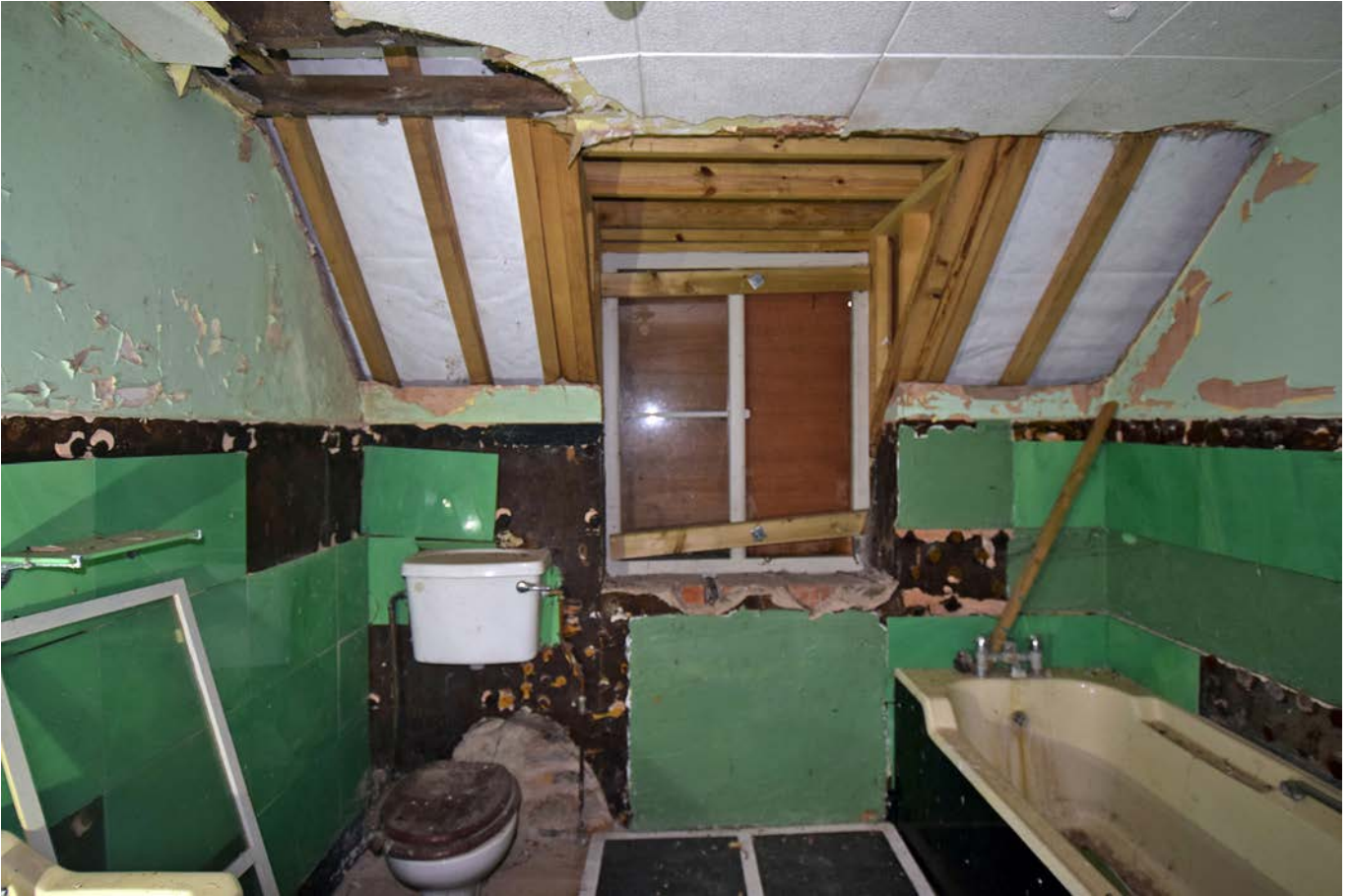
Plate 32: The first floor bathroom in the kitchen annex, looking west
