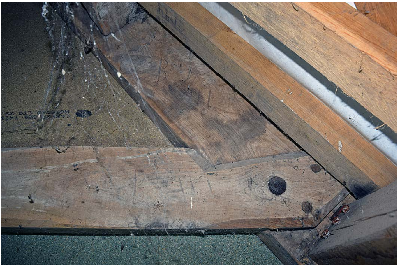
Plate 23: The east face of the third truss from the west in the attic space of Jobsgreen farmhouse, looking west
