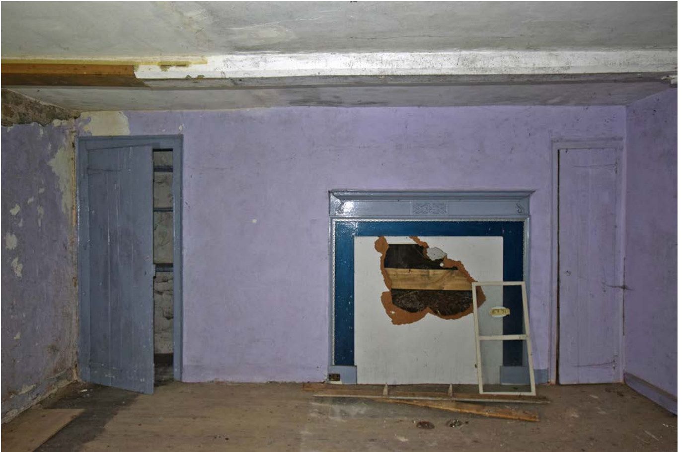
Plate 18: The east bedroom of Jobsgreen farmhouse, looking east
