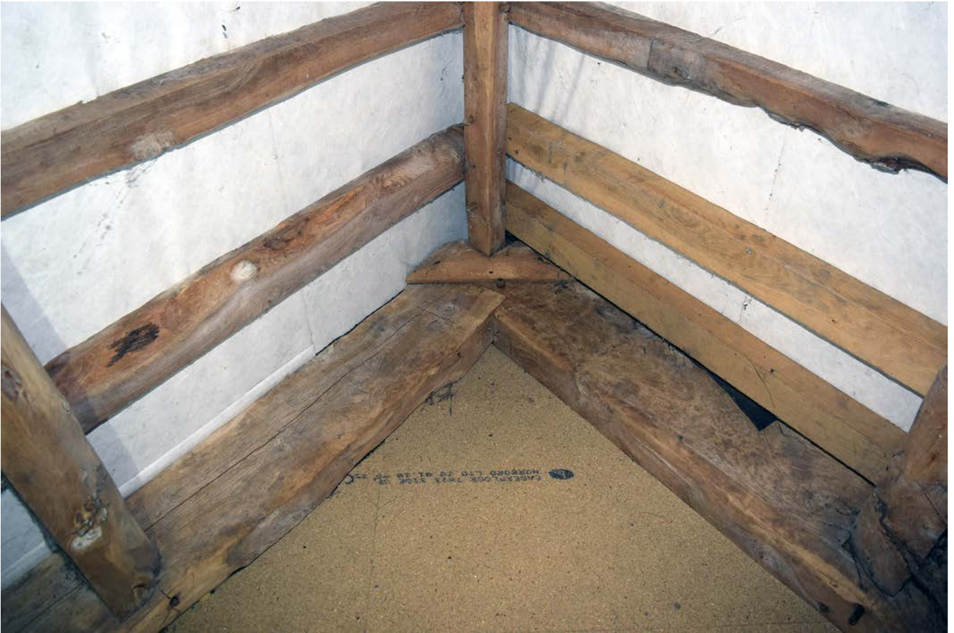
Plate 26: Detail of truss in the attic space of Jobsgreen farmhouse, showing apex and ridge piece, looking west
