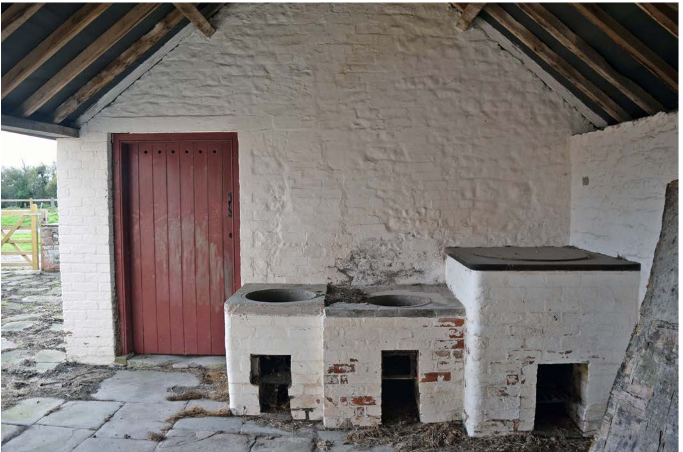
Plate 50: The interior of the east room of the dairy, looking west
