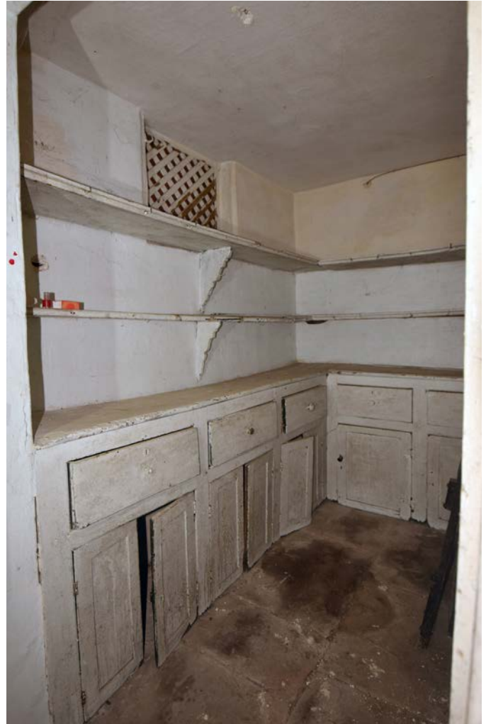
Plate 7: The store room on the ground floor of Jobsgreen Farmhouse, looking north-east
