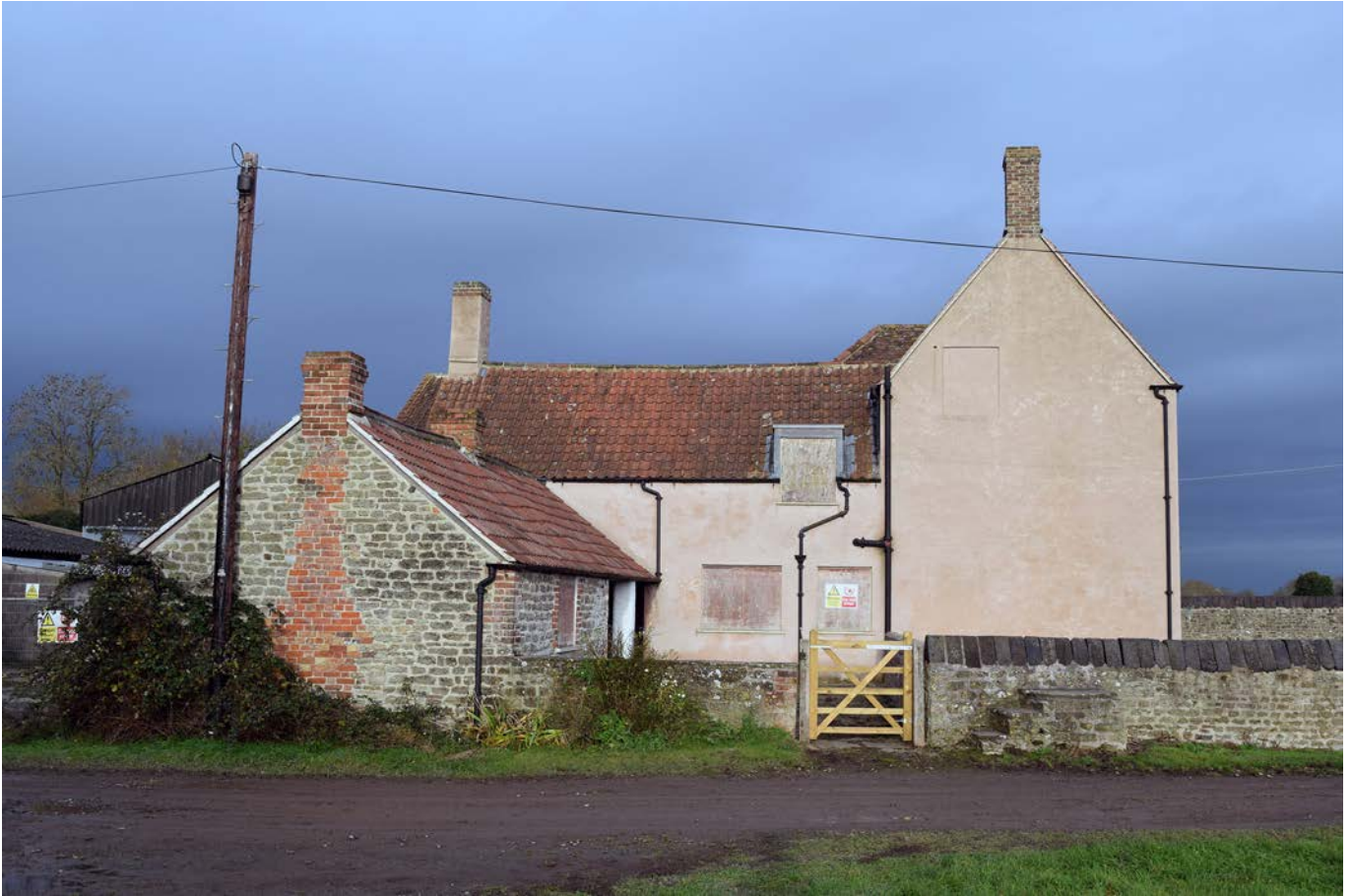
Plate 3: Jobsgreen Farm from the west
