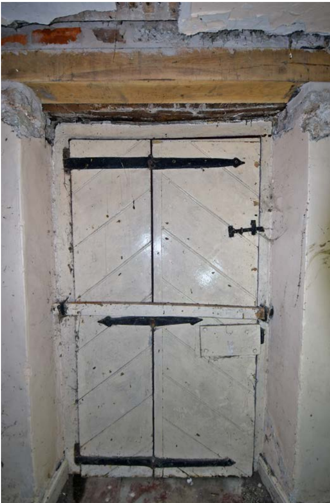
Plate 6: The interior of the front door of Jobsgreen Farmhouse, looking south
