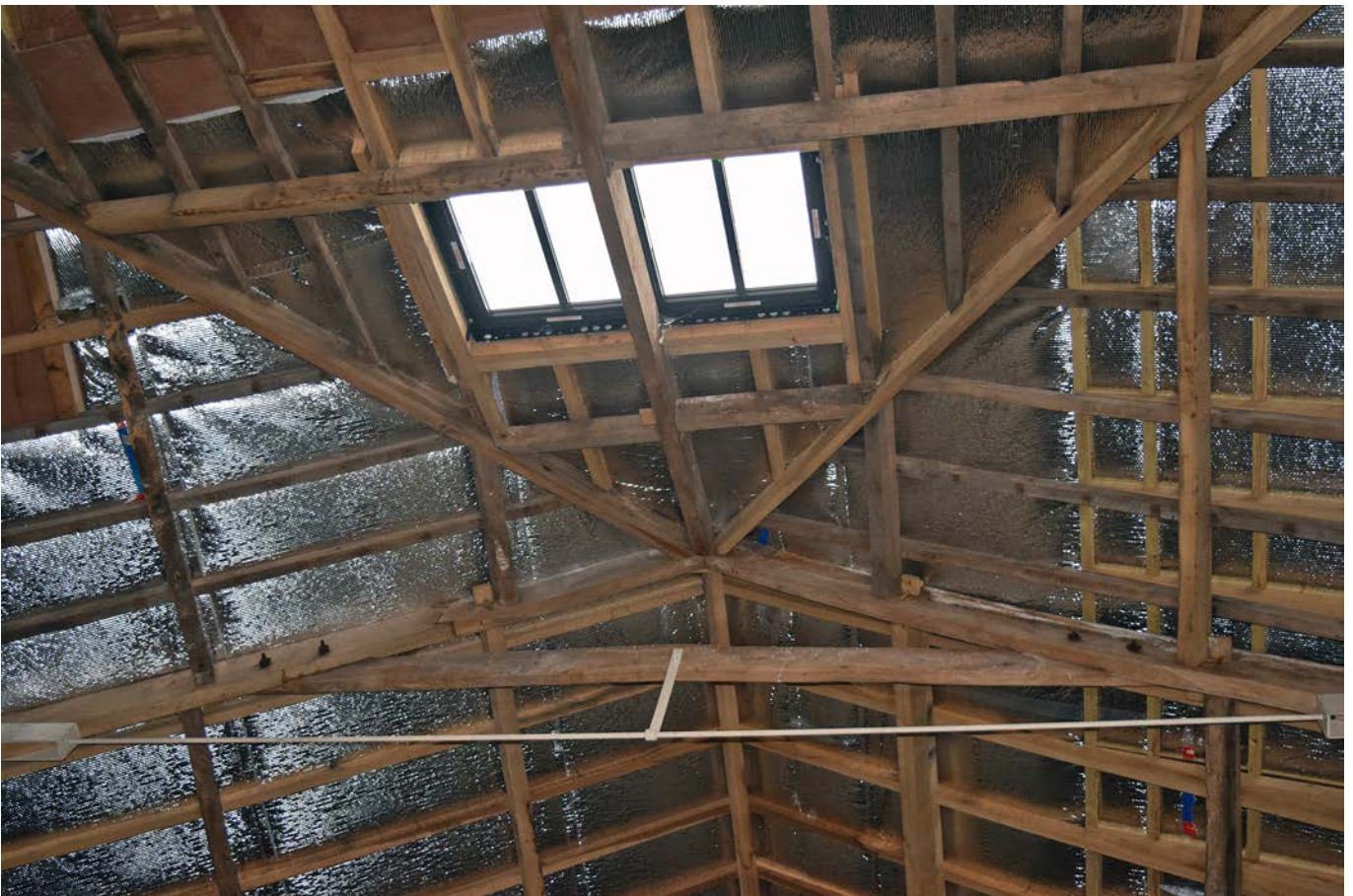
Plate 42: The roof structure of the central barn
