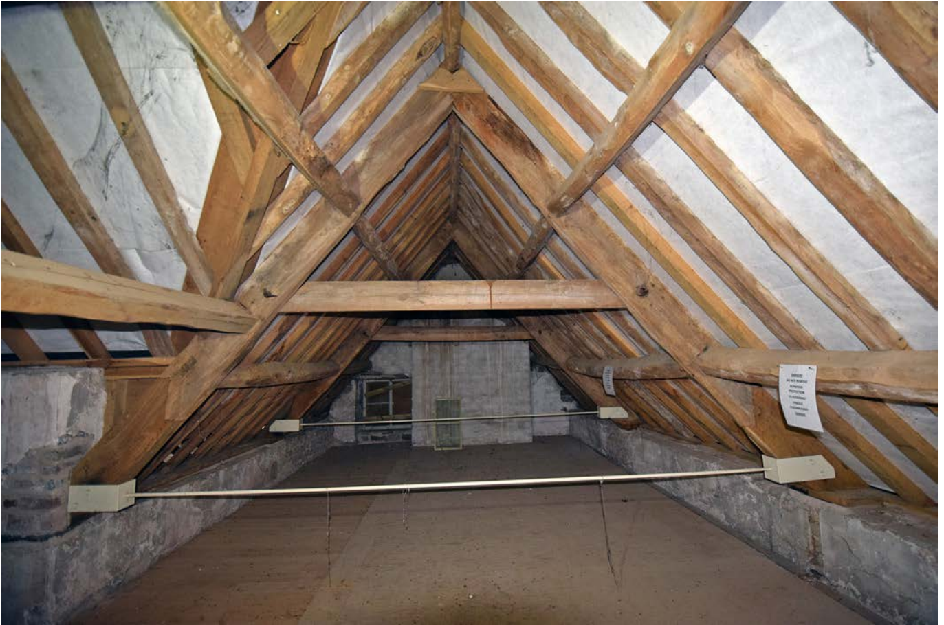
Plate 22: The attic space of Jobsgreen farmhouse, looking east
