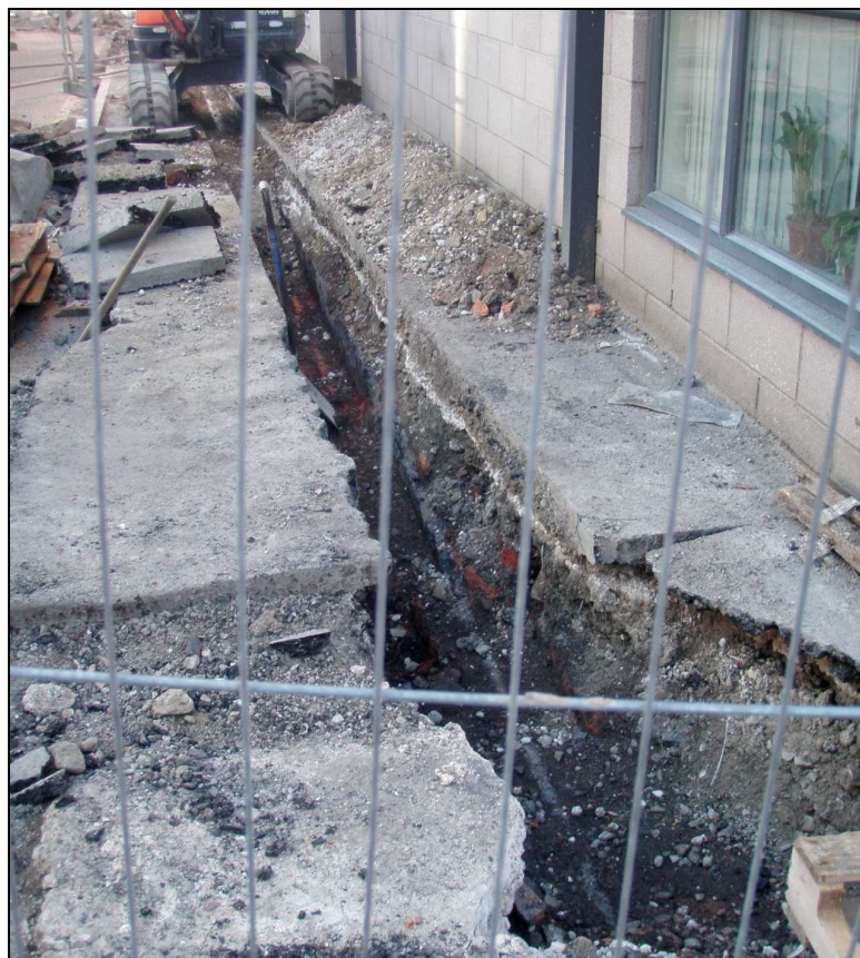
Plate 4: Exposed services along Style Street, looking south-west
