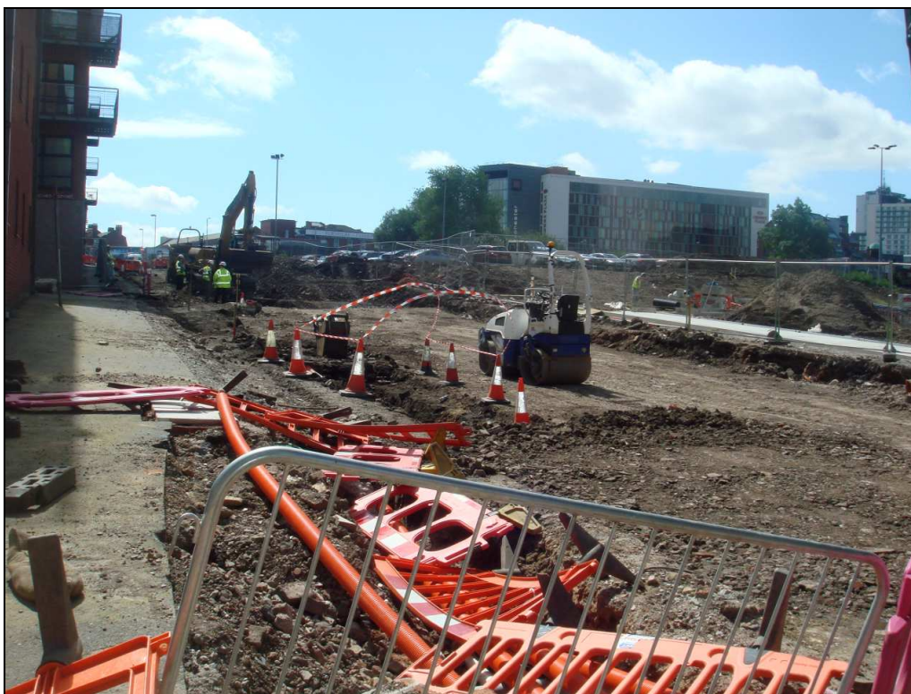
Plate 2: Depth of excavation along Angel Street, looking south-east
