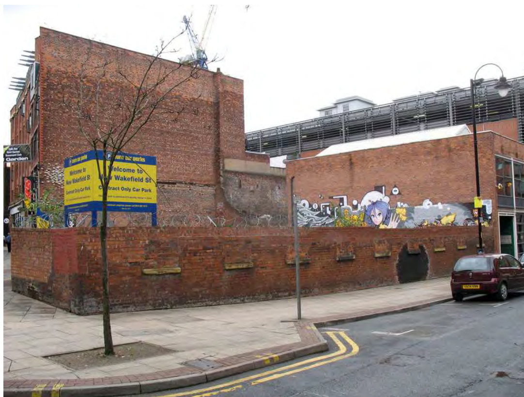
Plate 5: Walls on north-western corner of the car park within the proposed development area, looking east
