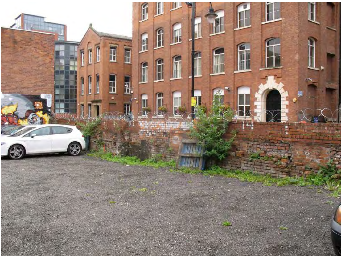
Plate 4: Western wall of car park at the northern extent of the proposed development area, looking south-west
