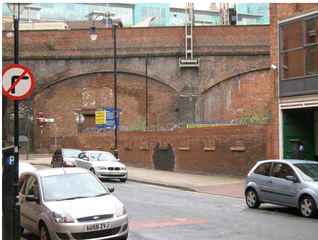
Plate 6: Western wall of the car park within the proposed development area, with the railway viaduct in the background, looking south
