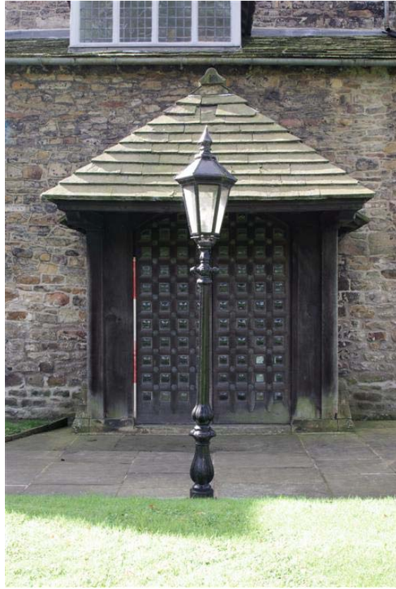
Plate 6: Exterior of north porch prior to works
