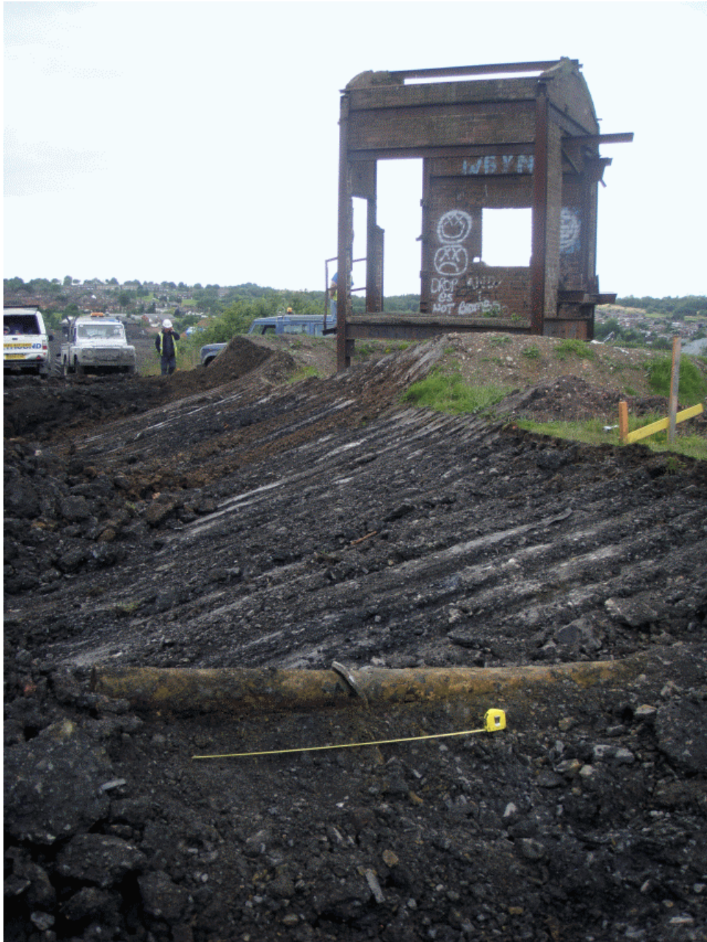
Plate 3: Cast iron slurry pipe exposed to the east of the dirt conveyor tower
