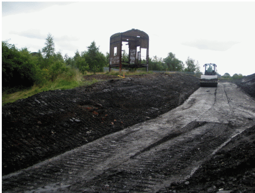
Plate 2: Footpath created alongside dirt conveyor tower
