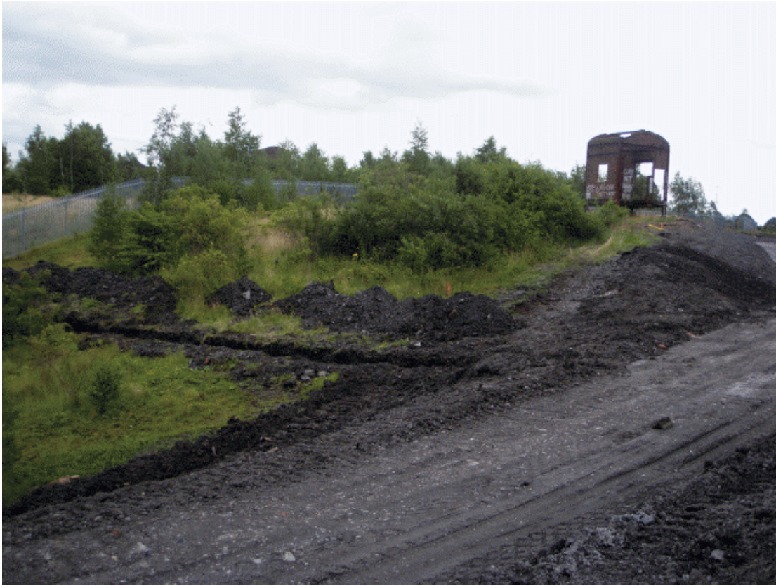
Plate 6: Service trench excavated to the south-west of dirt conveyor tower
