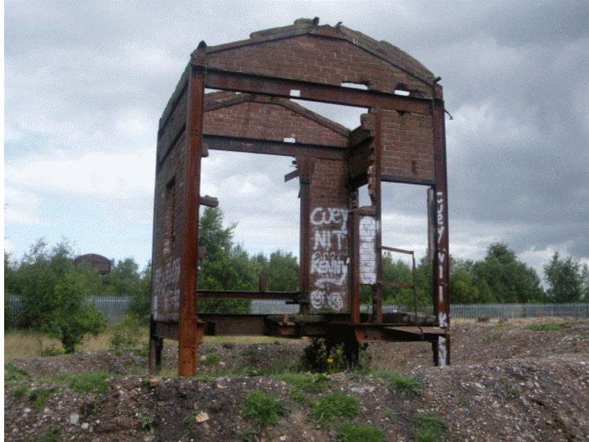
Plate 1: South-facing view of the dirt conveyor tower
